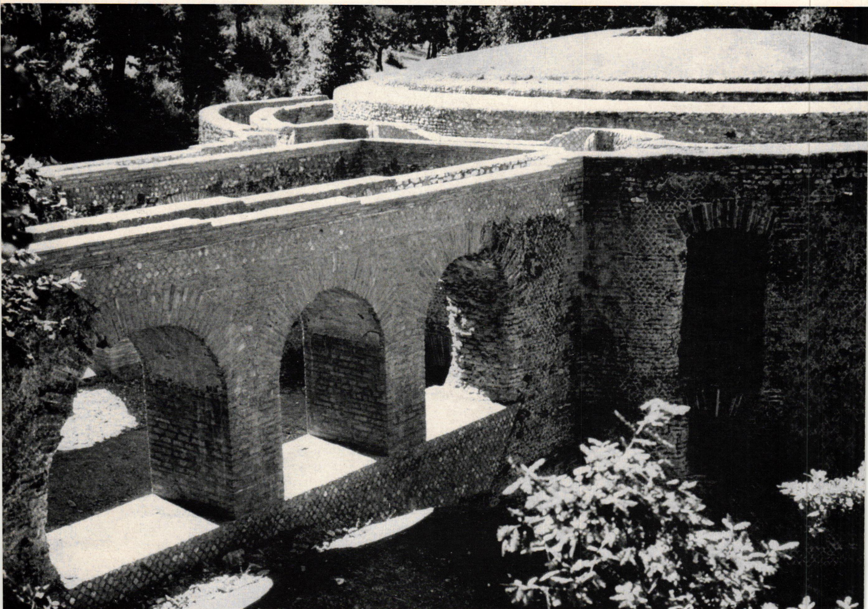
The Serapeion from the rear, showing the elevated water courses
