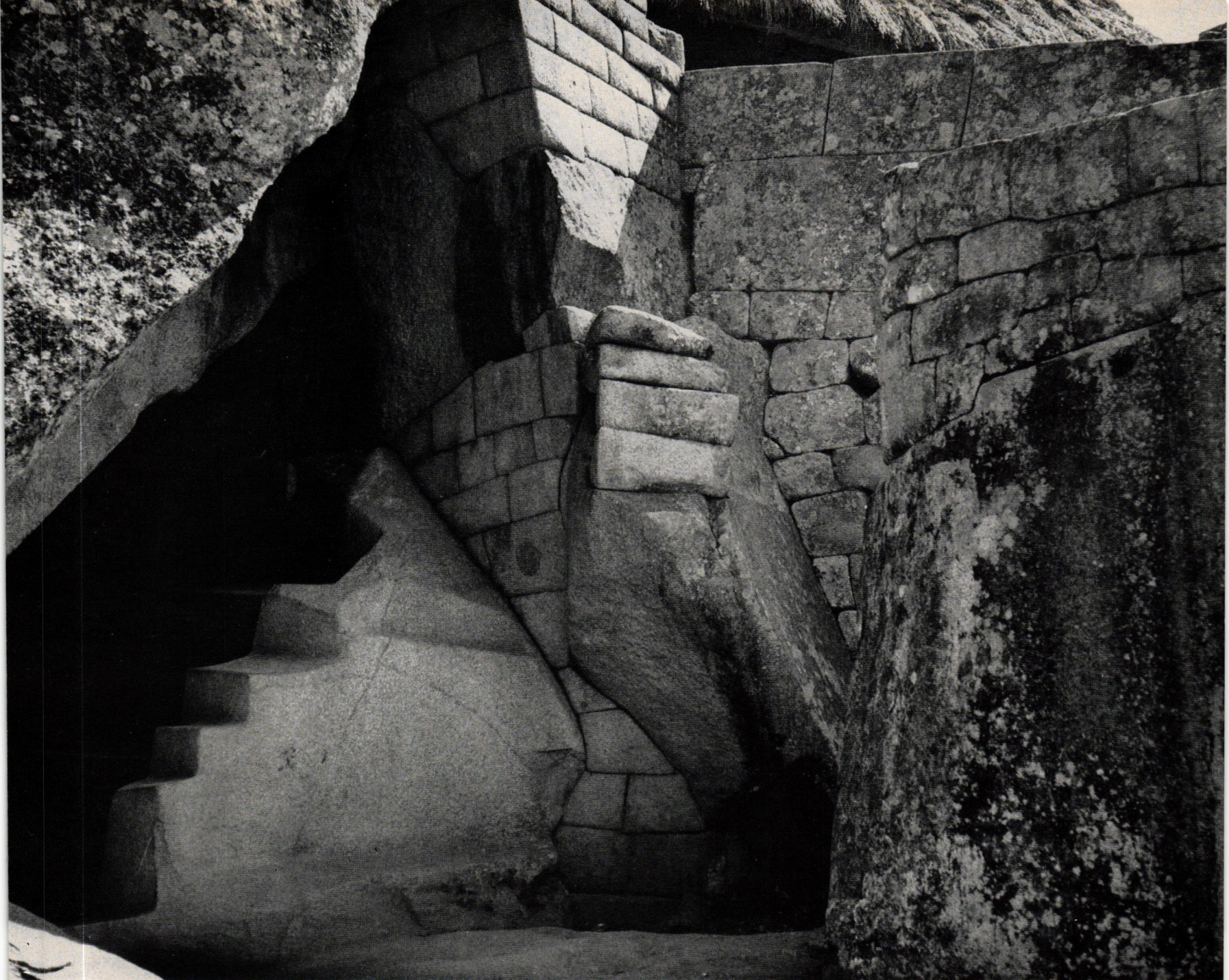
"Both methods of wall assembly — polygonal and rectangular — show extreme precision in the fitting of the stones."
