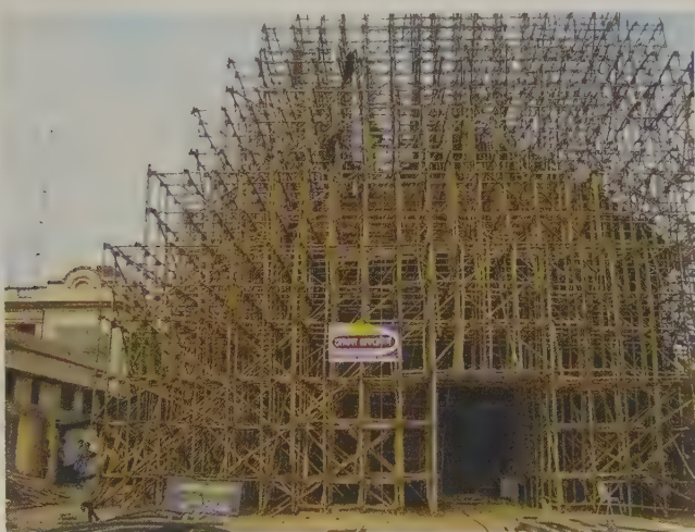
FIG 2 Mohammed Ali Park Puja pandal under construction, 2007.
