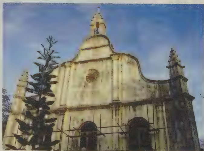
FIG 6 Facade of Saint Francis Church, Kochi.
