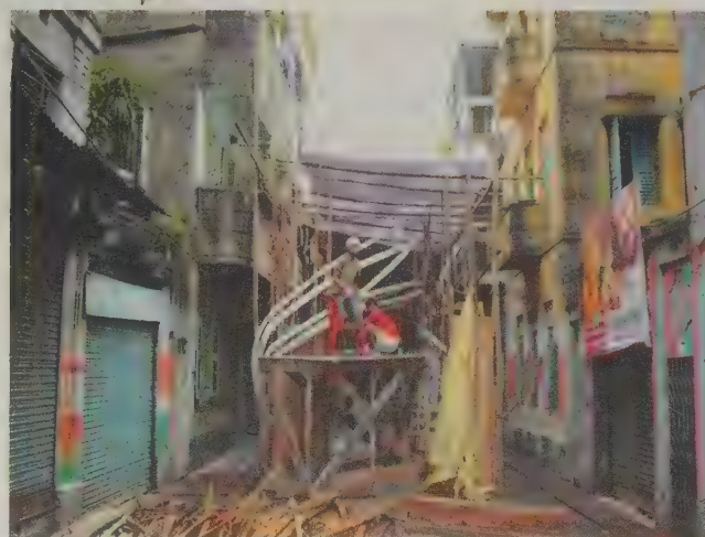
FIG 1 Puja pavilion construction, Nalin Sarkar Street, 2010.
