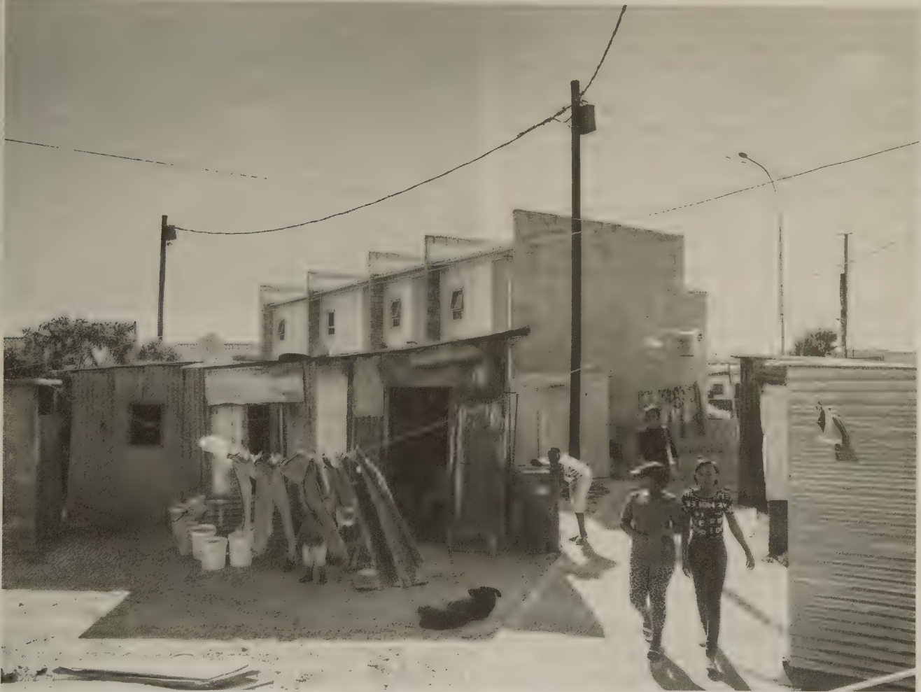
Rear view of the “BT South” Empower Shack pilot, was completed in December 2015. Courtesy of Jan Ras/U-TT. Fig 16.
