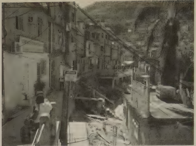
Precarious Cantagalo houses and pedestrian street
