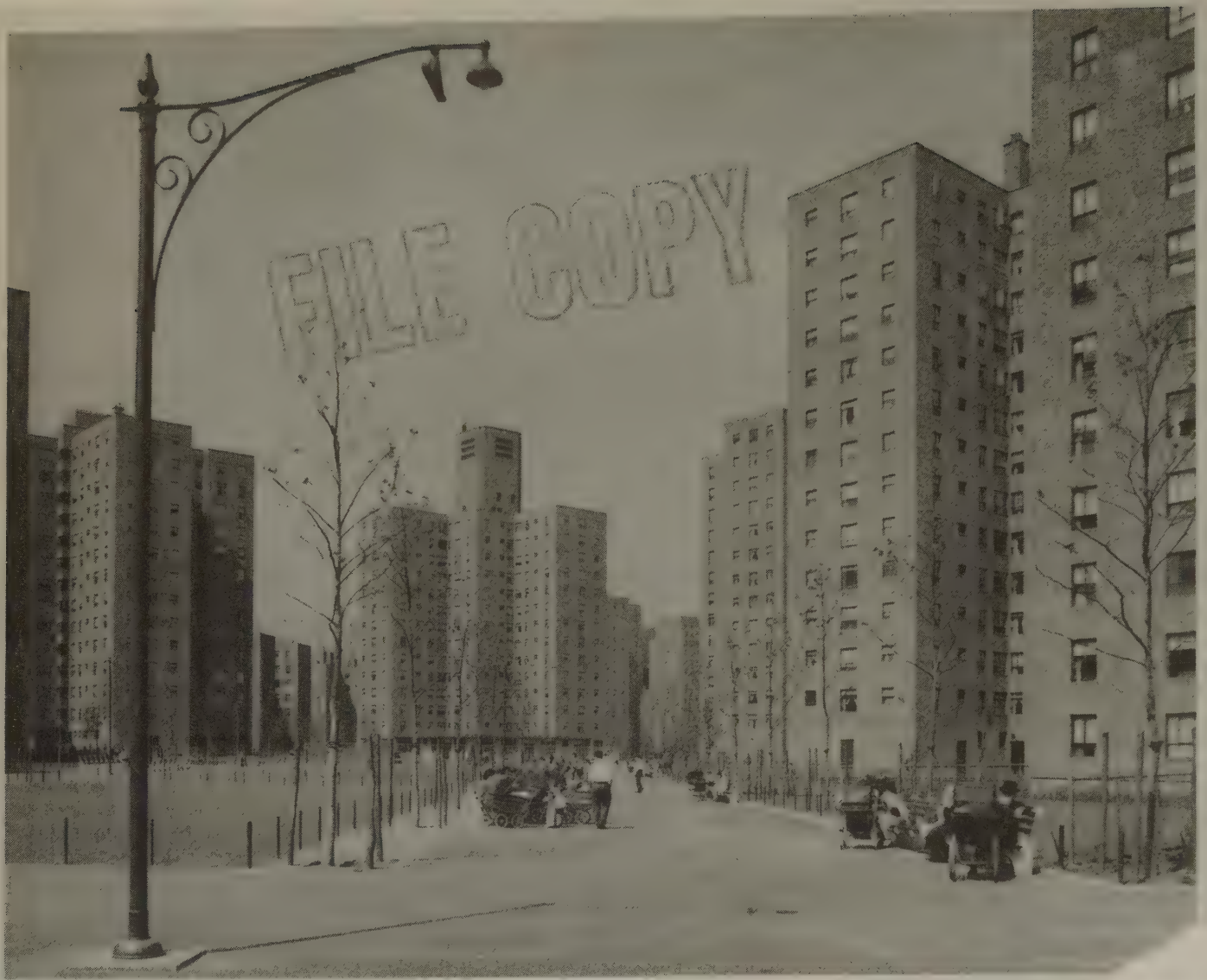
(Fig. 20) View of the Jacob Riis Houses. Photography courtesy of New York City Housing Authority.
