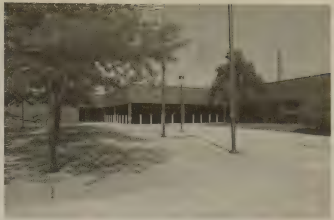
Fig 11. 24th District Police Station, Chicago, Illinois, 1977.
