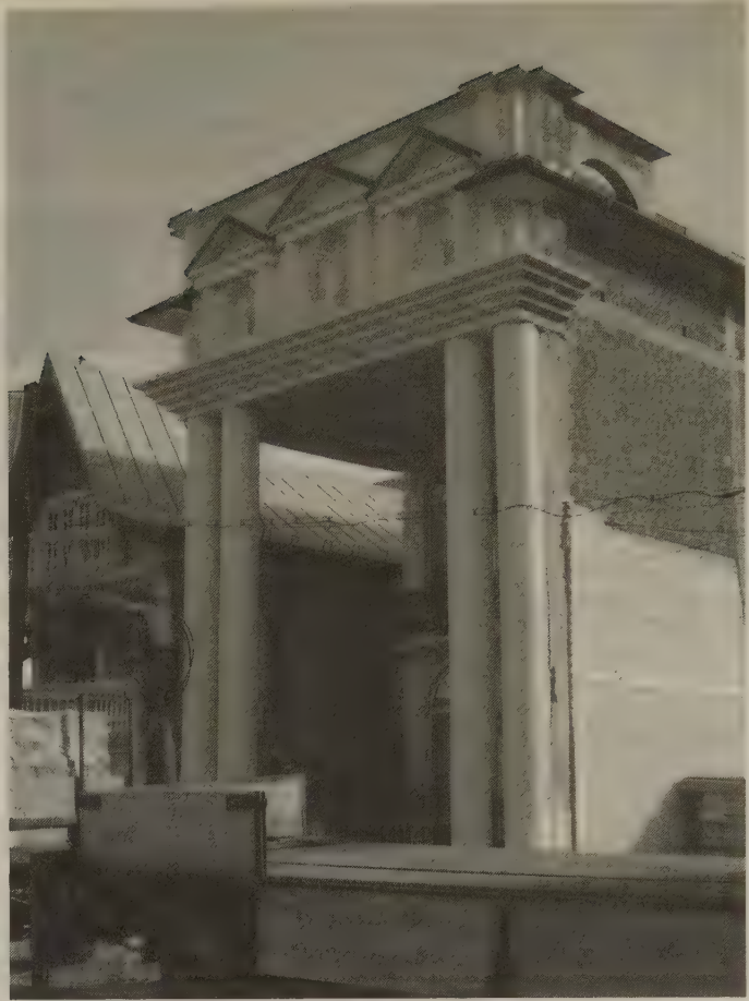
Gypsy mansion under construction on the main street in Buzescu, Teleorman County, Romania.
