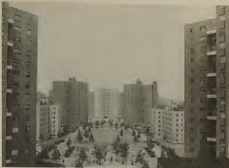
(Fig. 1) Kahn & Jacobs, Carver Houses, before Simon Breines and M. Paul Friedberg's design intervention. Photograph courtesy of the New York City Housing Authority.
