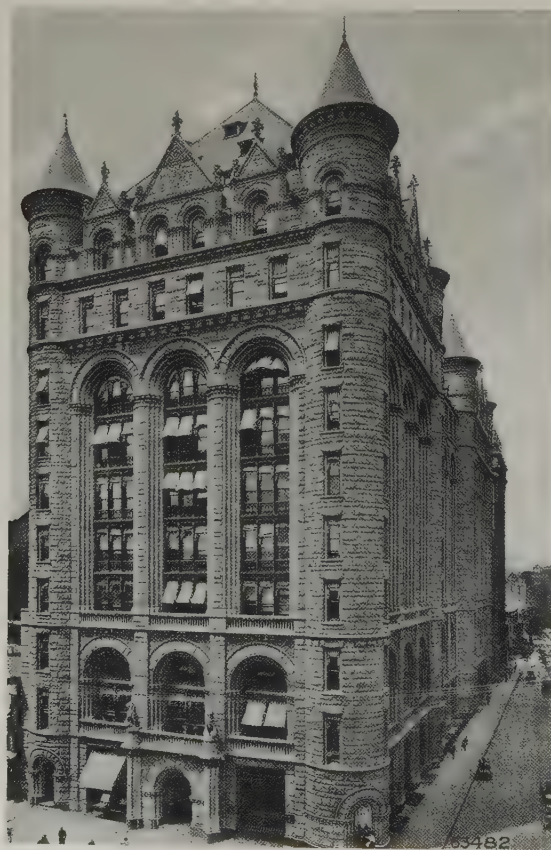
Fig. 5 The Prudential Building, Newark, 1892, George Post. It was destroyed in 1960 to make for a new headquarters structure in the same place
