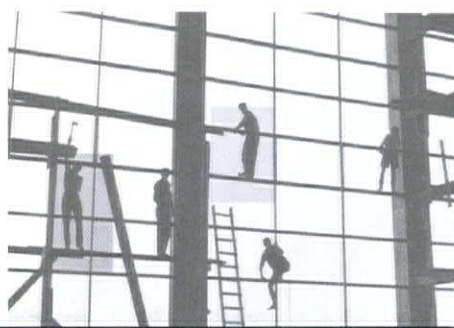
15 The Belgrade Fair under construction, 1957. Photograph by M. Pavlović. From Jugoslavija 15 (1958).
