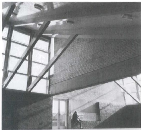
Photograph of the monumental small building: James Stirling and James Gowan, Brunswick Park Elementary School Extension , Camberwell. Photography by James Stirling with Eldred Evans.
