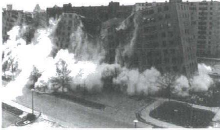
Minoru Yamasaki Pruitt-Igoe Housing , St. Louis, Missouri, 1952–55 (Demolished, 1972).
