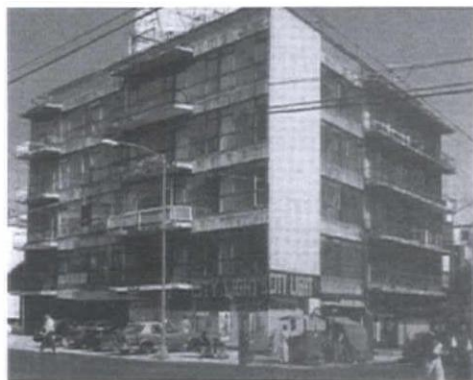
TEN Arquitectos, Arq. Enrique Norton, Hotel Habita, Mexico City, Col. Polonco, 2001. Existing abandoned apartment building on the site that was recycled.
