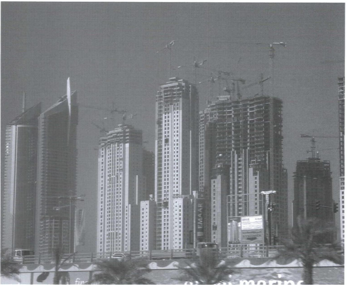
Construction site, Dubai.
