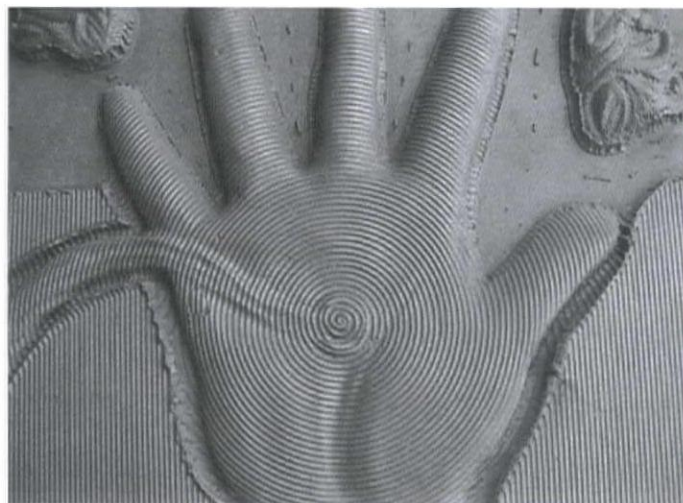
Doors of the Our Lady of Angels Cathedral, Los Angeles Left: bronze doors sculpted by Robert Graham Right: hand detail showing CNC milling path
