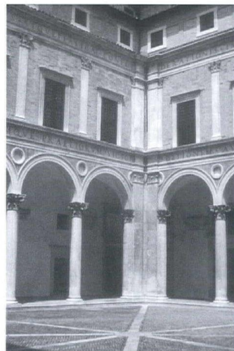
Fig. 5 Intersection of two columns at courtyard corner, Palazzo Ducale, Urbino, Luciano Laurana, 1450
