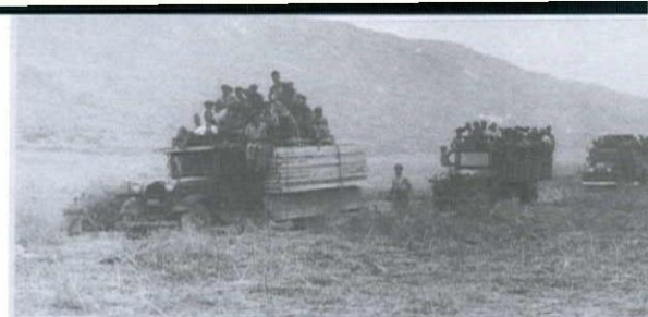
Trucks with building elements on their way to new settlement
