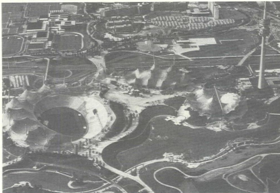
← Olympic Stadium, Munich 1972. Net wire, translucent acrylic sheeting, and tubular steel masts. Frei Otto and Günter Behnisch.
