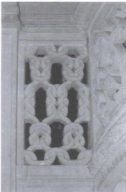
Top to bottom Interior of Sainte-Etienne Du Mont showing stone interlac- ing of the roodscreen, Paris, Philibert de l'Orme.
