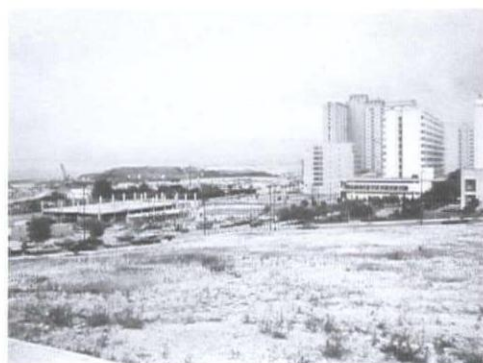
Above, middle, below Solidere redevelopment in central Beirut. Photograph by Michael Stanton.
