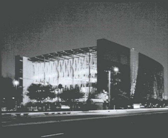
∧ Phoenix Central Library Phoenix, Arizona William P. Bruder, 1992.
