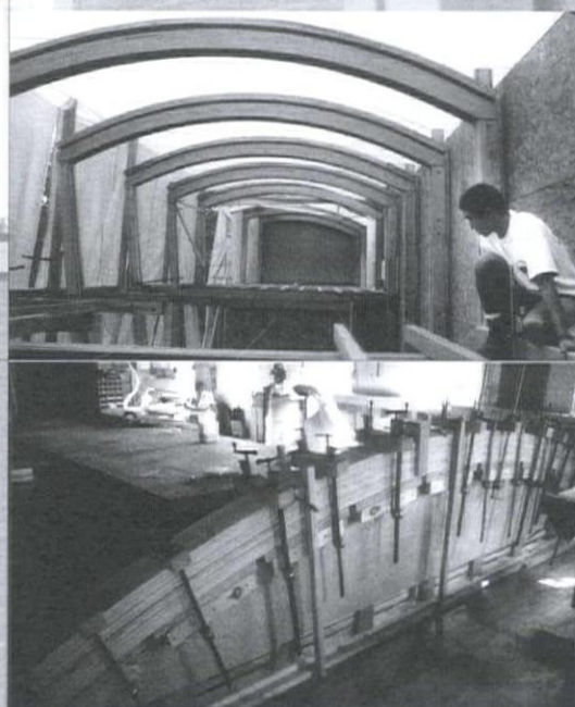
Construction of laminated beams and stressed skin panels Fabrication of laminated beam in Architect's workshop
