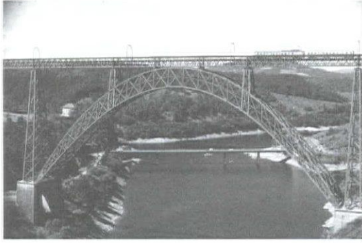
Garabit Viaduct over the Truyère, France, Gustave Eiffel (1884)
