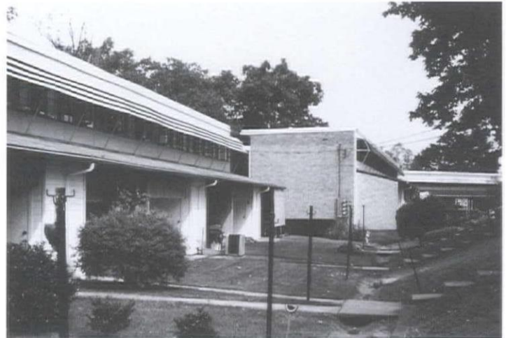
Row house terraces and walkways, 1998
