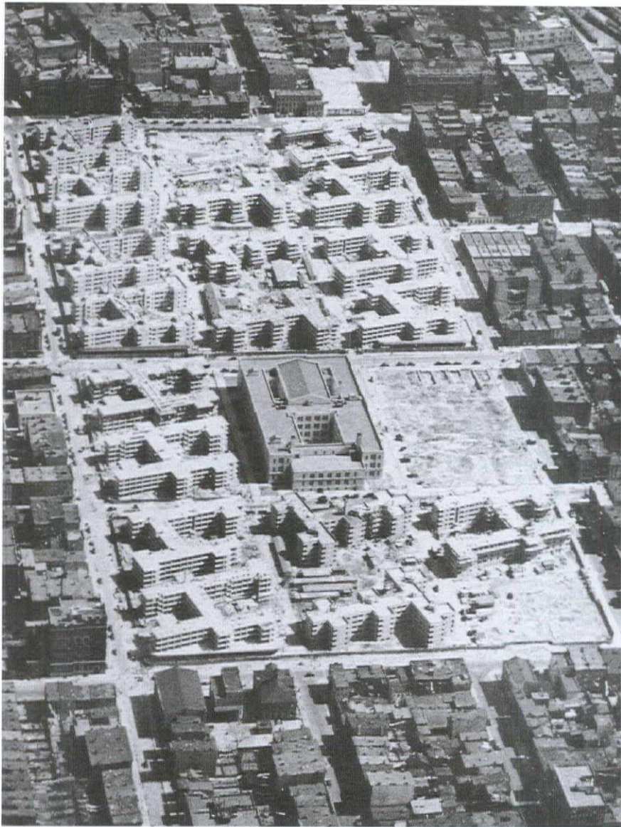
Williamsburg Houses under construction, 1937
