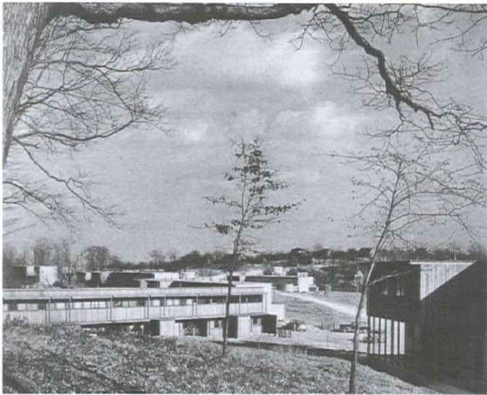
Terrace buildings from nearby hilltop, 1944
