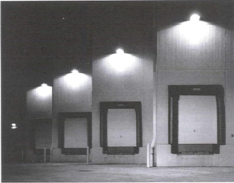
Loading dock, Newark, New Jersey, 1999. Jeffrey Sturges
