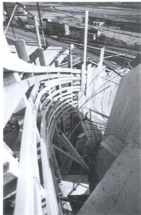
11 Church of Longarone, exterior spiral stair under construction.
