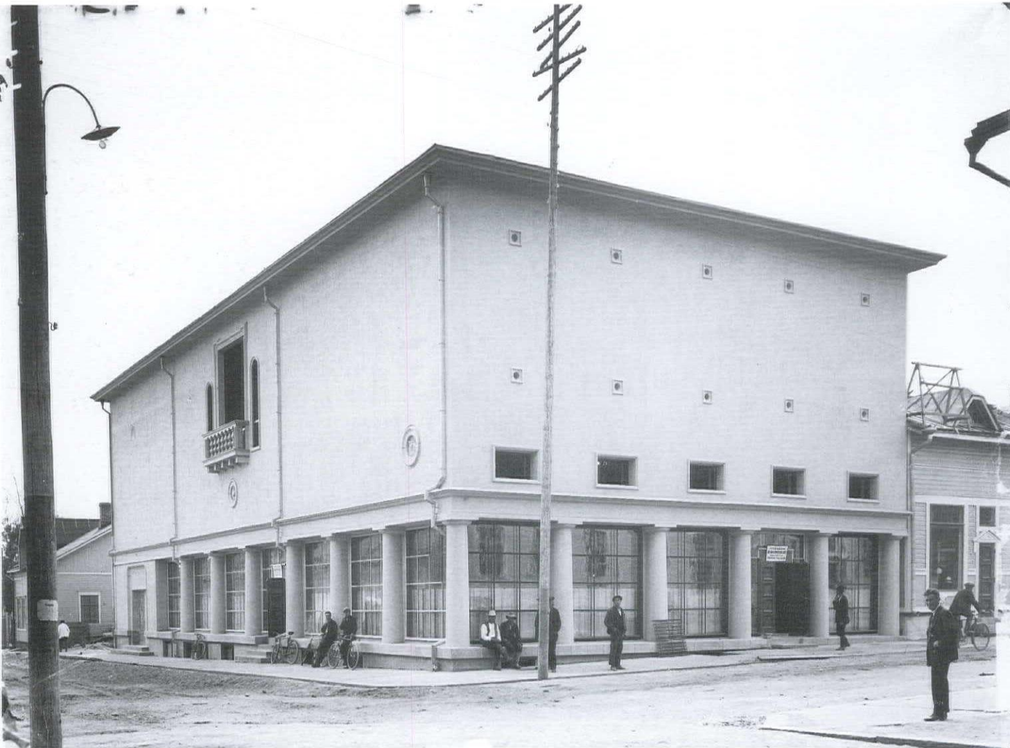
11 Workers' Club, corner view from Kauppakatu.
