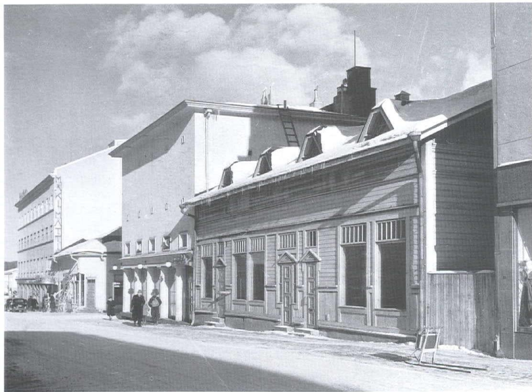
12 Workers' Club, view from Kauppakatu.
