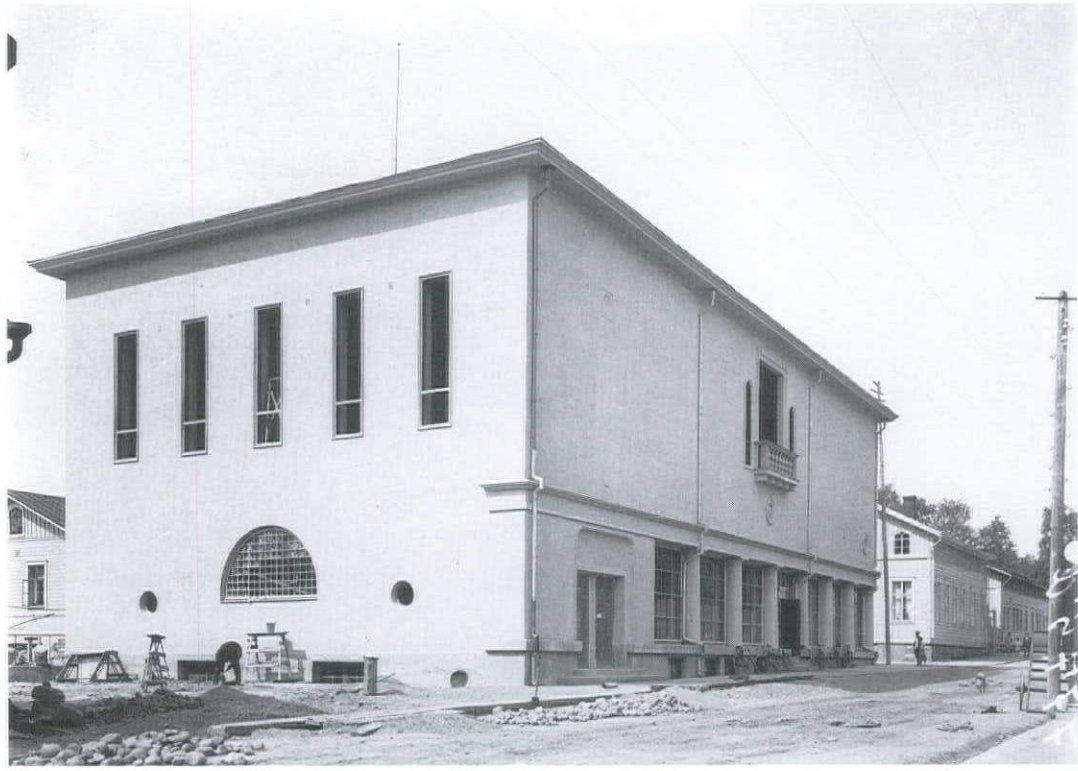
10 Workers' Club, corner view from Vainonkatu.
