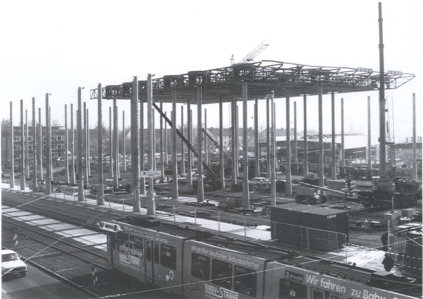
8 and 9 Construction of roof canopy.
