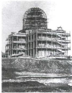
17b. Church Am Steinhof, construction photograph.
