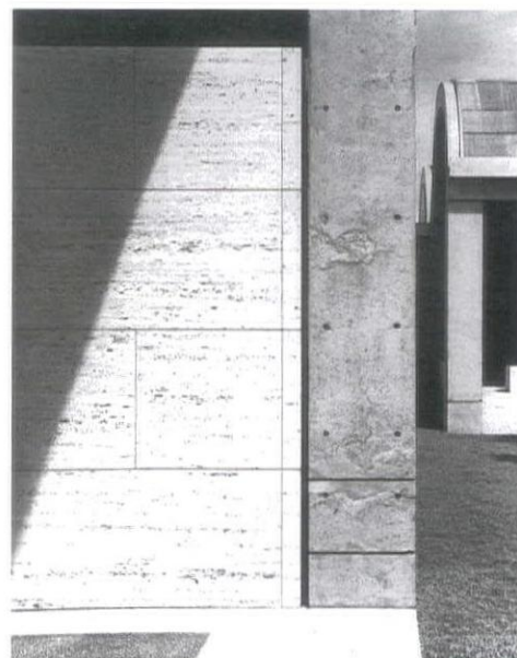
15. Kimbell Museum of Art, detail of travertine and concrete.
