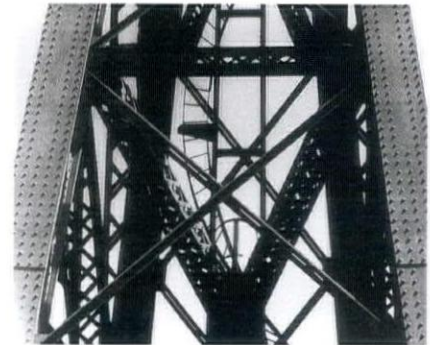
5b. Viaduct at Garabit (1880-84), Gustave Eiffel, detail.
