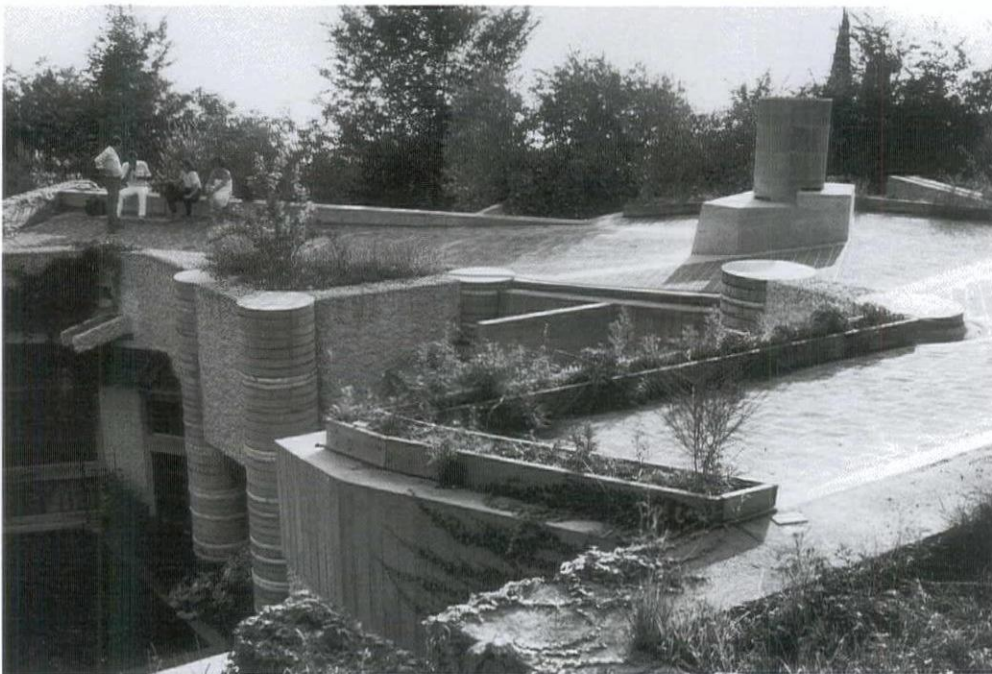
30. Ottolenghi House, Bardolino, Verona (1975), Carlo Scarpa, view of roof.
