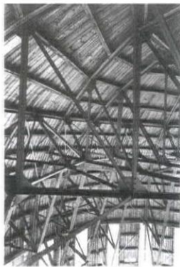
17e. Church Am Steinhof, structure between domes.
