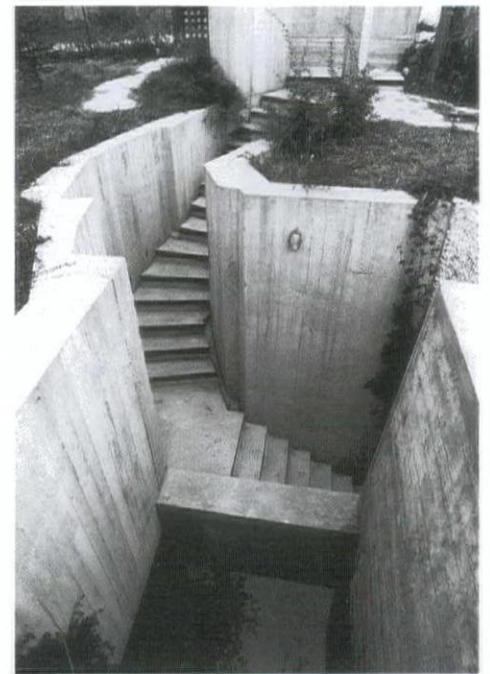
31. Ottolenghi House, passage to roof.
