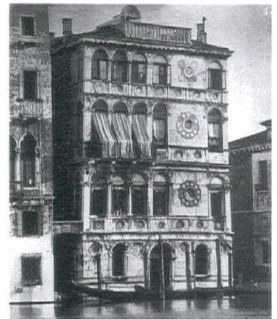
5. Ca'Dario, Venice (1487-97), view before restoration.
