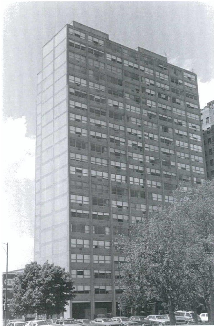
130 41 Aluminum-clad corner columns of Commonwealth Promenade, Chicago, 1955, detail, Mies van der Rohe
