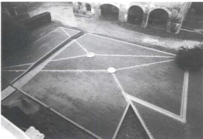
8 Roof of the Ottolenghi House; concrete and brick.
