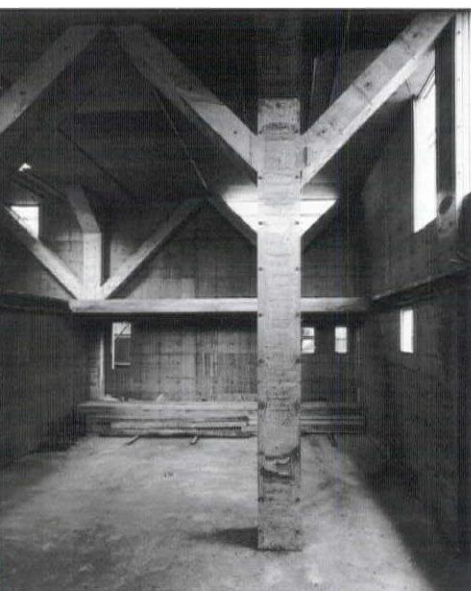
House in Uehara, interior during construction.
