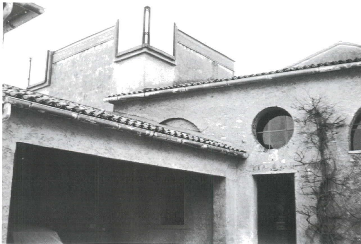
24 Gipsoteca Canoviana in Possagno, 1956-57. Window detail.
