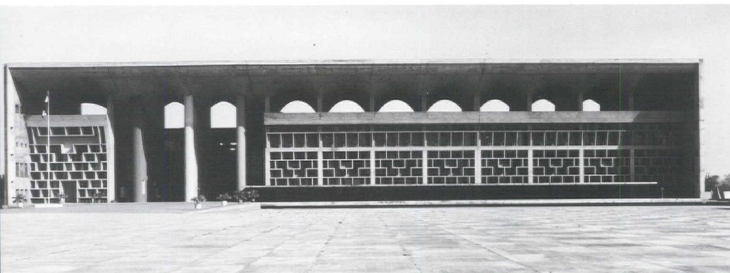
35 Le Corbusier, High Court, Chandigarh, 1951–55.
