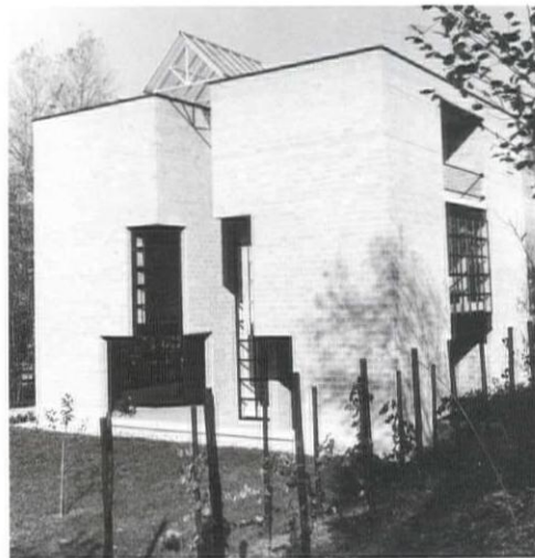
2 House in Pregassona, 1979.
