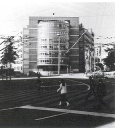
Fribourg Bank, 1977-82, exterior corner.
