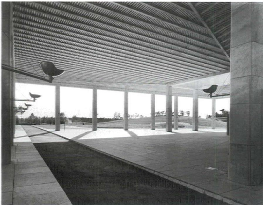
29 Woodland Crematorium, view from the loggia towards the meditation grove on the knoll.
