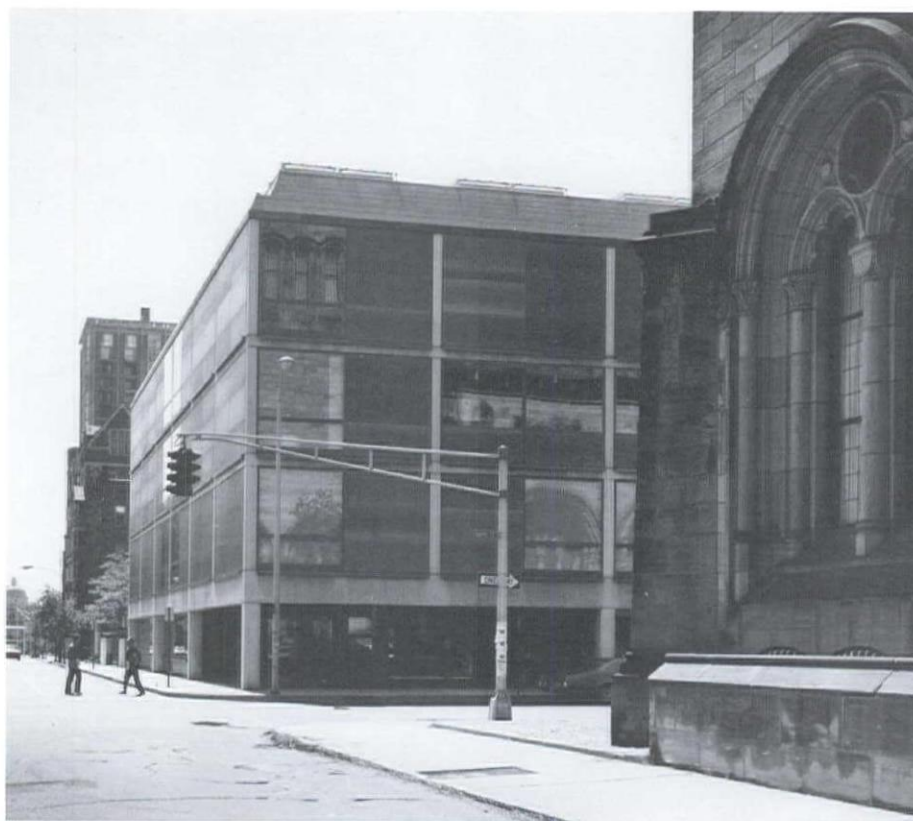
View from High Street (entrance)
