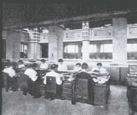
Frank Lloyd Wright Larkin Building View toward interior court
