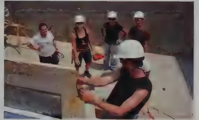
sill plate installation
