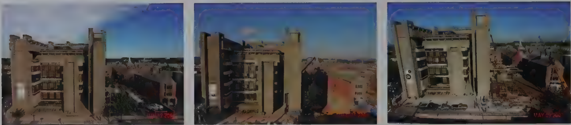
Center for the History of Art construction sequence
