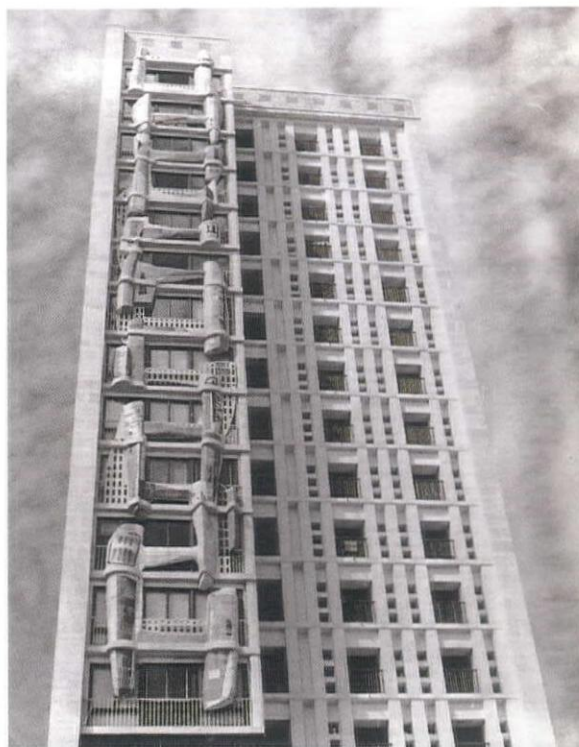
20-storey tower block, Algiers. Architect Pouillon plays with sculpture – with rather doubtful results.
