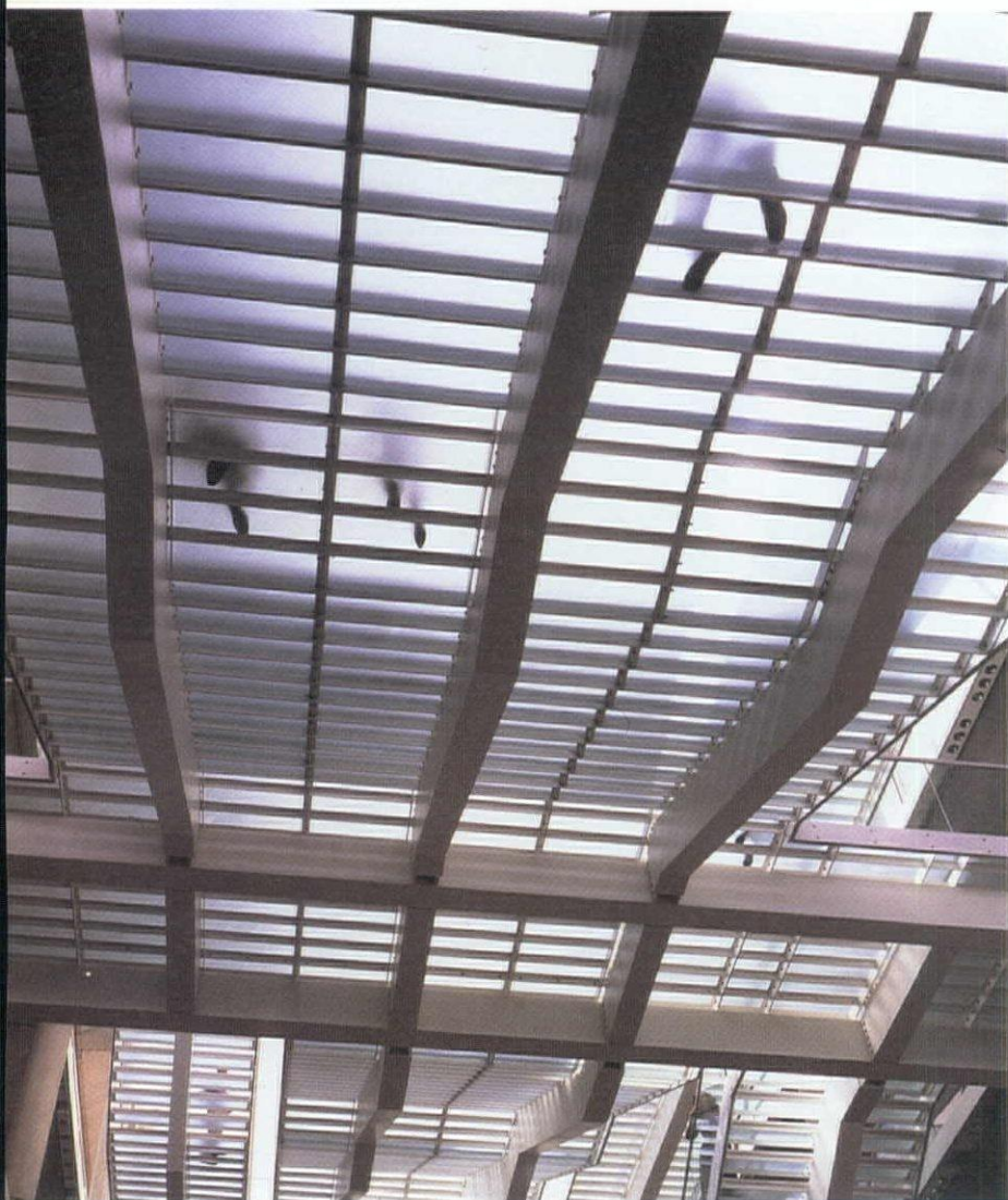
1: Glass floor of the staircase in Sir Norman Foster's Carré d'Art, Nîmes, France
