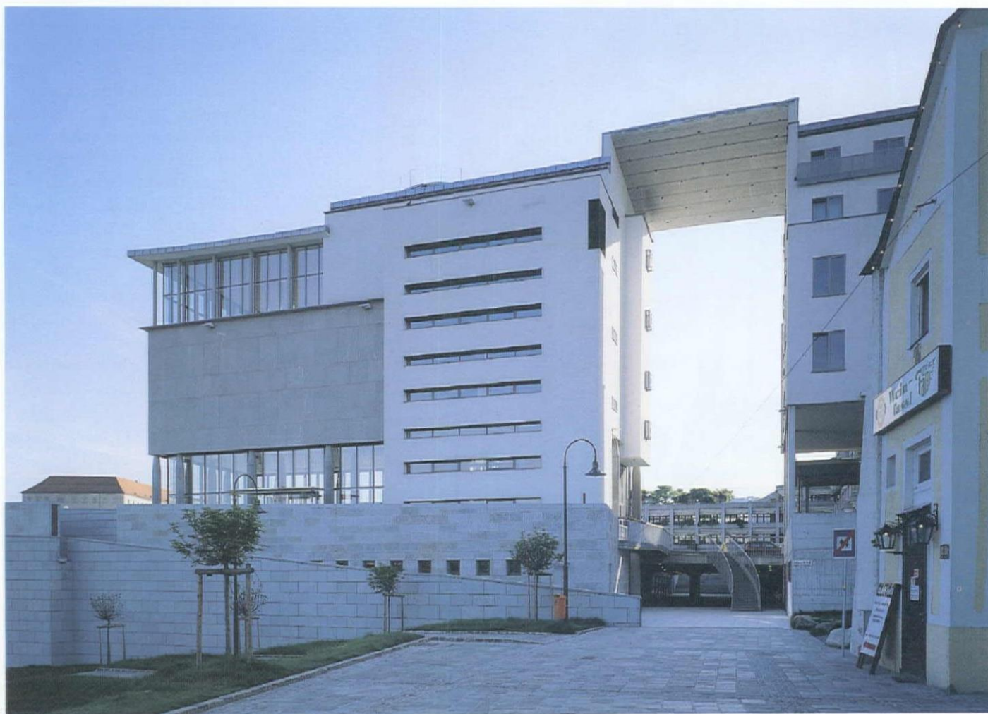
2: Solid wall of the main building with the transparent sections on the third and fifth floors
