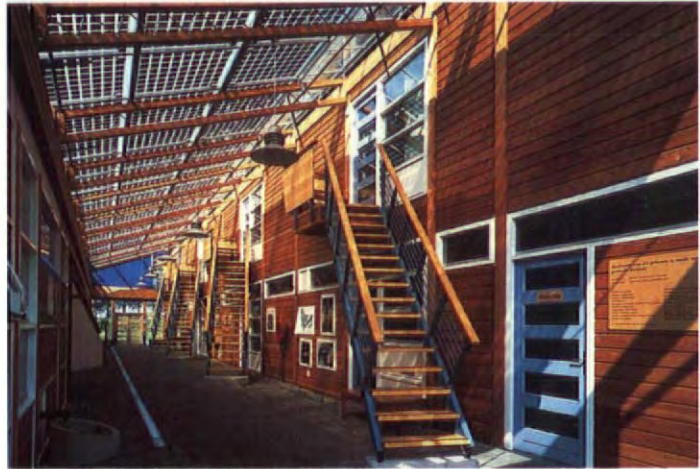
Architect Marc Rutschi designed the canopy of this railway station in Morges, Switzerland to generate electricity; facilitate natural daylight penetration and to comply with Swiss wind/snow loads
