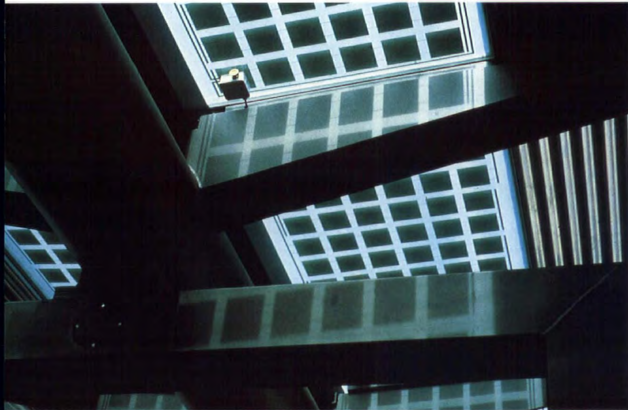
Architect Marc Rutschi designed the canopy of this railway station in Morges, Switzerland to generate electricity; facilitate natural daylight penetration and to comply with Swiss wind/snow loads
