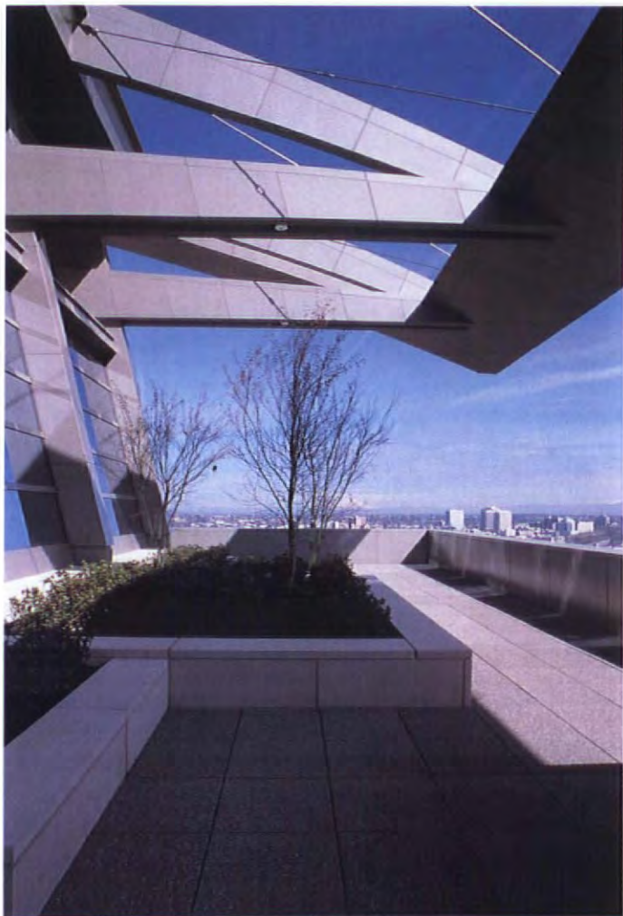
Roof gardens with cantilevered adjustable shades
