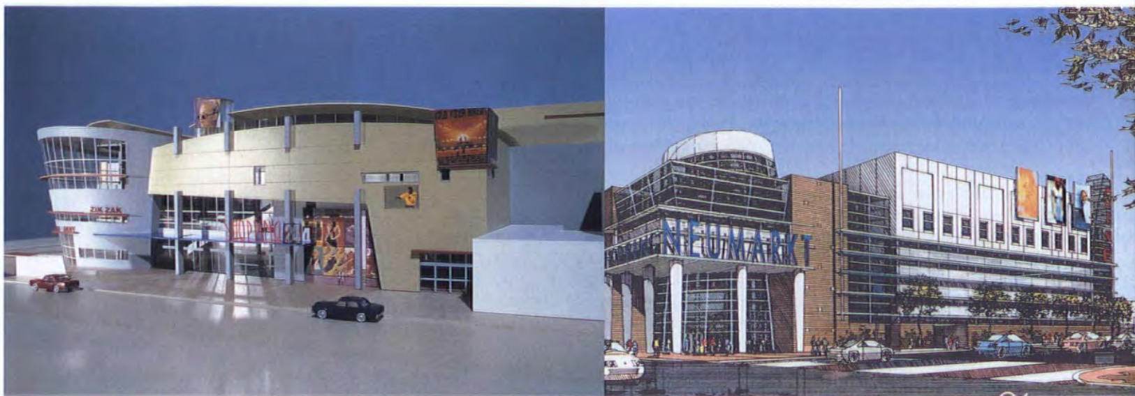
Facing page: Virgin Megastore, California, USA, 1996. Architect: Mark Dziewulski. Virgin has also employed SPFA for the development of concept stores
