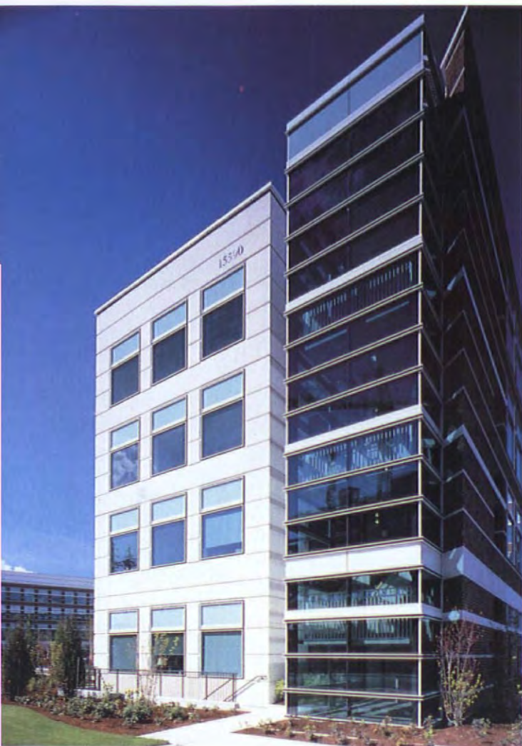
Above left: Careful articulation of the mod bays prevents the cold glare of a curtain wall
