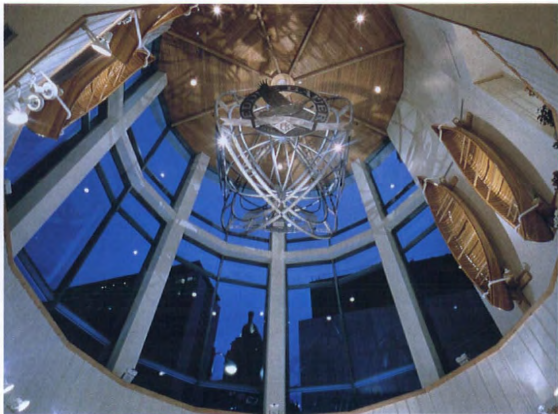
Eddie Bauer store, Michigan Avenue, Chicago, USA designed by the Cincinnati-based office, FRCH
