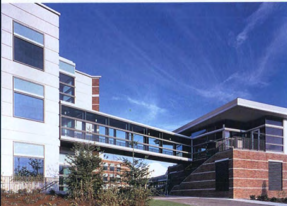
Below: Each building is joined at the base with a glass-enclosed bridge connector
