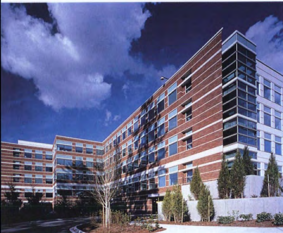
Above: L-shaped plan allows for maximum flexibility to accommodate expanding and contracting workforce
