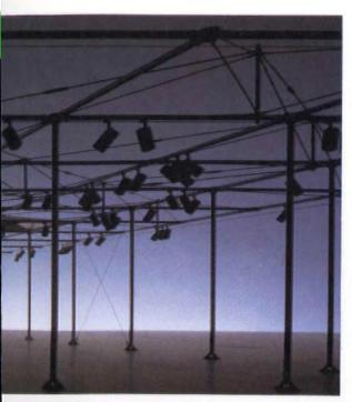
Each square module comprises four tubes joined to nodes at the corners. A module is braced by means of eight tension rods that run from the nodes to the upper and lower ends of the central hub.
