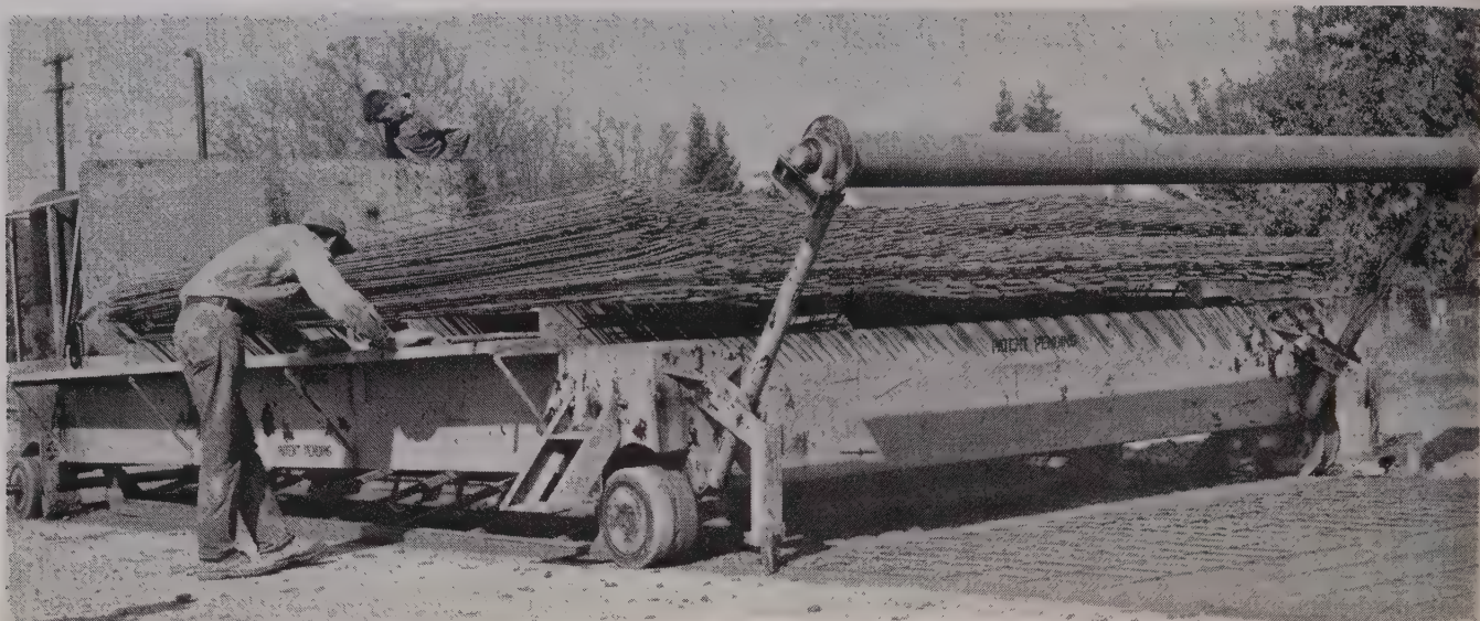
WIRE MESH is embedded in fresh concrete by vibrating grid beneath this machine designed by Houck and built by his crew. Engine driving
