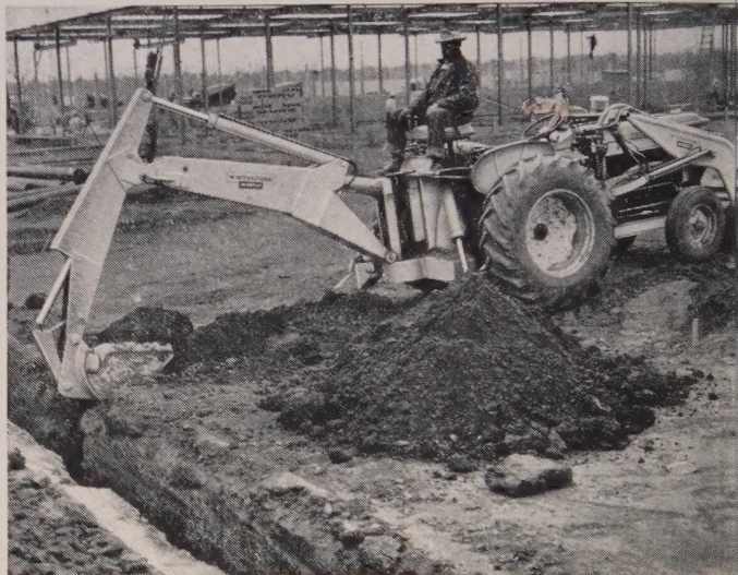
61 hp* International 460 with International Wagner loader and backhoe ... leads its field in trenching speed.
