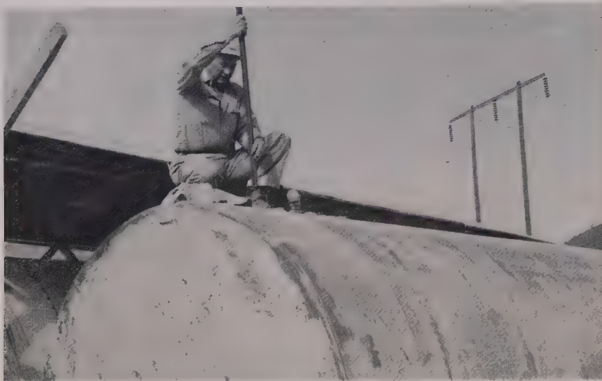
ADRIAN COX , Gibbons & Reed, measures fuel in job storage tank. Tank is kept full to reduce air chamber, and has filtered breather.
