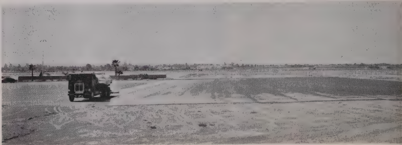
LARGE parking area north of Terminal Building at Meadows Field, Bakersfield, showing distributor applying 0.20 gsy. of Reclamite
