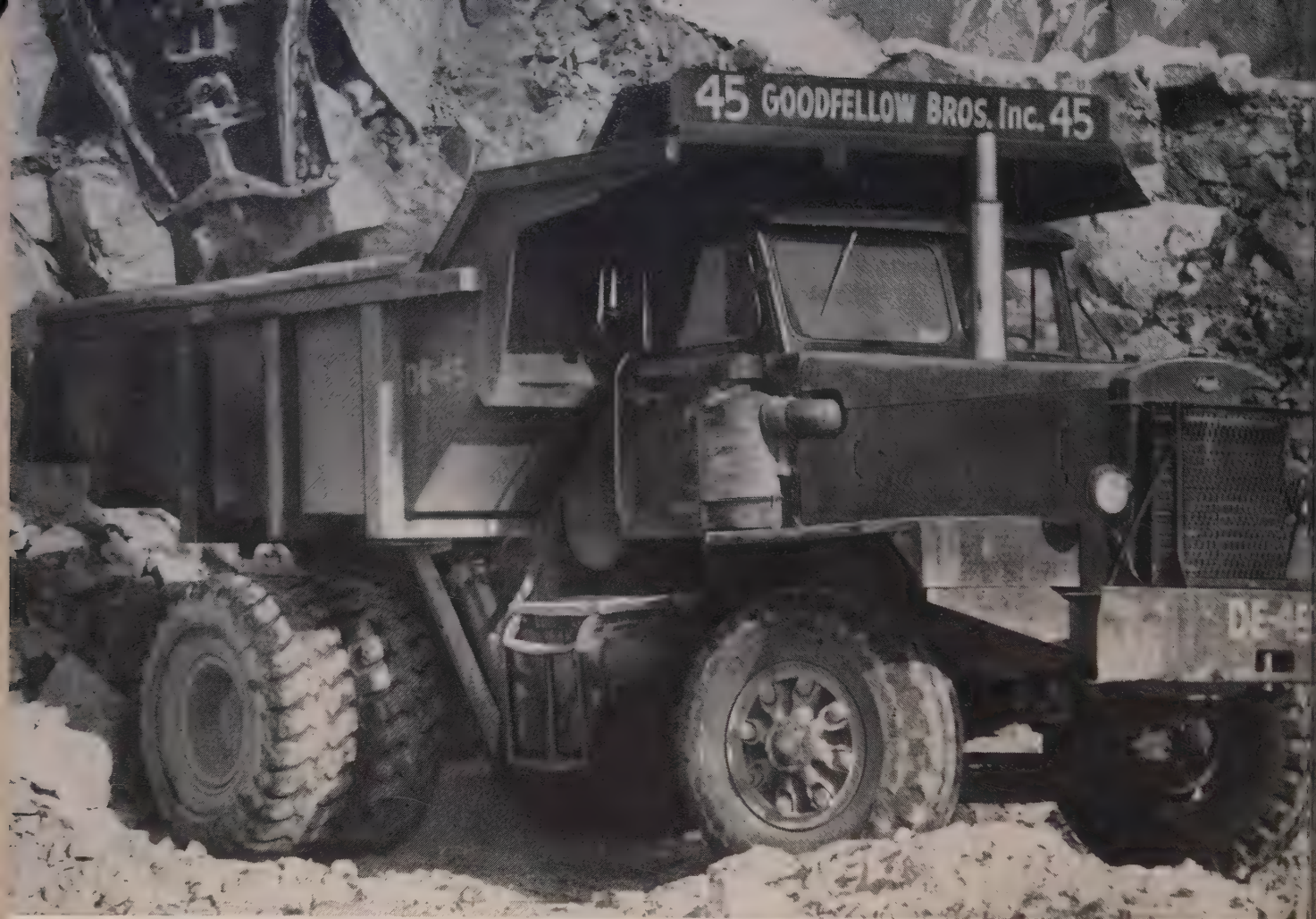
MACK LVX DUMPERS RIPRAP A RISING RIVER. When complete, Washington State's Rocky Reach Dam will raise a pool in the Columbia River that would have periled the track foundations of the Great Northern Railroad. To prevent this, Goodfellow Bros., Inc., of Wenatchee is using 15 big LVX Mack dumpers to move over a million tons of rock for riprapping and reinforcement of the roadbed.
