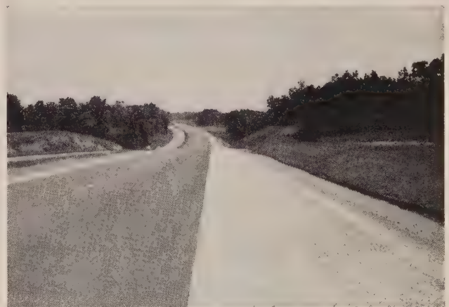
Outside Shoulders of stabilized aggregate base were Asphalt surface treated for width of 10 ft. One-half inch granite stone chips provide better traffic lane demarcation.
