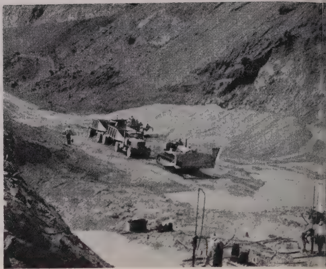
FILTER ROCK placed on foundation with aid of tractor which pulls rock trucks through the deposit area. Second tractor spreads gravel.
