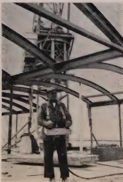
CRANE operator holds remote control panel which he carries around the work floor.
