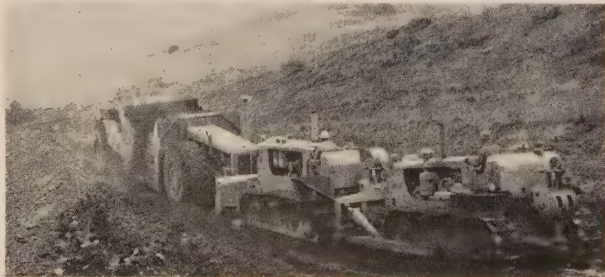
POWER in plenty is available for high speed earth-moving. Here a D9 and D8 push-load twin-engine Euclid TS24 scraper. Scrapers loaded out of gear to reduce tire wear.
