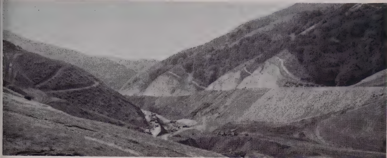
DOWNSTREAM view of dam site showing major road cuts along right side of canyon. Material for dam comes from borrow area at left.
