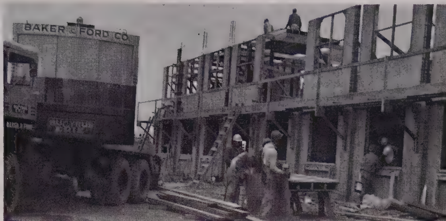
TILT-UP construction was used extensively to meet the tight time schedule. Careful study showed that the method could be applied to several units ordinarily overlooked—such as stairwell enclosures, firewalls and interior walls. The picture shows work on 300-man housing wings.
