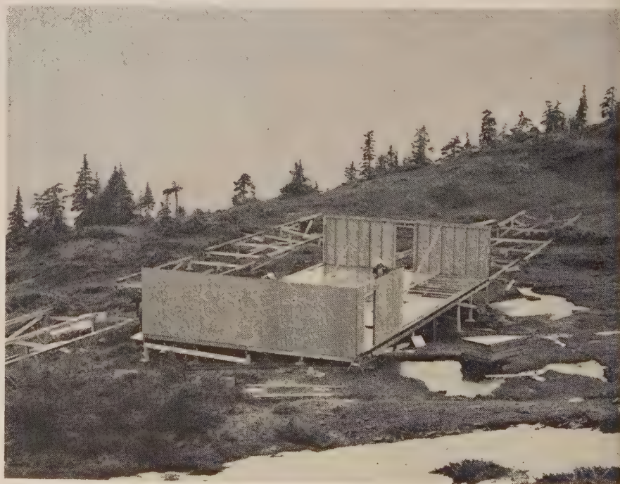
PRACTICALLY ALL of the material for a second camp on top of a mountain at Duncan Canal, Alaska, was flown to the site by a helicopter. Manson-Osberg workmen are shown here assembling prefabricated panels with some of the winter's snow still in the foreground.
