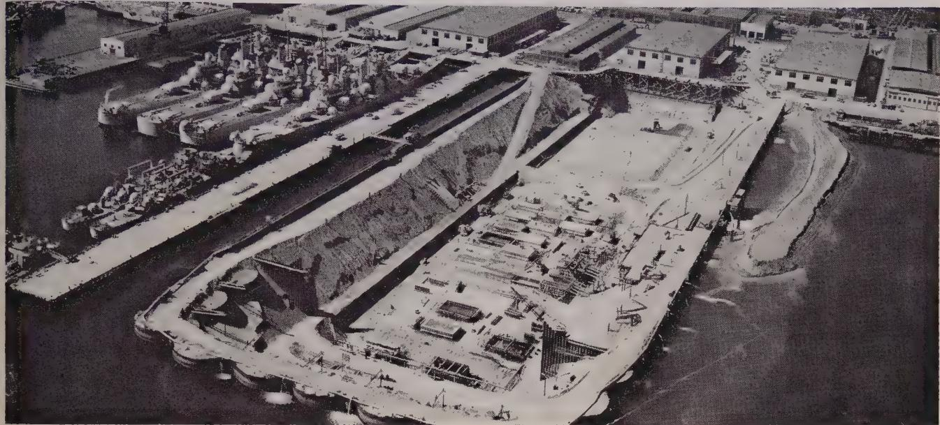
**DOCK SITE** is formed by parallel earthfill cofferdams 500 ft. apart which protrude 1,300 ft. into water from shore. Ends are joined by
