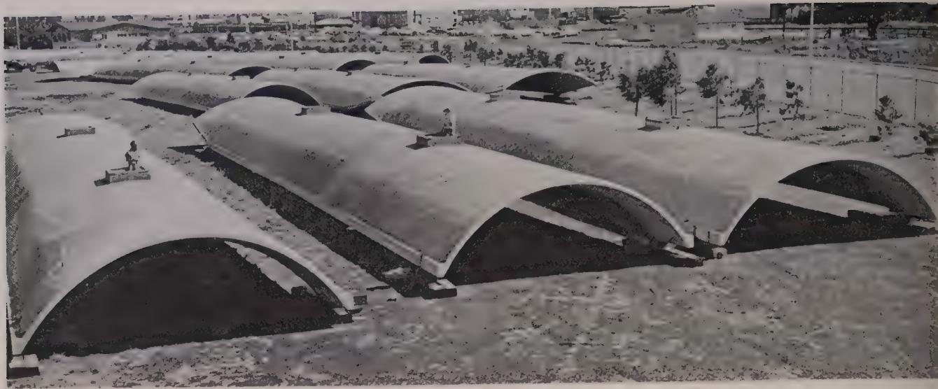
**STOCKPILE OF SHELLS** is located adjacent to casting yard and building. Availability of storage space made precasting feasible, as units are
