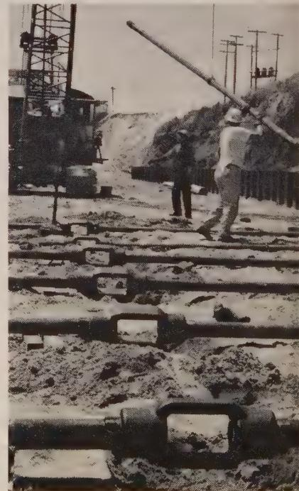
86 feet wide, made of steel sheet piling 60 feet high. The bottom of the canal will be 13 feet below mean tide level.
