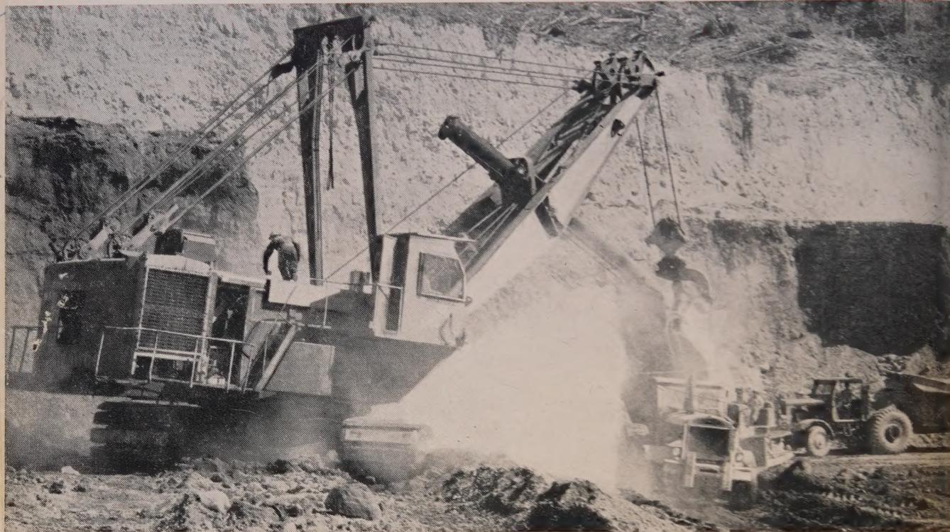
**At world's highest earth-filled dam** construction site near Woodland, Washington, three giant diesel shovels get immediate starts from Chevron Pressure Primer System, reports Jones-Tomkins, general contractors. System helps speed shovel's fill-borrowing operations for this \$51,000,000 project.
