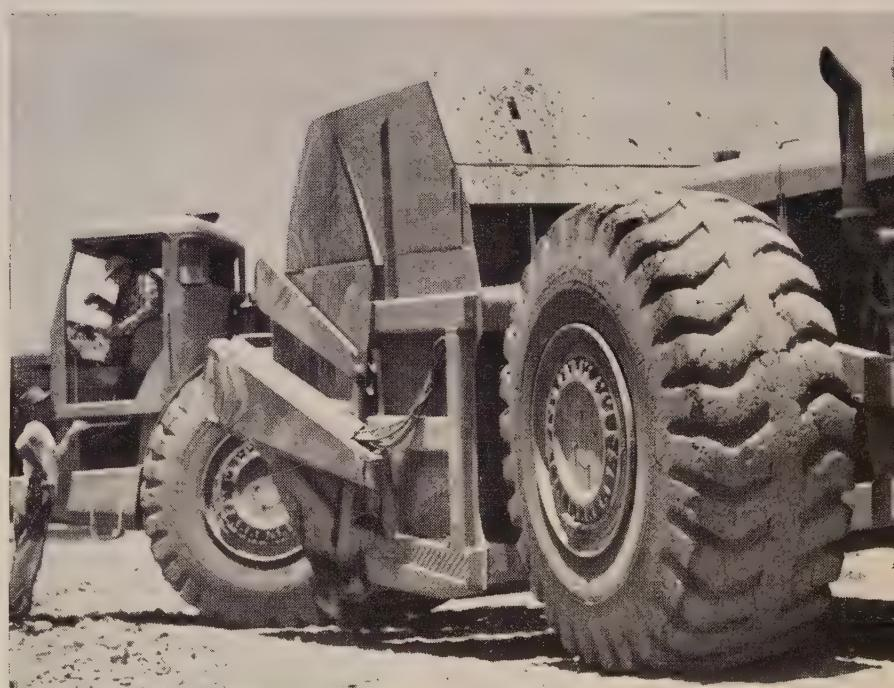
**RETREADED B.F. GOODRICH ROCK SERVICE TIRE** in foreground has already given over 2,200 hours of service (some tires on the project have worked over 3,200 hours). BFG builds the Rock Service in 3 compounds — Regular; Cut Protected (CP) for short hauls over jagged rock; and Heat Resistant (HR) for longer runs at higher speeds.
