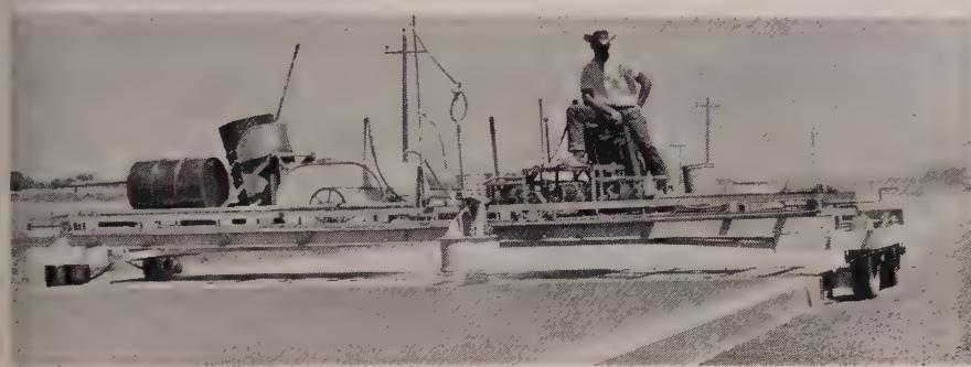
CURING COMPOUND placed with a self-propelled rig. Note the clean, sharp side of the slab.
