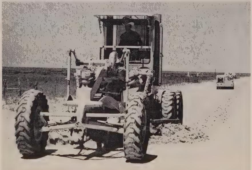
SHAPING up the stabilized base followed by pneumatic rolling. The roller is ballasted to 17 tons. As material tightens up more water is added to the surface.
