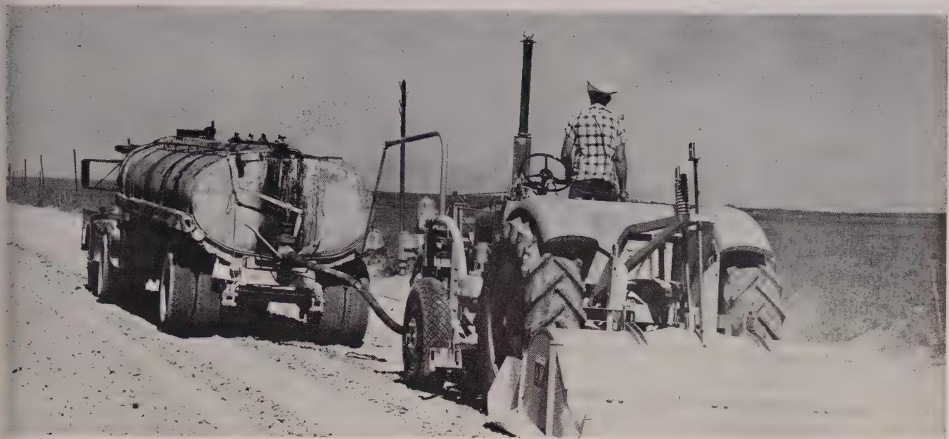
**FIRST PASS** of Trav-L-Plant mixes caliche and salt with water injected from the truck. The process moistens the entire lift. The 7-ft. swath
