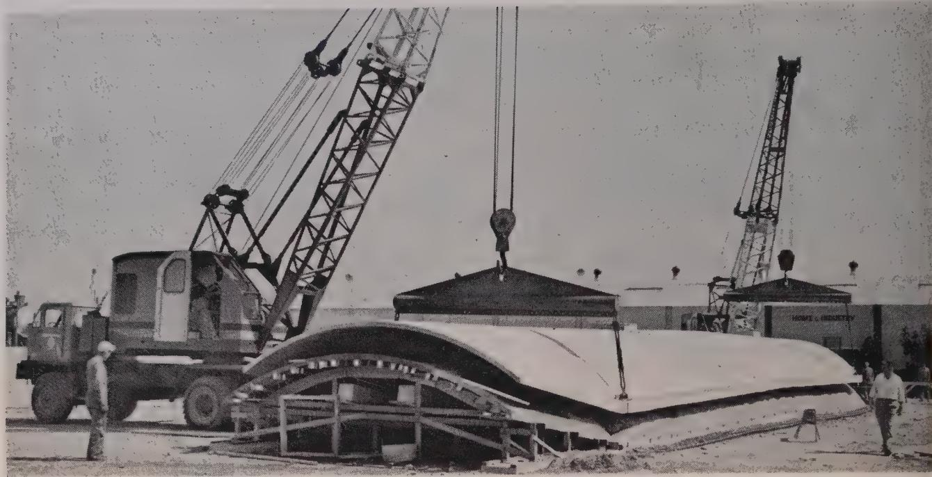
LIFTING SHELLS from form is done with two truck cranes after concrete has cured for seven days. As shells are lifted, steel tie rods
