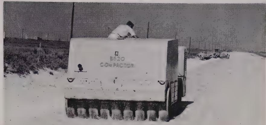
"SLUSH ROLLING" is a process of the Texas Highway Department and consists of pneumatic rolling to work the caliche surface to a paste-like consistency.
