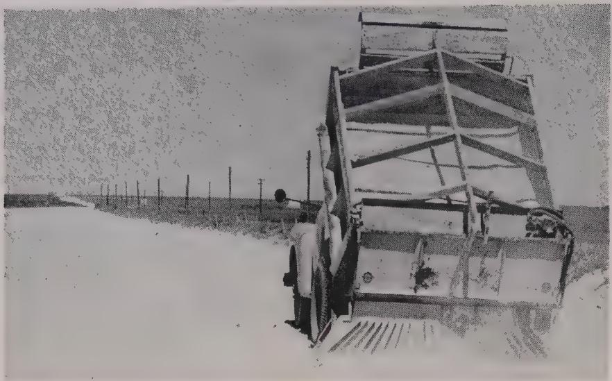
SALT being spread at a rate of .75 lb. per sq. yd. per inch of compacted thickness. Salt is loaded into truck by front-end loader from stockpiles along the road.
