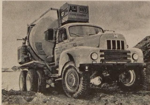
trucks announced by International Harvester Co. The new units are the R-210 (4x4) rated at 39,000 lb. gross vehicle weight, and RF-210 (6x6) at 49,000 lb. With optional front axles, the weight ratings of these units can be increased to 42,000 and 52,000 lb. respectively.
