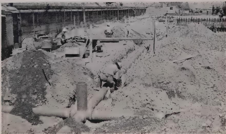
**NETWORK** of drainage pipes will underlie floor of dock to constantly remove ground-water, thus keeping uplift forces small. Permanent pumps will be electric, with diesel standing by.
