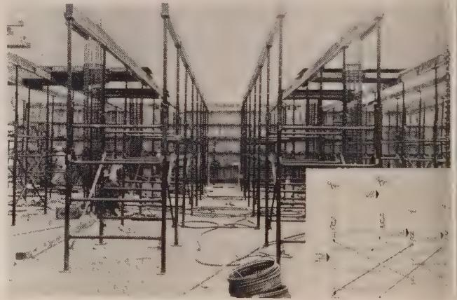
pacity of double that of conventional steel scaffolding, and yet can be erected with all the speed of the latter. Because of this speed, substantial savings can be realized in erection, stripping, forming, etc. The picture shows an installation for a county office building in San Jose, Calif. The contractor stated that the use of the "Hi-Load" shoring cut his costs of shoring erection time by more than 25%. ... Write No. 176
