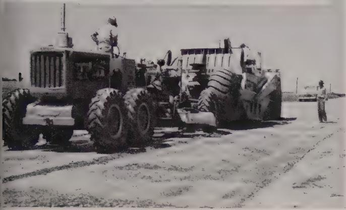
**Local sand** shaped in windrow, bladed to reduce moisture to less than 1%, reshaped into windrow, mixed with Asphalt through traveling mixer—aerated and compacted.
