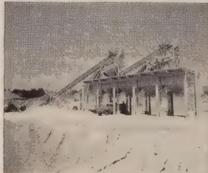
Stationary installation—Lima A-W line includes jaw and roll crushers, matching screens, elevators, conveyors and bins.
