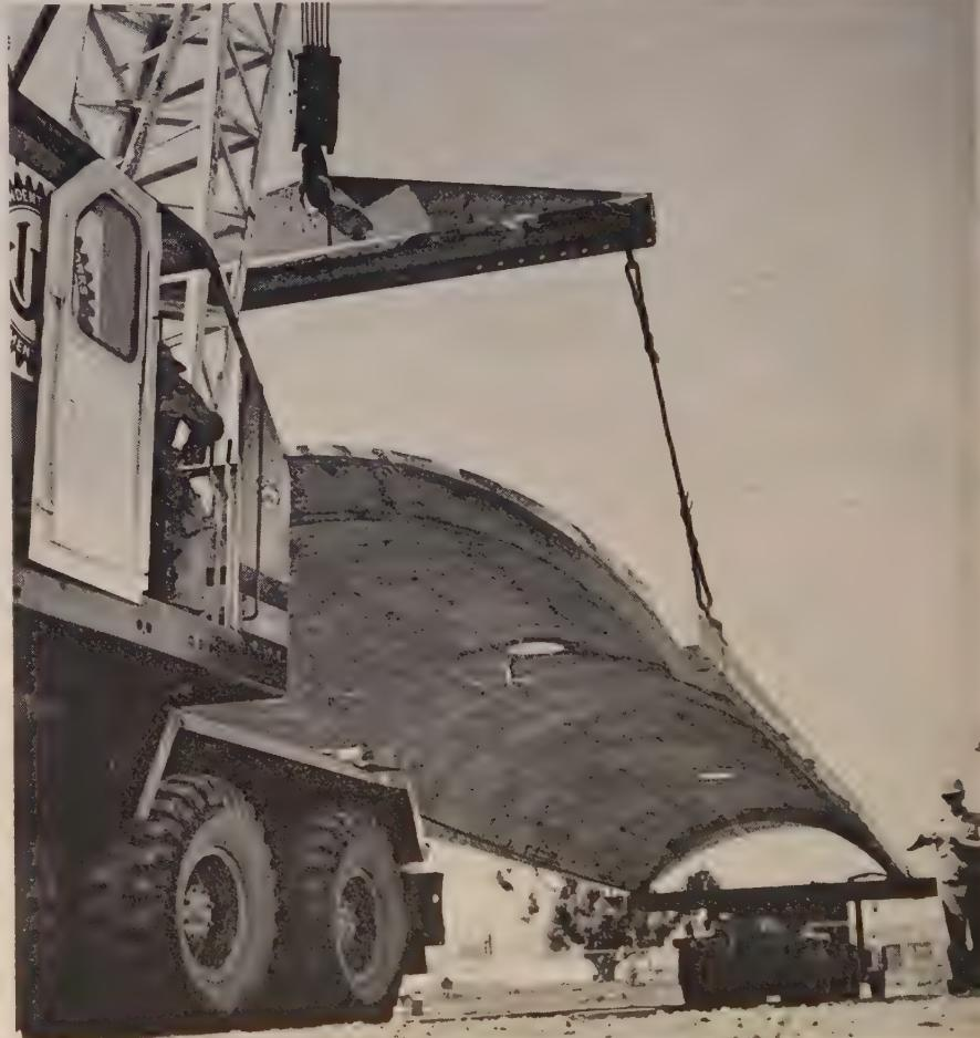
**MOVING SHELLS** was done with truck tractor in front and truck crane in back. Trick was horizontal beam on truck (background), compensating for haul road unevenness.
