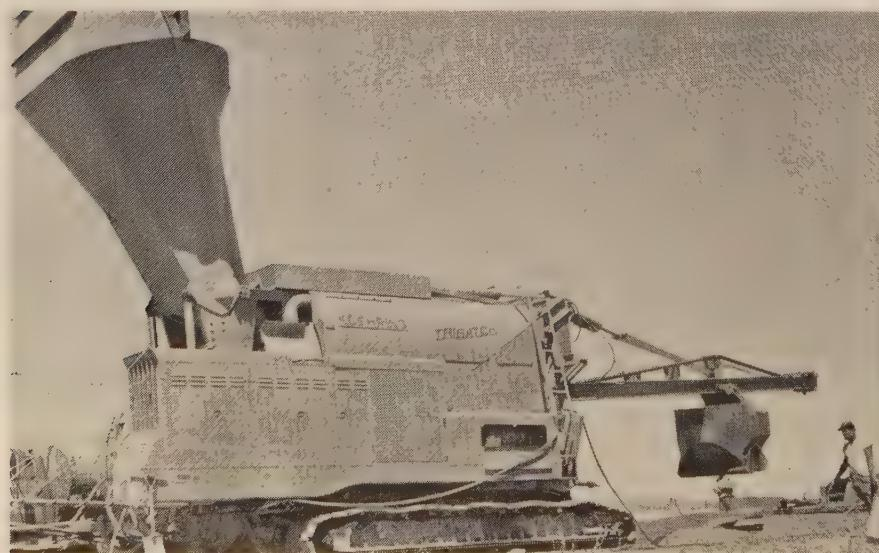
FIRST appearance of the Tribatch mixer on a Colorado highway job, and first combined use of this mixer and a slip-form paver in the state. The five-compartment truck (top of page) feeds the paver, with batches that move through the three drums in succession. Concrete is deposited on the base at a rate of about a batch every 29 sec.
