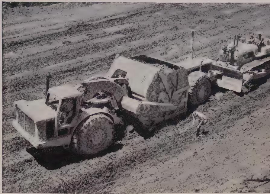
**FOREMAN SETS GRADE STAKES** as BFG Rock Service tires shoulder another 35-ton load of fill dirt. Finished 4-lane highway will be 60 feet wide, surfaced with 4-inch-thick asphalt, will have 4 bridges and 100,000 feet of 2" horizontal water drain pipe. B.F.Goodrich on-the-job tire service is available on projects such as this.
