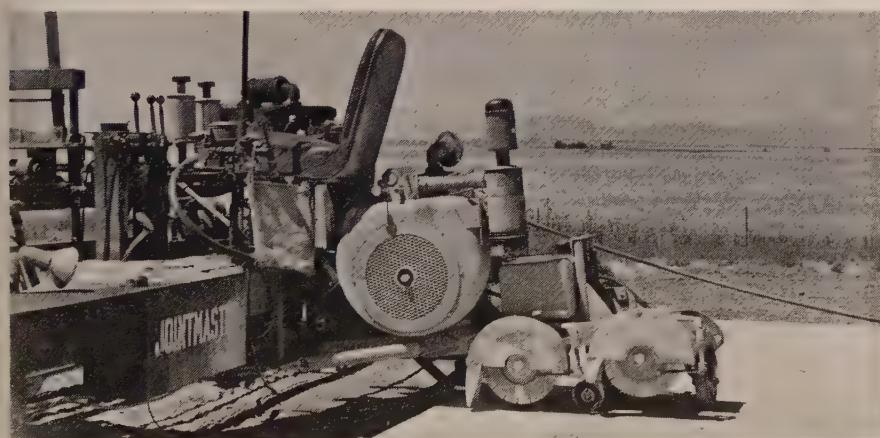
CUTTING both longitudinal and transverse (20-ft.) joints with a self-propelled Jointmaster saw.
