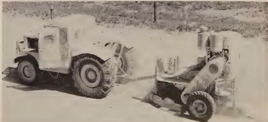
**REDUCTION** of pit-run caliche in place to a 3-in. maximum. This run of the Pulvi-Breaker, drawn by a Cat DW-10, precedes spreading the salt.
