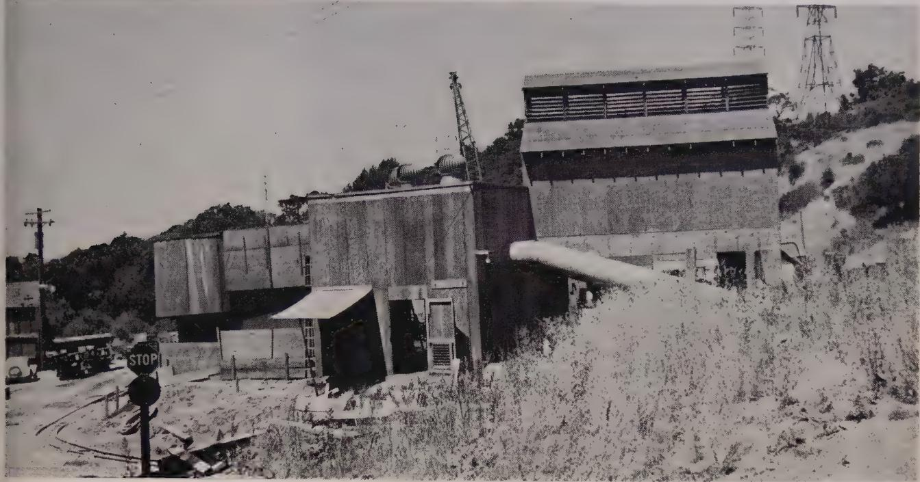
WINCHESTER HOUSE, the plywood building erected to enclose compressors and fan line. On left is noise suppression chamber.
