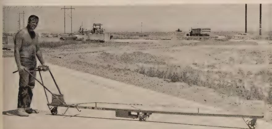
CONTRACTOR-BUILT thump-o-meter by men of Gardner Construction Co. to be sure that the slab had the smoothness required by the highway department.
