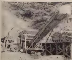
**SIERRA TOWBATCHER:** Portable towbatcher with capacity of 50 yards per hour. Unique "cement sandwich" feature protects cement in aggregate layers.
