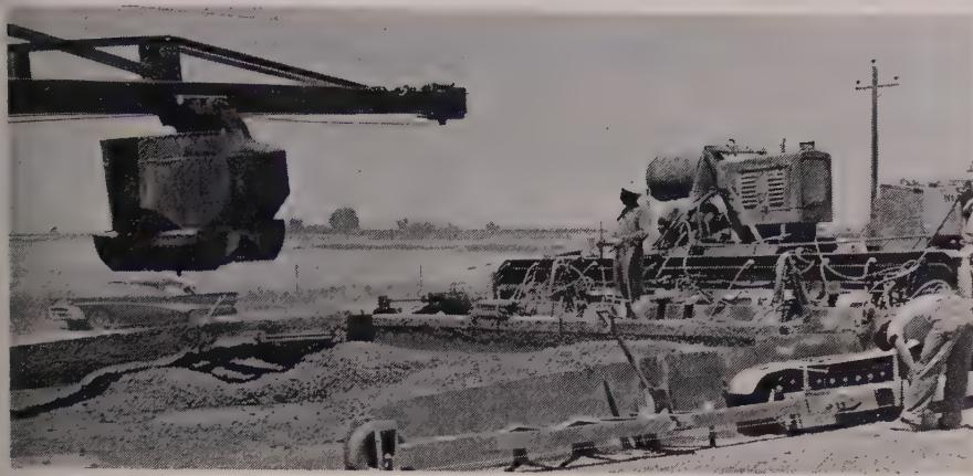
MOVING FORWARD on its crawlers the slip-form spreads and finishes the batches.
