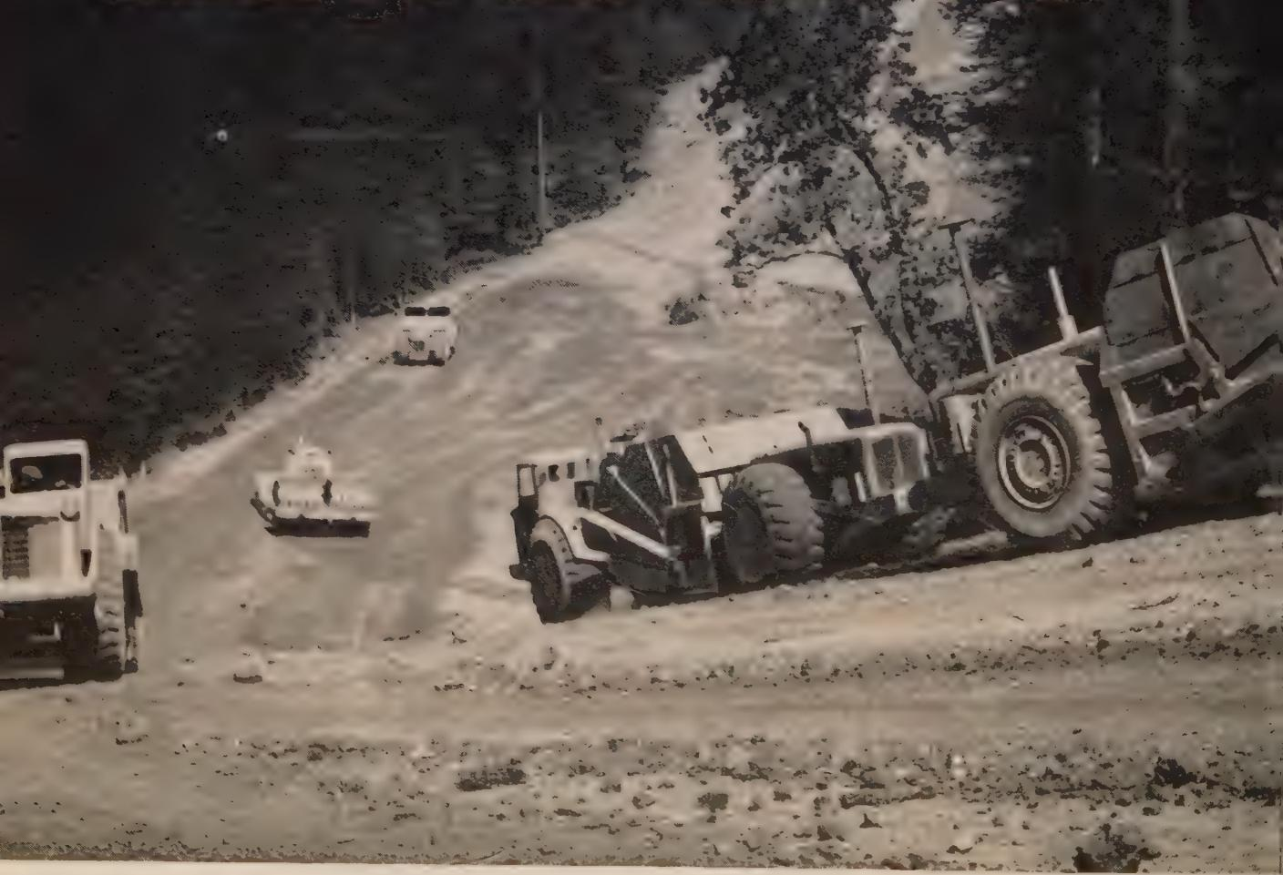
**MORRISON-KNUDSEN EARTH-MOVERS** climb 42% grade after delivering 35 tons of fill dirt. Equipment works 18 hours a day, 6 days a week, to speed completion of Redwood Highway bypass near Weott,
