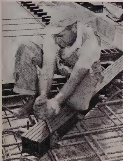
placed across the face of the joint. As soon as the concrete has sufficiently hardened, the precompression holding pin is removed releasing the pressure of the through bolt and allowing the unit freedom to contract or expand as it rides between the concrete panels. A neoprene plug is inserted to seal the hole left by removal of the through bolt. Ends of each joint are sealed, at the factory, with flexible neoprene diaphragms.
