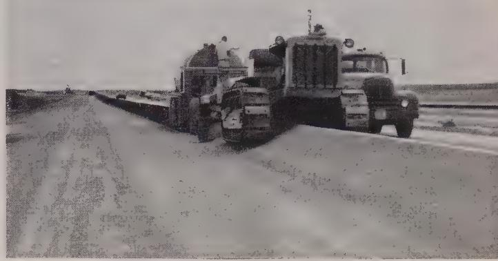
**Supporting courses** are compacted with high contact pressure pneumatic roller to assure smoother riding under all traffic weights to come. Contractor's equipment was permitted on base course during construction of successive layers, which assisted in obtaining maximum density and reducing haul costs.
