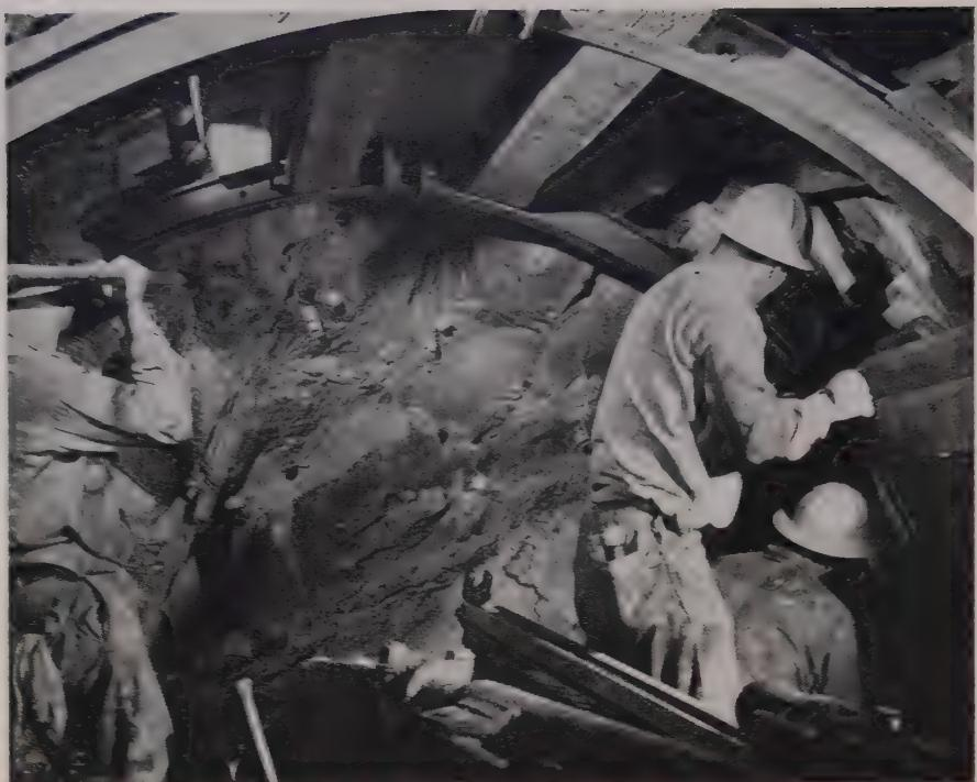
MINERS tamp powder in 5-ft. drill holes. Typical round consists of 40 holes in pyramid pattern using 50 lb. of powder fired on eight delays with 1 primer per hole.
