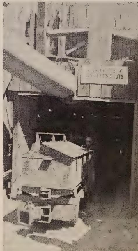
PORAL with thick reefer doors to reduce noise. Blast chute emerges from roof.
