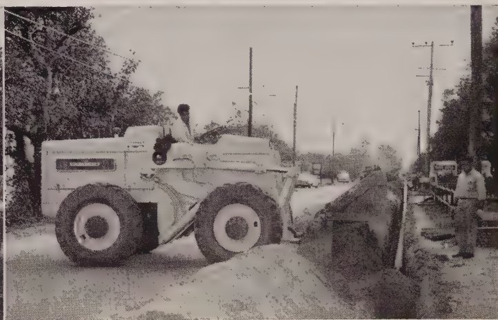
Backfilling. (same job as at left.) The user says, "versatility of the 'PAYLOADER' tractor-shovel with Drott '4-in-1' Bucket pays off continuously."
