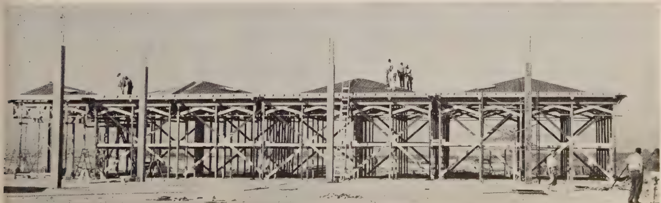
FOUR forms in place for pouring. Shoring is not complete at left where mobile gantries still support roof units. Roof is made up of
