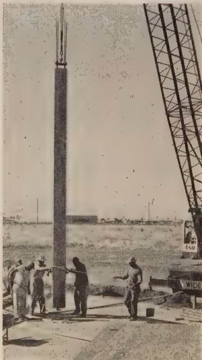
COLUMN is lowered in "socket" 18 in. deep cast with 1-in. clearance.
