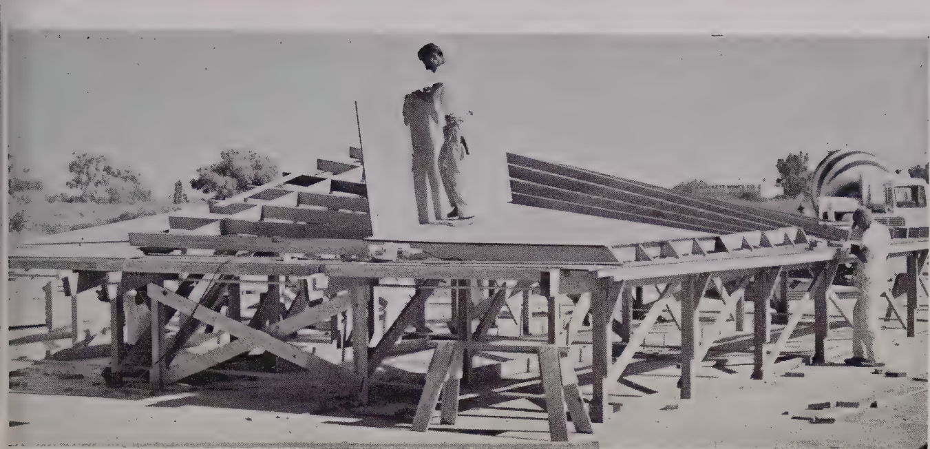
PLYWOOD sheets are warped over stringers to make skin of form for umbrella section. Forms were built in two halves to facilitate moving.
