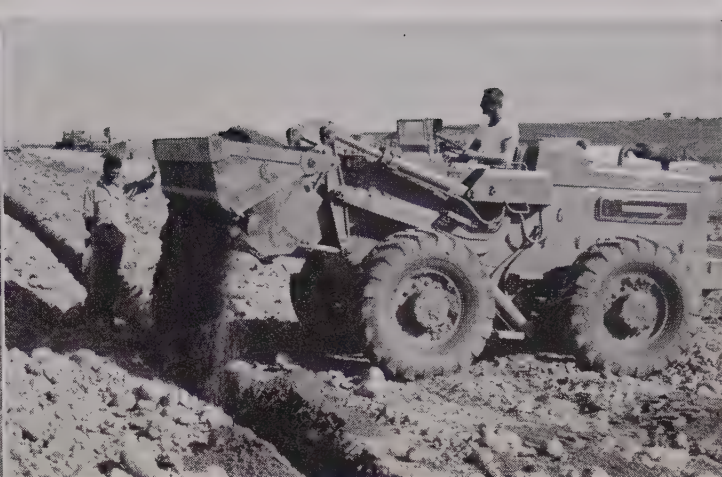
Padding Trench. Drott "4-in-1" Bucket accurately meters dirt padding into rocky trench bottom for gas distribution line — also lowered-in, backfilled and cleaned-up on this job.
