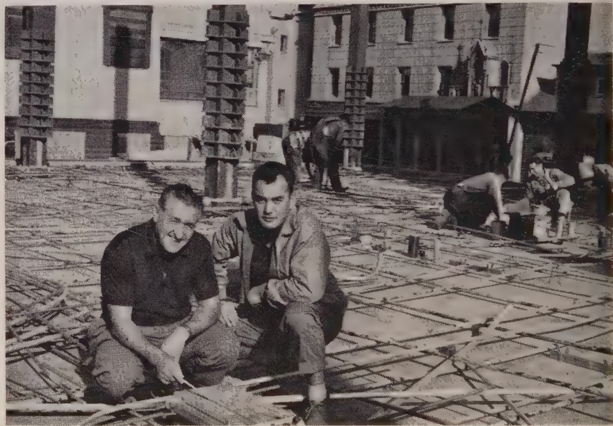
KEY MEN on project were (left) George P. Belcher, contractor-owner, and Herbert Korner, engineer-in-charge. Note maze of reinforcing and utility conduits in floor slab. On columns in background are steel collars which are cast into each slab to facilitate lifting.
