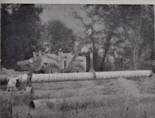
Cross-country Pipelining. Holding 22" natural gas pipe for tack-welding. Side-boom capacities are available up to 12,000 lbs. at 4 ft. overhang and 6,000 lbs. at 8 ft. overhang.
