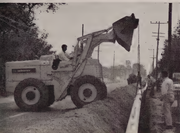
Lowering-In. Installing 8" gas main along highway. Tires do not injure pavement, traffic is maintained and "PAYLOADER" moves quickly to any part of the job.
