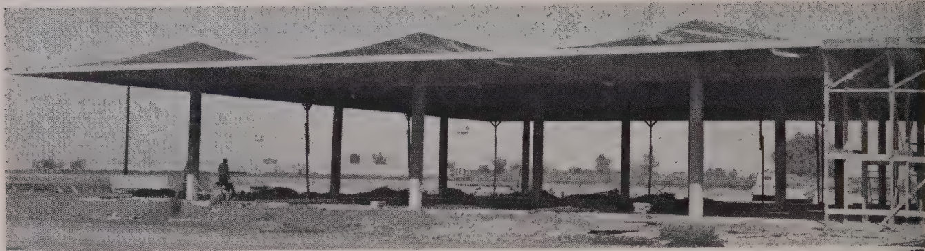
THREE BAYS of four shells each are completed and forms, far right, in place for next pour. Walls were tilt-up concrete panels hoisted in
