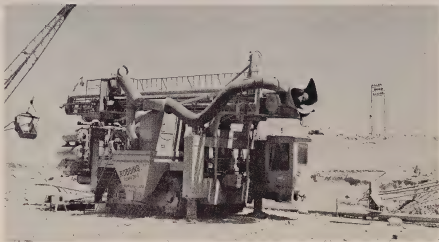
ROBBINS DRILL will be used to sink 17-in. holes 70 ft. into bedrock for anchoring part of powerhouse. In photo, mast is lying over top of machine. At upper right is three-part bit with rubber shield and hose for controlling dust. Rig is crawler-mounted.
