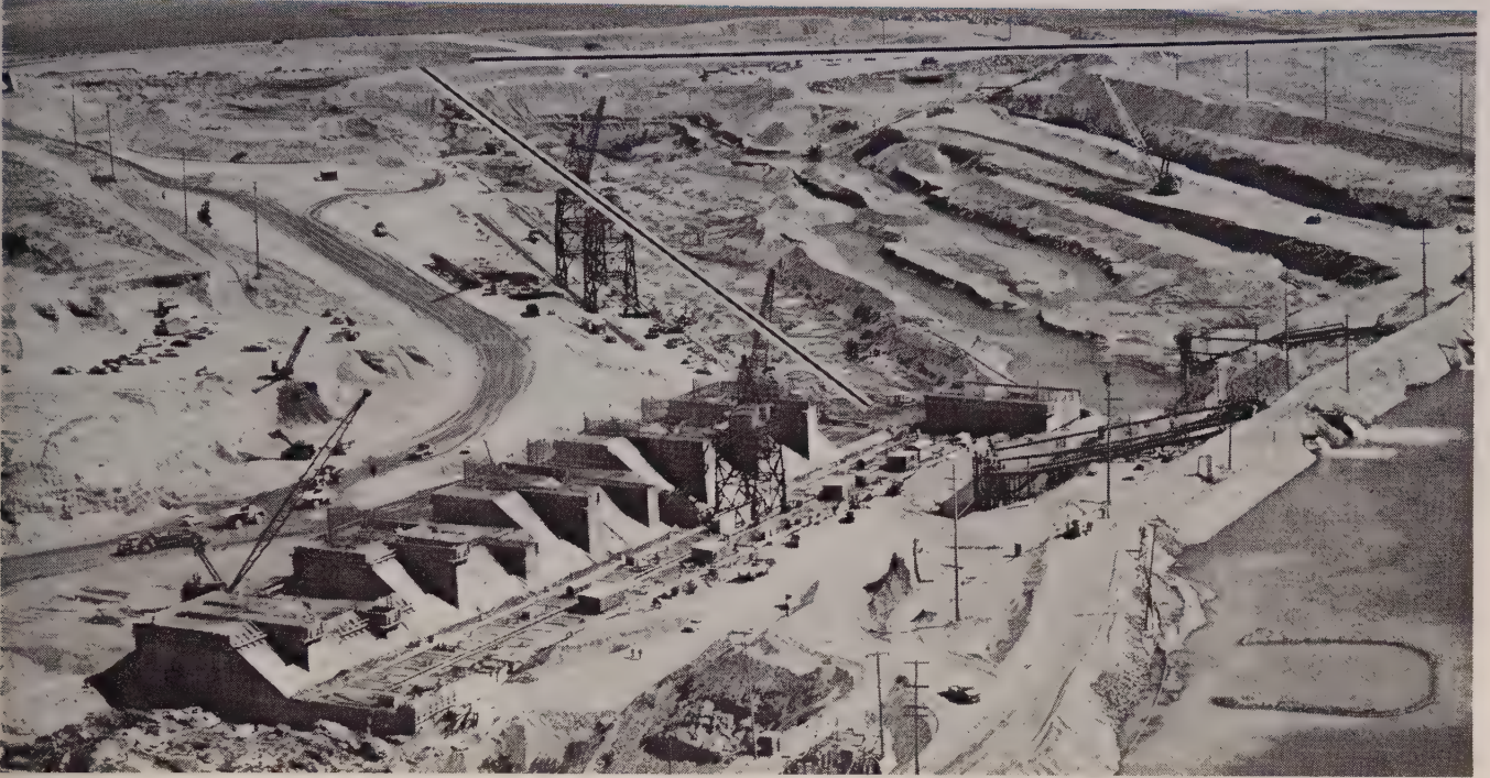
AERIAL VIEW of Wanapum Dam on Columbia River shows spillway concreting well advanced. Superimposed diagonal line is approximate
