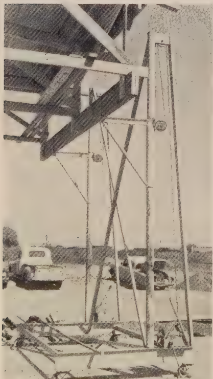
GANTRY on casters supports roof form. Unit rolls into place and is shored for pour.
