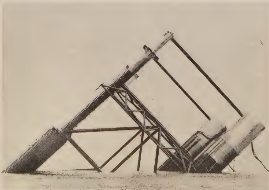
BALLASTED legs swing downward to bring the top of the tower base out of the water. Hoses, right, carry compressed air from barge to control rate of flooding in compartmented tanks.
