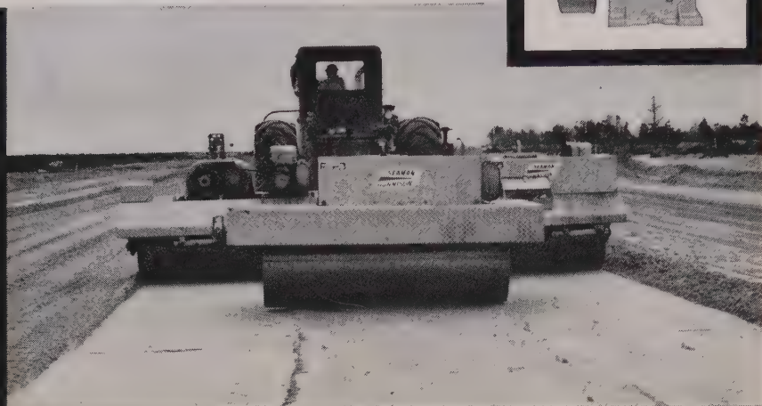
VIBRATORY IMPACTORS — made by Seaman-Gunnison Corp., Milwaukee, Wis. — pack a 13-ton impact wallop at amplitudes up to two inches. Units are powered by 18-hp Model THD Wisconsin Engines.
