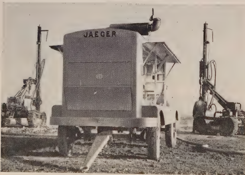
Maintains 100 psig behind two Thor TR-5 air-and-hydraulic crawlers with 4½" drifters without running faster than 1400 rpm.
