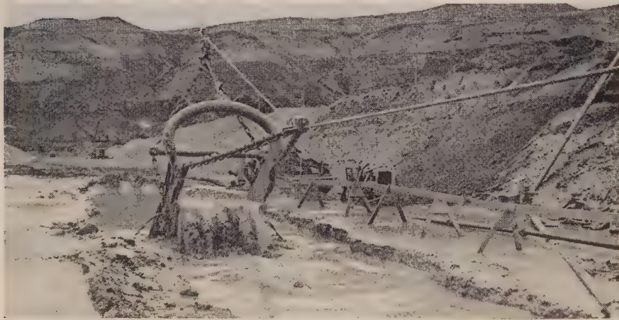
DRAGLINE excavates slurry-filled trench 80 ft. deep with vertical walls through gravel. Heavy slurry displaces ground-water. Clamshell bucket and air-lift handled clean-up.
