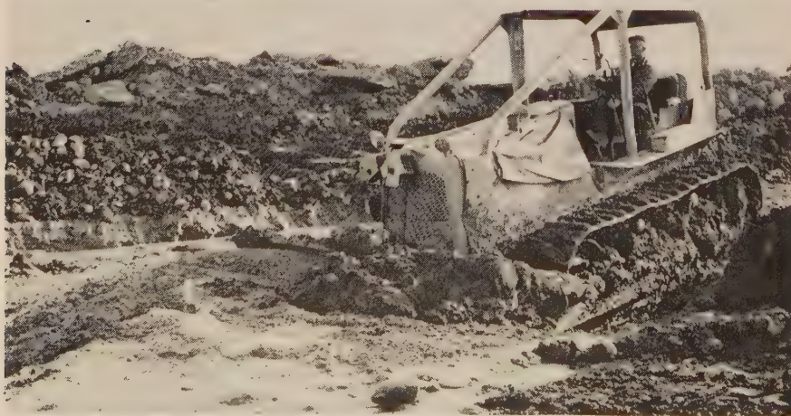
CRAWLER TRACTOR backfills trench with bulldozer using slurry-saturated material which had been excavated. In permanent embankments 3 ft. of tremie concrete was first placed on bedrock.
