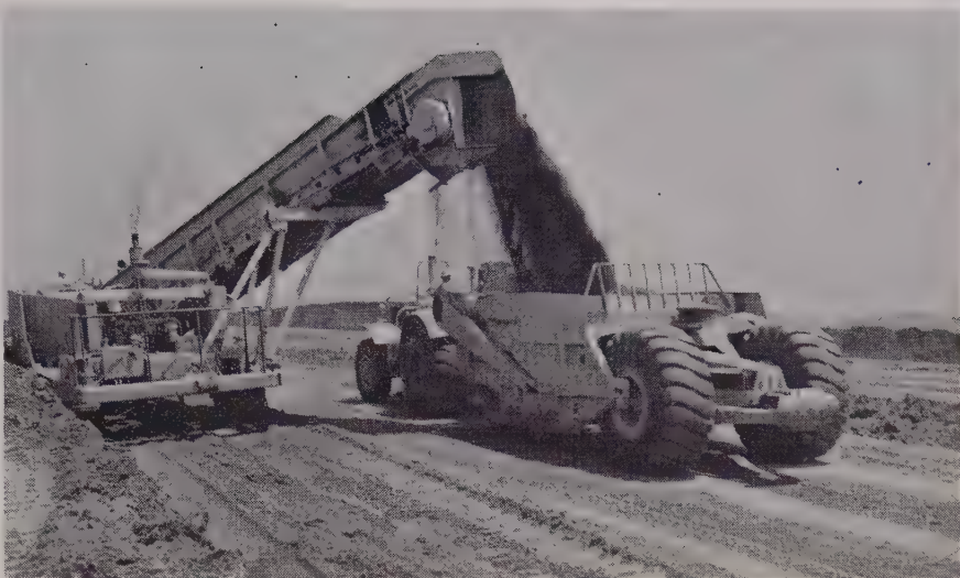
EUCLID BELT LOADER makes such fast work of loading a scraper it takes a dozen DW 20's to keep it busy. Loader is pulled by a turbocharged D-9. Borrow area is ripped in advance.
