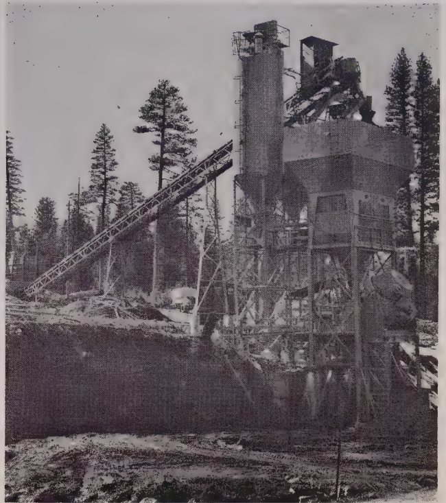
BATCH PLANT above dam. Aggregates are drawn from stockpiles at left, weighed, and mixed in 4-yd. mixer. Trucks drive under mixer.
