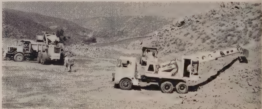
MODERN MACHINES speed slope trimming and clean-up. At left a rubber-tired Michigan loader fills a Euclid rear-dump. Versatile Gradall quickly removes excess material from slope.
