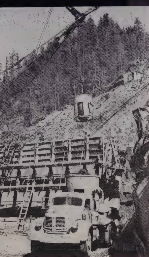
CONCRETE bucket delivered to site by truck is picked up with crane and spotted over dam block.
