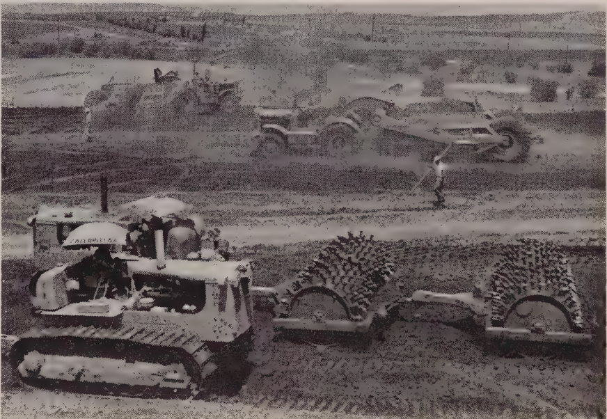
DIKE can be a busy place even though it is 7,800 ft. long. Compaction specs are rigid, requiring two scarifier passes and 12 sheepfoot passes on each 8-in. layer of embankment.
