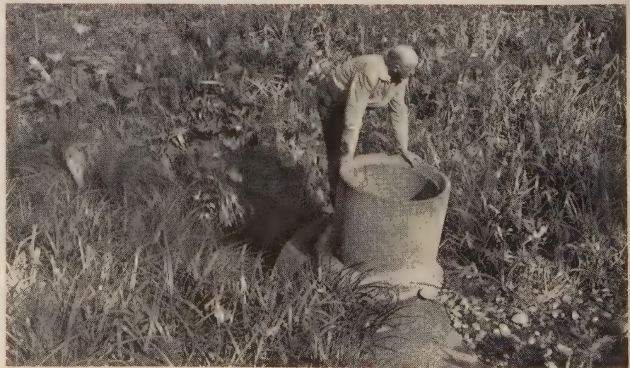
TEE CULVERTS are used to cope with debris from logging operations. When end of culvert becomes clogged, water rises in pool to upper opening. Shown is George Farquarson, maintenance superintendent at Hoquiam.
