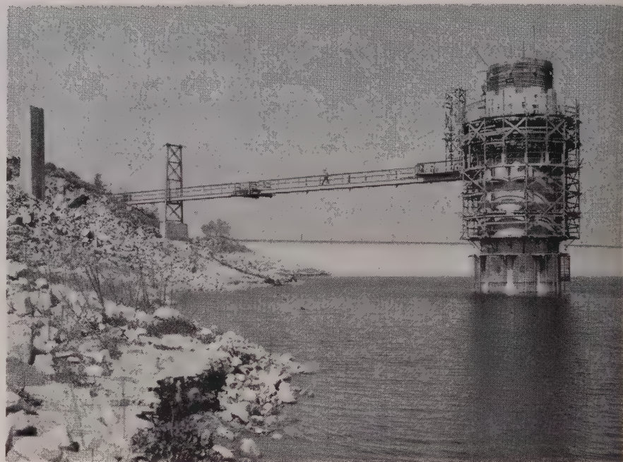
OUTLET TOWER is being raised by removing roof and extending walls. Nine more hydraulic gate valves will be installed. Note new pier at left for suspension access bridge at higher elevation.
