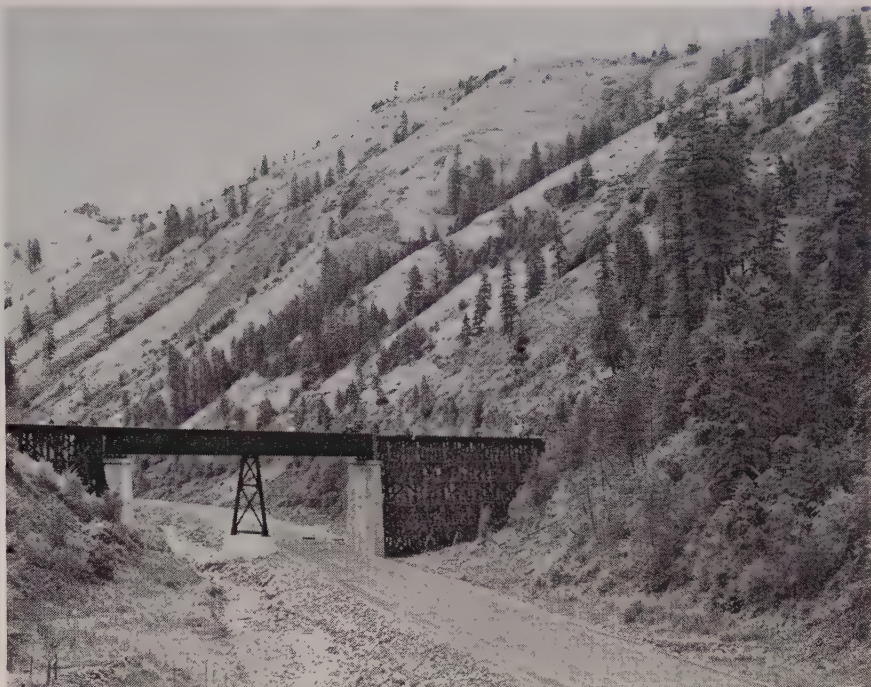
TIMBER railroad trestle, on section of completed grade, converted into underpass. Placid Lapwai Creek frequently becomes a mountain torrent, washing out temporary bridges and haul roads.
