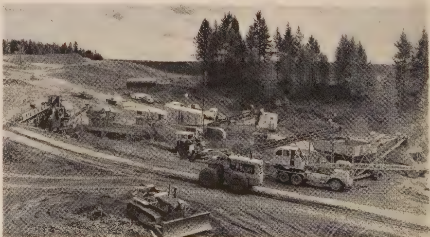
CRUSHING PLANT producing surfacing material for Grant Construction Co. paving operations. The project required 208,600 tons of base and 41,385 tons of plant mix.
