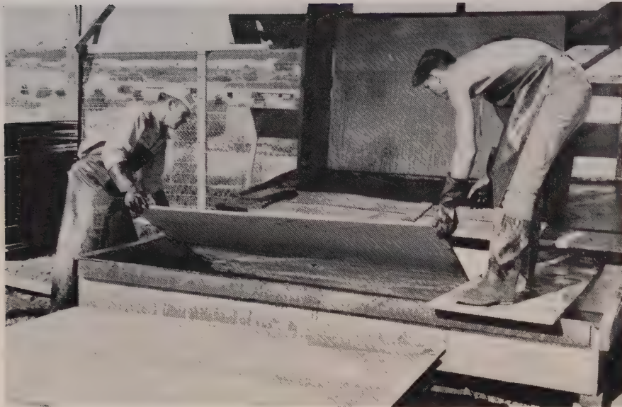
METAL trough holds coating solution in which plywood form panels are dipped. Wet panels stand on notched rack, rear, to drain. Process is five times faster than old method.
