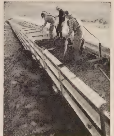
Tamping fill material in bins provides necessary stability.
