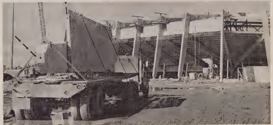
PRESTRESSED CONCRETE sections numbering about 1,600 were used in the grandstand. Arrows show precast ducts in the spandrel and main columns through which tendons were threaded.
