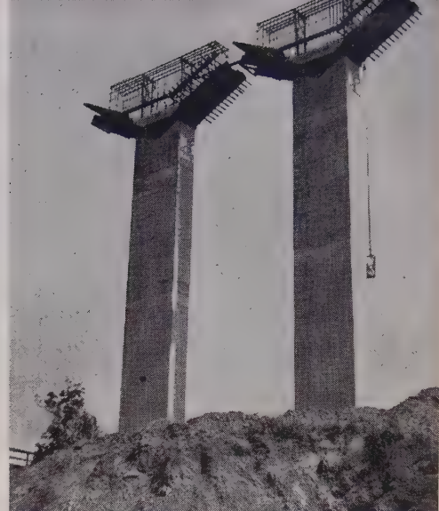
LAND PIER caps formed without falsework using steel frames bolted to stems.
