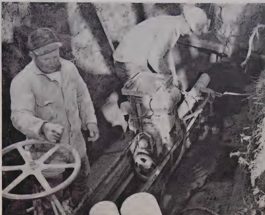
IN OPERATION , the drill is advanced by turning on the tractor steering-wheel, as shown. Water is pumped into the drill head to remove cuttings.
