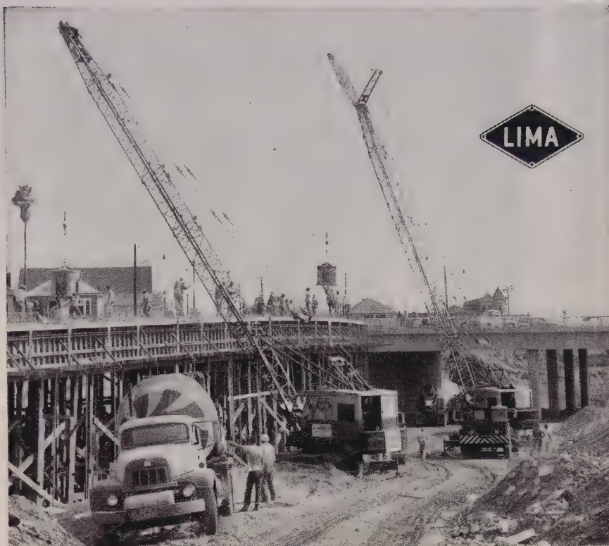
California's Golden State Freeway construction is speeded as two Lima truck cranes pour concrete on 1¼-mi. section near Los Angeles.
