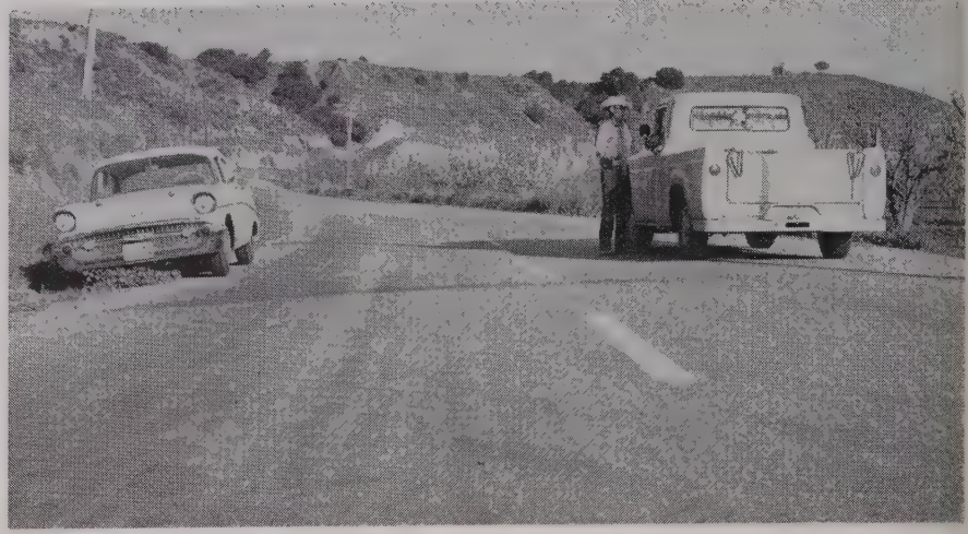
COUNTY road paved with heavy single armor coat of MC-5 at .25 gal. and crushed screenings at 28 lb. per sq. yd. over a regular MC-1 or MC-2 seal coat.
