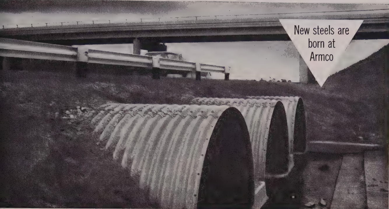
Three lines of Armco MULTI-PLATE® Pipe-Arch provide waterway for creek crossing new relocated freeway in Ohio.
