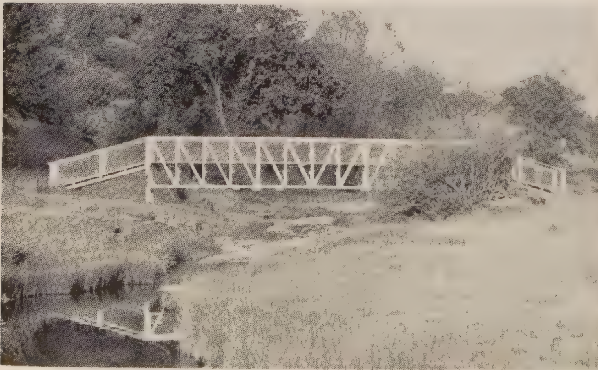
FOOTBRIDGE made of boxcar sideframes welded to form through truss. Road Department builds these in isolated locations where traffic doesn't justify a highway bridge.
