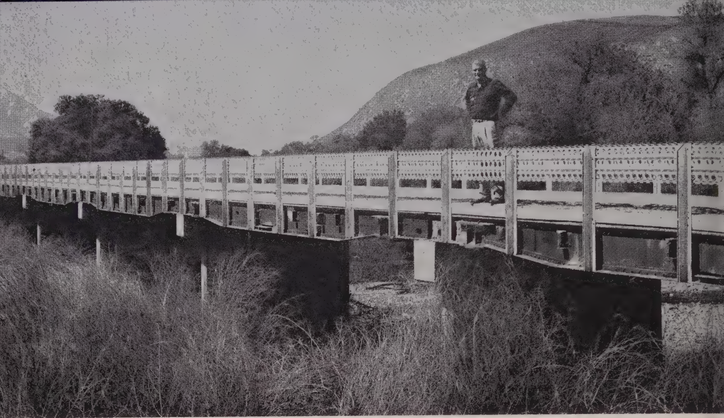
BOXCAR bridge uses steel underframes on concrete piers to support a concrete deck. Railing is made of surplus landing mat.
