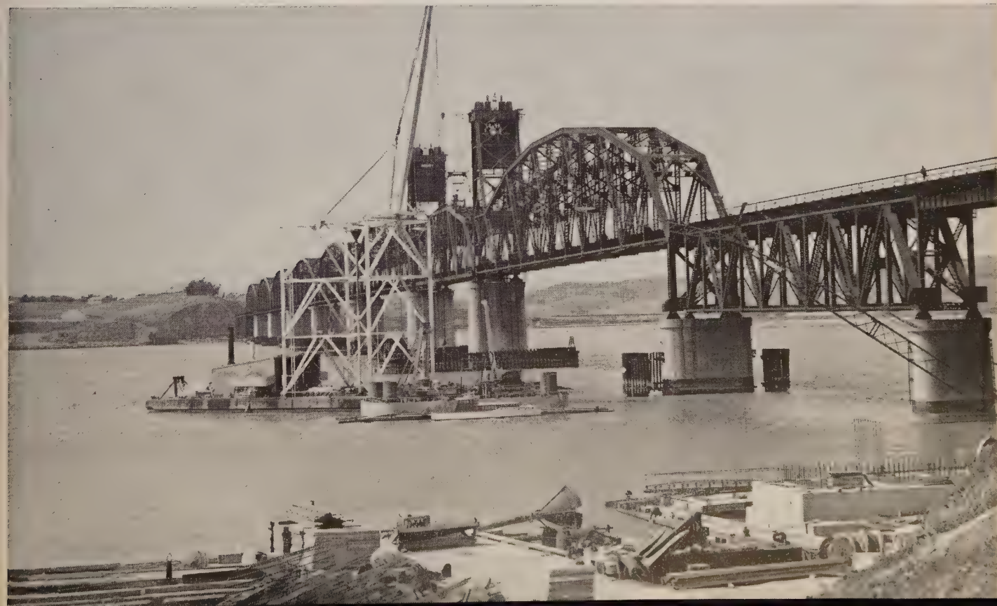
BRIDGE site from Benicia shore shows giant tower crane moored beside first floating footing. Contractor's work dock and conventional bridge
