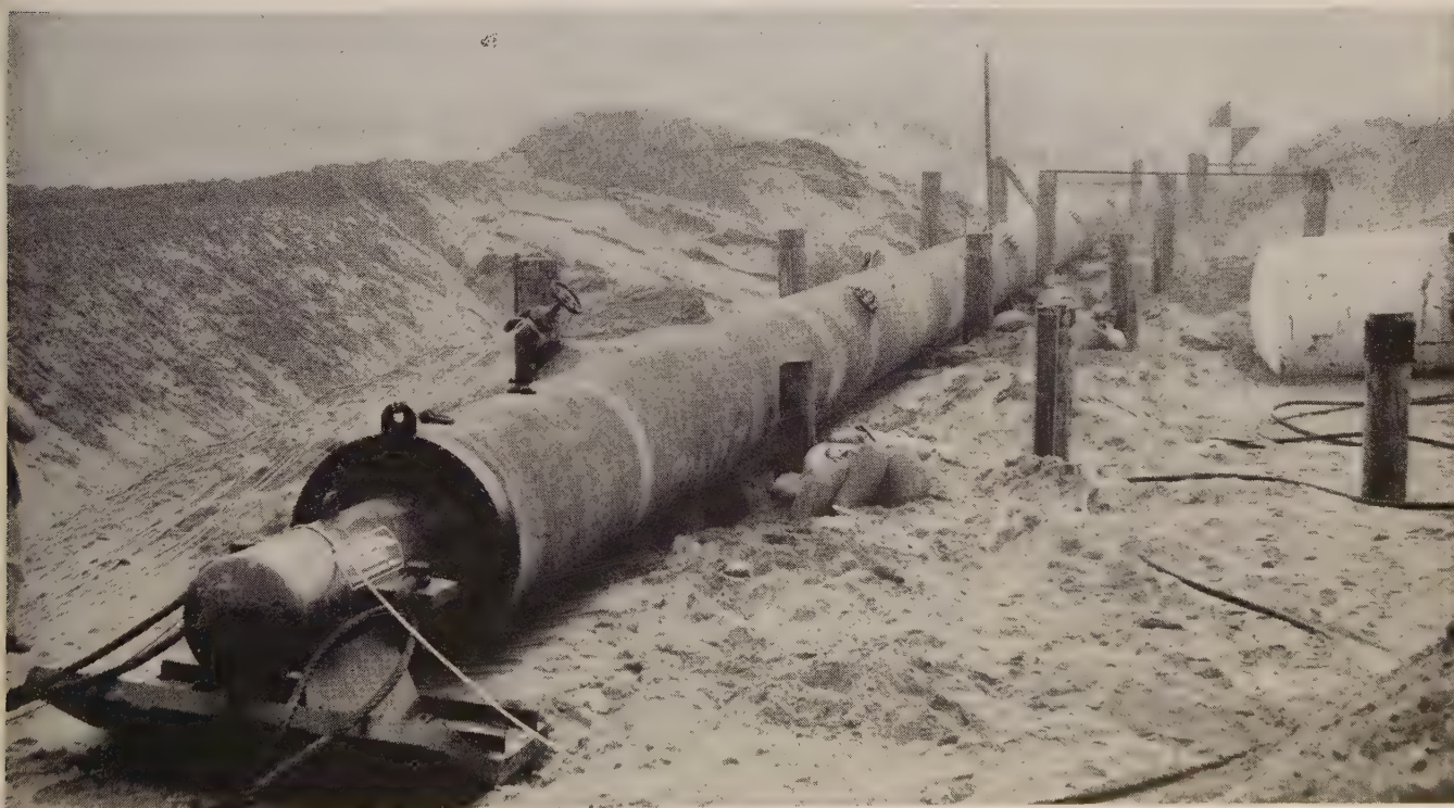
PULLING head attached to front end of pipe ready for the trip through the surf. Pipe travels over rollers set between each pair
