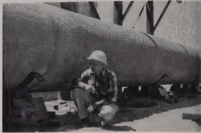
ROTATION of pipe during welding was done with curved plates made of two pieces of steel with grease between them.
