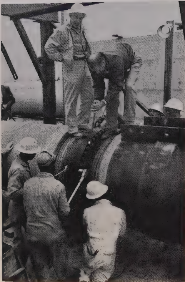
SUPERINTENDENT Ted Nielsen and co-owner Pete Price atop pipe check bolts on completed joint. Steel sleeve will be slipped over joint.
