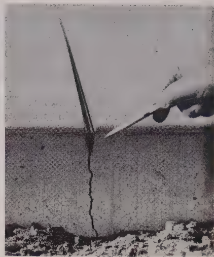
CONTROLLED CRACKING of slab with metal insert shown.
