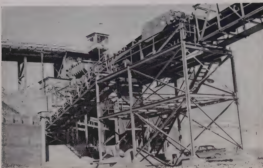
LOADING STATION on the 4,300-ft. conveyor. Oversize is scalped off and wasted. The control tower located above the plant has a closed circuit TV which permits the operator to observe the loading of the belt and the discharge.
