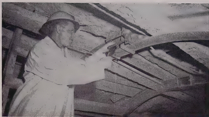
LINE being established on a roof scale near the bottom of the shaft. Transits took their line from the "sway scales" of the plumb-bob wires and projected it to this scale about 375 ft. into each heading from the center of the shaft. A series of 20 readings on each roof scale constituted a "run."
