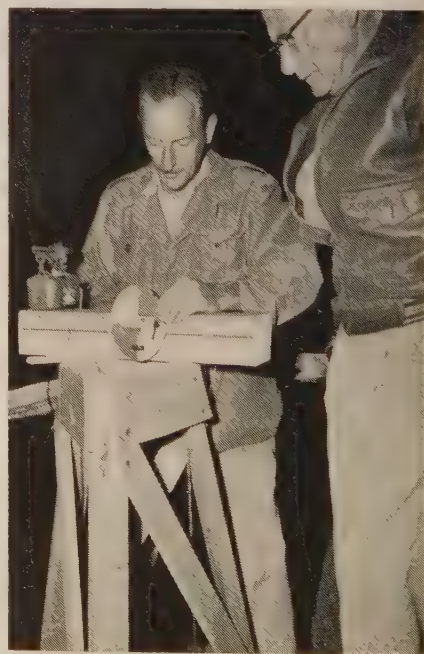
MICRO ROD illuminated for establishing points on the tunnel tangent line over the Continental Divide.
