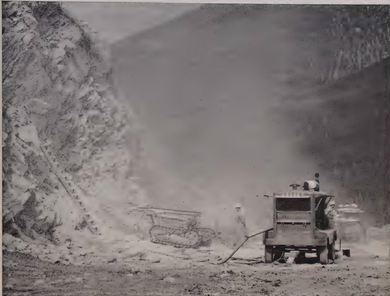
TOUGH ROCK. On this Rocky Mountain excavation nearly all of the rock was badly fractured and schisted as well as being highly abrasive.
