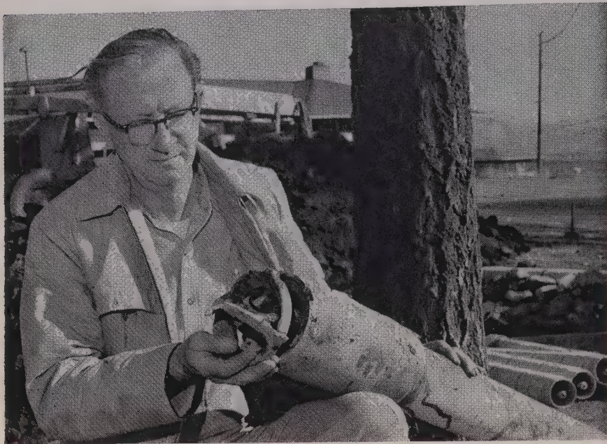
MAURICE GUNDERSON, project manager for the South Suburban Sanitary District, examines a drill removed from its metal shield. Unit has a slightly larger diameter than the service pipe. Design of the cutting head of the drill was the key to this time-saving process.
