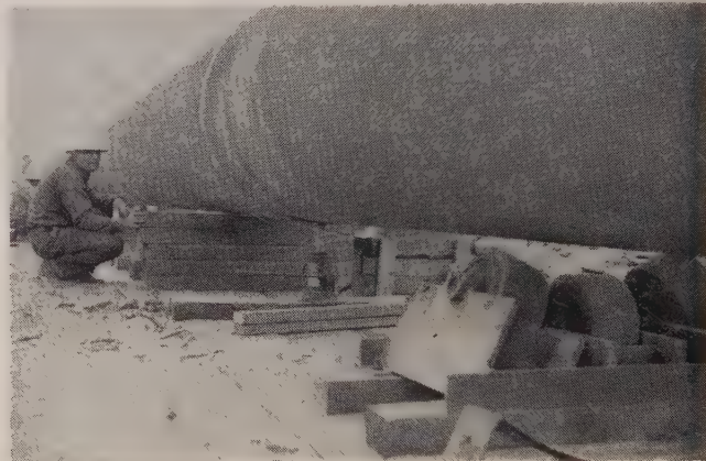
PIPE string from storage bed is lowered on to roller track. Jack, center, supports 200-ton pipe while short timbers are withdrawn.
