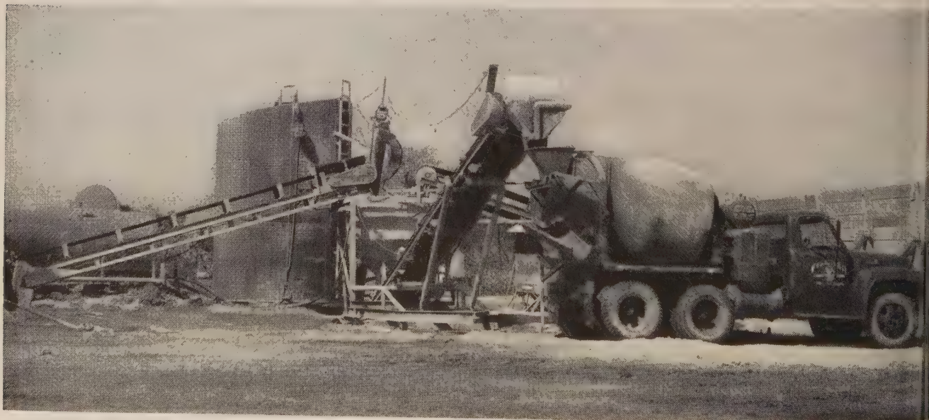
This C.I.T.-financed ready-mix plant made it possible for the Fischer Construction Company to do on-the-job casting of over 12,000 lineal feet of piling.
