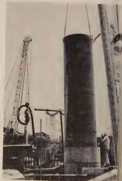
CAISSON shell suspended from derrick barge slides inside drill casing, which will be withdrawn.
