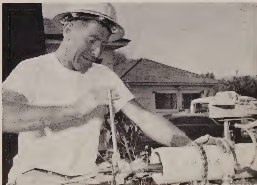
LOCKING ON another section of pipe, and extending the drilling shaft. In ordinary soil the drill placed a service pipe under a 25-ft. street width in about 1/2 hr.
