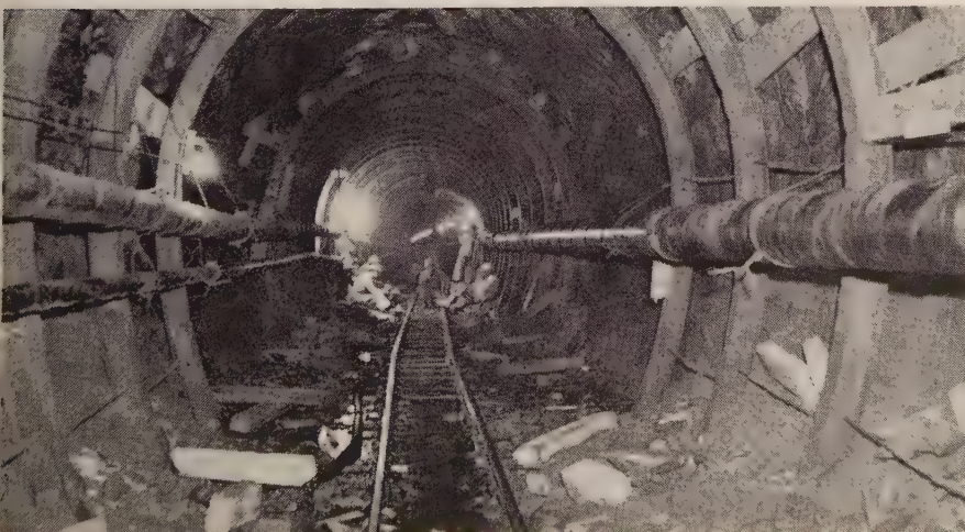
HOLING-THROUGH station (Sta. 712) in the east leg of the tunnel. Note the flat angle in the tunnel track at this holing-through point.
