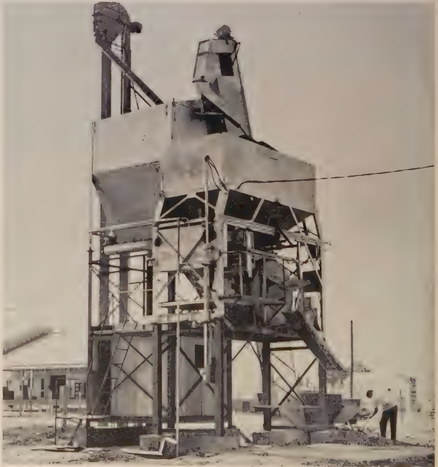
BATCH plant measures and mixes concrete in 1-yd. batches for small contract jobs and week-end do-it-yourself patio and driveway builders. Built for Trail-A-Mix Co. in Scottsdale, Ariz.
