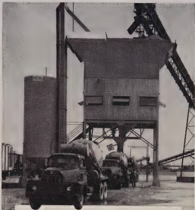
Savannah, Georgia: Heltzel 200-ton, five-compartment, portable combination bin with sealed cement compartment. Set of 7 cubic yard split batchers. 609 bbl. portable recirculating cement tank. 250 bbl. per hour cement elevator. Undertrack screw conveyor.
