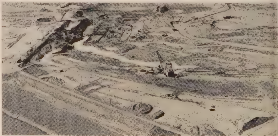
AT Wanapum Dam site a large yardage of preliminary excavation is required. In the center of the photo is a Monighan dragline with 17-yd. bucket excavating in the powerhouse section. About 600 men are employed by the contractor, Grant County Constructors, and this number is expected to more than double by the end of this year. The dam is being built 6 mi. below Vantage, Wash., on the Columbia River.
