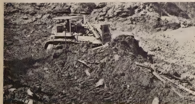
33% more production! Overburden, running to 60', is blasted and then cleared by a D9E. Owner: McCoy Coal Company, Gorgas, Alabama. 1,800,000 yards is moved to mine 150,000 tons of coal per year.
