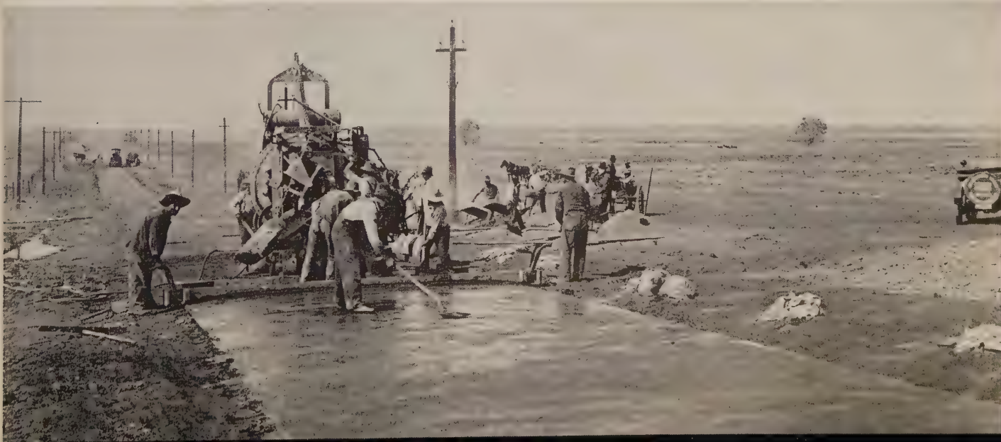
CONCRETE paving train finishes road across the Central Valley about 1914. Aggregates were fed to the mixer by wheelbarrow, and bagged
