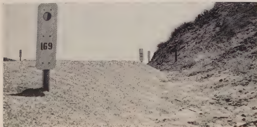
RETARDING element is heavy depth of pea-gravel.
