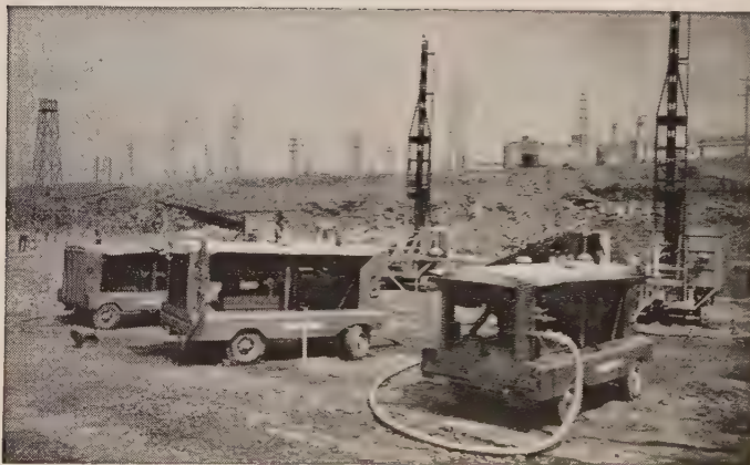
Gardner-Denver RP900 rotaries provide power for 5½" drills on Niagara power project.
