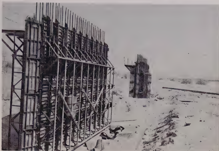
TWIN BRIDGES 1,006 ft. long carry roadway across Mojave River, which flows underground most of the time. Steel forms for piers were originally built for channel lining work.
