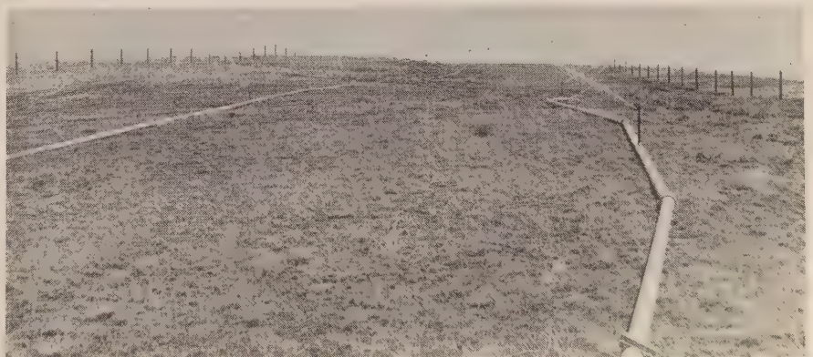
PRE-WETTING MATERIAL with a 2-line layout, using 60-ft. spacing and sprinklers at 20-ft. intervals. Aluminum pipe is 6-in. size. Operating pressure is 35 to 45 psi.
