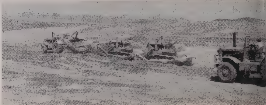
PREWETTING borrow pits makes excavation easier but tandem pushing is still needed. Ten crawler tractors and twenty earthmovers work two shifts on 2,200,000 cu. yd. of excavation.
