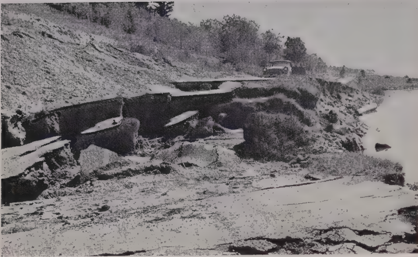
HIGHWAY 287 along the reservoir behind Hebgen Dam. Sections of highway were literally shaken to pieces, and several faults showed displacements of 9 to 10 ft.
