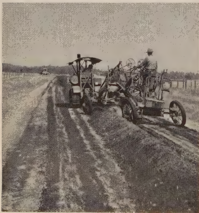
PAVING project in Amador County, Calif., in 1927. Here a crawler-drawn grader windrows road mix. Operator works 8 hand controls and has no power steering.
