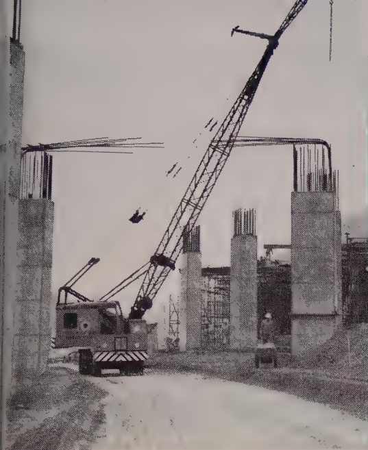
Overpass at Albany —Steel girders will be placed on top of these steel-reinforced concrete columns to form an overpass at Albany, California. USS Di-Lok Concrete Reinforcing Bars are used for all types of concrete work; and Universal Atlas Cement Division of United States Steel, offers a wide variety of portland cements. Tiger Brand Wire Rope is used in cranes, pavers, shovels, ditchers, trenchers, derricks, mixers and road scrapers.
