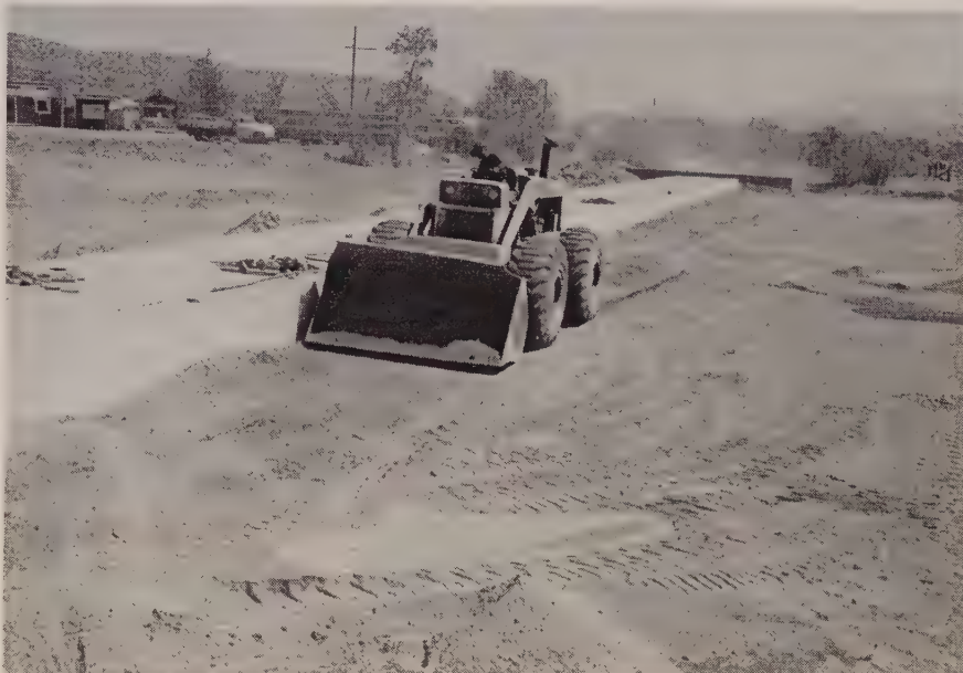
VERSATILE RIG is this Michigan 175A front-end loader, shown on structural backfill clean-up. Wide bucket permits it to work flush against reinforced concrete cast-in-place culvert.
