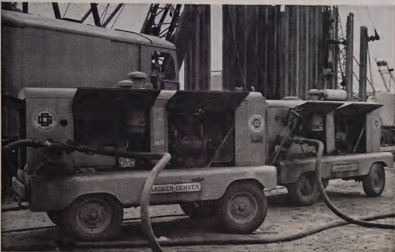
Gardner-Denver RP600 rotary portable compressors at work on sewer job.
