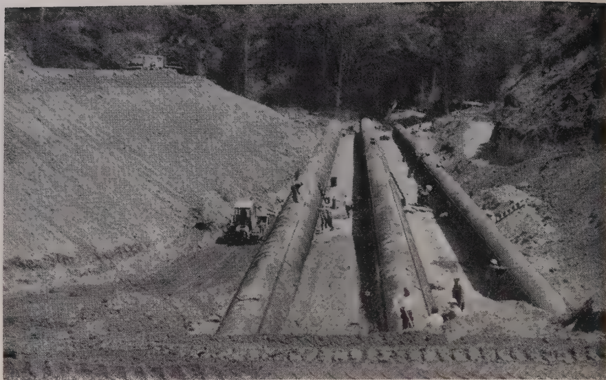
MULTIPLE culvert installation includes three 96-in. pipes to carry stream through the fill. Two of these installations were damaged by floods which bent culverts upright.
