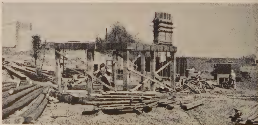
TIMBER CAGE forms template for sheet pile cofferdam driven for pier footing excavation. Piers supported on 40-ft. piling in deep gravel underlying riverbed. Completed piers in background.
