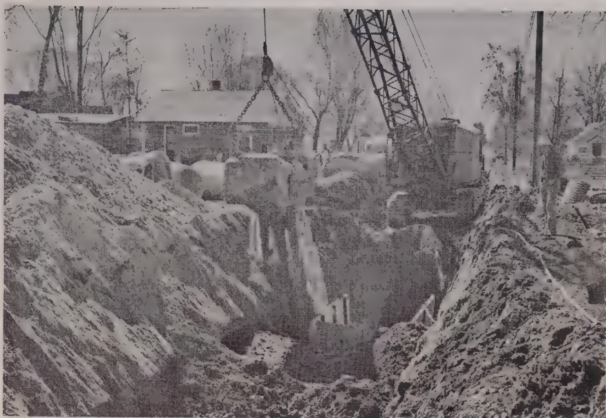
A 70-FT. BOOM on a Northwest dragline had sufficient reach to permit excavated material to be dumped back into the trench. Pipe laying was carried forward directly behind the dragline, using a protective shield for the crew, as shown.
