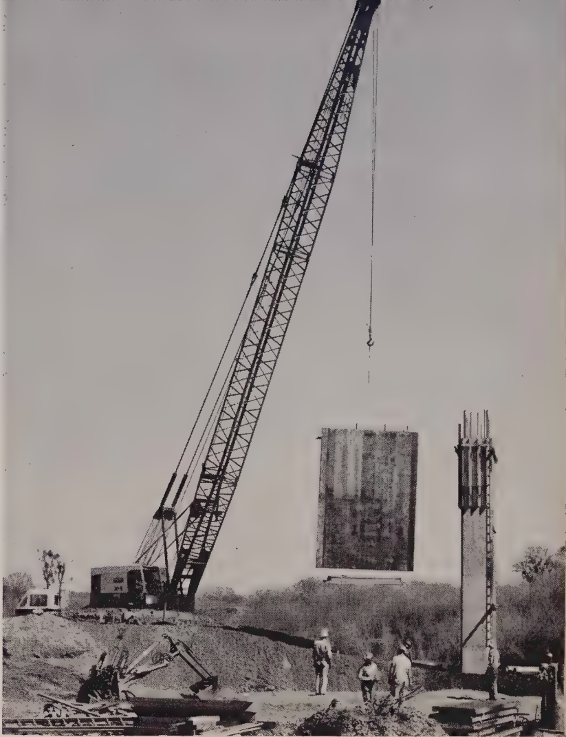
FORM panel and work platform swung away from completed pier by crane rigged with two cables. The unit is a Bucyrus-Erie 30B truck crane.
