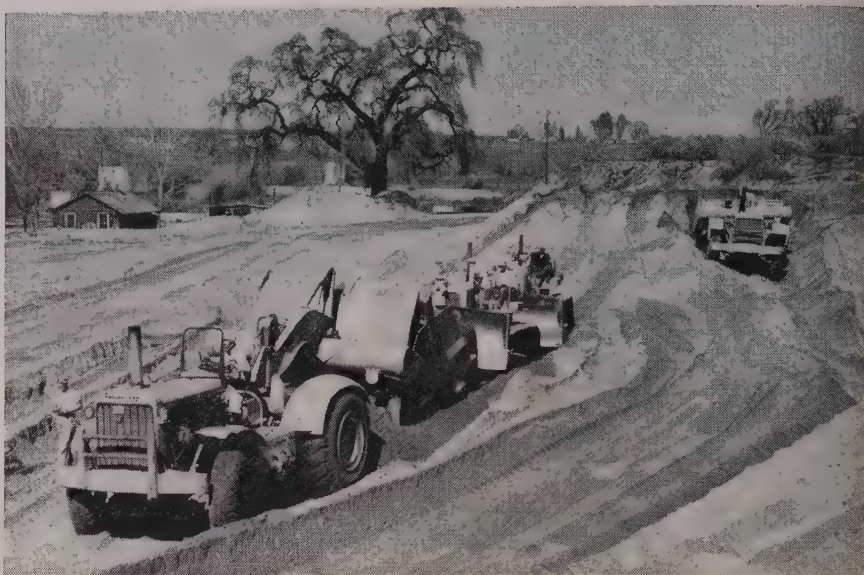
BORROW for road fill loaded from bank by Cat D8 crawlers pushing in tandem. Modified Caterpillar DW20 gets 25-ton load of fine sandy material without prior ripping.
