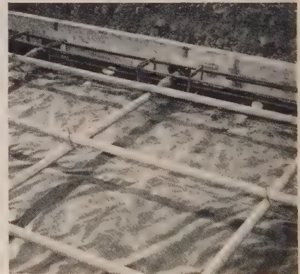
Close-up of post-tensioning tendons. Note that re-bars are only required along edges of slab at top of picture.
