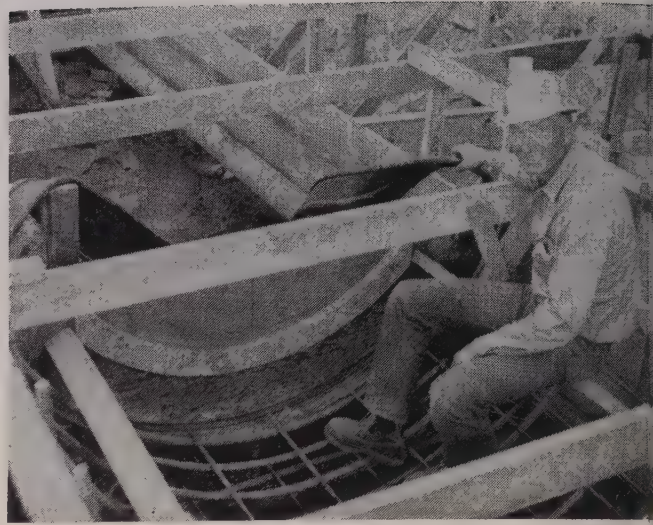
SUPERINTENDENT Arch Martin holds continuous rubber waterstop held in place by plywood template. Curved rail guides invert screed.
