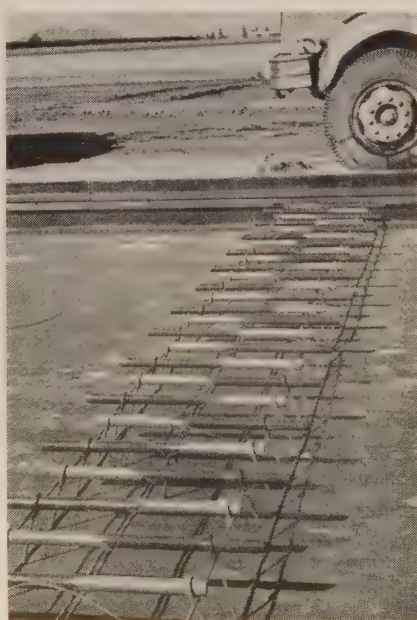
TYPICAL load-transfer dowel assembly placed at every third contraction joint in reinforced pavement.
