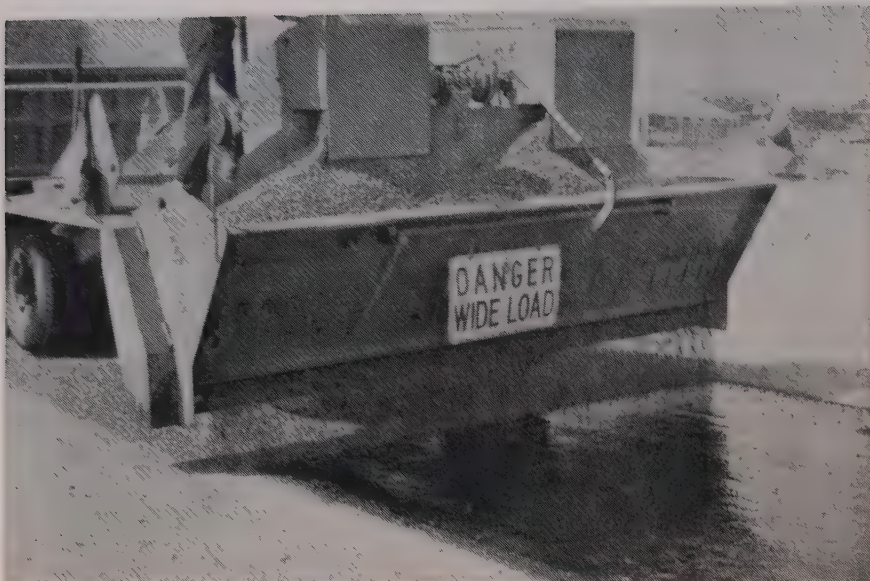
FOLLOWING immediately behind the application of the emulsion is the self-propelled Spread-master. Chips are elevated from the truck-filled hopper and feed at 18 lb. per sq. yd.
