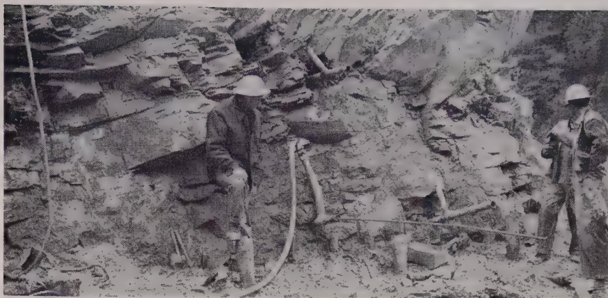
GROUTING rock bolts was needed because of seamy nature of rock. Note small pipe extending from bolt hole toward right of photo. This is vent pipe to bleed air and water from hole allowing grout to reach rear of hole. See drawing on page 50.
