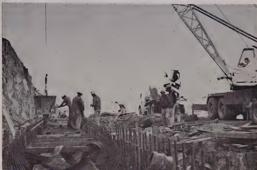
POURING invert section of outlet tube with Michigan truck crane. Transit-mix concrete is delivered with two trucks. Invert is hand finished. Note waterstop in foreground.
