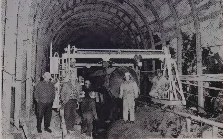
SPECIAL FRAMEWORK mounted on rails was used to carry by-pass pipe sections into the diversion tunnel and lower them into place in trench below invert. At far left is James F. Grafton, resident engineer, with chief assistant Jack Monarch.
