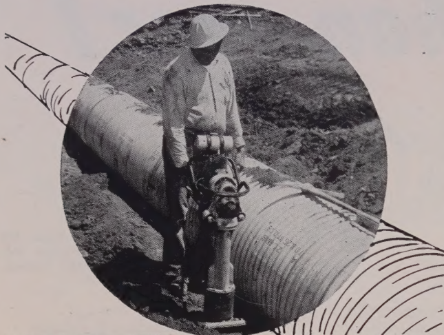
GVR 100-C RAMMER — Weighs only 115 lbs. Lightest weight Rammer on the market BUT delivers more compaction than any other compactor POUND FOR POUND OF MACHINE WEIGHT. Designed for use on heavy soils including clay.
