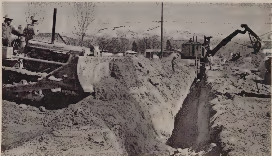
MORE CONVENTIONAL was the third method, that used a Northwest backhoe for excavating the trench and piling material along the side, where street-space permitted.
