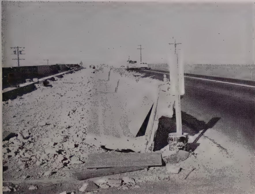
SECTION of sidewalk and railing tipped over from its original position onto the new addition and ready to be removed as a 40-ft. unit weighing 15 tons.
