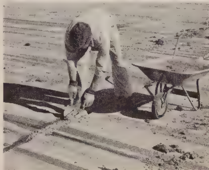
Economical repairing of spalled concrete joints by simple troweling-in of CONCRESE mortar, followed in hours by saw-cutting to receive sealing compound and free slabs.
