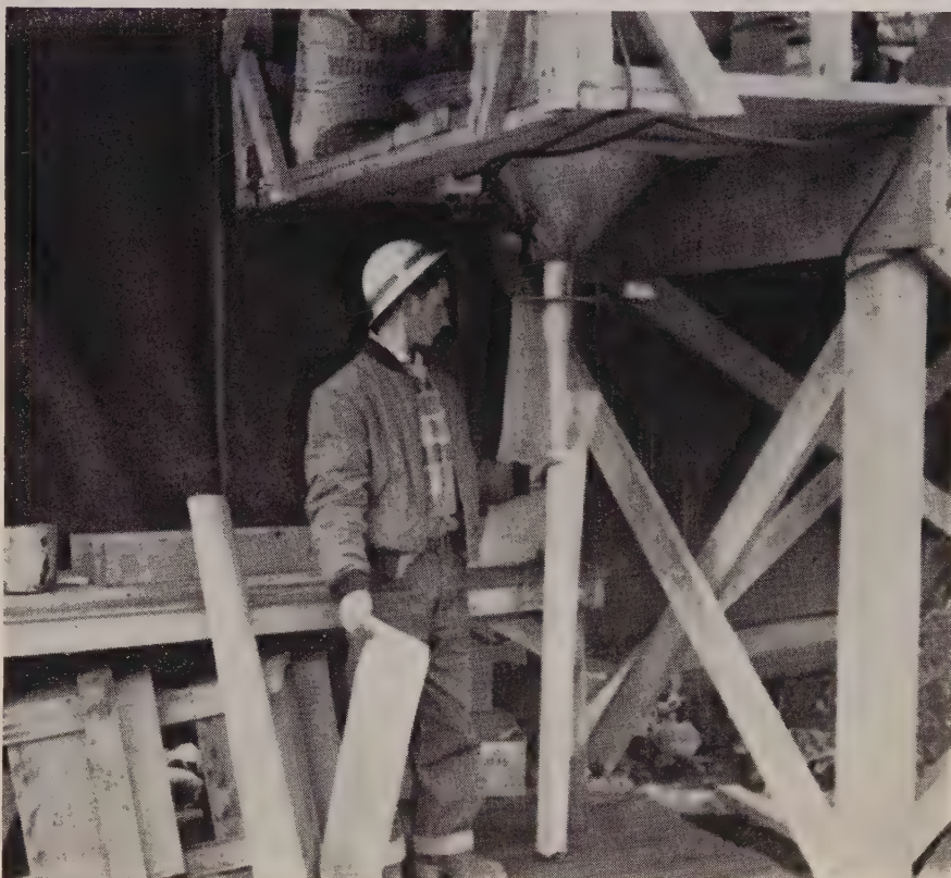
BLASTING with ammonium nitrate in wet ground required packaging nitrate in bags. Inner bag is plastic, for waterproofing, outer bag is heavy paper to resist puncturing. On upper platform is mortar mixer in which nitrate particles are coated with diesel oil.
