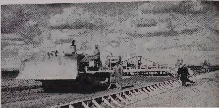
FORM-riding planer leads the paving train. It trims base course to 1/4 in. above grade prior to windrowing and cement treating.
