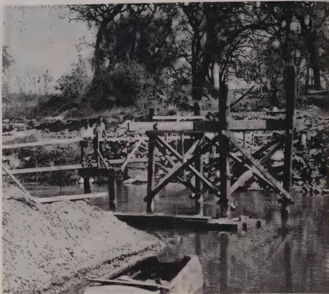
TEMPORARY piling in channel will support timber cage on projecting beams. When sheet pile is in place, interior timbers will be removed.
