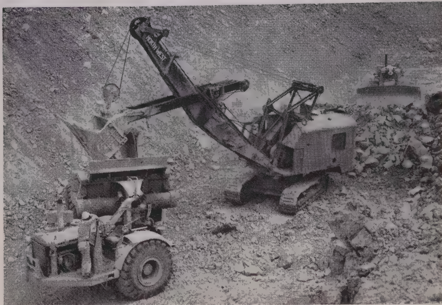
LOADING in the rock cut was done by Northwest 80D; using a fleet of DU21-PR21 tractor-rock wagons for hauling. Most of the material was wasted. The D8 is used for cleanup work.
