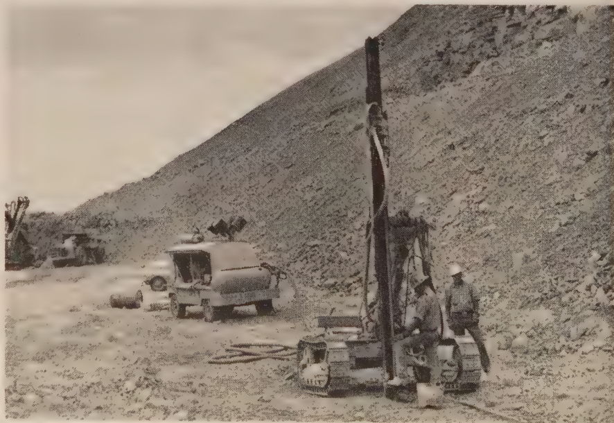
CRAWL-I-R powered by an Ingersoll-Rand compressor drilled 3-in. holes from 10 to 30 ft. deep. Blasting was done by ammonium nitrate.
