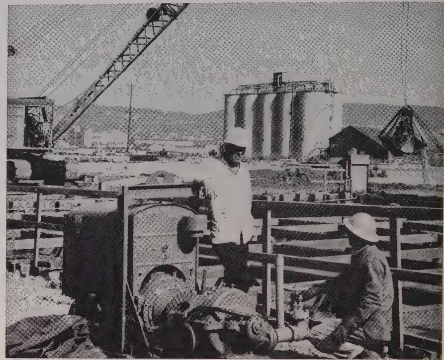
DIVER Dick Clements, right, and John Bugbee, field engineer, check high pressure pump which will power water hose to clean sides of cofferdam before placing 4-ft. concrete slab floor.
