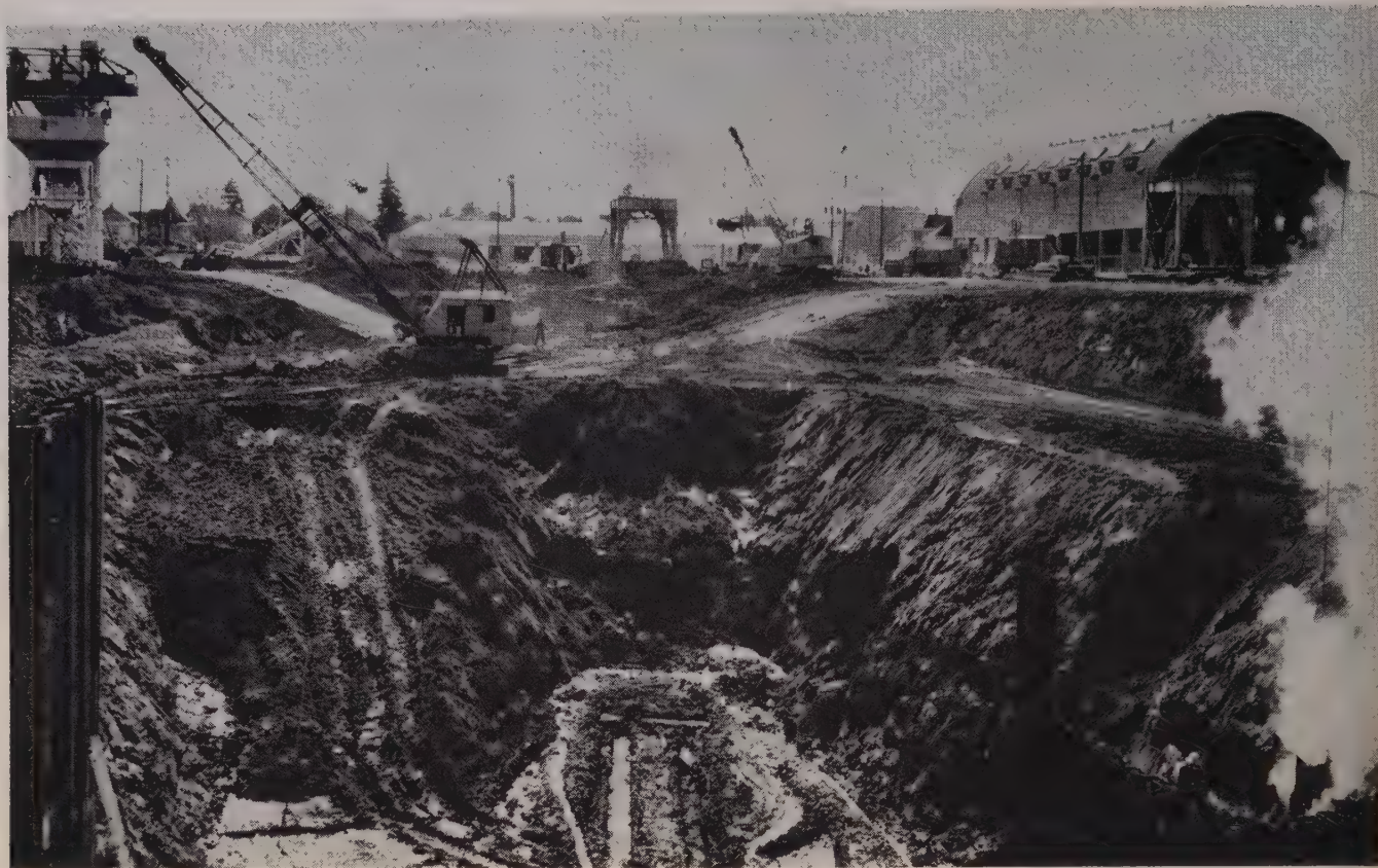
EXCAVATION for drydock where huge tube sections will be cast seen from gate end. Sheet piling being driven for gate portal in fore-
