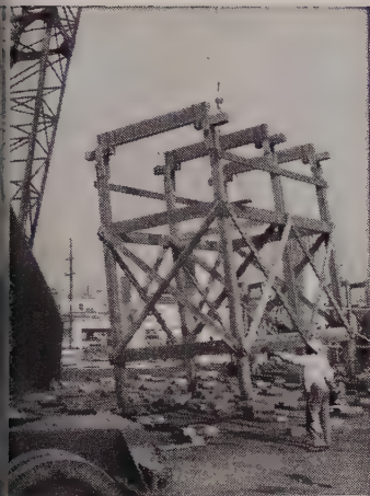
In carefully planned sequence of operations, prefabricated shoring towers were positioned, screw-jacked to required height. Deck form sections were then crane lifted into position.
