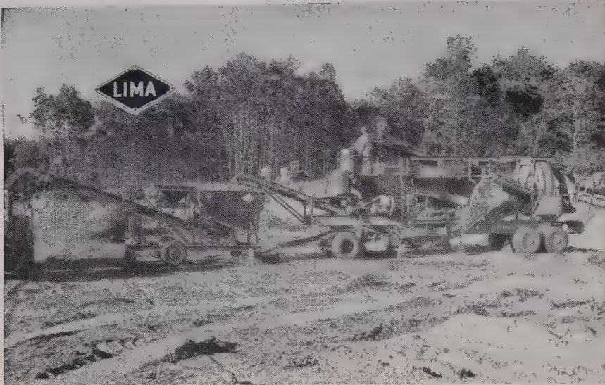
Portable Lima Austin-Western 101-SE crushing plant spews pit-run stone and gravel into mobile surge bin.
