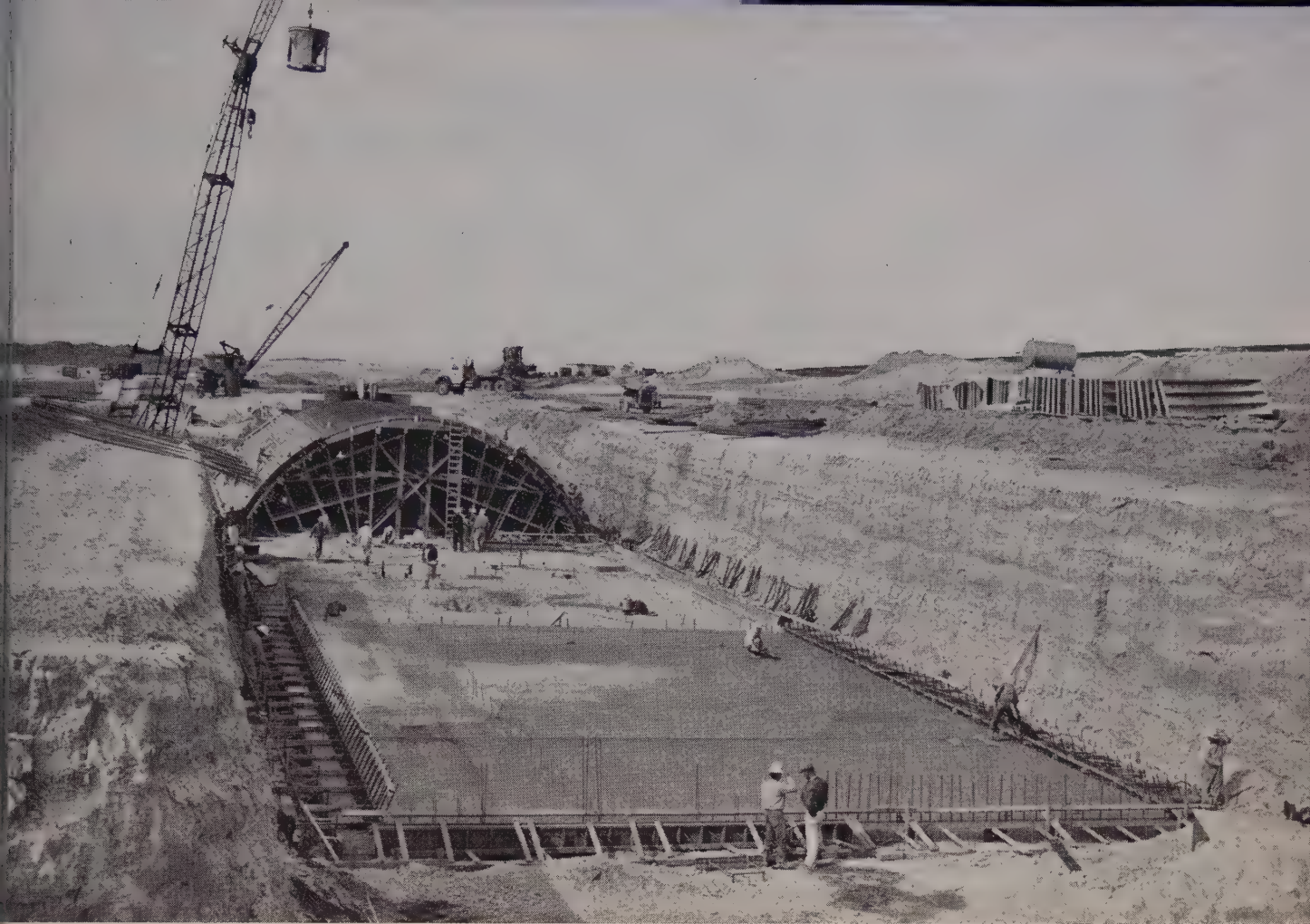
COMMAND CONTROL CENTER is under construction. Floor slab is being finished in foreground while roof concreting is carried out in
