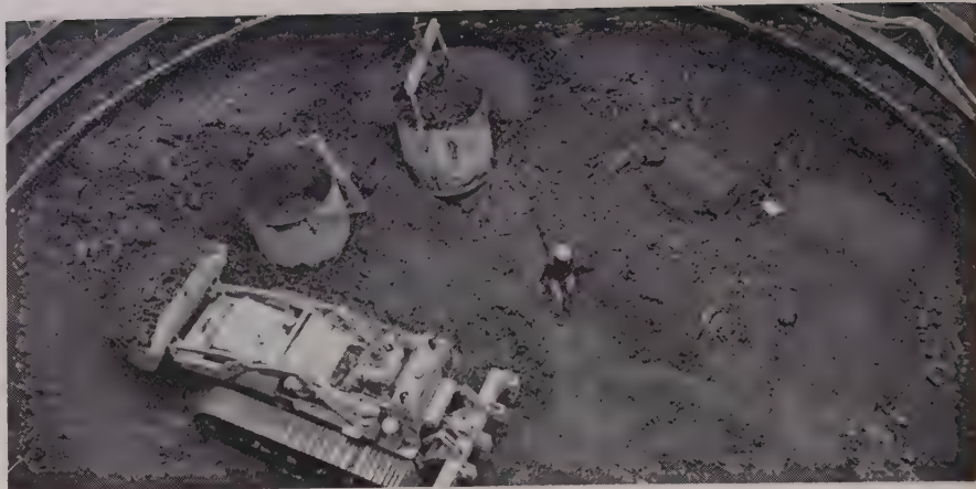
EXCAVATION OF SILOS was done with front-end loader. Crane at surface removed one bucket of material while other was being loaded. Hand tools were used at periphery to minimize over-excavating. Walls are lined with mesh, steel rings, and gunite as excavation is under way.
