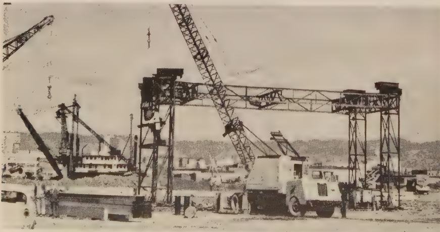
LIFT BRIDGE designed by contractor to speed passage of barges through channel which will be dredged from estuary to portal. Tube sections will be floated into channel and sunk.
