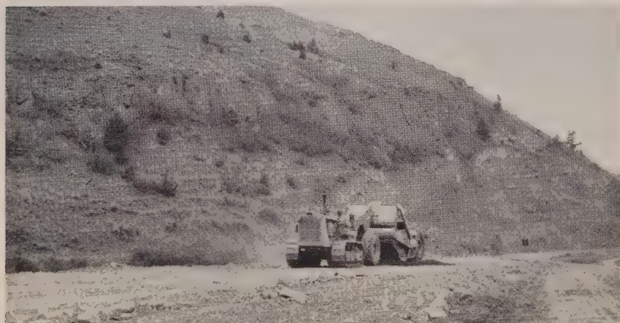
ROADBED material was spread by D8 Tractor-80 Scraper combination. About half of the base course gravel was spread last season.
