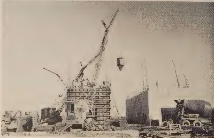
WALLS of the two cells, each requiring more than 200 cu. yd. of concrete, were poured in one continuous 10-hr. pour. Cells are 106 ft. long and 22 ft. wide.
