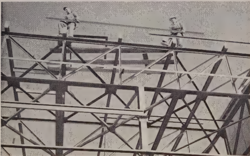
STRUCTURAL STEEL frame of the engine service building is supported on its own foundation and has no common wall with the test cells.
