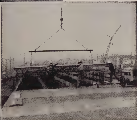
In carefully planned sequence of operations, prefabricated shoring towers were positioned, screw-jacked to required height. Deck form sections were then crane lifted into position.
