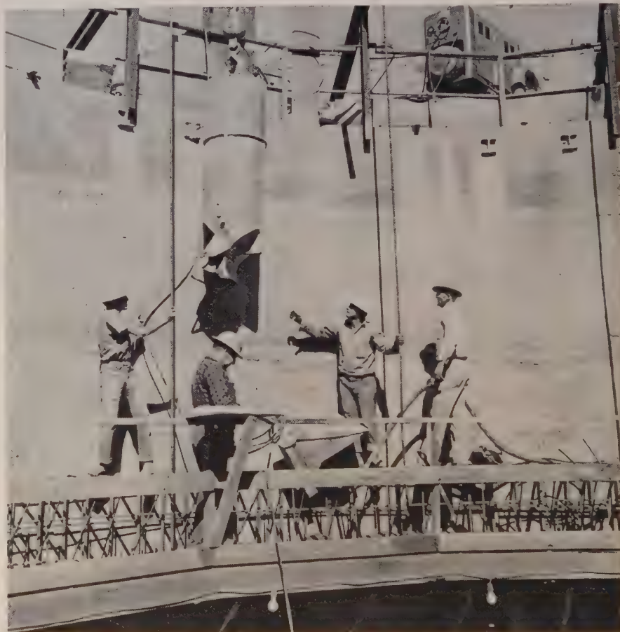
SLIP FORM advanced about 8 in. per hour. Transit mix trucks brought concrete to site where it was transferred to small diameter buckets for placement in form. Scaffold suspended beneath concrete placement level is used by finishers. Note 1-in. rods, suspended from I-beams, up which the form travels. See also cover photo.
