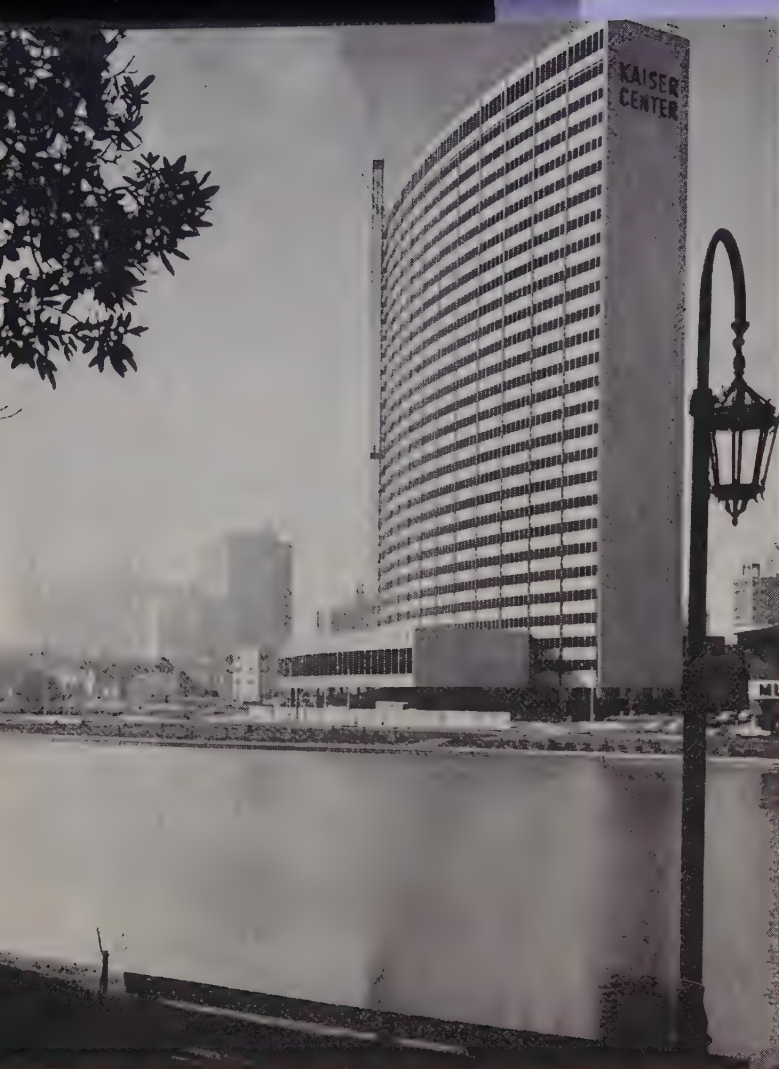
GRACEFUL curving front of Kaiser Center on the shore of Oakland's Lake Merritt. The 28-story, 390-ft. office structure has gross area of 976,000 sq. ft., making it the largest building west of Chicago. Curtain walls use 1,230,000 lb. of aluminum. Extension in front houses cafeteria and auditorium.
