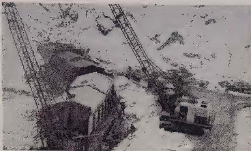
FIRST BLOCKS of Junction Dam are under construction in a cold-weather concreting program by contractor Fruin-Colnon. The dam will be a concrete arch 170 ft. high, 520 ft. long at crest.
