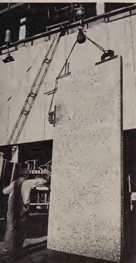
FAST concrete-dolomite panel weighing 1 ton hoisted into position on building end-wall. Panels are mounted singly to permit individual movement. Window walls use gold-anodized aluminum and glass tinted gray to cut down glare.
