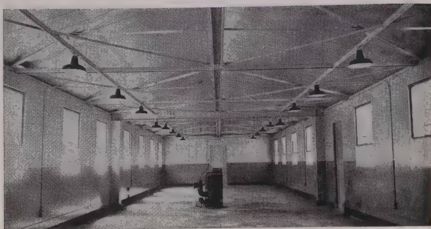
INTERIORS are completely finished in plywood nailed directly to the panel ribs (see drawing). This enables the panel walls to be dismantled in sections. Mild climate does not require insulation.
