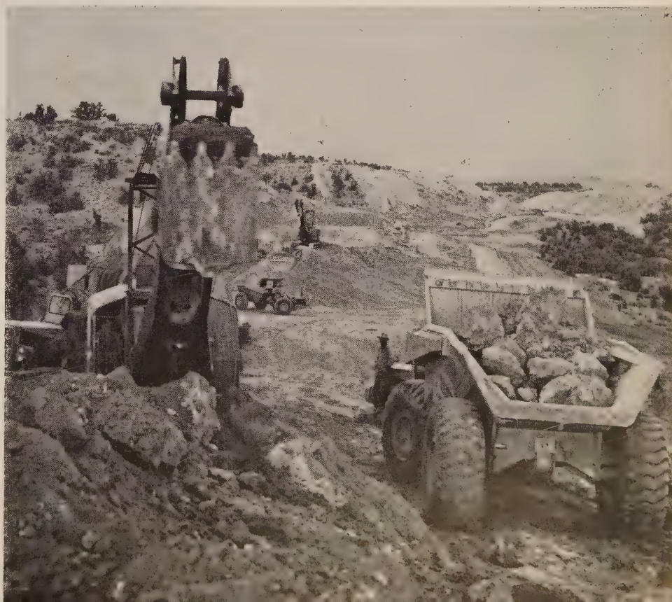
SHOVEL SPREAD develops cuts for new alignment. Earth and boulders are sandwiched in between strata of limestone.
