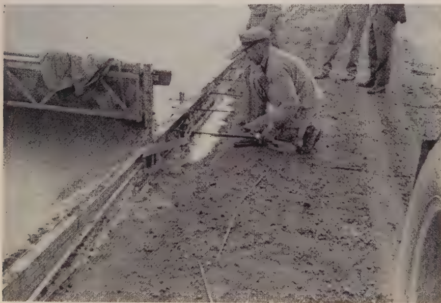
DOWEL BARS are inserted in slot near end of trailing forms by workman with hollow tube of proper length. Bars pass through holes in keyway blockouts which will be removed later. Tubular steel framework keeps trailing forms at proper width and carries burlap drag.
