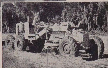
FLORIDA —Galion T-500 Grader working on construction of Route #1.
