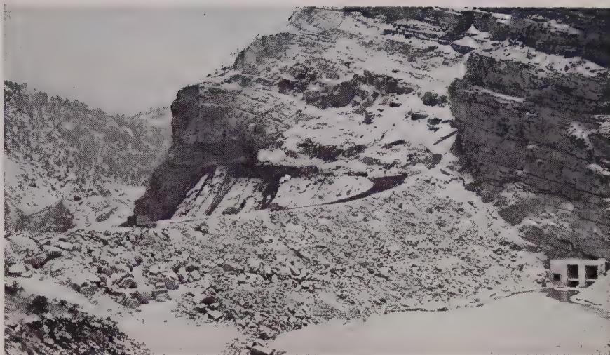
DIVERSION DAM AT FLAMING GORGE PROJECT IN NEW MEXICO Upper cofferdam, at Flaming George Dam project, looking downstream. It is approximately 85 ft. in height above river level, 500 ft. in length and 350 ft. thick through base. Note intake structure of diversion tunnel in lower right. Right keyway (being excavated) for Flaming George Dam is in upper center. An extended review of construction operations appeared in WESTERN CONSTRUCTION , Dec. 1959.
