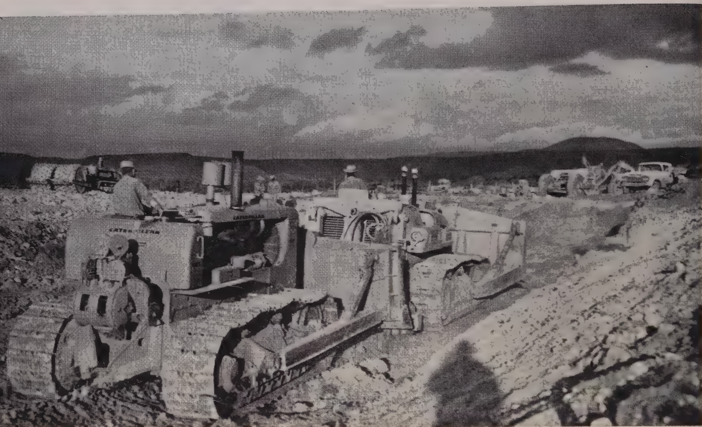
MIGHTY ripping team is composed of Euclid TC12, in front, mounting two ATECO rippers, pushed by Caterpillar D9, working in limestone.
