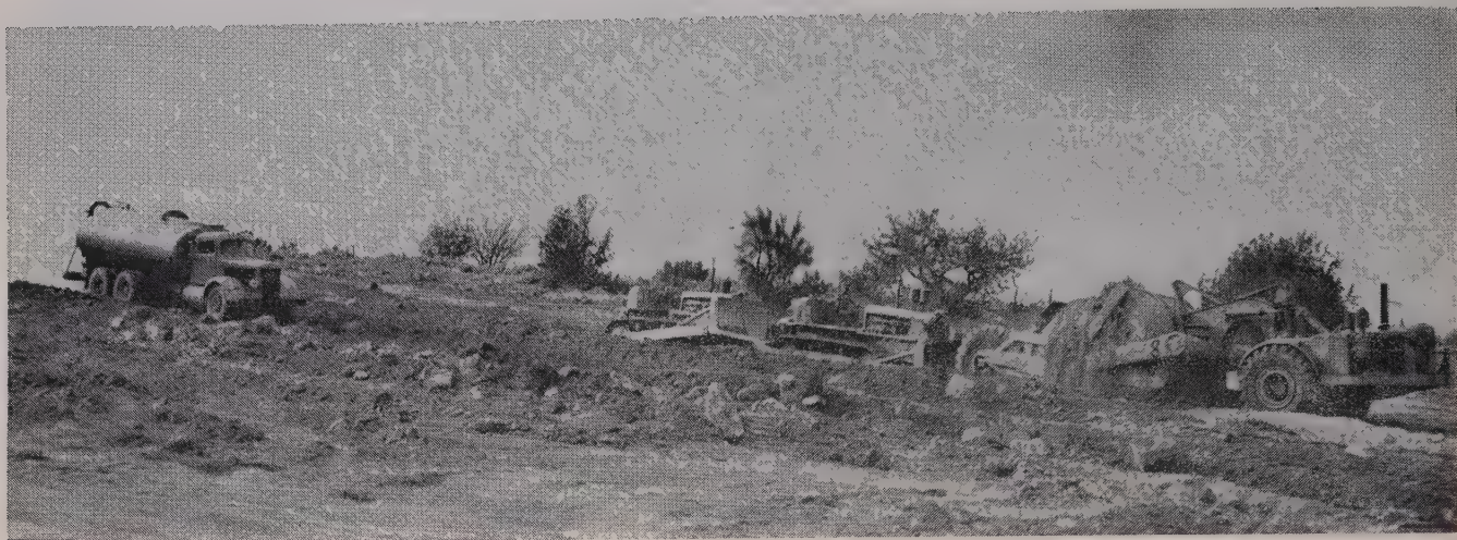
WATER truck sprays cut as tractors double-push scraper. Material is so dry in Arizona that cuts are customarily watered before and during
