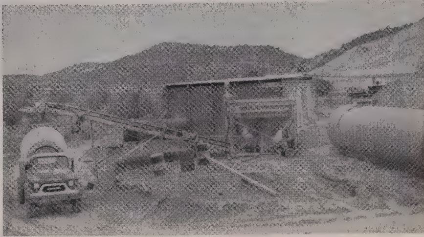
SMALL BATCH plant furnishes concrete for crossing structure at remote location. Hopper, center, is charged with dry materials by loader and belt loads transit truck.
