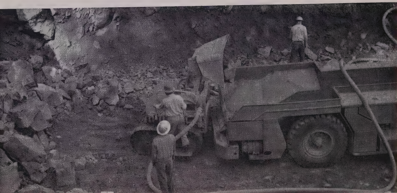
RUBBER-TIRED shuttle cars show up in this view of mucking operation during portalling-in. Fast-acting Joy JSL7 mucking machine is throwing
