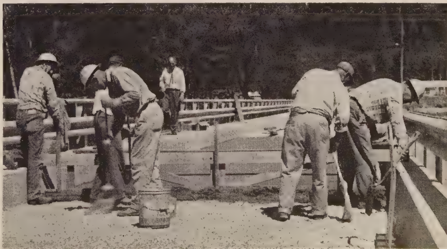
SKAGIT RIVER BRIDGE. Brushing liquid epoxy adhesive over sound concrete just prior to application of fresh concrete overlay. New concrete is bonded permanently to old concrete. Application of adhesive and concrete topping was made in 3 hr.
