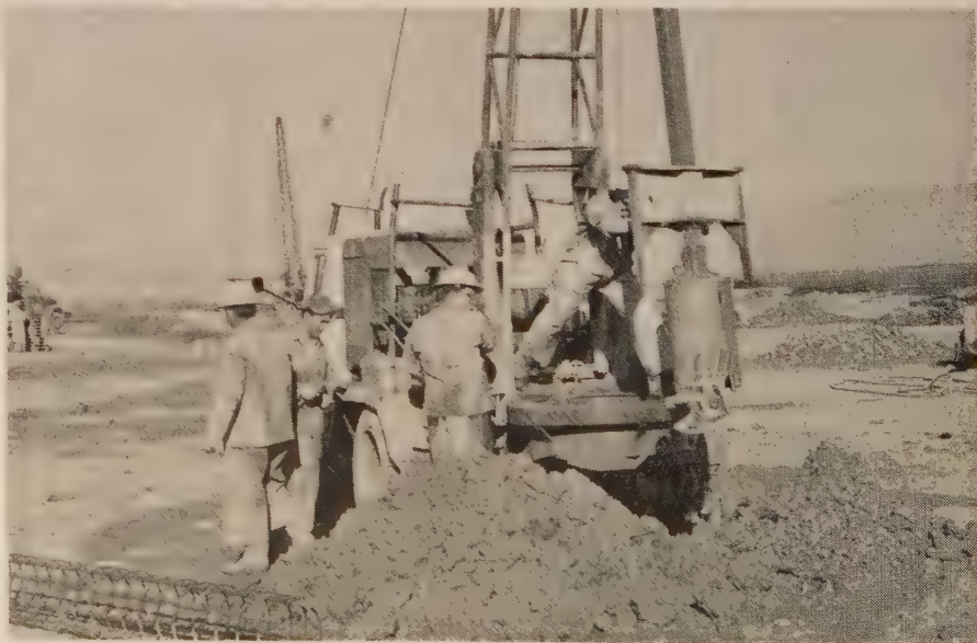
DRILLED caissons went down 31-38 ft. and had to be cased because of high ground-water.
