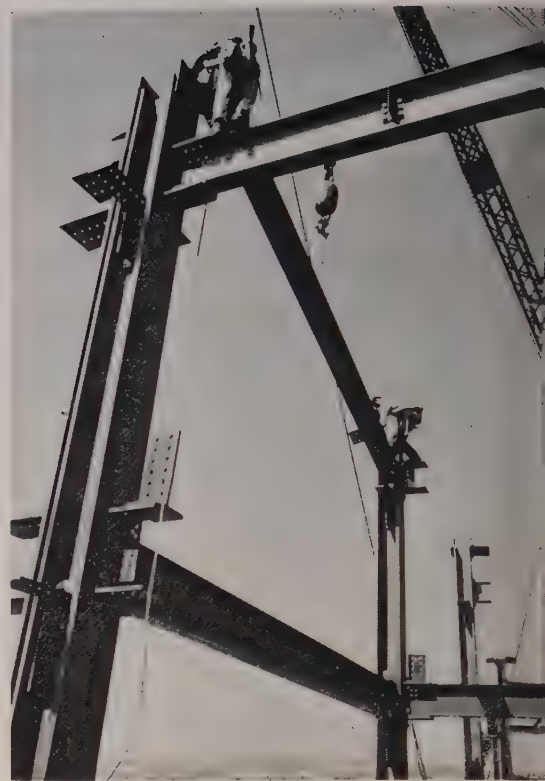
BOLTED steel framework was erected at a rate of more than a floor a week. Building was topped 10 months after foundation was placed, using record 13,400 tons of structural steel. Horizontal members were carefully cut to fit prism-shaped bays of curved structure.
