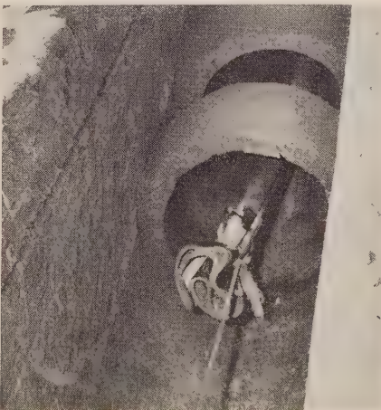
COLLAPSED form is pulled out of pipe with nylon rope and motor patrol 2 hr. after placing.
