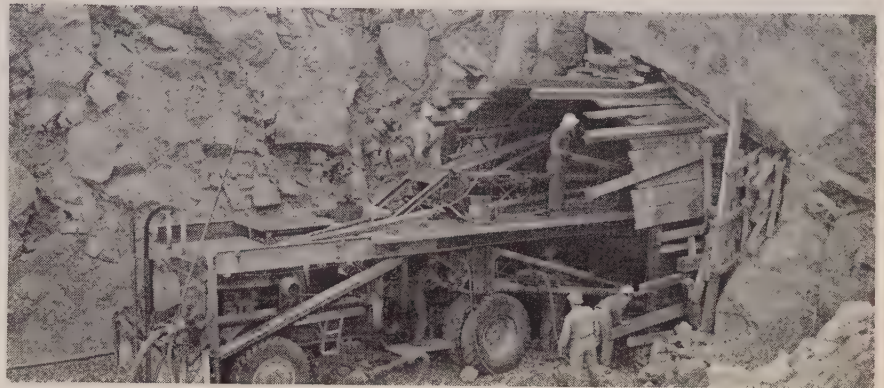
TWO-LEVEL JUMBO , shown at portal, was built from Euclid truck. Each of two jumbos mounts five Gardner-Denver 93 drills and a G-D 43 burn drill for 5-in. burn hole in center of pattern.
