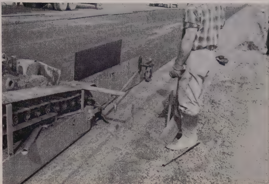
PLUMB BOB suspended over string line enables paver operator to keep machine on course. Gear motors on each track are controlled separately for steering. Adjustments affecting thickness of slab are not made while machine is in motion. Note job-mounted sideboard.
