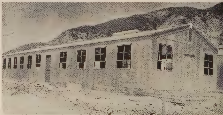
DISMANTLING of this typical building for a move will include removal of roof panels individually, removing of rib bolts at top and bottom, and tipping the wall panels outward.
