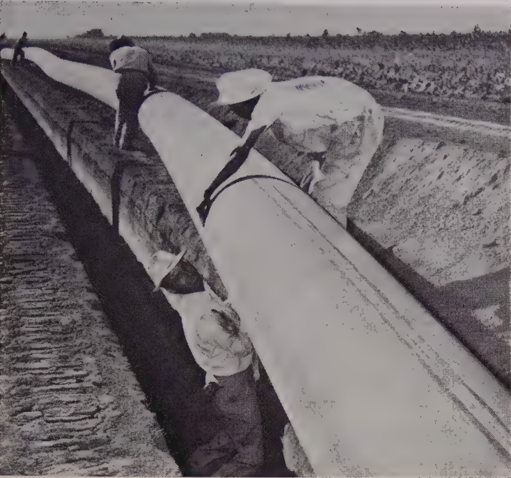
INFLATABLE rubber and fabric hose-like form, core of new continuous pipe casting process developed by Phoenix man, used to form irrigation pipe.
