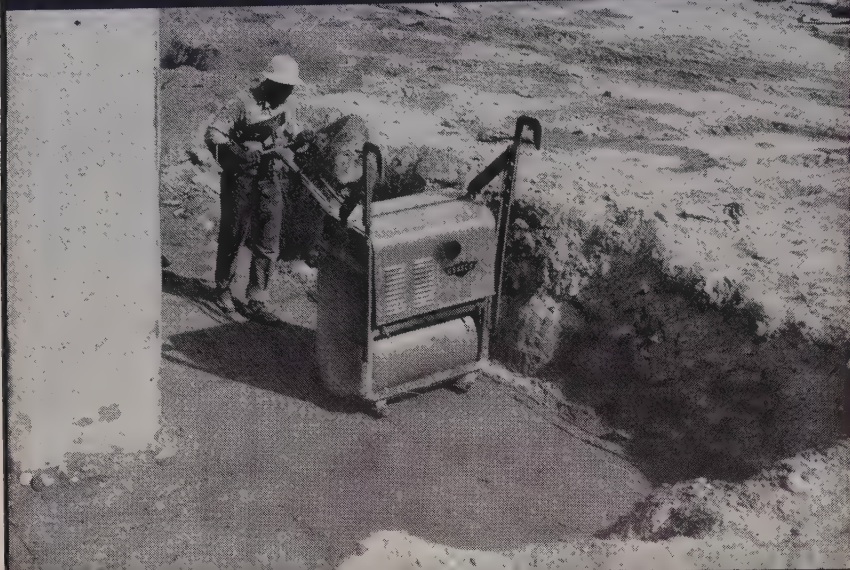
Essick VR-28-W Self-Propelled Vibrating Compactor on Golden State Freeway
