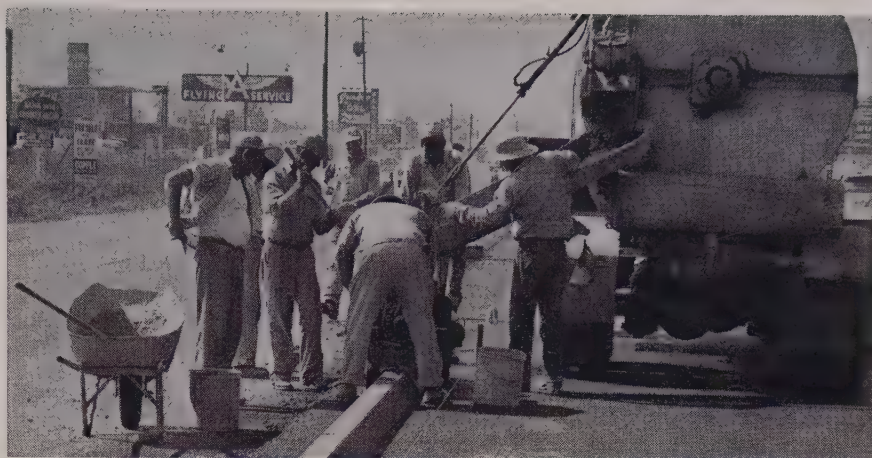
JUST BEFORE concrete curbing is extruded by machine, liquid adhesive is brushed onto existing pavement. Concrete and adhesive cure together, anchoring the curb securely.
