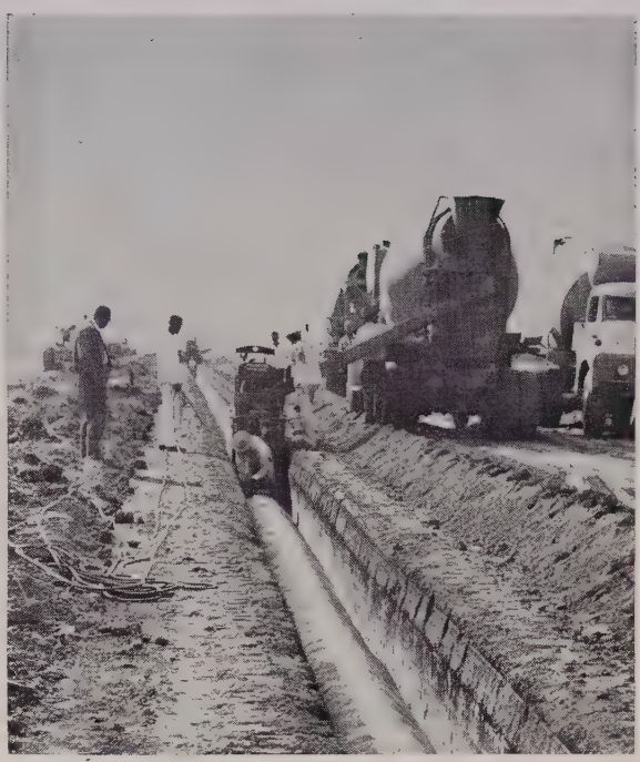
PIPE CASTING machine works along trench, placing concrete at 8 to 10 Ft. per min. Machine picks up form to place invert.
