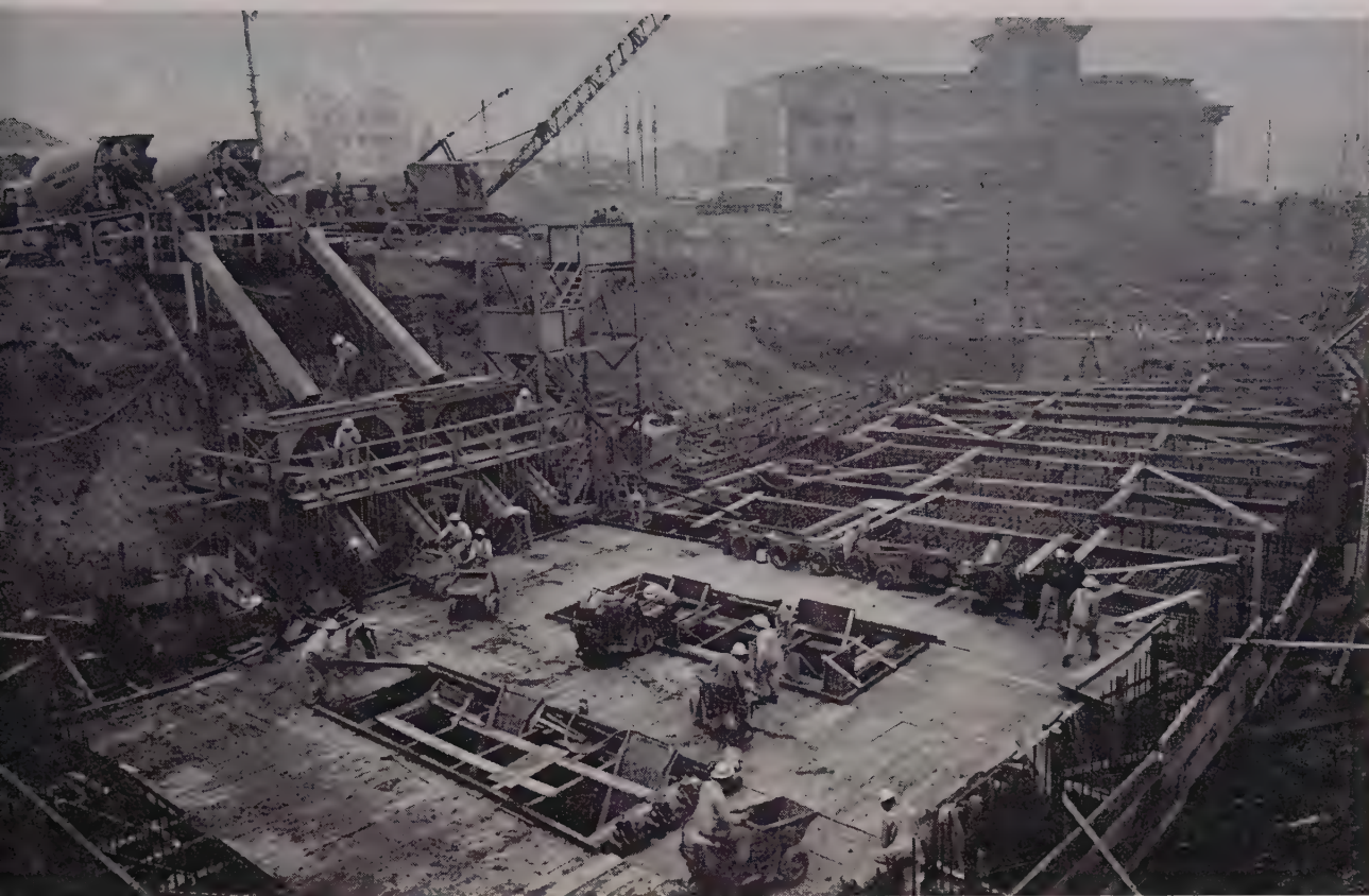
FLOATING foundation of the office structure is a steel-reinforced slab 5 ft. thick, 62 ft. wide, and 420 ft. long. More than 130,000 cu. yd. of material was excavated for foundation which was placed 40 ft. below surface. Here transit trucks discharge through chutes into mobile surge hoppers which are used to feed concrete buggies 4 at a time. Subsurface work was done by MacDonald, Young & Nelson, Inc. General contractor was Robert E. McKee, Inc.
