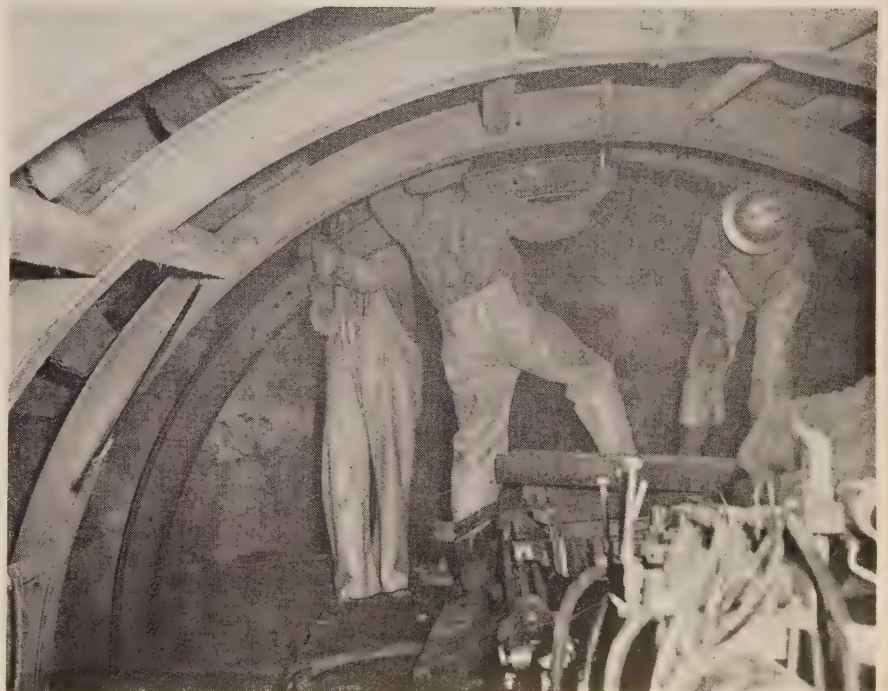
MINERS standing on top deck of jumbo set steel arch. About one-third of the tunnel had to be supported. Supported sections will be lined with concrete. Holing through is expected in April.
