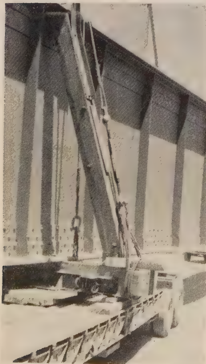
HAULING equipment to move the girder the 5 mi. from railhead to the site included a 20-tire trailer with its own compressor for brakes and steering. Blocking, timber struts and slings tensioned by turnbuckles held the girder in position during the move.
