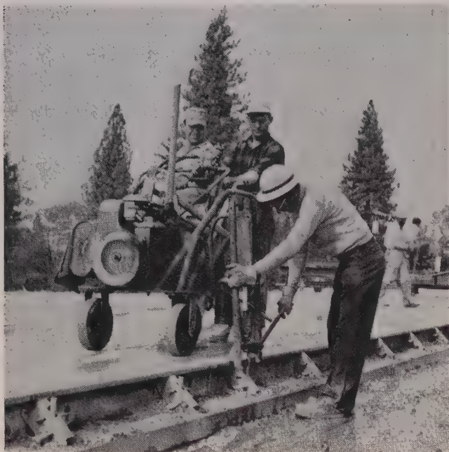
STAKES are pulled with this hydraulic rig powered by small gas engine. Fork hooks around end of stake, and cylinder pulls against frame.
