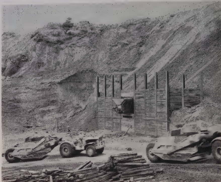
BIN and conveyor used to load out broken rock after drilling and shooting on the 1,500,000-cu. yd. Jamestown Cut. About half the cut required blasting.
