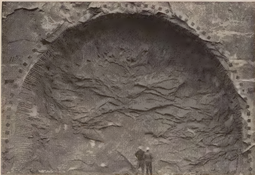
INITIAL FACE of a diversion tunnel at Glen Canyon Dam project showing the rock bolts and plate washers used to support the arch of the roof and the brow profile of the portal.
