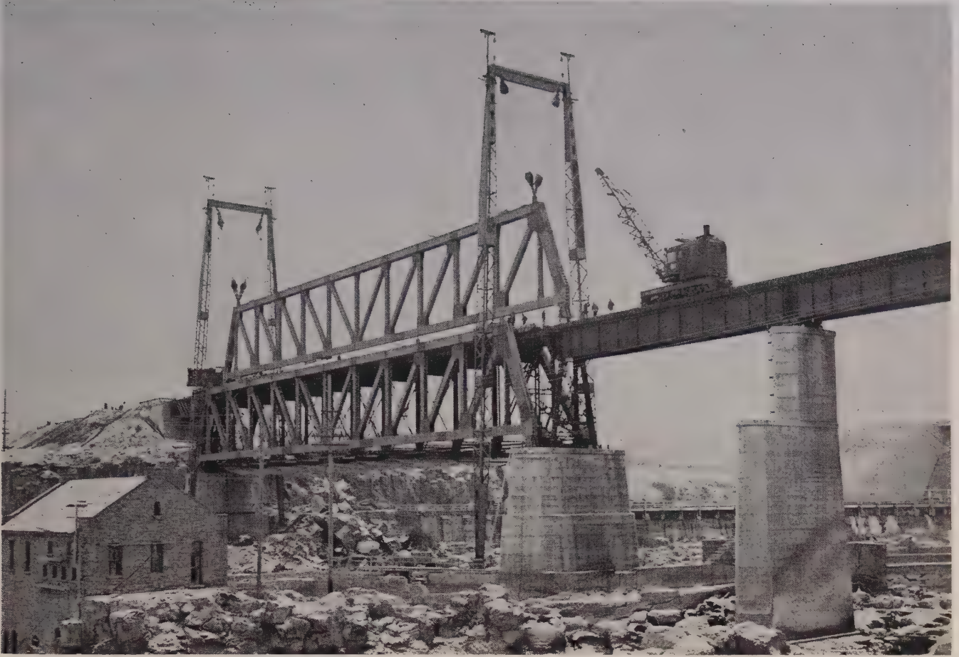
4. TWO PAIRS of 150-ft. steel poles with steel headframes were supplied by Pacific Crane & Rigging Co. Div. of Macco Corp., Paramount, Calif., for lifting the trusses. Two load blocks were hooked into lifting lugs at each end of the truss, taking the load to permit removal of outriggers and running gear. Blocks on one side were slacked to drift truss to edge of bridge.
