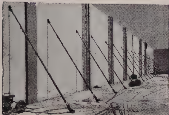
ADJUSTABLE BRACES used for quick and easy alignment of panels
