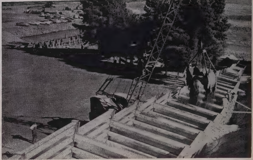
STEEL bin wall forms retaining wall along Ingerson Avenue. Wall has maximum height of 25 ft.; was constructed without mishap in dry year.
