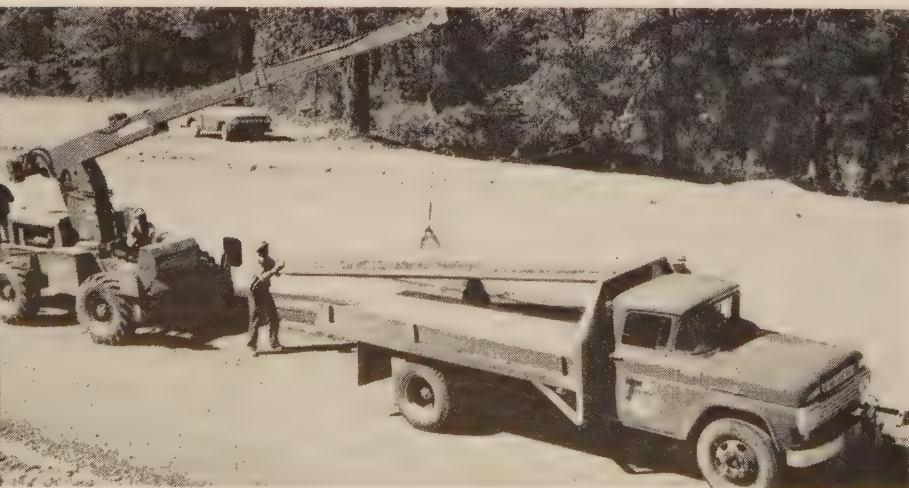
UTILITY crane loads headers on flat rack for transport to front of job. Each unit made up of 2 steel headers bolted to 20-ft. timber for additional height to accommodate sub base.
