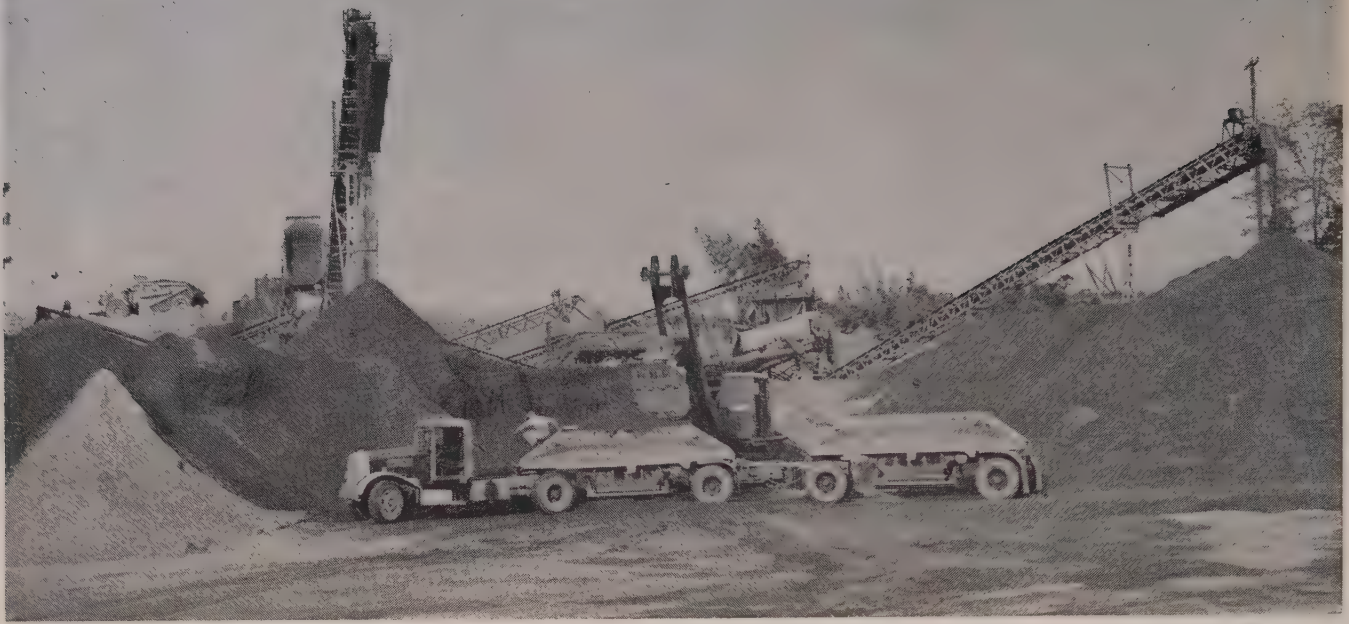
BASE MATERIAL pit and processing plant located just off road at highest point on job. End-dumps, top, deliver material from pit to
