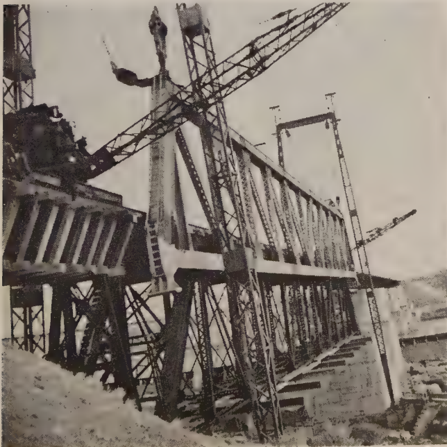
5. CRANES with booms at wide angle pull truss outward for final lowering into position. Crane and drum hoists were coordinated by Jim Curran, UP bridge engineer with mike in center of bridge. Job was done in 8 deg. weather.
