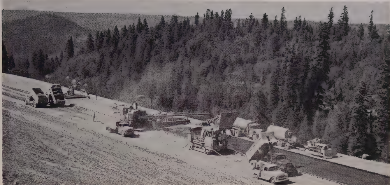
PAVING SPREAD rounds curve in new roadway. String includes two Koehring 34E pavers, a Blaw-Knox spreader, Jaeger finisher and Lewis
