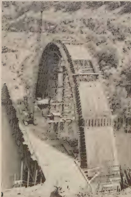
POUR NO. 6 going into the main arch (left) near the crown. Placements were made in pairs to keep the arch in balance. Top-forms in 3-ft. panels were used in pouring the arches, except near the crown. The timber tower under the arch was used in erecting and removal of the steel arch centering. Center arch completed (right) with truss in position for the third arch.
