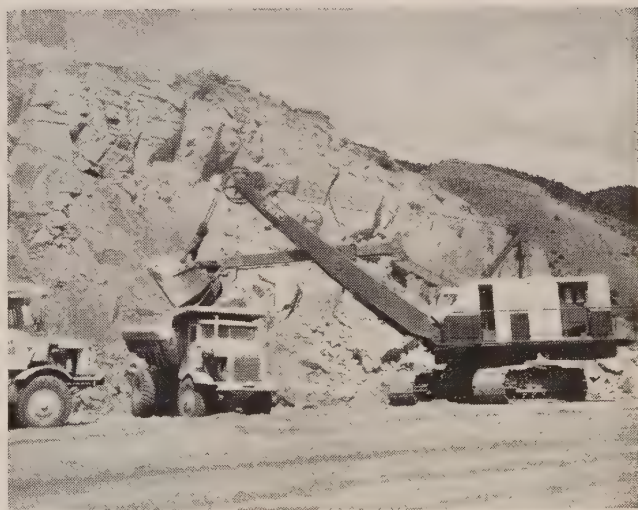
Pioneer's Bucyrus-Erie 3 cubic yard shovel—the first of its kind in Colorado—loads a dump truck to keep the job moving on its 150-day schedule.
