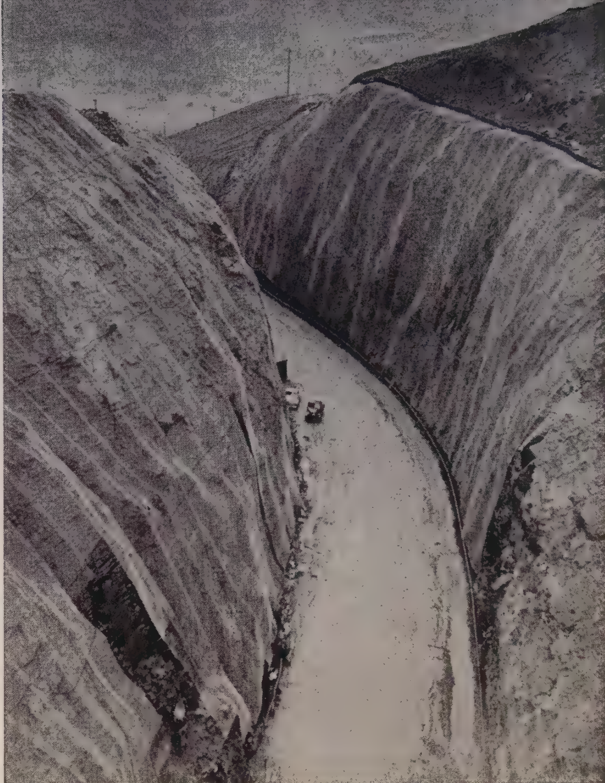
ABOUT 70 ac. of chain link fabric are used to support these rock walls of the forebay channel at Swift Creek Dam. Lengths of fabric were unrolled from the top of the 200-ft. high walls, with an 8-in. overlap. The fabric was secured by rock bolts spaced 20 ft. apart.
