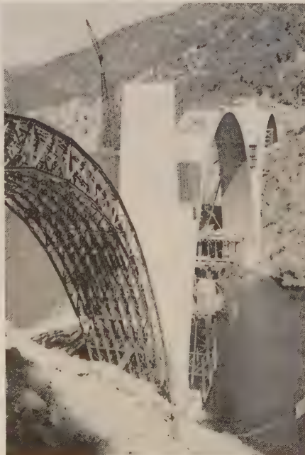
POUR NO. 6 going into the main arch (left) near the crown. Placements were made in pairs to keep the arch in balance. Top-forms in 3-ft. panels were used in pouring the arches, except near the crown. The timber tower under the arch was used in erecting and removal of the steel arch centering. Center arch completed (right) with truss in position for the third arch.
