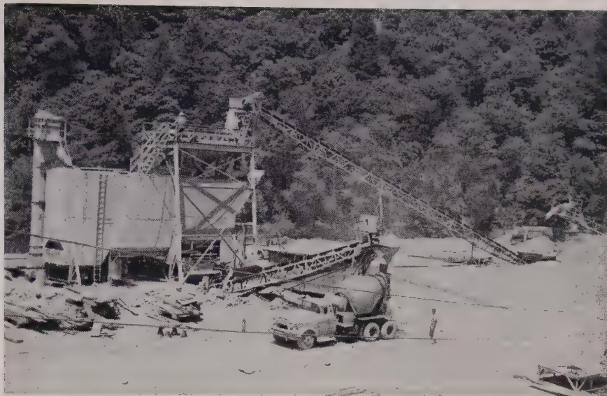
CONCRETE PLANT on the sandbar about .5 mi. upstream from the bridge site. The Noble batch plant is supplied with 3 sizes of aggregate and sand.
