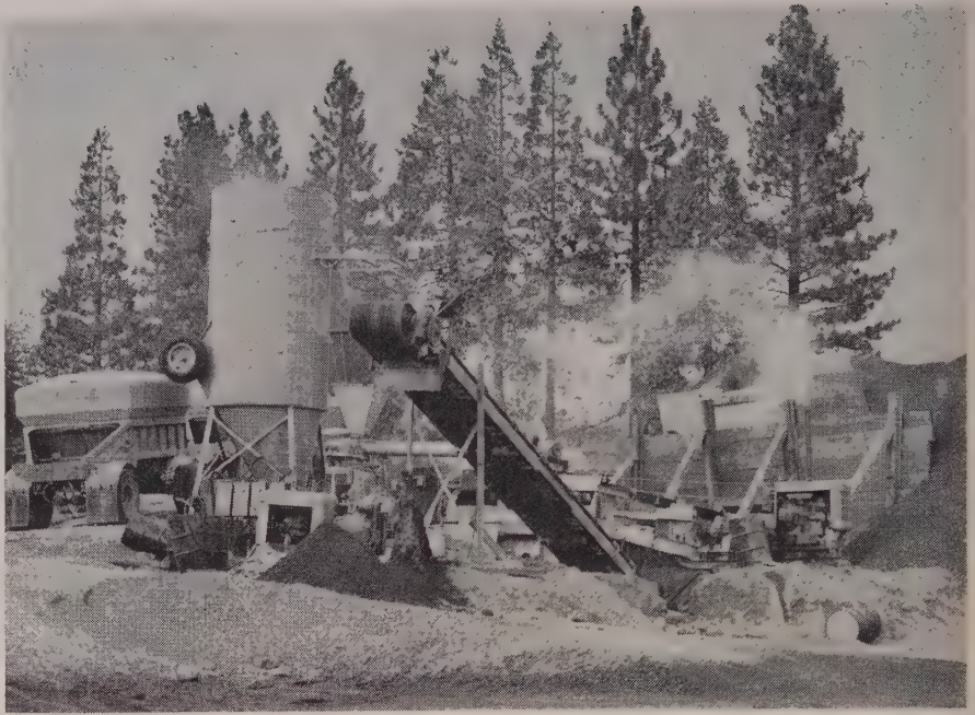
CEMENT treated sub-grade was pre-mixed in this continuous type plant. Cement stored in hopper at left, and aggregate drawn from bank behind bulkhead. Trucks were loaded from belt.
