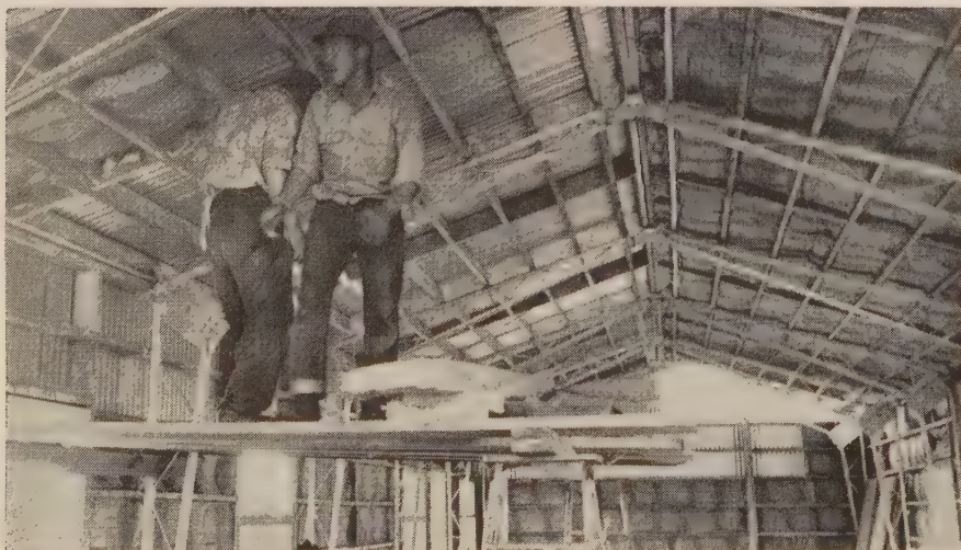
ESKIMO Guardsmen, hired by the contractor, install insulation in pre-fabricated structure at Kipnuk.
