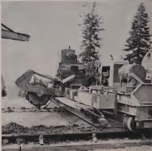
STEEL tie bars are imbedded with this reel. Bar set in notches of projecting arms is carried around steel and deposited below saw depth.
