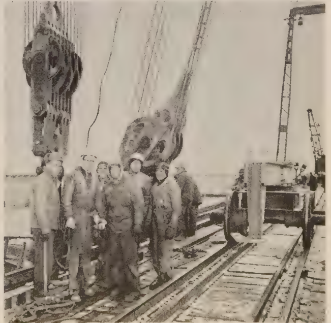
6. CREW grins after completing lowering on schedule. Big blocks in background use 17 parts of 7/8-in. steel cable. Louis Stec, left, was project supervisor for Pacific Crane who planned operation. Steel supplied by Paxton & Verling Steel Co.
