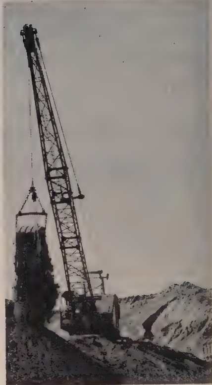
P & H Harnischfeger dragline operated by a student excavating for sanitary landfill. This is one of three combination machines.
