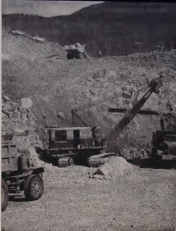
From the base of one of the huge rock slides these Macks worked back and forth to the river bed on a round-the-clock schedule. F & S Contracting Company of Butte, Montana, owns and operates the big trucks.
