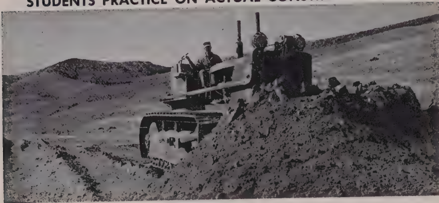
STUDENT on TD-24 International, bulldozing excess dirt from grade after backsloping.
