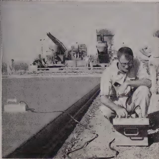
NUCLEAR instrument, operated by Douglas Howard, Materials & Research Laboratory, to measure density in new non-destructive test
