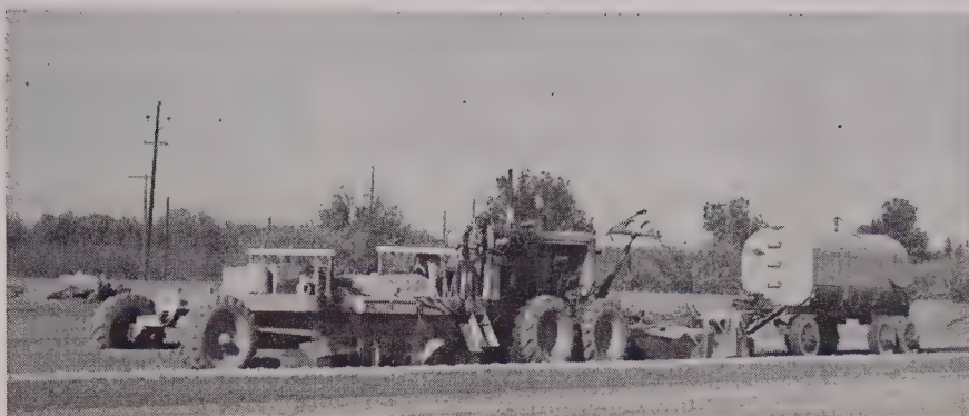
CEMENT-treated subgrade was prepared with two Wood mixers. Unit above is equipped with spreader to knock down windrow, behind the mixer. Water trailer towed at rear.
