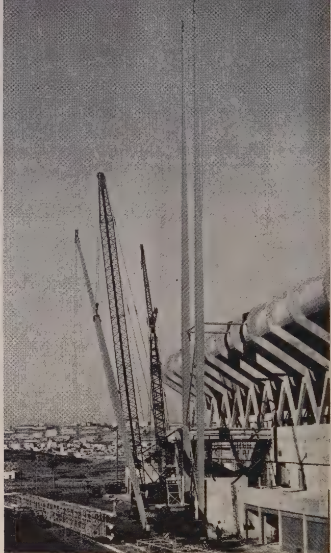
TWO CRANES of Bigge Crane & Rigging Co. used to hoist 197-ft. welded steel pole into position. Aluminum T used to raise light cages.
