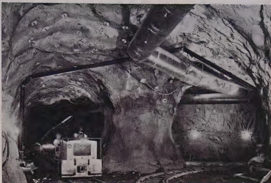
AT the adit-tunnel junction in the clear, the creek tunnel rock bolts are thick and wire mesh has been added to catch rock fall-outs. Rock bolts were used for support for 6,700 ft. downstream, and 6,000 ft. upstream from the adit. Steel plate washers 10 x 10 in. were used with wood blocks and wedges. The two photos are from the Bureau of Reclamation.
