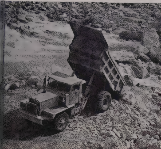
Thousands upon thousands of tons of rock were dumped along the base of the earthquake-made dam to form a "stilling basin." Here a Mack LVX dumper adds its load of rock to the river bed.
