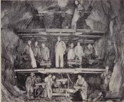
Construction ran months ahead of schedule on this 3-mile, 21 ft dia. Fremont power tunnel drilled thru hard granite, heavy with silica. Brunner & Lay 1 1/4" type H carbide Rok-Bits used exclusively.
