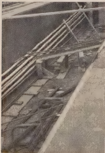
SEVEN TENDONS (six 40-wire units and one 12-wire unit) draped in position for 156-foot bridge girder.
