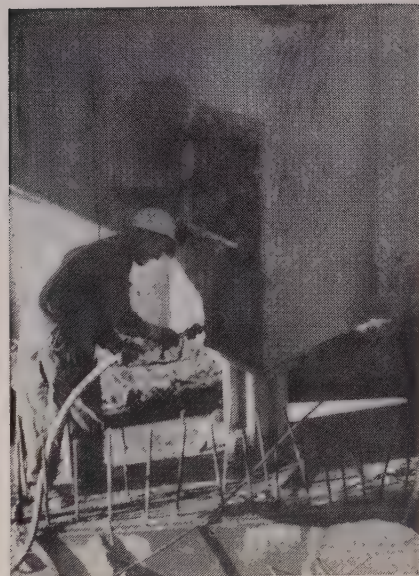
GROUTING MIXTURE is forced into tendons and around wires after stressing. Pressure injectors and venting procedures assure positive filling of all casing and trumpet voids.
