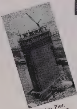
Bridge Pier, San Francisco
