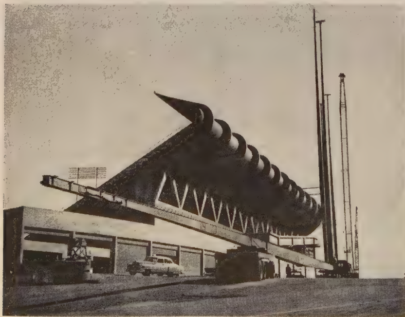
TAPERED steel pole, one of 19 built by Weld-Rite Co., Oakland, for Candlestick Park lighting, is hauled to site by truck-trailer. Long poles were shipped on 5 flatcars.
