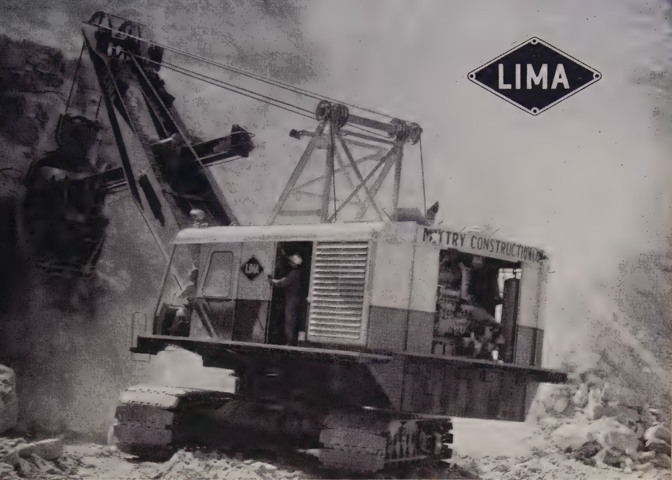
type 1800 5-yd. shovel—one of five Limas owned by Mittry Construction, Los Angeles. Shown excavating at Abiquiu earth fill dam project, Shama N. Mex.
