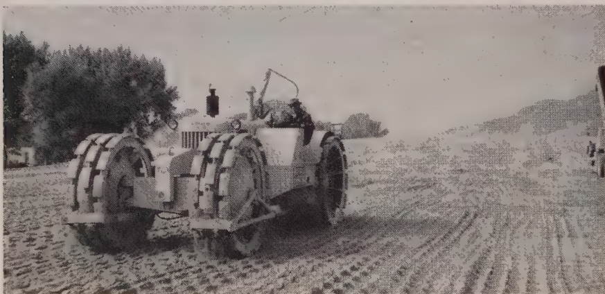
COMPACTION of 8,000 cu. yd. per day is handled by this Buffalo-Springfield Kompactor. One of its big advantages is its speed, which enables it to work without getting in way of haulers.
