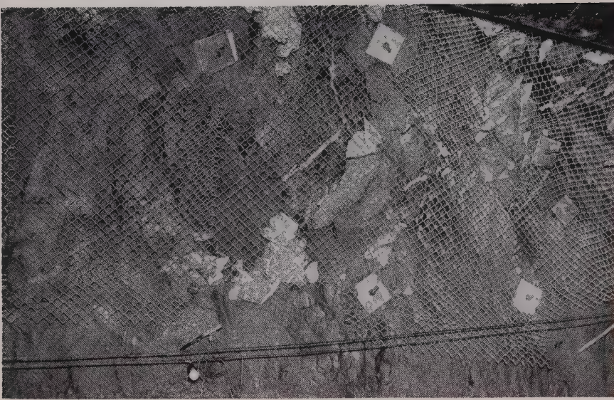
CLOSE-UP of wire mesh in the Clear Creek Tunnel showing rock-bolt pattern and loose rock fragments caught in the mesh. Tunnel was driven through hard, coarse grained granite.
