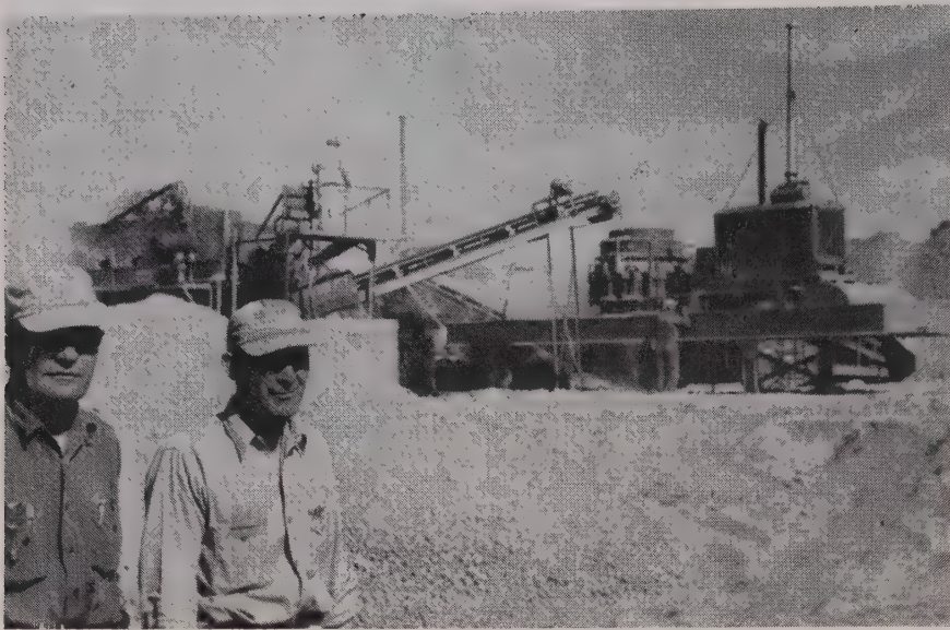
D. A. WAGNER (left), superintendent for Woodward Construction Co., with L. Vosika, foreman, are shown at the site of a $109,979 job recently awarded. Covering a 6-mi. stretch, work consists of draining, grading, and road-mix surfacing in Lincoln County, Wyo. D. Boom is another foreman on this job, which will be ready for oil early this year.
