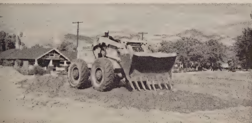
HANDYMAN on project is this Michigan loader. One of its jobs is removing oversize material from zone 3 by means of heavy steel teeth spaced along leading edge of bucket.
