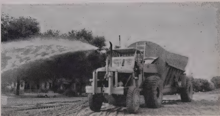
WATER TRUCK is an 8,000-gal. tank pulled by a Euclid truck. Contents can be emptied in 12 minutes. Front side spray takes care of hard-to-reach areas like side slopes.
