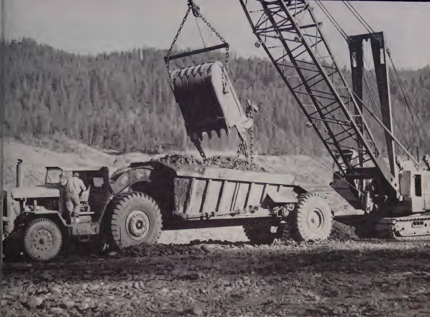
A 7½ yd. dragline loads a Model LDT Bottom-Dump Euclid with 40 yds. of river gravel for 2½ mile haul to the fill. Green-Tecon have 13 of these big "Eucs" that are powered by 12 cylinder GM diesel engines of 432 h.p. with Torqmatic Drive.
