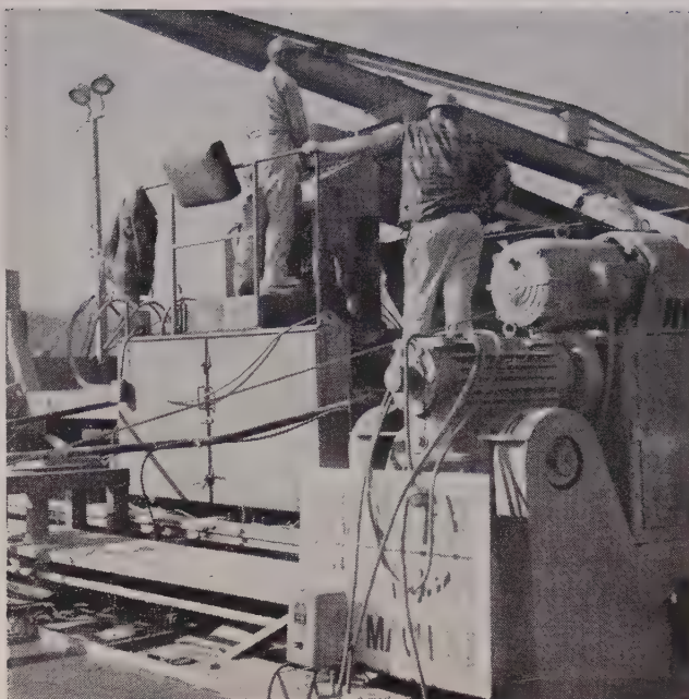
OPERATOR'S platform gives unrestricted view of job. Form can be maneuvered manually as well as automatically. Note lights on form.
