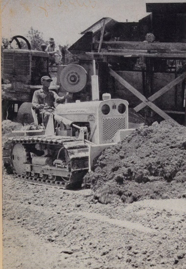
Seven-foot IH Bullgrader is raised, lowered, angled, and tilted hydraulically—with complete control of all actions from the tractor seat.
