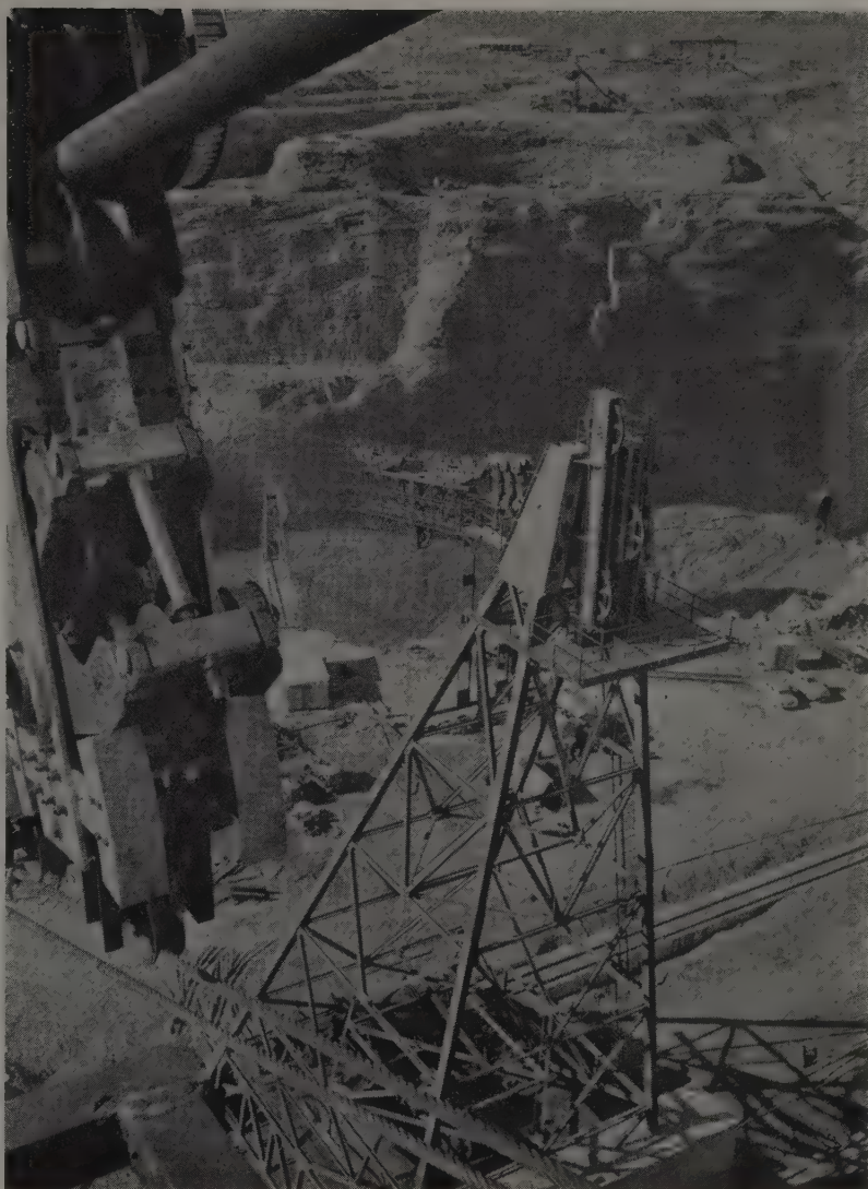
LOOKING from one head tower to the other, with the canyon in the background. Tower legs are wide-flange beams. Note the plate stiffening and design of the supports for the tower sheaves. The service platforms have adequate guard railing for the safety of personnel.
