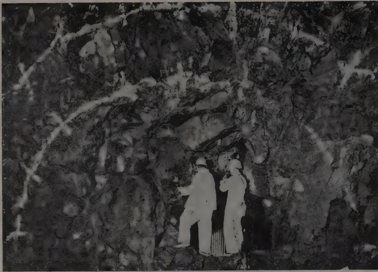
LOADING holes as the 7 x 8-ft. pilot hole was started from the old face through the remaining 60 ft. to daylight. The paint marking for the drill pattern for the crown section is four years old, dating back to when work stopped on the original job.
