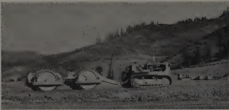
TWO PAIRS of 6x6 ft. sheepsfoot rollers are hooked to crawler. Hydraulic cylinders connecting front and back pairs enable rig to move backward as well as forward. Six passes required.
