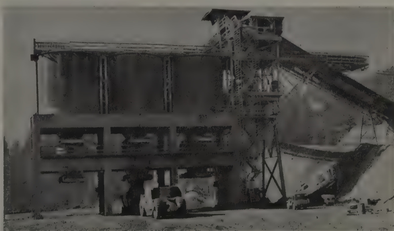
TERMINAL structure includes 3 bins of 400-ton capacity, each with automatic hopper scale below. Shuttle belt controlled by operator in tower fills bins. Scrapers are shown loading at center bin.
