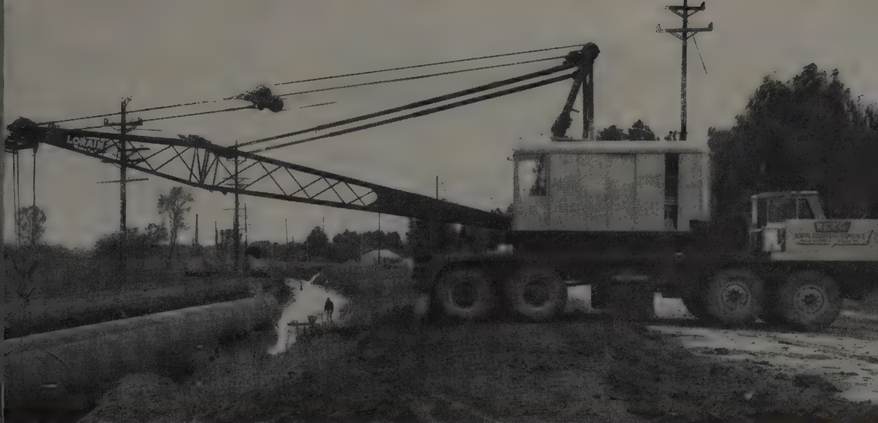
65-ton MC-760 spots 84-ft. long pipe with 78-in. diameter with pinpoint accuracy. Only ¼-in. tolerance is permitted for welding. Moto-Crane moves to new location every hour.
