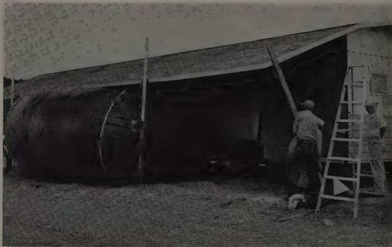
WORKMEN raise side roof of three-bedroom houses manufactured by TransaHomes Corp. with combination of large pneumatic bag and special jacks. Roof will be held in place until sides are folded out. Project community of Dutch John may reach population of 3,000.
