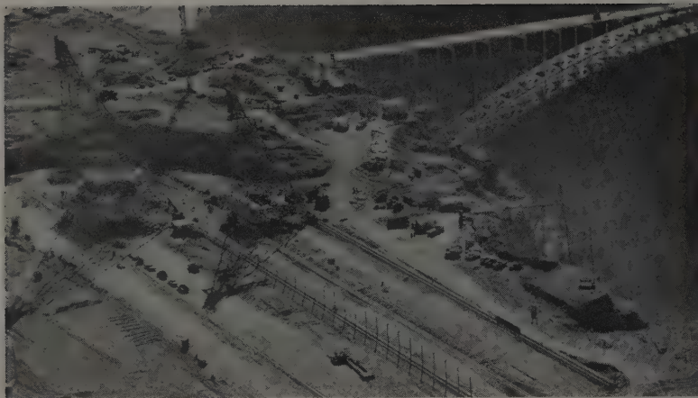
AIR VIEW of the head towers and trackways at a time when the machinery was being installed. The already famous highway bridge spanning the canyon is shown nearing completion.
