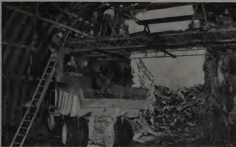
FINISHING the 860 ft. of 41-ft. tunnel with the crew dismantling the platform used to help install the steel sets. Diesel equipment was all equipped with gas scrubbers.
