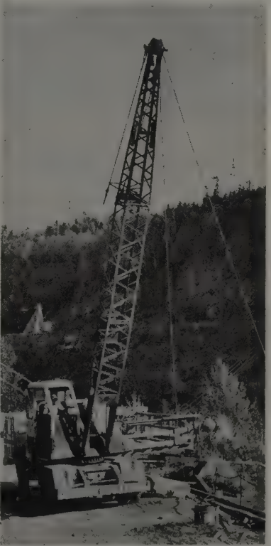
HARD TO BELIEVE , but this crane operator is helping to set supporting steel in the tunnel. With a line extending down through a drilled hole, the arch sections of the sets were lifted into position.
