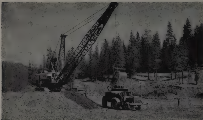
RIVER BED excavation is done with electric-powered draglines and shovels. Material for Zone 3 is hauled in fleet of 30-yd. bottom-dumps. Note light tower on skids. River directed to ditch.
