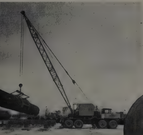
35-ton MC-530W with 70-ft. boom and clamps eases 42-ft. pipe sections onto rack in welding yard where they are welded into 84-ft. lengths. These are loaded out at the rate of 32 a day.
