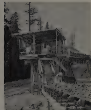
TRANSFER station on belt line. Short belt section, center, connects two main flights.
