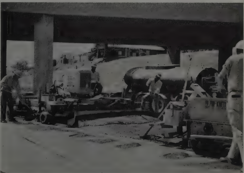
FOLLOWING spreader is this Blaw-Knox tamper. Paving train is completed by a Johnson float finisher. Both metal strip and sawed joints were used.
