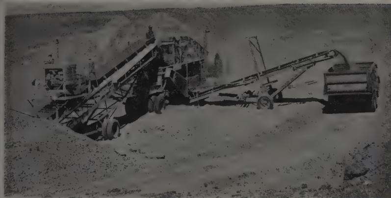
SOURCE of aggregate was close, but its quality presented the problem. Pit material was reduced to ¾-in. maximum size in this Cedarapids plant.
