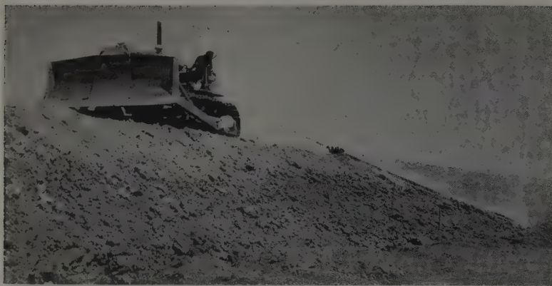
STEEP 2:1 dike slopes on the land side are brought to grade by dragging an old set of tractor track links behind a Cat D8 tractor. F&K later replaced this with a Briscoe backsloper mounted on the D8, permitting closer control of slopes.
