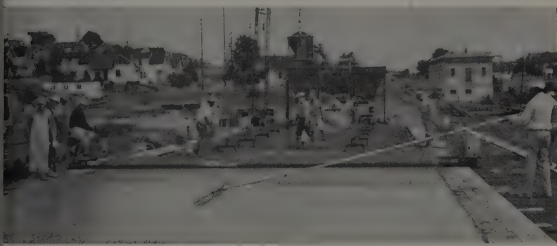
RAILPORTER and Clary screed team up to make 26-ft. wide section of deck slab. A 10-ft. aluminum bull float in foreground. For this pour, Railporter was operated on parallel shuttle tracks each served by loading hopper.
