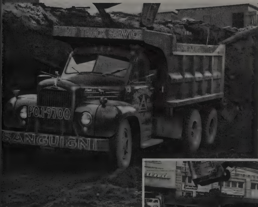
Brawny Mack Model B-63SX 47,000 lbs. GVW dumper helps in excavation for Pittsburgh hotel foundation.
