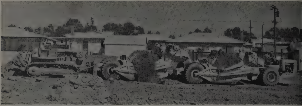
HEAPING loads are picked up by these two 18-yd. LeTourneau-Westinghouse scrapers hooked up in tandem and pulled by Model C prime mover. The electric power system for the controls simplifies the hook-up.
