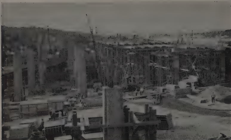
GENERAL view of project looking south toward Lake Washington Ship Canal. Falsework at right is for four south-bound lanes of upper deck. Ramp at left is off-ramp from lower deck. Columns left center are for support of four north-bound lanes of upper deck.
