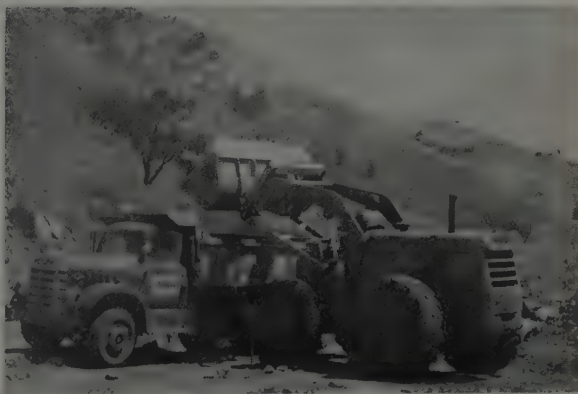
BROKEN concrete from old road loaded in trucks for disposal in fill area. Resteel in old road was cut with torch to separate chunks.
