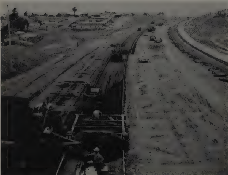
CEMENT-treated base mixed at plant and spread inside headers. Spreading, compacting and grade cutting operations are shown in this over-all view of project.
