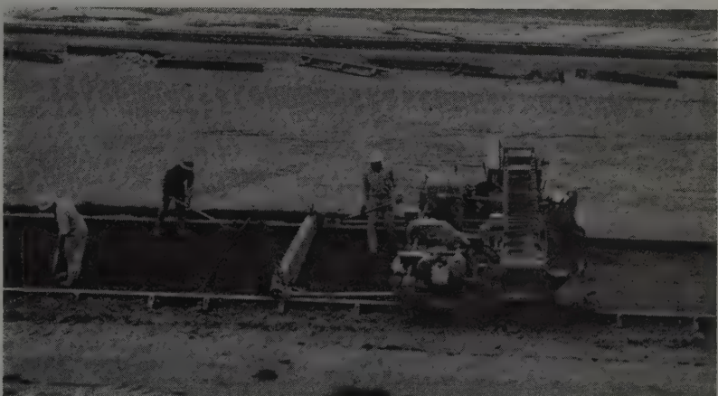
FINAL trimming of base material is done with Blaw-Knox grade cutter with minimum of handwork. Compacted subgrade is then ready for seal coat and concrete surfacing.
