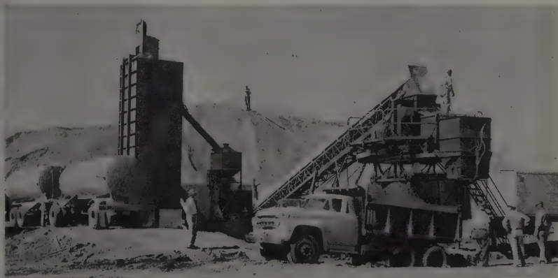
PLANT or road mixing was permitted in the specifications, and the contractor elected to use this Barber-Greene plant, conveyor and hopper for the stabilized base.
