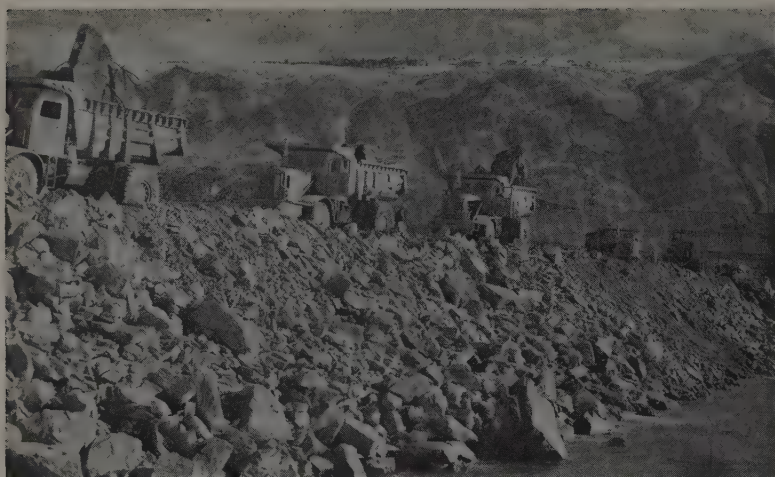
LINED UP for the final closure, these Euclids are loaded with "Siamese" boulders, some as heavy as 25 tons. Pairs of rocks had been drilled, fastened together with heavy cables and stockpiled. When dumped, one rock went into the opening and the other was pushed over the upstream face of the groin. About 10,000 tons of rock were used.
