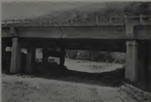
TWO BRIDGES , concrete in foreground and steel, must be removed. Concrete will be burned out to prevent damage to salvageable steel.
