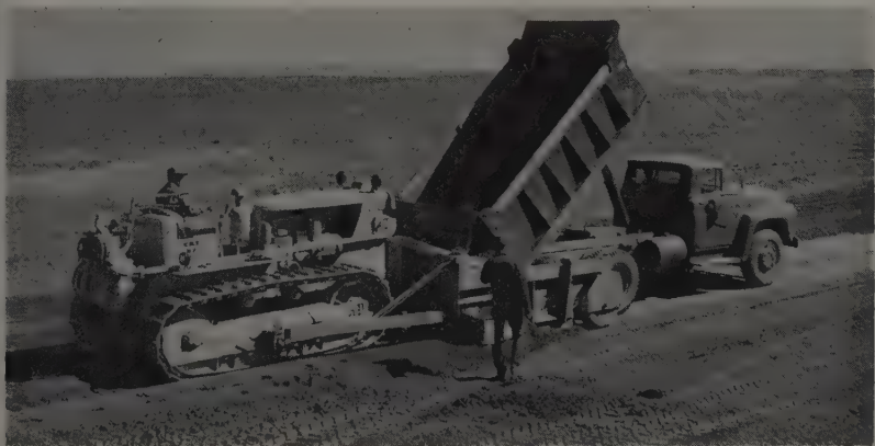
ON THE ROAD the loads of cement stabilized material were dumped into a Jersey spreader and laid at a 10-in. depth for a specified compacted thickness of 7.2 in.
