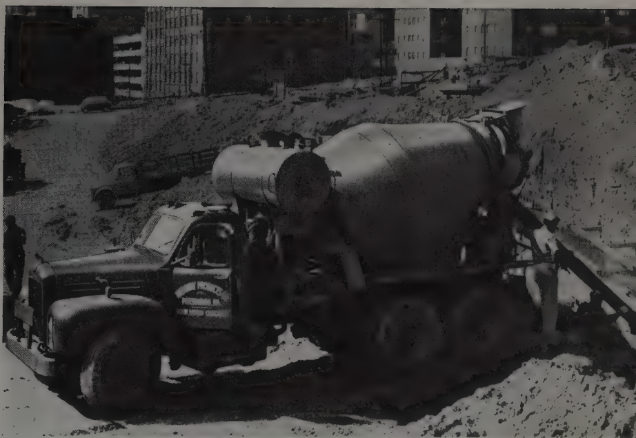
Yard after yard of ready-mix concrete hauled by Mack trucks is used to build retaining wall at construction site.
