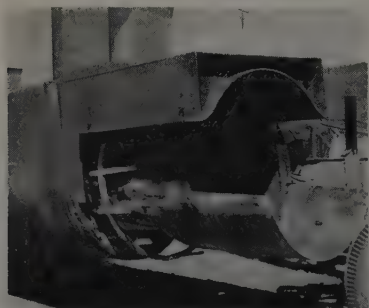
PIPE FORM on display showing new consolidating ring, and removable aluminum form.
