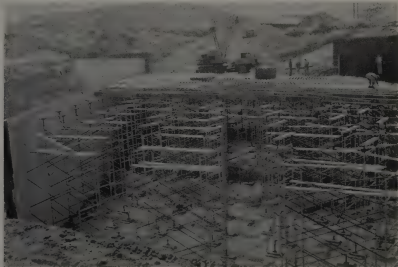
STEEL scaffolding falsework for box girder bridge. Steel frames can be re-used on many of the 32 bridges which make up project. Units work best on level footing.
