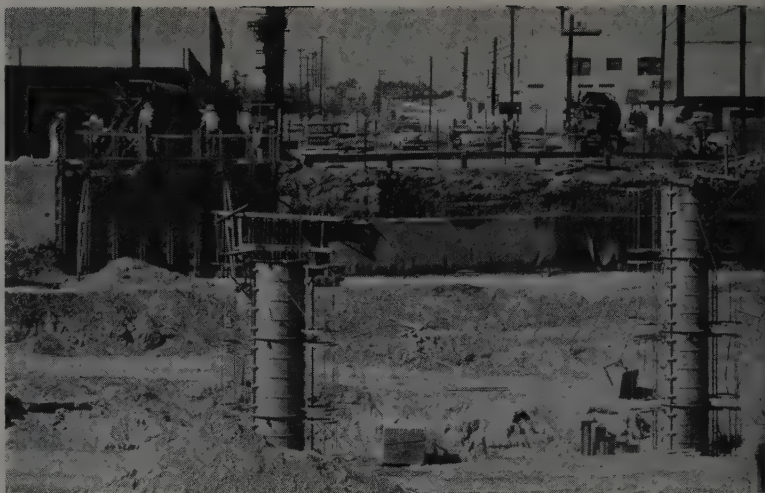
Cylindrical columns are formed with half-circle steel sections flanged at top and side. Four-foot diameter sections can be bolted together for column of any height.
