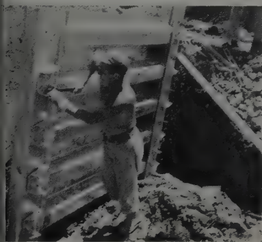
Assembling Armco Retaining Wall
