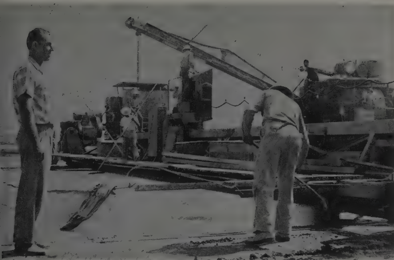
FINISHING operations watched by Gordon McGrew, superintendent, left. One man works float, and two others work the edges behind slip-form. Burlap drag completes finishing.
