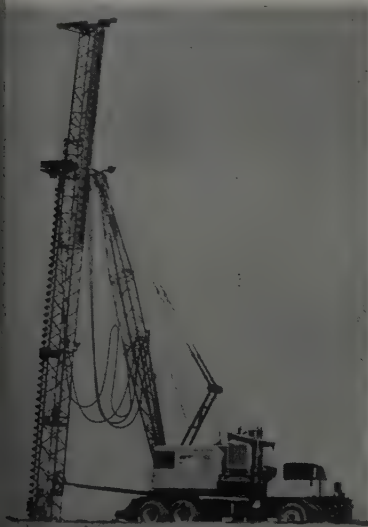
GIANT auger built by contractor used to drill 10-ft. holes for concrete piles.
