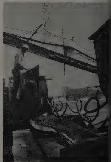
OPERATOR guides slip-form and handles all operations from push-button control panel.
