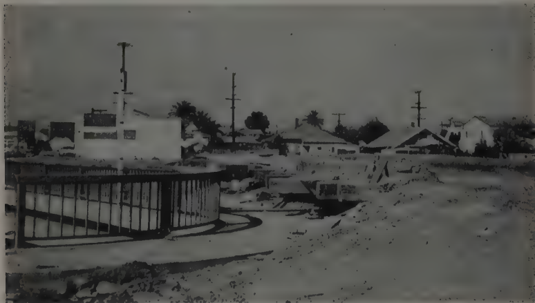
BRIDGE on a bridge permits heavy earth-movers to cross freeway. Timber haul bridge rests on steel girders erected over concrete deck of existing structure.
