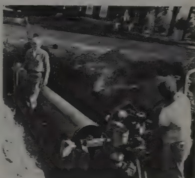
Boring with Armco Welded Steel Pipe
