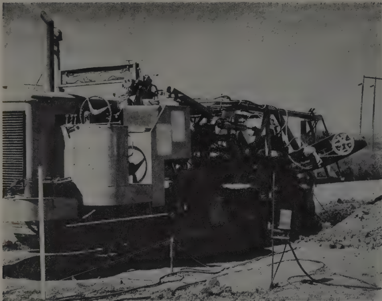
TRENCHING machine equipped with control. Note control head in foreground set on blue-top. Unit regulates exact depth of digging wheel. Torque converter powers forward motion.
