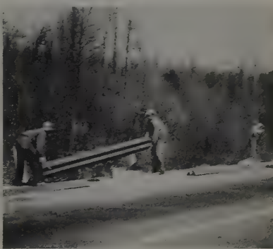
Installing Armco Guardrail
