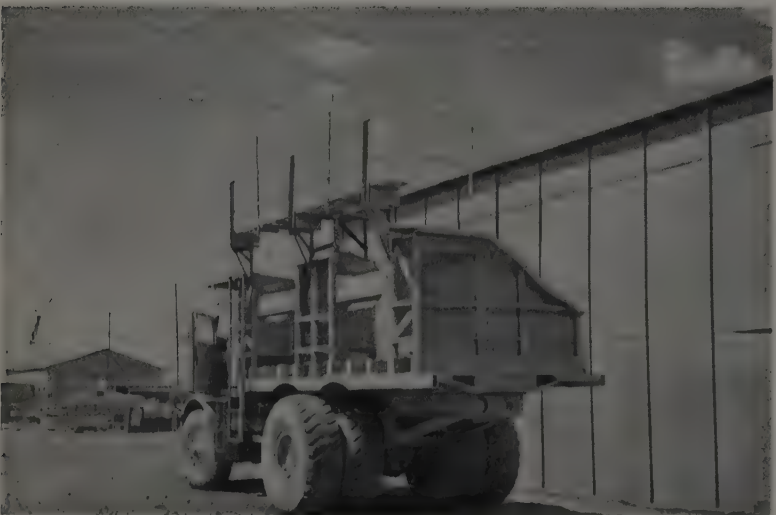
CONCRETE HAULING TRUCK is a converted Euclid end-dump. Dump body was replaced with platform which receives two buckets. Walkway is no longer needed because of automatic hooks.
