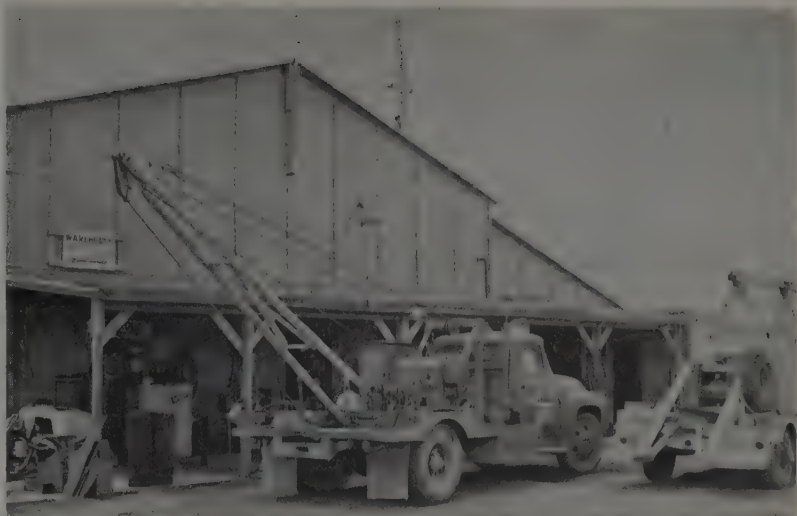
HANDY TOOL is light truck equipped with boom. Nine boom-equipped Ford trucks are on job serving the various crafts. Complex, spread-out project calls for such fast, mobile rigs.
