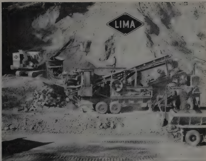
Lima Austin-Western portable 101-SE Crushing and Screening Plant processes gravel and rock fed into its mechanical feeder in 1-cu.-yd. bites by Lima Type 44 Shovel. Accurately sized gravel travels conveyor direct to waiting State Highway truck at this Buchanan, Mich., site.
