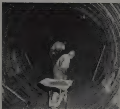
Tunneling with Armco Liner Plates
