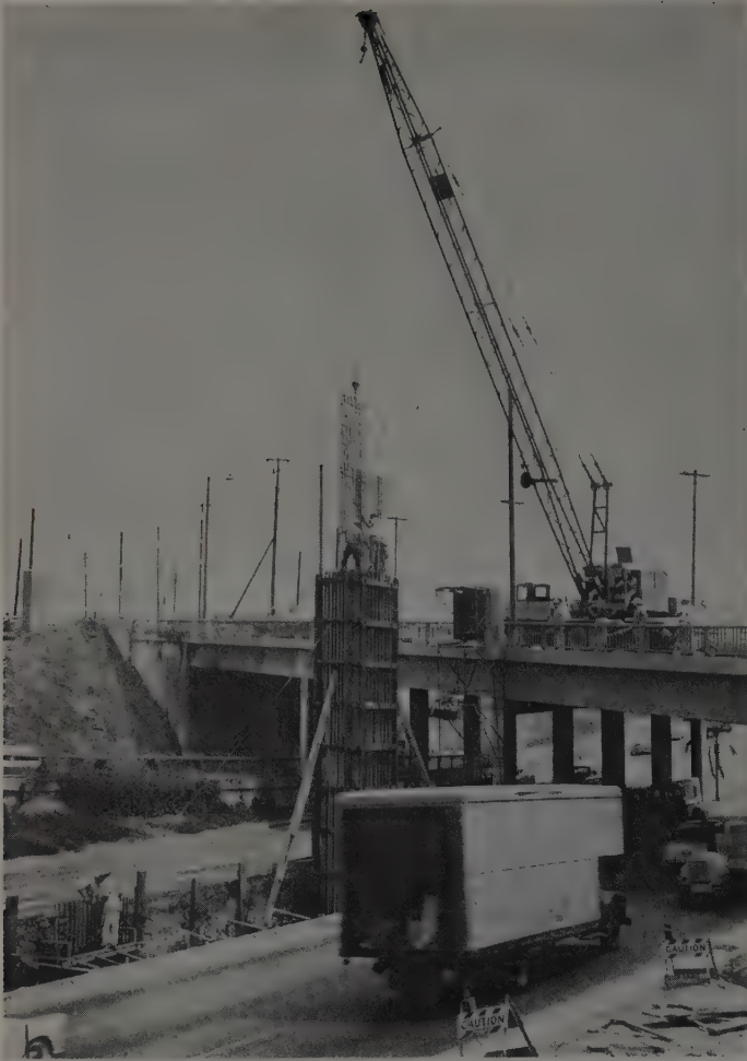
TWO-TON steel mat is lowered into pier form in middle of Santa Ana Freeway.
