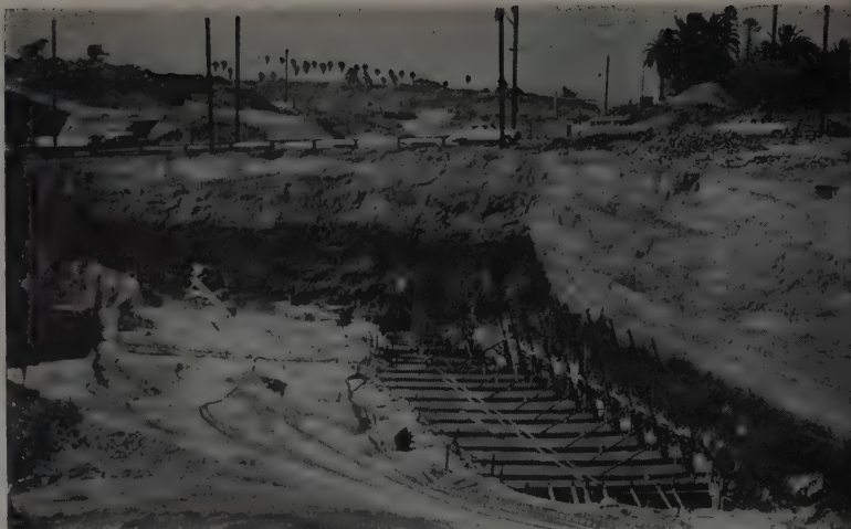
BLACK BELT at base of cut is road oil sprayed on sandy bank to retain moisture and prevent fall-out. Steep cut necessary because of restricted site.
