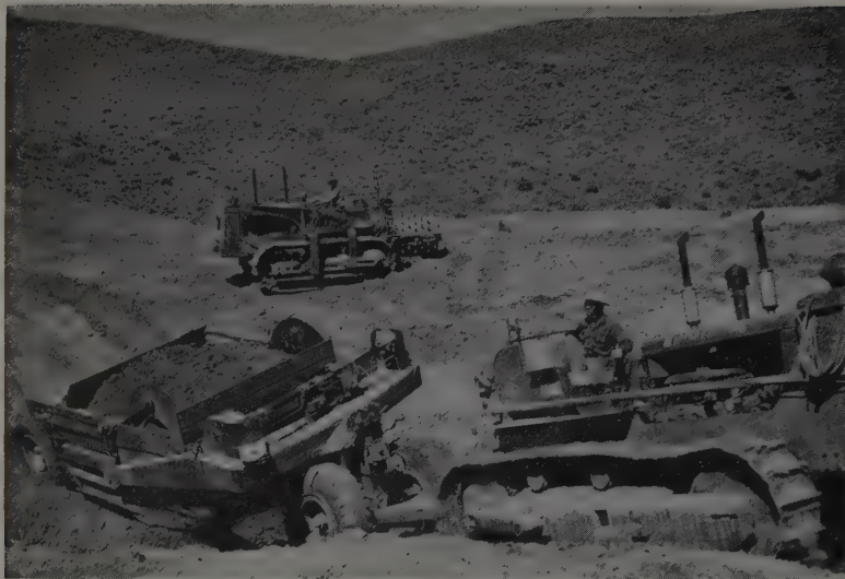
CONSTRUCTION activity on typical projects of the Small Watershed Act will involve excavation, earth fill, rock fill, channel improvement, pipe drains and ditching. The average project will be of a size that will provide work for small fleets of equipment. Contracts will be awarded by the local agency.
