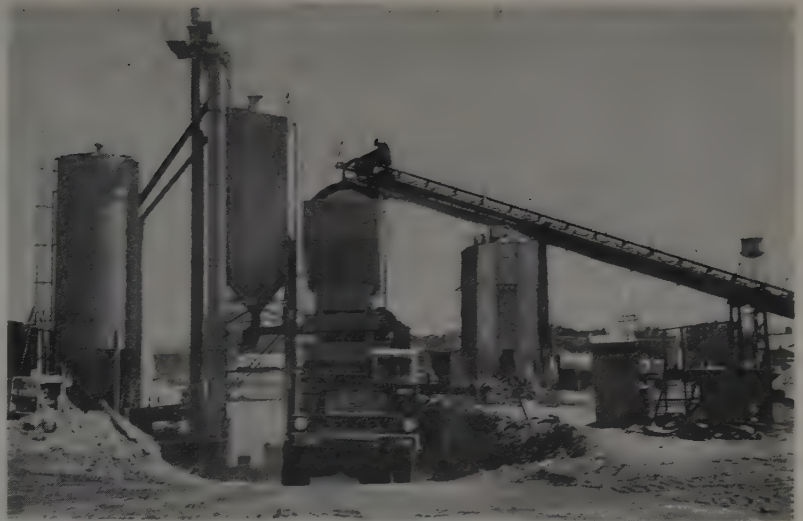
BATCH PLANT weighs out 5,000 tons of aggregate per shift, drops a 1\frac{1}{2} -yd. batch in 13 sec. Cement is received from rail cars at left, and aggregate conveyed from stockpiles at right.
