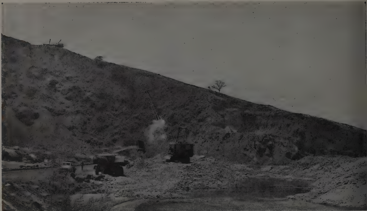
LEFT abutment ridge from upstream. Dragline in foreground is excavating channel for river diversion. Blast crater in ridge will be site
