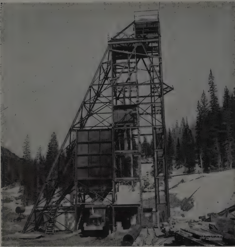
HEADFRAME at access shaft has separate hoists for personnel, materials, and muck. In photo truck receives load of muck from storage hopper. Access shaft is 916 ft. deep.
