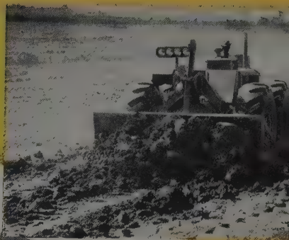
Cleans up in borrow pit
