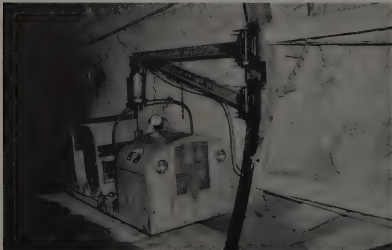
DIESEL UTILITY CAR is removed from track by special swivel boom mounted on steel set. Hoist at boom end is air-operated. Muck train locomotives are both diesel and battery-operated with changes now being made to combination engines.
