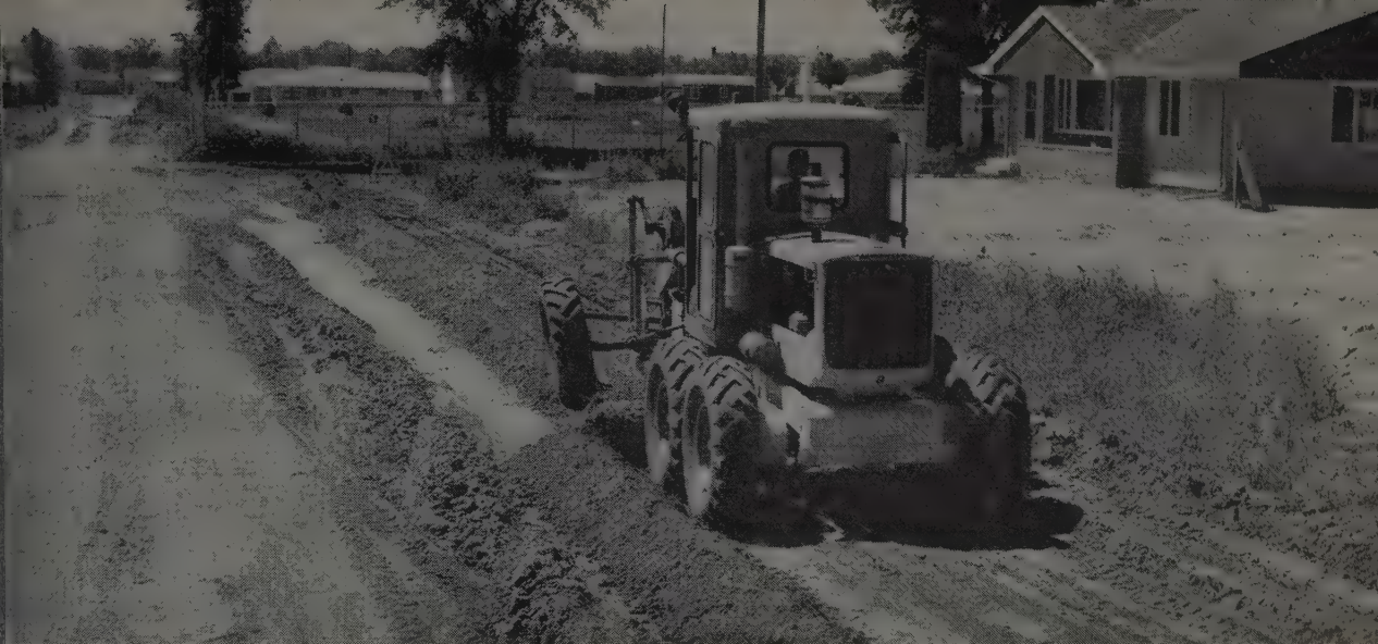
This Cat No. 12 Motor Grader is undercutting banks down 28 inches deep in St. Anthony Village, Minnesota. Cutting both sides, it averages about 8 blocks a 10-hour day in compacted hardpan. Owner: J. A. Denens & Son, Inc., Minneapolis, Minn.
