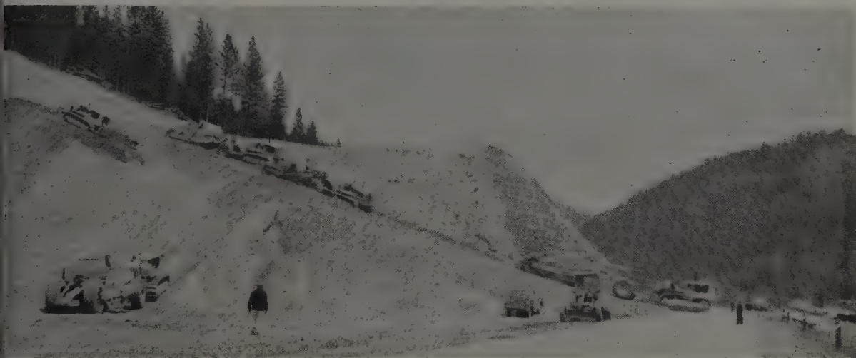
INTERCHANGE cut at the start of Idaho Interstate project. Spread includes four scrapers with 45-yd. heaped capacity pulled by D9 tractors.
