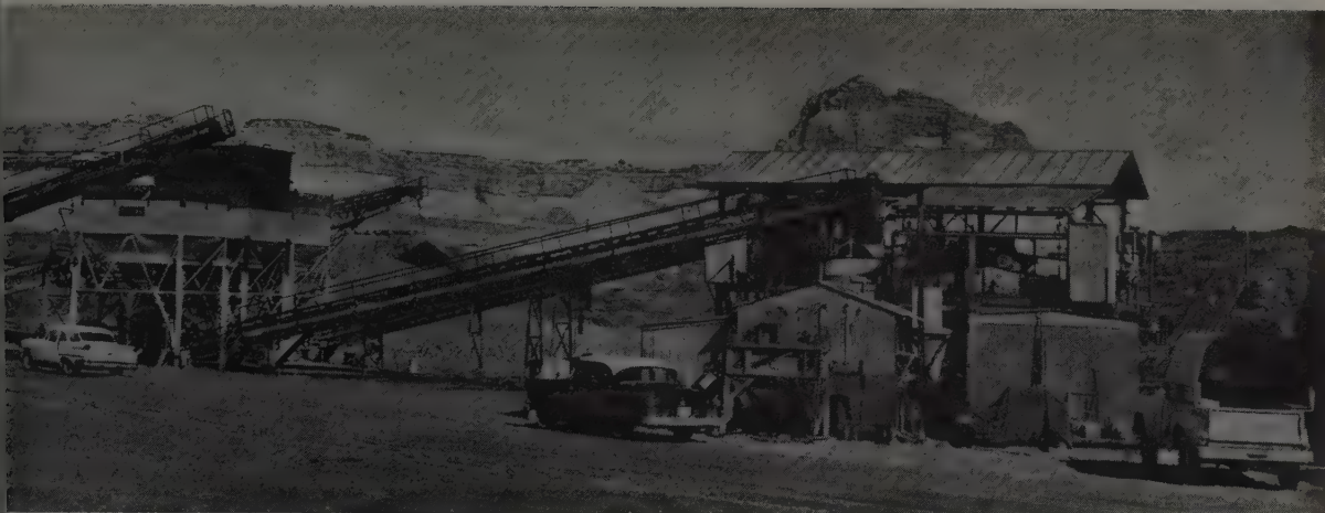
AT GLEN CANYON DAM these two HMS plants (right) are processing more than 95 tons of aggregate per hour. The improved product is
