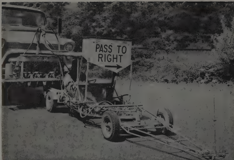
STRIPING PATTERN follows the national standard of painting 15 ft. and skipping 25 ft. Cost of this type of 4-in. stripe is $30 per mile. Use of hot paint has reduced drying time by 50%.
