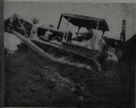
Kero dozer shoves fill dirt into position on Center part of the south marginal street area on the side. Big new equipment like this will see the job ahead of schedule.
