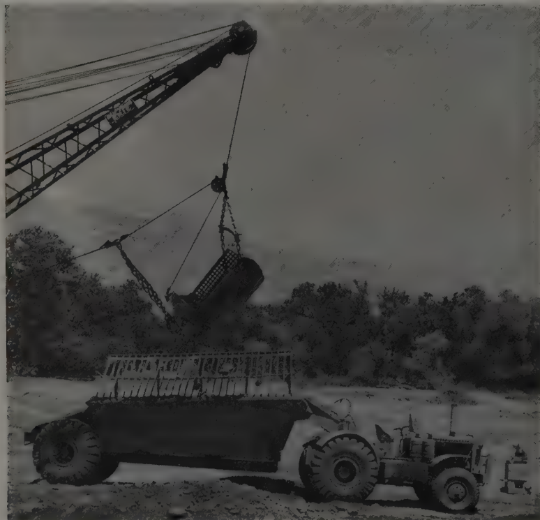
GRIZZLY welded to top of 30-yd. Athey bottom-dump trailer scalps off oversize rocks as dragline loads unit. Material comes from borrow in downstream riverbed.
