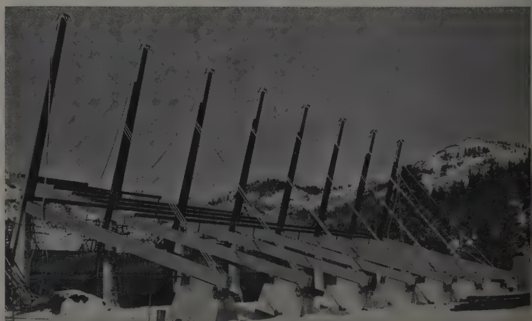
ROOF GIRDERS , extending to left in above photo, are partially in place, suspended by cables from column tops. By tensioning cables at backstay columns were given initial deflection which will be balanced when roof is under full load.
