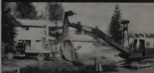
This versatile 35-M is excavating foundations for a $1,600,000 building project on the coast. It carries a 60-ft. boom and 20-ft. jib.
