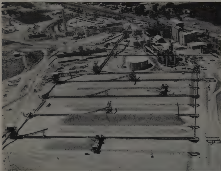
STORAGE area at the Oro Grande plant with the reclaimer working on the nearest pile while the stacker builds another pile in the next line. These machines can be operated by remote control and are interlocked with conveyors.
