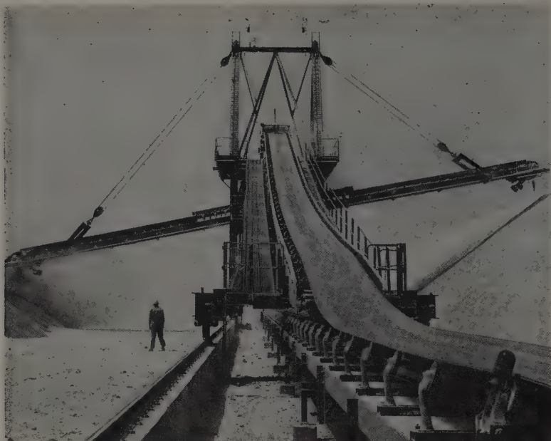
STACKER delivering material to one or two boom conveyors building piles 36 ft. high and 517 ft. long, or about 35,000 tons. This stacking operation is interlocked with the secondary crushing and must be running before the crusher will start.
