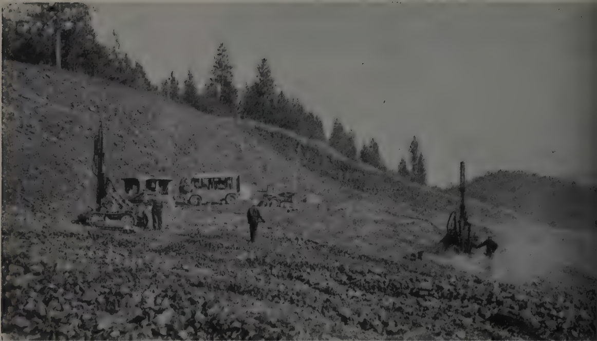
CRAWLER drills on basalt outcrop outside Coeur d'Alene. Half-pound of powder per cu. yd. dices the rock without damage to nearby houses.
