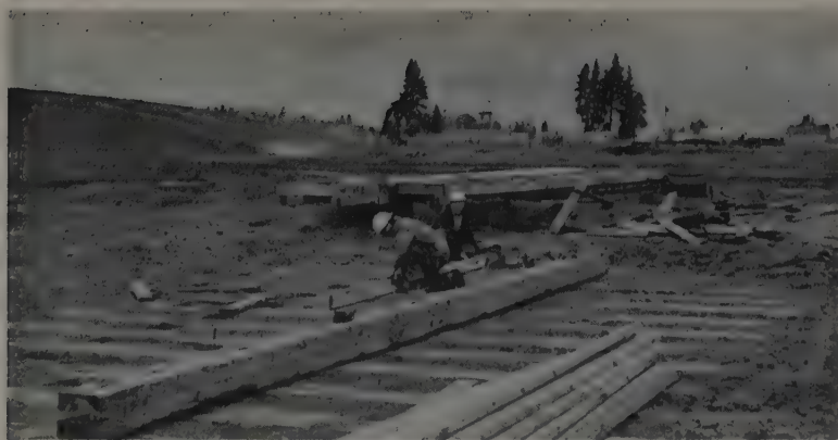
CARPENTERS set up forms for reinforced bridge members on timber casting bed near job site. Forms can be nailed directly to the imbedded timbers. Steel cages for beams in background.
