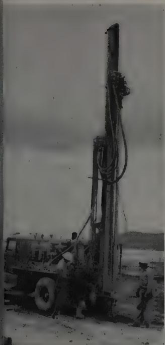
DUTY drill equipped for percussion drilling produces 4\frac{3}{8} -in. hole.
