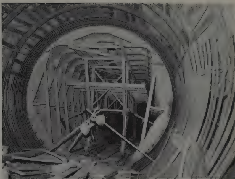
LINING diversion tunnel with concrete is under way now with Blaw-Knox steel form 48 ft. long. Rail-mounted dolly carries form and hydraulic rams collapse it when it moves ahead.
