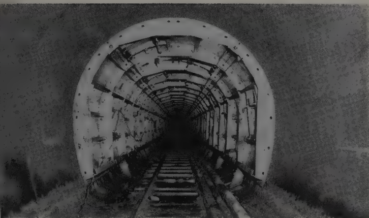
COMPLETED LINER, with forms stripped away, shown in foreground. Both vertical and sloping forms were used and proved equally satisfactory. Placement averaged 265 cu. yd. per day.
