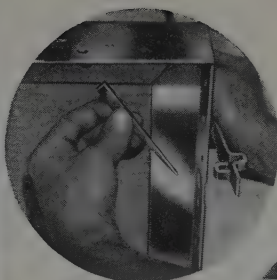
1. UNI-FORM Tie Loop placed in square tie hole of Panel.
