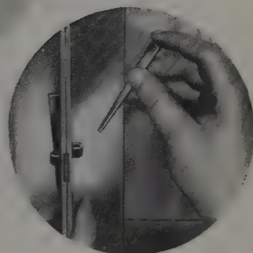
3. Next UNI-FORM Panel is placed in position. Tie Loop automatically enters square tie hole. Key is dropped in—assembly is complete. NO COMING BACK TO "FISH" TIES.
