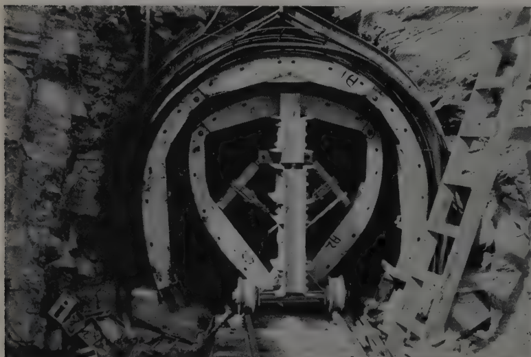
MOVEMENT of one arch form through another is clearly shown. One form is in position against tunnel ribs, while other with hinged sides fully retracted rides through on hydraulic dolly.
