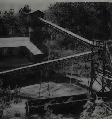
CLEANING ORE. U. S. Pipe ore cleaning plant at a mine where ore is crushed and passed through separators to float off impurities.
