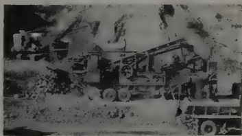
Lima Austin-Western portable 101-SE crushing and screening plant with mechanical feeder is served by 1-yd. Type 44 Lima shovel.
