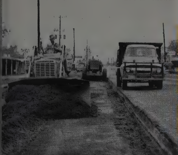
No. 955 excavates part of a total of 19,000 yd., preparing for base an area 20 ft. wide, 12-13 in. deep. Cuts are made by Cat No. 12 Motor Grader and windrowed. Job is part of a $1,828,366 project by Gulf Bitulithic Co. on U. S. 75, to be part of the Interstate Highway System.
