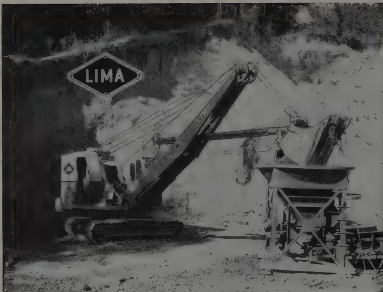
Crawler-mounted Lima Type 44 1-cu. yd. shovel loads sand and gravel into automatic feeder of Lima Austin-Western 101-SE Crushing and Screening Plant.
