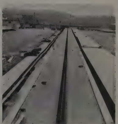
PRESTRESSING bed at Spokane Premix Co. set up for roof beams. Length is 462 ft.
