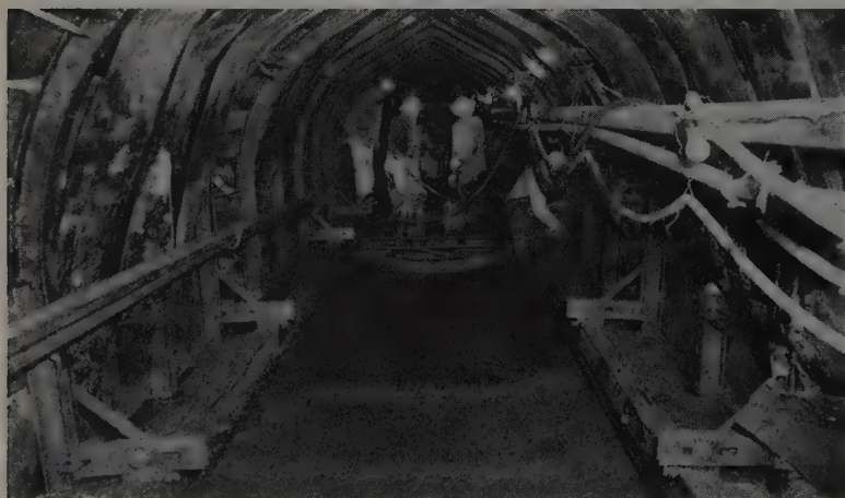
PLACING INVERT. Slip form in center moves along tunnel guided by steel side forms. Side forms made of welded steel channel are attached to tunnel ribs by adjustable supports.
