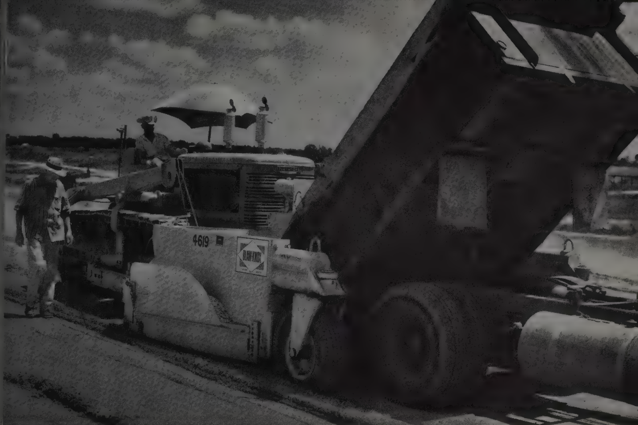
Blaw-Knox P-160 at work on Interstate By-Pass 35 outside Oklahoma City. Pugmill mix was laid down to 8-inch depth, 14-foot width at a rate averaging better than 600 TPH.
