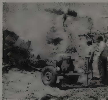
STUMP BURNER devised by "Chick" Dwyer (with hat), construction superintendent of M. W. Brown Co., Redding, Calif., examined by Dwyer and R. J. Felton, California Highway Division construction engineer. Burner consists of a salvaged blower fan driven by a small gasoline engine. Air stream directed at base of stump pile speeds burning and keeps hot fire going.
