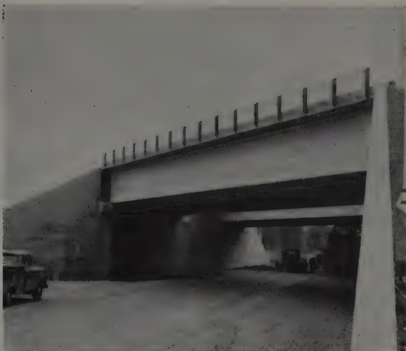
PRESTRESSED girders , 99 ft. long, are used in this overcrossing. Job included 124 prestressed beams, the first such application in Idaho. Beams were poured in Spokane, 32 miles away.
