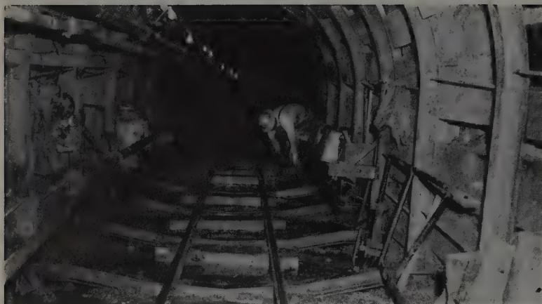
CLEANING invert. Loose material was hand shoveled into skip feeding slusher-loaded cars. Only a few tunnel ribs had to be re-aligned from original placement.
