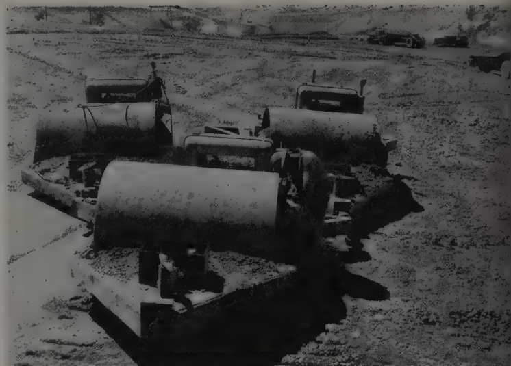
COMPACTION of Zone 2 material is speeded by this trio of Essick steel drum vibratory rollers drawn by a single crawler tractor. Results are excellent and there is less equipment on the
