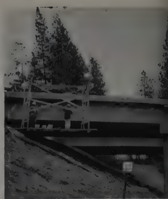
MONORAIL scaffold speeds stripping forms from beneath bridge sidewalk.
