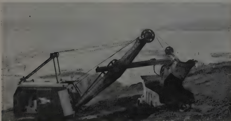
BLAST ROCK and dirt shoveled into 18-yd. Euclid by Manitowoc 3600 with 3½-yd. dipper. Lake Coeur d'Alene and lumber mill in background. This cut involves 900,000 cu. yd. of blasting.
