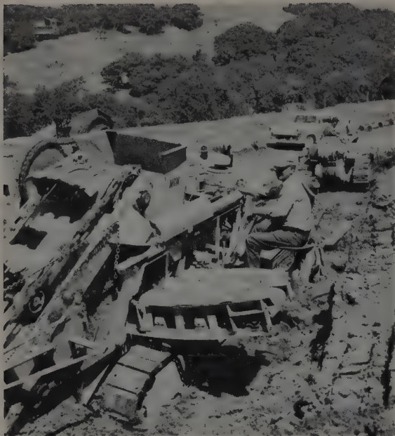
MUDHOLE caused by underground spring makes tough going for trencher which gets extra pull from tractor. Cave-ins are likely here.
