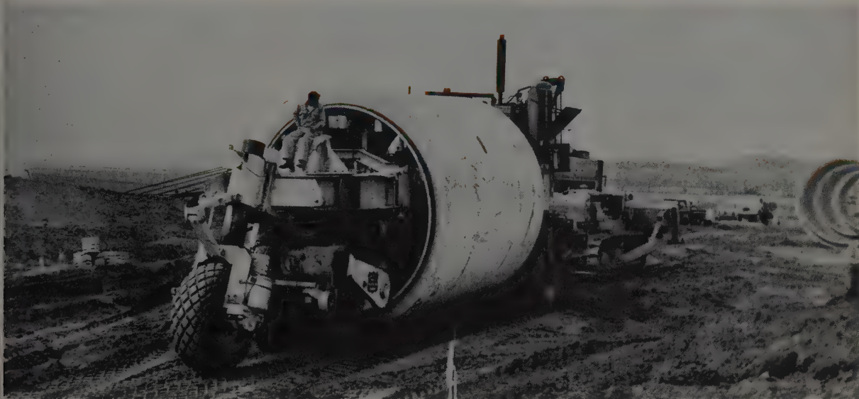
PIPEMOBILE, carrying a 63-ton pipe section, moves down ramp to bottom of trench. Nose tire and double front tires are raised and
