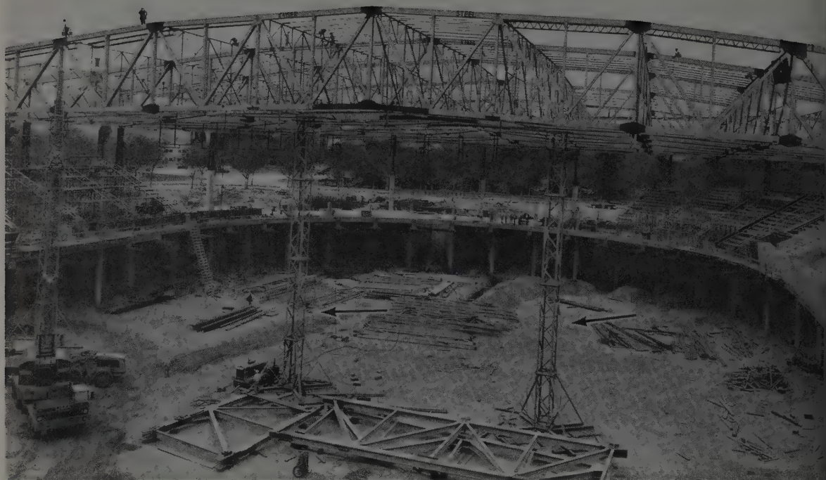
FALSEWORK TOWERS (arrows) made of angle iron were used to support truss sections until field connections were made with high
