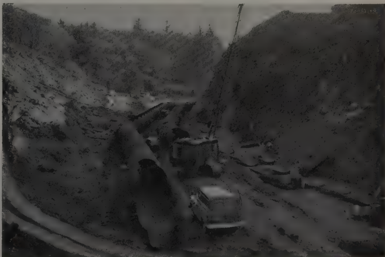
CULVERT under construction rests on random fill above original stream bed. Road fill will be placed over double structure. Photos all show same fill at Burnt Hill Creek on the Oregon project.
