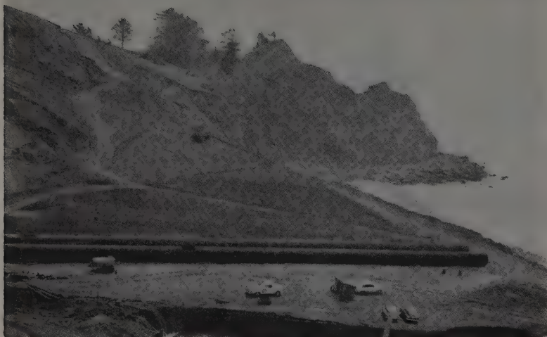
HOOSKENADEN Creek, draining part of the 250-ac. slide area will flow through these two 8-ft. diameter multiplate pipes. Channel will be filled in, and extensive fill placed over pipes.
