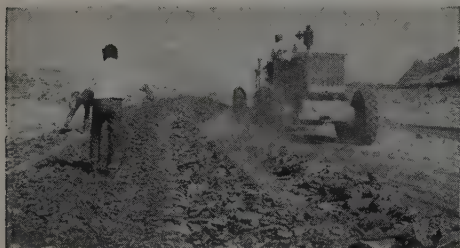
Old asphalt cake is ripped up for pulverization and re-processing by the Seaman-Andwall TRAV-L-PLANT.
