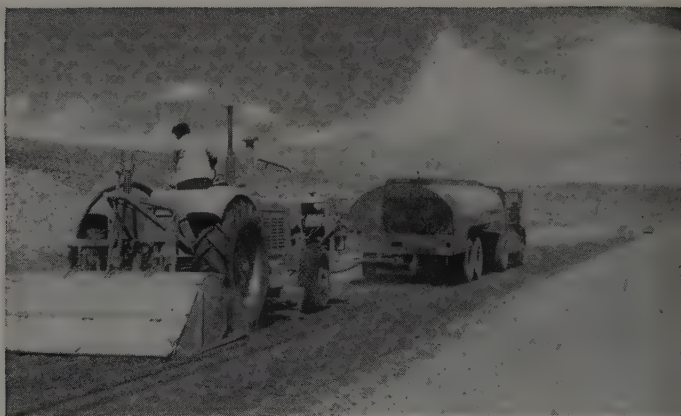
Wet mixing and water admixture are performed simultaneously with the Seaman-Andwall TRAV-L-PLANT.
