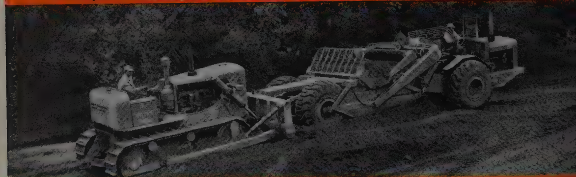
TS-160, heaped loads in 20 seconds, 9½ yards heaped
