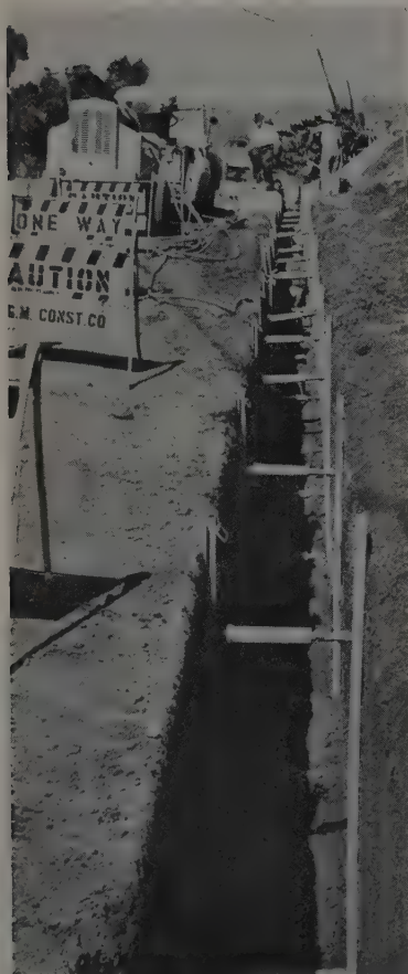
SHORING in place and ready for pipe laying. Note the bulge on the nearest shore.
