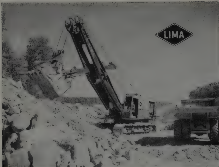
Lima 1250 3½-yd. Shovel nears end of million-and-a-quarter-yd. excavating job on highway reconstruction project near Knapp, Wis.
