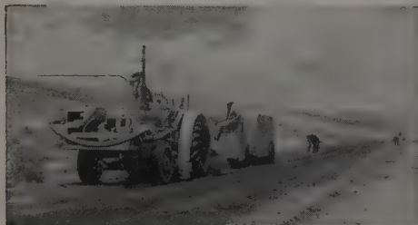
Rolling by Seaman-Andwall 5620 pneumatic compactor closely follows the final mixing pass of the TRAV-L-PLANT.
