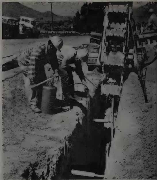
PRESSURE is applied quickly by a hydraulic pump that actuates both jacks. Installation is made from the top of the trench.
