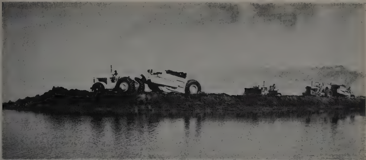
EARTHMOVING equipment advances first stage of Willard Dam across a shallow arm of Great Salt Lake. Dam will create a fresh-water reservoir.
