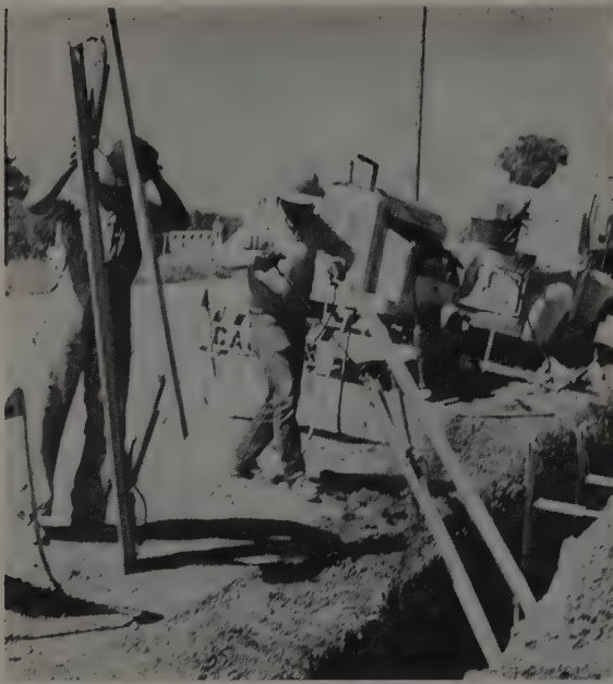
CARRYING and placing is a 1-man job. Each pair is a complete unit. With extension rods shores can be used for a 72-in. trench.
