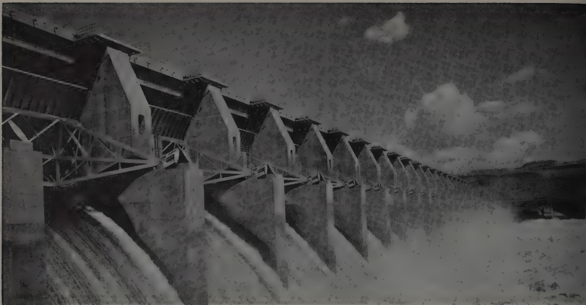
FROM wet-to-dry and from cold-to-hot, exposed steel on a hydroelectric project represents a problem in selection and application of protective coatings. Modern materials are providing better service. Vinyl type of paint was used on these spillway gates at The Dalles Dam, built by the Corps of Engineers.
