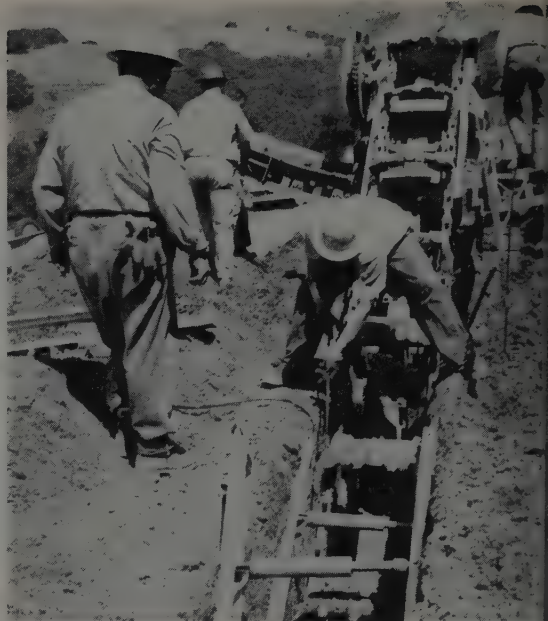
SPECIAL placement of shores on diagonal directly over boom prevents cave-in of slippery ground as trench cuts through the mudhole area.
