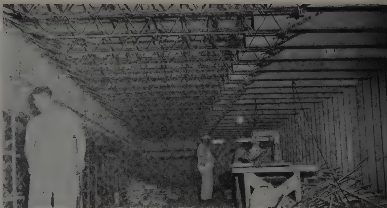
WORKING and storage space provided by Beatty horizontal shores which eliminate vertical shoring is put to good use in city lot building by Oakland contractor.
