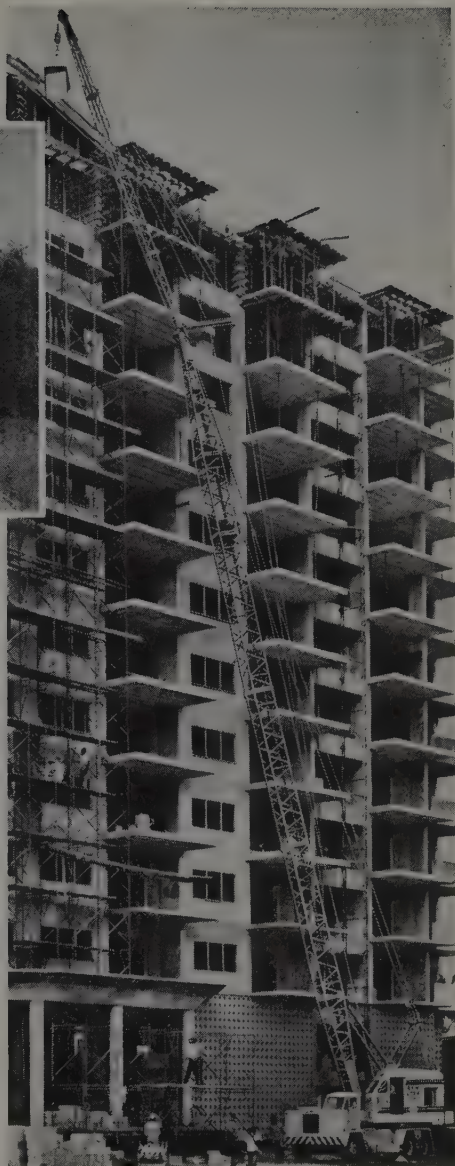
Construction of cast-in-place sections of Miami, Florida hotel called for long reach and pin-point precision. The contractor got both with this Gar Wood truck crane.
