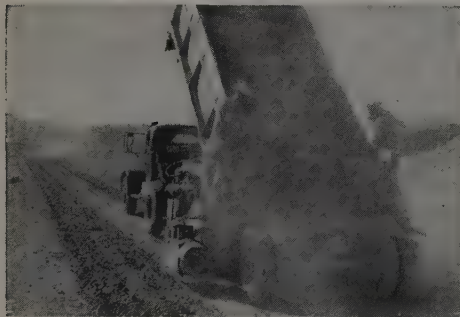
Cement is spread with Seaman-Andwall mechanical Spreader.
