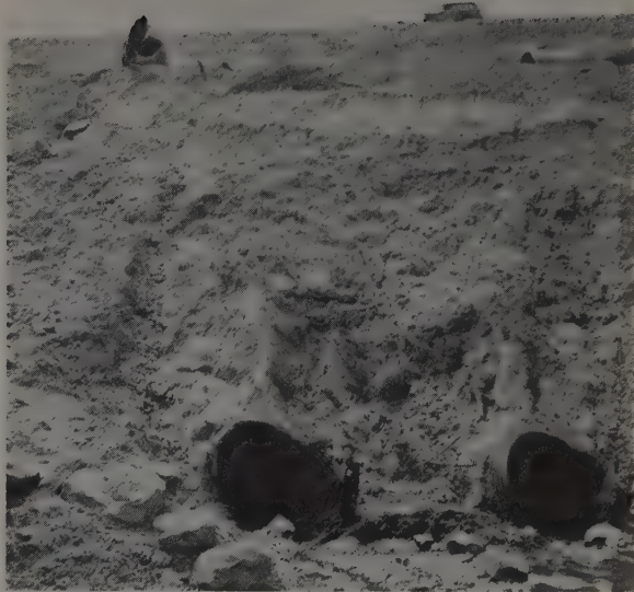
THE FILL as it now looks. Remains of pipes can be seen on shelf above. Same area under water shown at extreme left.
