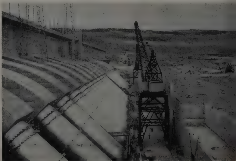
INSIDE coating on these sixteen 25-ft. diameter penstocks posed a preparation problem on the 42-deg. incline. Mechanized equipment for sand-blasting reduced time required and improved the condition of the steel surface, as compared to older hand methods. Penstocks are at Chief Joe Dam built by the Corps of Engineers.
