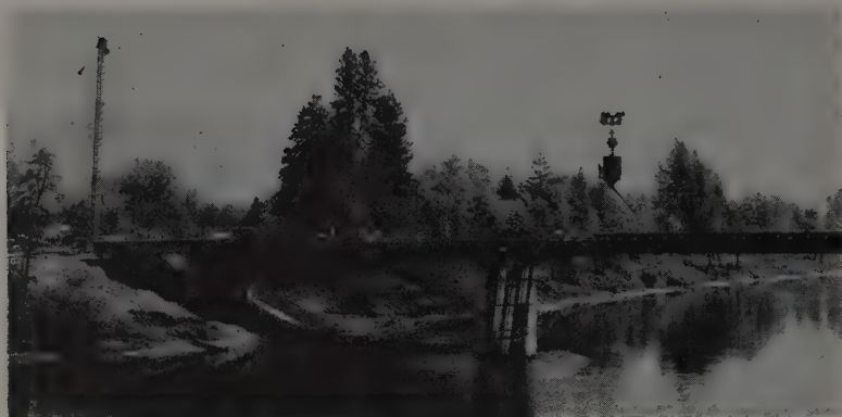
FOUR-YARD bucket attached to cableway brings concrete for bridge deck. Highline was set up to place steel bridge girders which were cantilevered out from hollow concrete piers, and welded.
