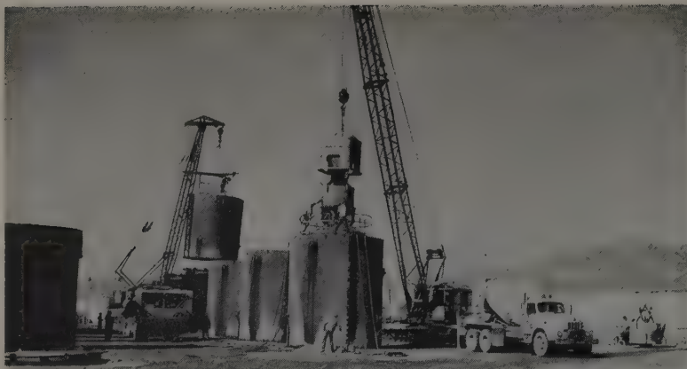
SCENE AT CASTING YARD. At left edge of photo a completed section is being steam-cured under canvas "sock." Crane at left is placing outside steel form. Note hammerhead fixture at top of boom to ease handling of wide load. In center, concrete bucket discharges automatically into surge hopper. Operator at hopper keeps concrete flowing evenly over steel cone into space between forms. Batch plant is several hundred yards away.
