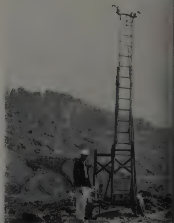
EXTENSION ladder on generator trailer. Twenty-foot ladder can be operated by one man.
