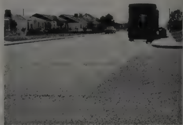
IN ADDITION to improving appearance, leveling the surface and reducing raveling, slurry seals prevent further oxidation and make streets easier to wash and maintain.
