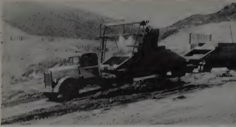
WATER SPRAY is applied to loads as trucks leave pit. Spray helps stop dust and spillage, important because trucks travel city streets. Material is light, but loads can't be heaped.
