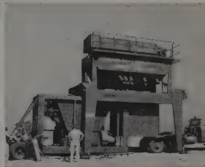
3 MIX-AND-WEIGH SECTION IS MOVING INTO PLACE.
