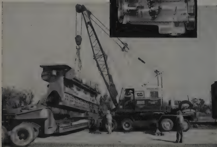
Powering Crane (boom)—140-GK Waukesha Gasoline, six cylinders, 4½-in. x 5½-in., 525 cu. in. displ.
