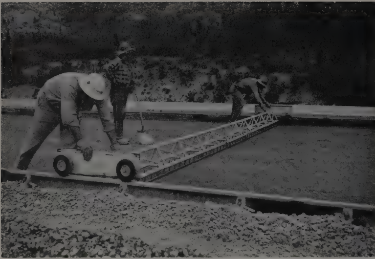
SCRATCH TEMPLATE checks final subgrade depth. Man with shovel corrects small irregularities. Photo taken on Floriston job, first 24-ft. wide paving project undertaken by Gordon H. Ball.
