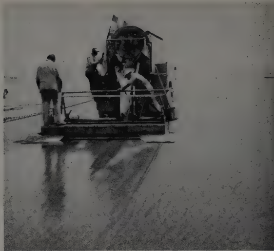
JOINTS between two applications present a problem sometimes, and one solution is to drag weighted sacks along attached to the corners of the spreader box, as shown.
