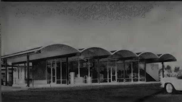
Multiple arch roof composed of curved components creates unusual and attractive profile. Panels have 5/16" upper, 1/4" lower plywood skins glued to 3/4" honeycomb paper core, with 1 x 3 framing.
