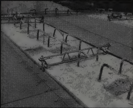
↑ PRESCON HANGERS with deck forms in position. Safe working loads up to 10,000 lbs.
