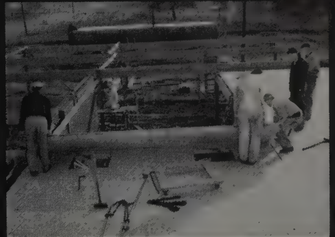
Flat stressed-skin panels used on rear section of the building have 1/2" upper, 3/8" lower Exterior fir plywood skins glued to light lumber framing.
