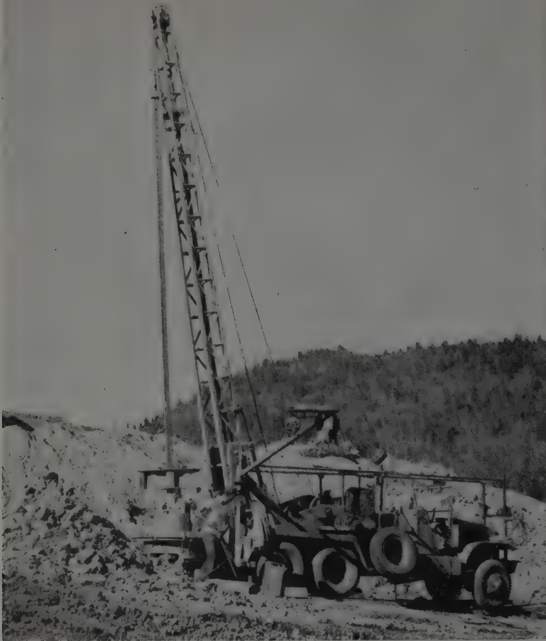
BUCKET auger drill rig set up by contractor on Dunsmuir site prepares to sink a 40-ft. drain well.
