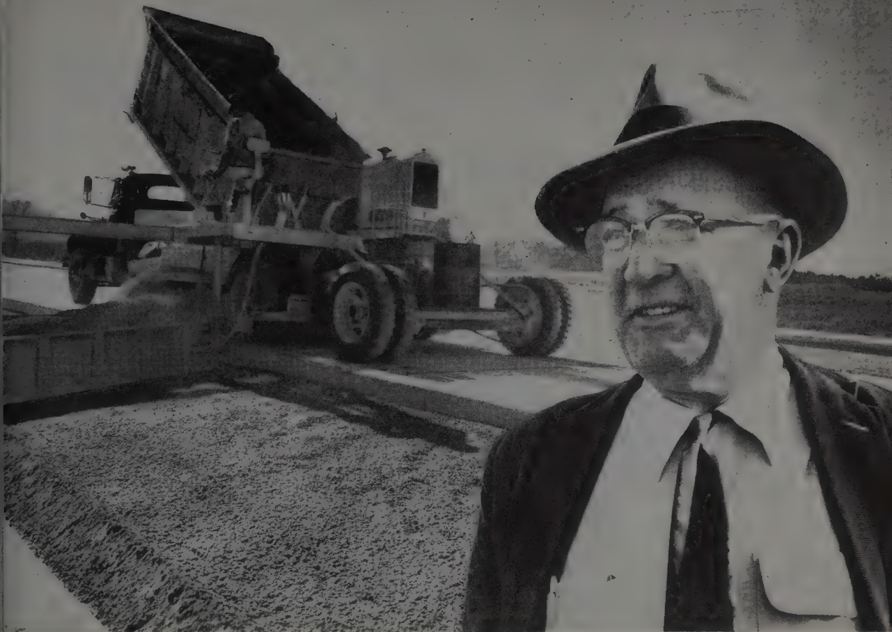
Blaw-Knox Road Widener lays aggregate for shoulders in conversion of U.S. Highway 31 to Interstate Highway 65 near Birmingham, Alabama. A. E. Burgess Company bought the Blaw-Knox machine especially for the 250,000-yard job.
