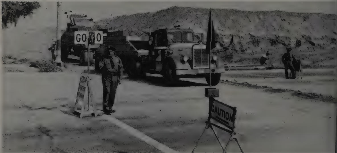
UNIFORMED GUARDS control traffic, an important contractor innovation. Atkinson found that traffic is much more easily controlled by
