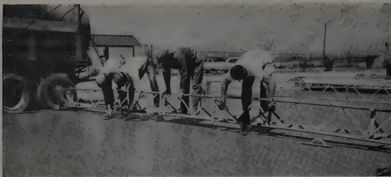
FINISHERS work from bridges that span between the trailing forms. On this first bridge two men are cutting the wire mesh at joints which later will be sawed.
