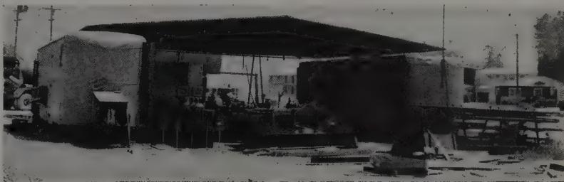
MAINTENANCE YARD on Kiewit job consists of two parts-vans spanned by light roof. Trucks are cared for in one yard, other equipment in another. Both are models of efficiency.
