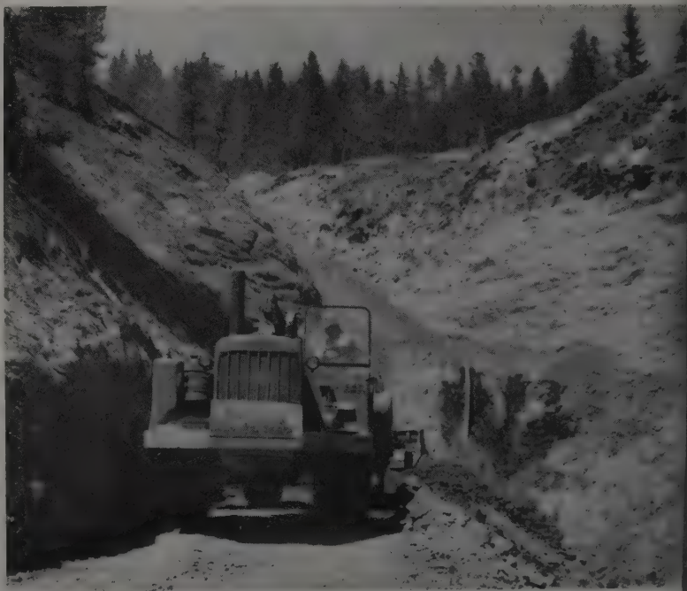
OUTLET for stabilization trench descends ravine too steep for earthmovers, and must be backfilled from haul road. Portion of drain pipe can be seen at right of scraper.
