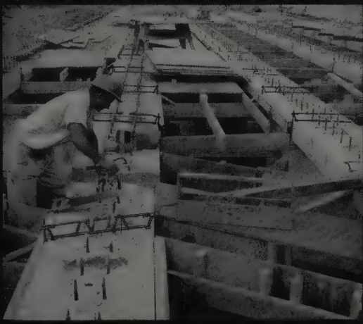
↓ WITH SUPERIOR PRESCON HANGERS the necessary adjustment to bring the deck form up to grade is made conveniently from the TOP.
