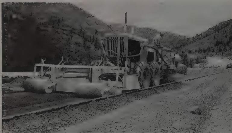
WOOD MIXER travels over windrow after cement is placed by bulk cement dispenser. Attached to travelling mixer is a spreader which levels mixed windrow to plane surface 12 ft. wide.
