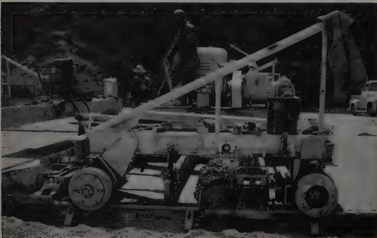
BLAW-KNOX transverse finisher follows spreader. Finisher has two transverse oscillating screeds and a tamping bar. This machine is self-propelled and has 10-ft. wheelbase.
