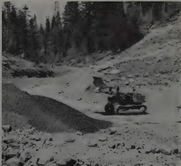
GRAVEL placement in trenches is done with loader which piles rock against steep side. Trench then is backfilled to that level.
