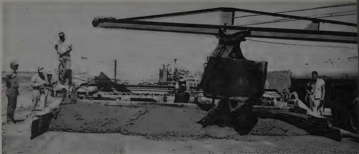
FRONT end of paver moves ahead without the usual forms. Concrete is spread by a hydraulic ram followed by a vibrator. A cam-actuated tamping bar follows, moving just ahead of the screed.
