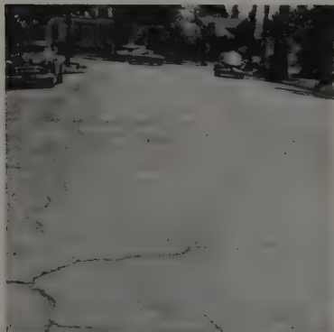
WITH squeegee riding on the surface, the slurry seal fills cracks and minor depressions, but wipes the high spots clean. After about six months of wear and weathering the surface tends to have a mottled appearance.
