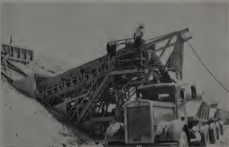
KO-CAL belt loader on Atkinson job loads Kenworth truck with tandem trailers. Loader hopper is fed by six crawler tractors. Belt operator signals truck driver with loud auto horn.
