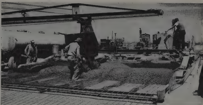
INNOVATION of last season by contractor Roberts-Western was this sled pushed ahead of the paver. This device allows reinforcing mesh to be inserted in the slab.
