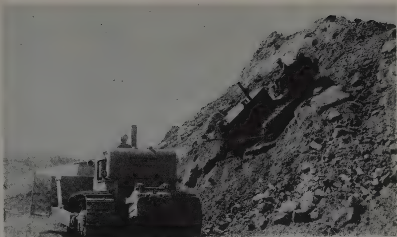
DOZING BOULDERS away from belt loader is job for these two Cats. D9 at left has largest dozer blade available. Specs allow rocks up to 2 ft. in longest dimension to go in fill.
