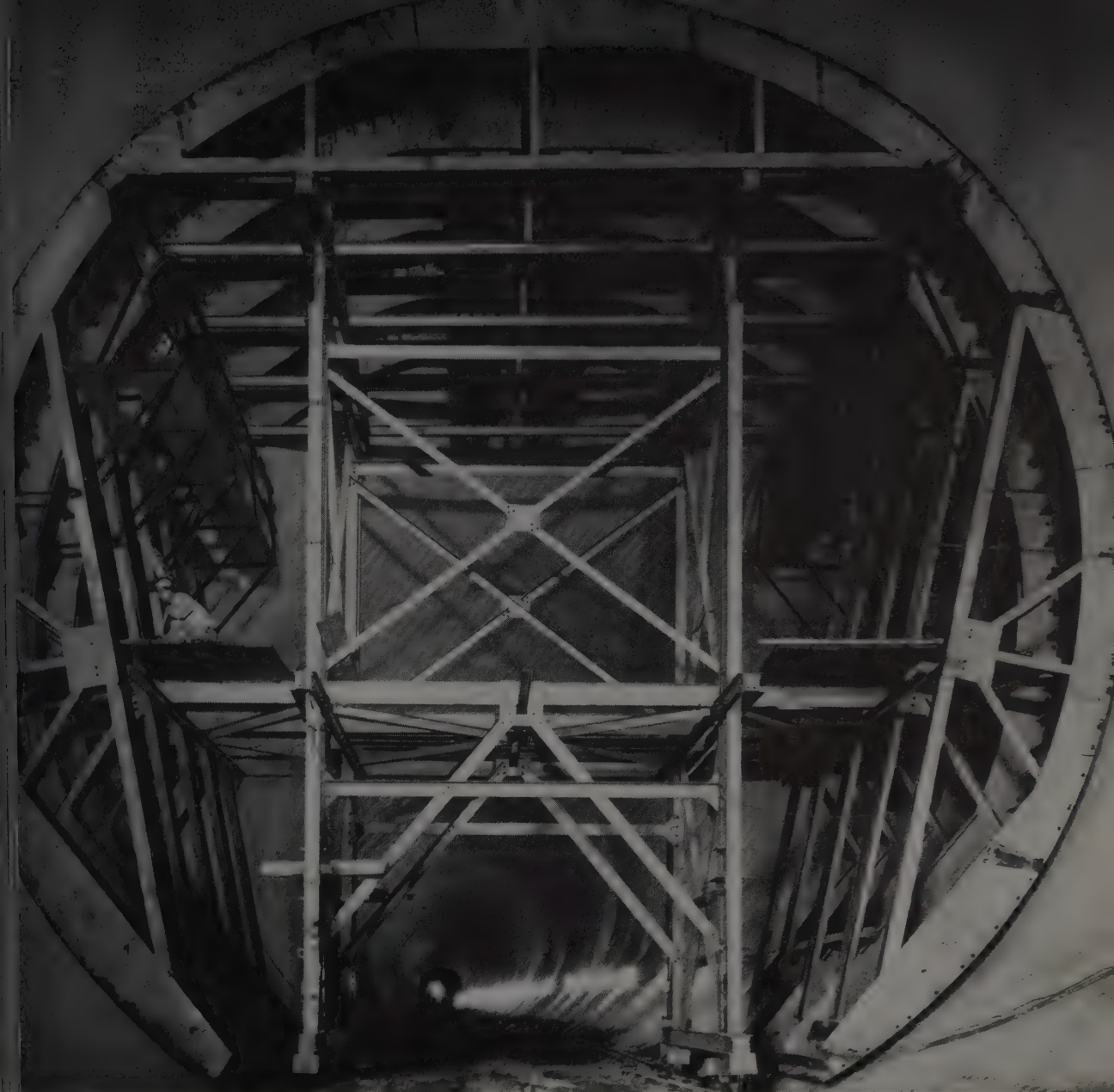
60-foot long Blaw-Knox tunnel form in position inside east diversion tunnel at Glen Canyon Dam. Each linear foot of the 33-inch tunnel wall required 20 cubic yards of concrete. Blaw-Knox Forms consistently met accuracy requirements.
