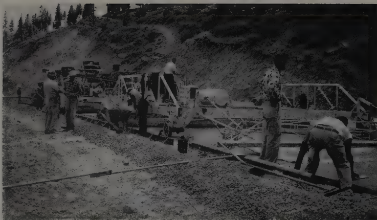
FINAL FINISHING is performed with a Lewis longitudinal float. Machine has 30-ft. wheel base and two oscillating screeds suspended midway. Note burlap drag at right above.
