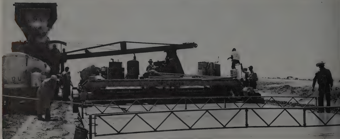
FRONT end of paver moves ahead without the usual forms. Concrete is spread by a hydraulic ram followed by a vibrator. A cam-actuated tamping bar follows, moving just ahead of the screed.
