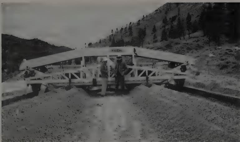
WINDROW SIZER made by Koehring of California is first machine in wide paving train. It shapes subgrade material into two windrows with trough for cement, and discharges excess.
