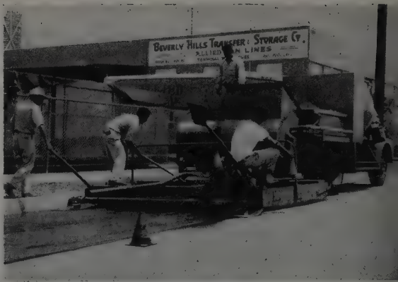
IN MANY localities the mixing is handled by mounting a pugmill on the back of a maintenance truck. Tanks of water and emulsified asphalt also are carried on the truck and proportioned by volume. Over-mixing should be avoided.
