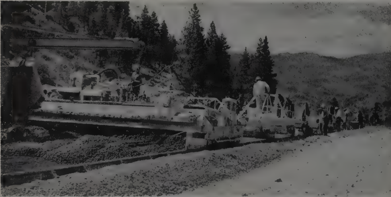
CONCRETE is placed by Koehring paver as evenly as possible in front of Blaw-Knox spreader. Towed by spreader is 25-ft. levelling attachment tried on Floriston project.
