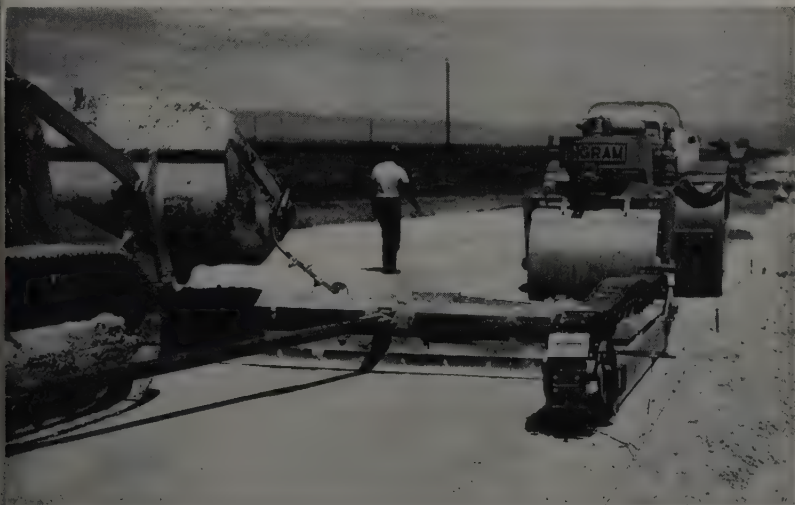
FINAL RIDEABILITY is tied directly to the base and its preparation. This is particularly true since the crawler treads of the paver ride directly on the base. Binder may be needed to stabilize for proper traction of the paver.
