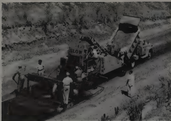
THIS MACHINE, developed by the California-Fresno Oil Co., is essentially a travel pugmill. Aggregate is fed by belt, mixed with the water and emulsion, and then deposited in the slurry box. Note the truck unloading aggregate.
