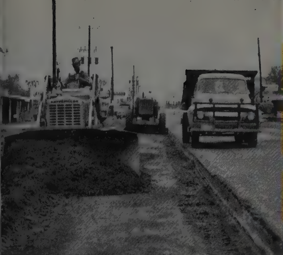
No. 955 excavates part of a total of 19,000 yd., preparing for base on area 20 ft. wide, 12-13 in. deep. Cuts are made by Cat No. 12 Motor Grader and windrowed. Job is part of a $1,828,366 project by Gulf Bitulithic Co. on U. S. 75, to be part of the Interstate Highway System.
