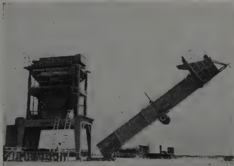
4 HOIST HAS RAISED BIN SECTION AND MIXING SECTION INTO FINAL POSITION. HOT ELEVATOR IS BEING RAISED.
