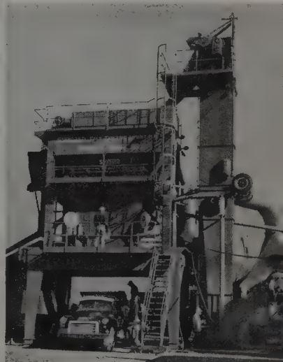
3 MIX-AND-WEIGH SECTION IS MOVING INTO PLACE.
