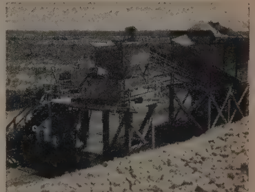
Contractor blends stabilized air strip base materials at Columbus, Miss., air base, with an Eagle Mixer.
