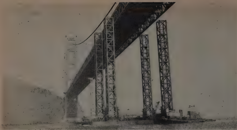
TIGHT SQUEEZE as pipe-laying platform passes Golden Gate Bridge on way to job. Platform was fabricated and assembled in San Francisco Bay area, then towed 450 mi. to Los Angeles.
