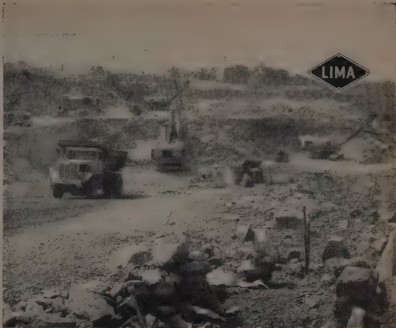
Four of Merritt-Chapman & Scott's seven 6-yd. Lima Type 2400 Shovels are shown working on the excavation site of the Niagara Power Project's main generating plant at Lewiston, N. Y.
