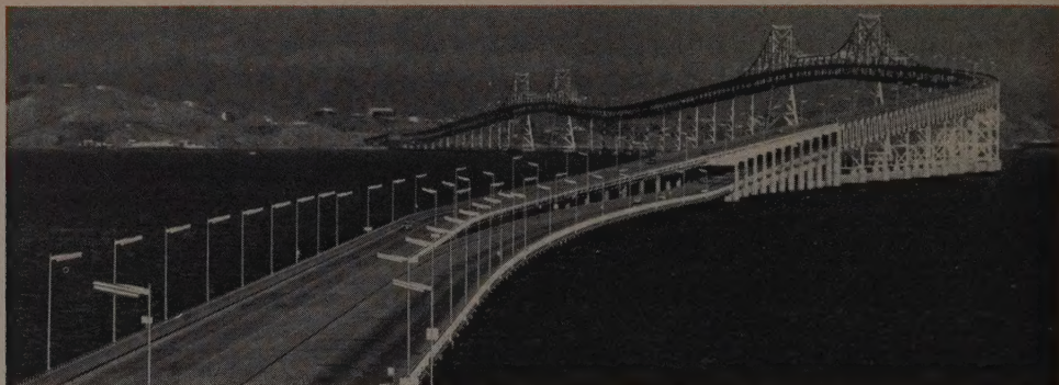
The world-renowned $63 million Richmond-San Rafael Bridge, crossing upper San Francisco Bay, used some 50,000 tons of steel—most of which was fabricated in Yuba plants in the area, and erected by Yuba field crews, including all the trusses on the 36 spans—each 289 ft.
