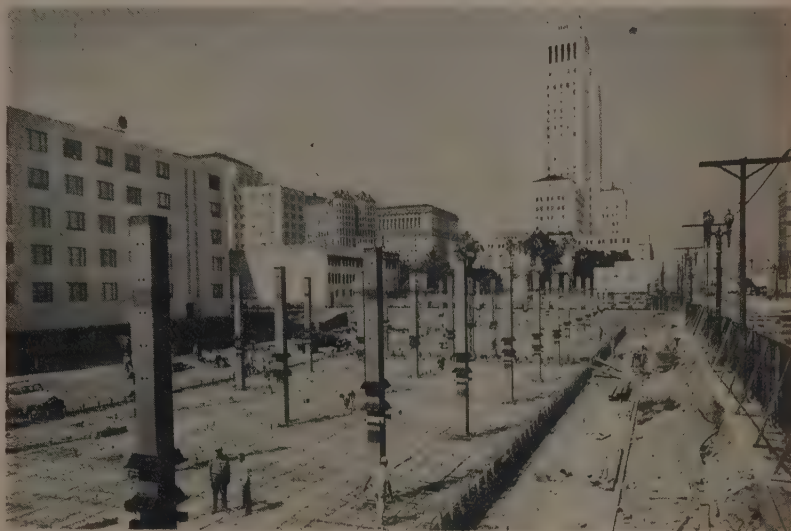
PLACING RE-STEEL and prestressing cables for fourth slab in stack of six is under way. Note collars on columns which will be imbedded in next two slabs. Pairs of holes in columns admit large bolts which temporarily support slabs while columns are extended and jacks reset.
