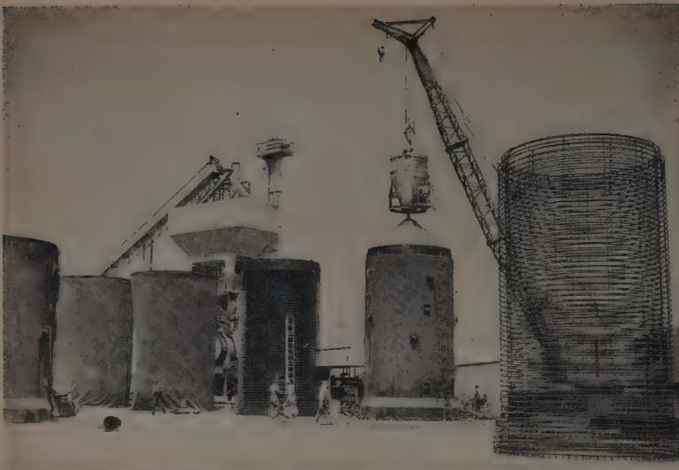
PIPE CASTING at United Concrete Pipe yard. Reinforcing steel cage at right contains one mile of bars. Note operator located on concrete bucket. Steam curing under canvas is shown at left.
