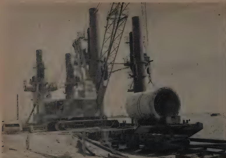
ANOTHER 4-LEGGED PLATFORM stands at dock near pipe-casting yard. Photo shows crane placing section on rail-mounted dolly on platform deck. When eight sections have been placed and all joints tested, platform and pipe "string" are submerged by jacks on legs to permit pontoon to be floated into place above pipe. Then platform is jacked up, lifting pipe and pontoon into position shown in next photograph.
