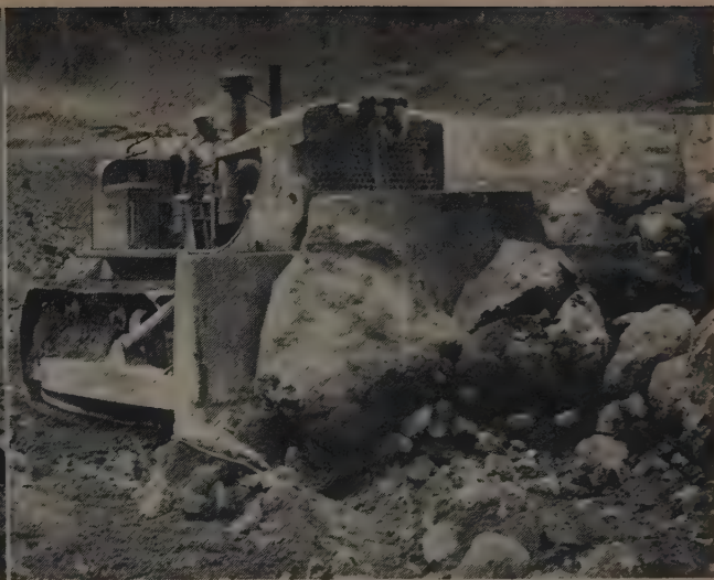
Jones and Tompkins used Allis-Chalmers torque converter crawler tractors to handle the tough dozing work on this, the world's highest earthfill.
