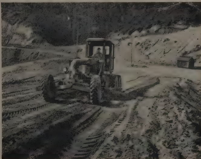
This Allis-Chalmers FORTY FIVE motor grader helped keep the Swift Creek Dam rising rapidly by keeping haul roads and fill in high-speed condition.
