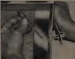
1. UNI-FORM Tie Loop is placed into the square tie hole of Panel.
