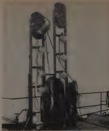
TWO TV CAMERAS observe underwater operation. Cameras are mounted on brackets with four lights each as shown. Brackets are secured to each side of split tremie tube when pontoon is ready to be submerged. Movable tremie tube permits full length of pipe string to be inspected.
