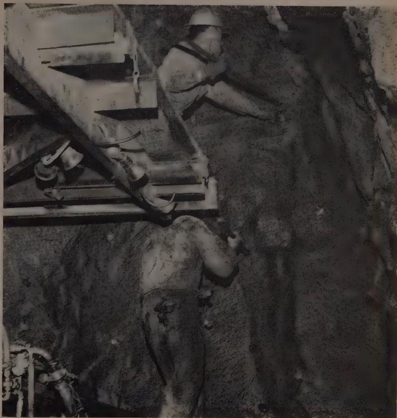
BLASTING POWDER is placed by miners in a pattern which averages about 85 holes with a 3-in. center burn. Combination of millisecond and regular delays was found to give the best breakage.
