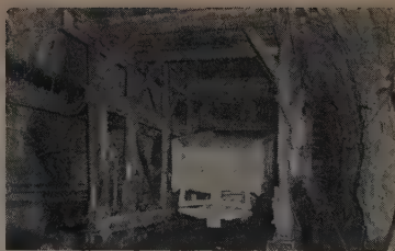
CAR PASSING is done with "cherry pickers" on the gantry jumbos and motorized car-passers behind the mainline jumbo.
