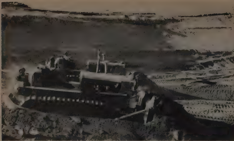
PRODUCTION was speeded in the dozing of loose beach sand and by using two Cat D8's teamed up side by side. About 1,750,000 sq. yd. of finished grade had to be prepared.
