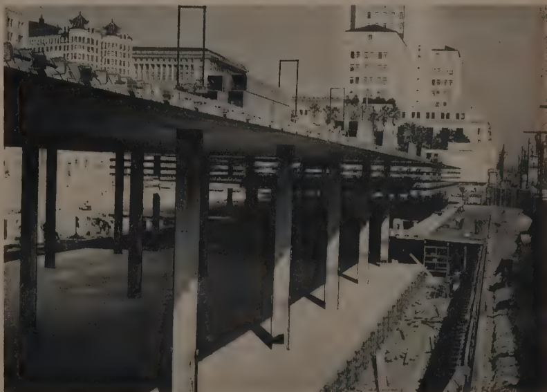
FIRST PHASE of lifting has been completed in background, while in foreground roof slab has been raised to top of first column lift. Note column extensions which ride up on top slab.
