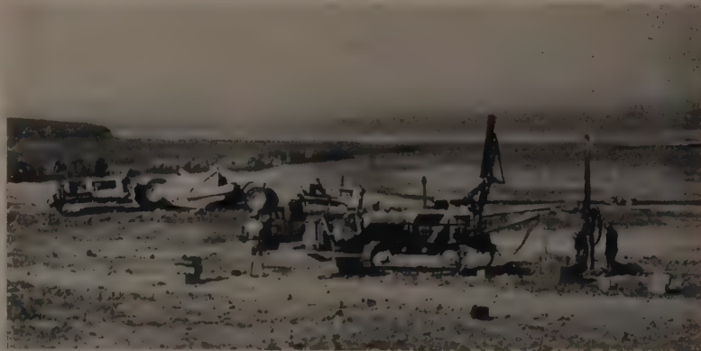
TOUGH andesite rock was readied for blasting by twin drills powered by a 600-cfm. Gardner-Denver compressor, mounted on a Cat D8. Some of the rock was ripped by a D9, which doubled as a pusher to help load D8s pulling Cat No. 491 scrapers in the broken rock.
