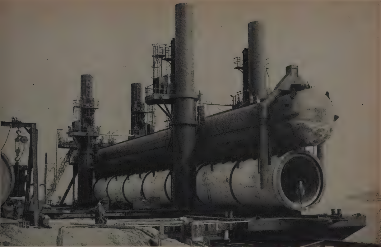
LAUNCHING PLATFORM has been jacked upward, lifting pipe and pontoon out of water so that pipe can be securely lashed to pontoon. When platform is lowered again pontoon with cargo of pipe can be towed away. Note double tremie tube at right for placing ballast.
