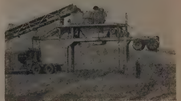
Western Contracting Co., Sioux City, Ia., mixes sand, clay and water producing an amalgam to form the base for concrete slabs and blacktop shoulders on a highway from Omaha to Lincoln, Neb.
