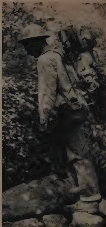
ROCK DRILL weighs only 53 lb., enabling one man to carry it easily over rough terrain.
