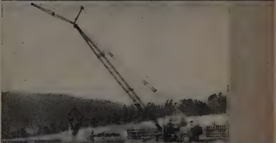
This versatile 35-M is excavating foundations for a $1,600,000 building project on the coast. It carries a 60-ft. boom and 20-ft. jib.
