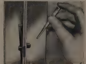
3. Bring next UNI-FORM Panel into position. Insert Tie Key in other Tie loop. Assembly is completed.
