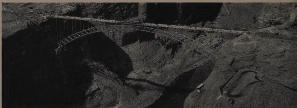
The recently completed Glen Canyon Bridge in Arizona is the world's highest (750 ft.) arch bridge. Completely fabricated and assembled at Yuba's Judson Pacific-Murphy plant, this structure used 4,000 tons of steel, was erected ahead of schedule.
