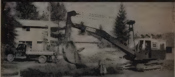
This versatile 35-M is excavating foundations for a $1,600,000 building project on the coast. It carries a 60-ft. boom and 20-ft. jib.
