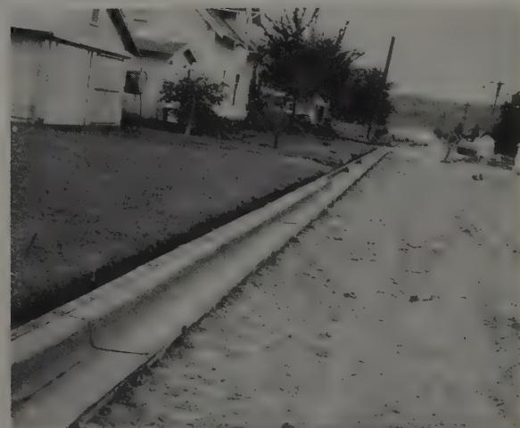
STEEL form curb and gutter. Cost was \$1.35 per front foot and quality was superior to old type. Contractor averaged 2,000 ft. per day.
