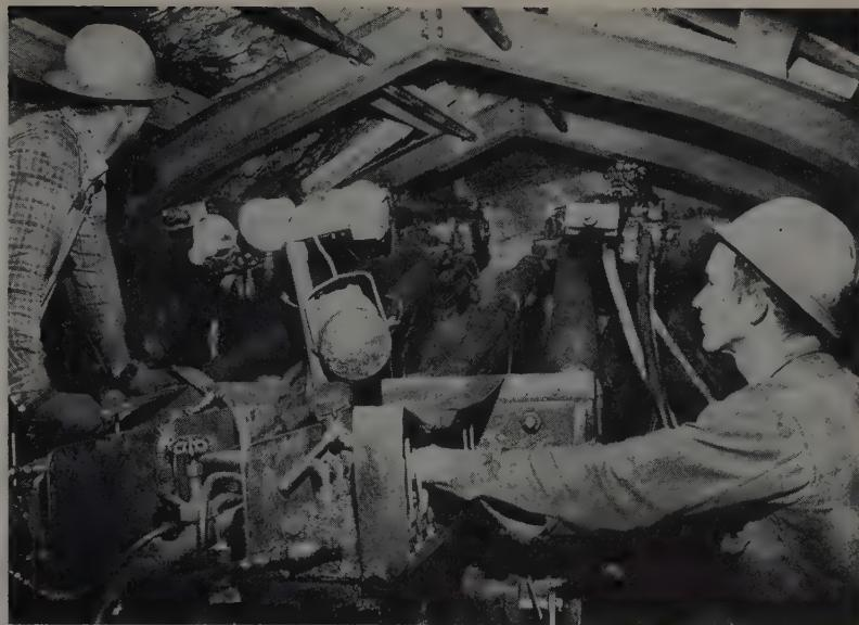
DRIFTERS are mounted on hydraulic jibs and controls are located 20 ft. from the face to keep miners in safe position. Rounds are 10 to 12 ft. without a change of steel. Holes are 1 3/4 in.
