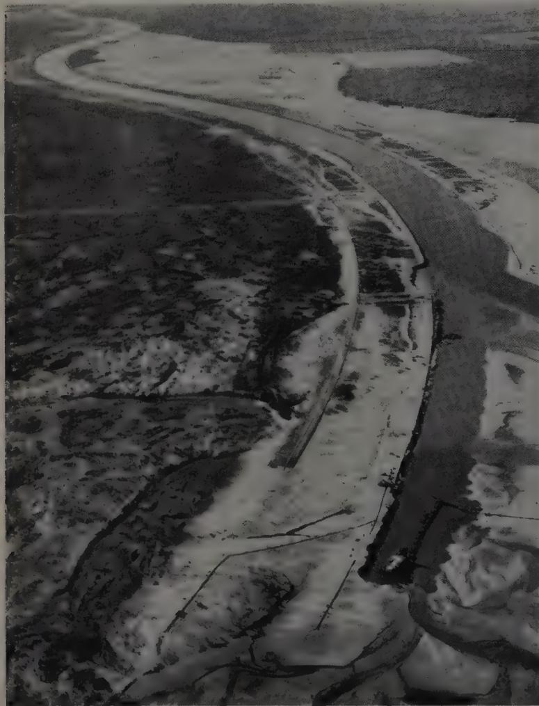
The Colorado River snakes its way southward through a new man-made channel below Davis Dam. This aerial photograph shows the Bureau of Reclamation's dredge "The Colorado" cutting a 400-ft. new channel through the meandering sections of the Colorado River downstream from Fort Mohave.
