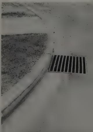
OLD grating in wood-formed curb and gutter. Wide spacing was a menace to bicycles.
