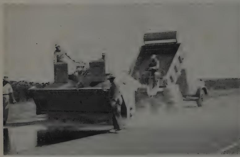
ASPHALT from the Husky refinery at Cody, Wyo. started with a 200 F. temperature at loading, which was maintained during the five-day shipping period in insulated tank cars.
