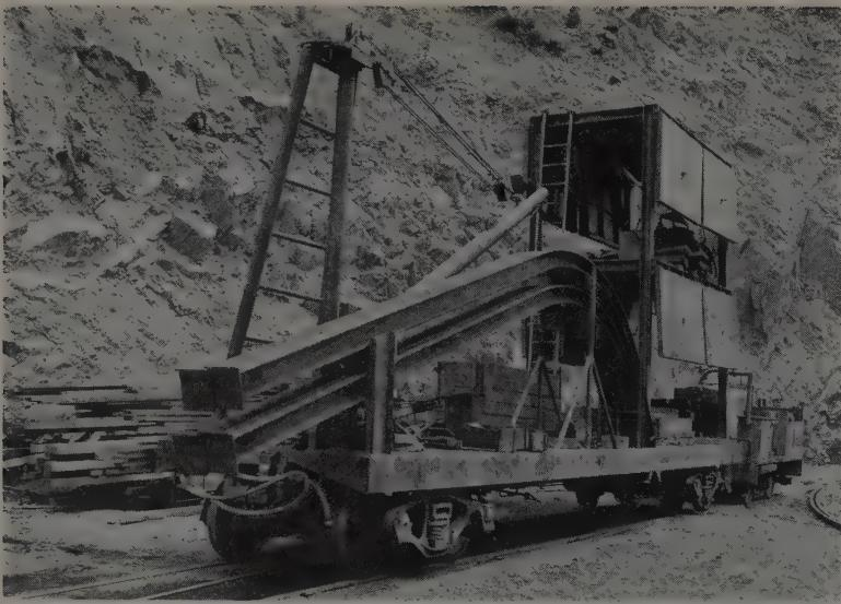
ODD RIG called the "high car" serves two functions. It has hinged platforms used by workmen when installing timber lagging between steel supports and rock, and it has a stiff-leg derrick for installing steel supports which it also carries to the heading.
