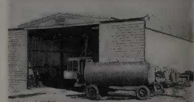
out use of cranes or heavy equipment has been developed by Stran-Steel Corp., division of National Steel Corp. All framing connections of the Stran-Master building are made through factory-drilled holes for bolting. Building is available in widths from 12 to 120 ft.
