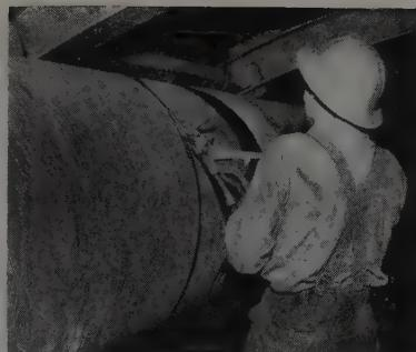
**STEEL STRAPPING**, a common industrial device, is new to tunnel work. Here it is used to attach 3-ft. ventilation pipe to supports.
