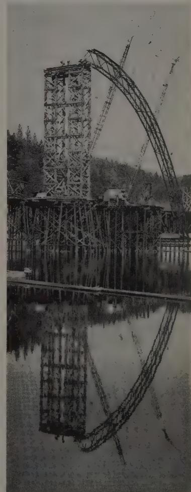
**TWO CRANES** on the construction trestle work together to lift the first section of falsework into place on the temporary supporting tower. Supporting piles for trestle and tower are as long as 95 ft.
