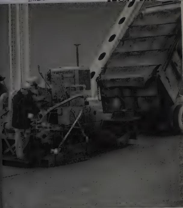
pecially-equipped trucks bring mix to finishers. Insulated truck beds and tarpaulin covers protect mix, bring it to job at best laying temperature. Canvas aprons on spray bars of distributors keep prime from blowing on curbs and sidewalks.
