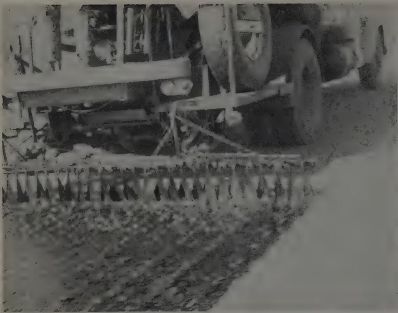
WITH 1½% of natural rubber plus 0.15% dispersed sulfur, this material was placed at temperatures as high as 230 deg., but trouble was experienced with viscosity.
