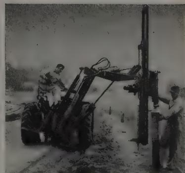
Pneumatractor guard rail driving is one example of its versatility. It also plows snow, sweeps sand or gravel, operates 3-gang tamper or four single tampers, powers a host of air tools.
