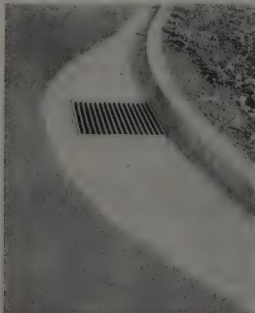
NEW design is safe for small-tired bikes, the equal in capacity and \$10 cheaper.
