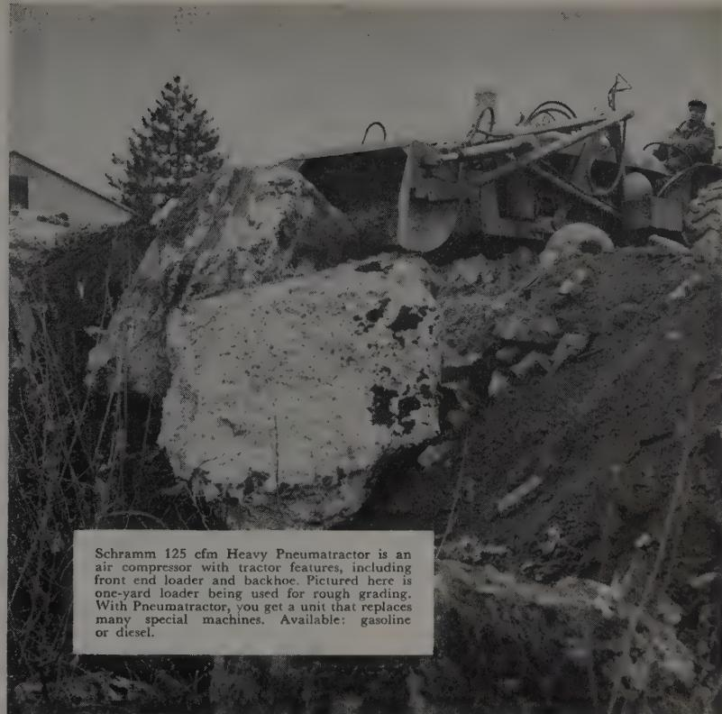
Schramm 125 cfm Heavy Pneumatractor is an air compressor with tractor features, including front end loader and backhoe. Pictured here is one-yard loader being used for rough grading. With Pneumatractor, you get a unit that replaces many special machines. Available: gasoline or diesel.
