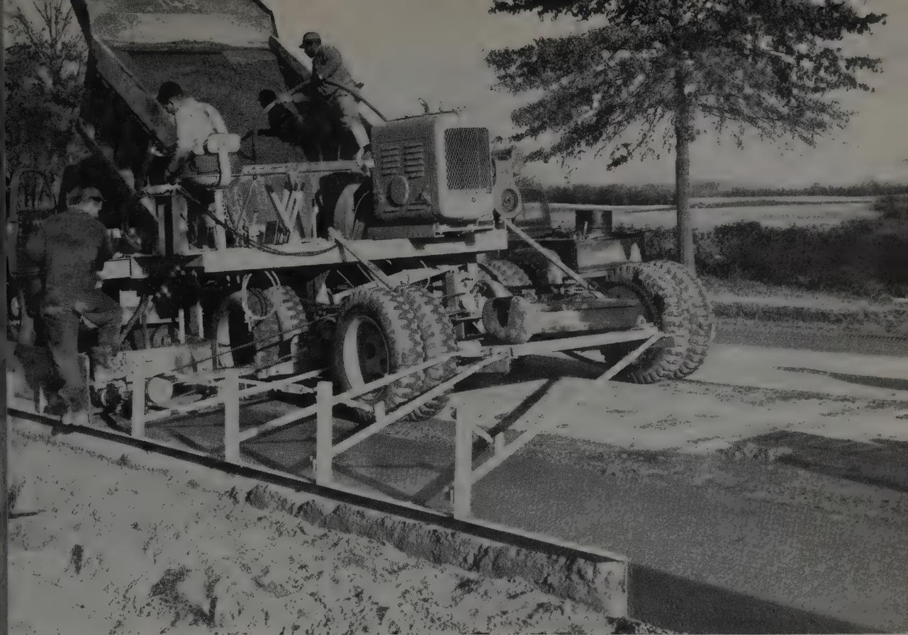
aw-Knox slip form Widener at work on DuPont highway outside New Castle, Delaware. The contract, let by Delaware State Highway Department, calls for widening a 6 1/4 mile stretch of roadway from 20 to 24 feet. Bituminous Mix will be used for resurfacing.
