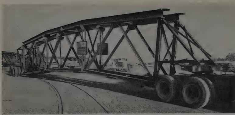
FALSEWORK consists of 8 arches and was brought to job in sections preassembled into pairs. Additional framework at each end of trusses was needed for mounting on truck and dolly.
