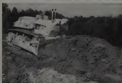
**TC-12 Crawler** has 2 engines and independent track-drive...402 net h.p....full power shift...top speed of 7.8 mph. This "Euc" tractor has unequalled work-ability for heavy dozing, ripping and similar work in construction, mining and logging.
