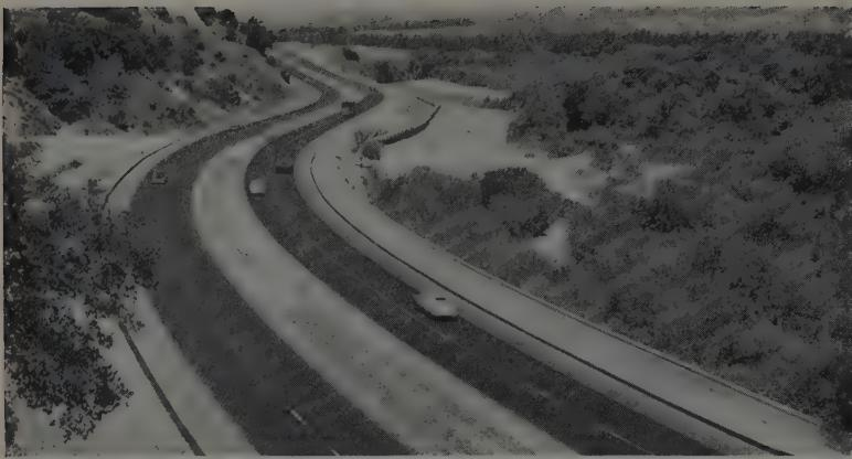
PAVED shoulders can be identified for the driver by use of a seal coat with a distinctive color as shown in this view. This is a common practice of District VII, California Division of Highways. The WASHO Test Road proved that the paved shoulder provided lateral support to strengthen the pavement under the outer wheel track.
