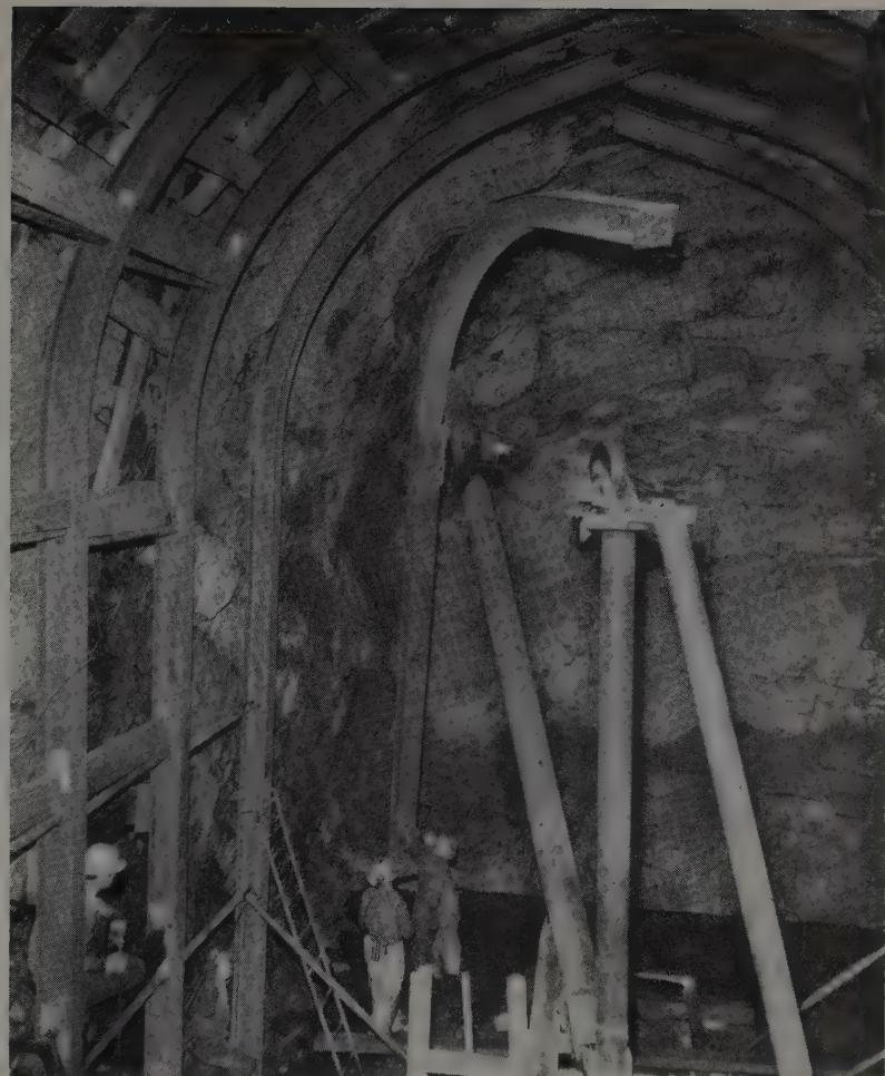
**SETTING STEEL** with stiff-leg derrick mounted at front of "high car." Derrick is made of pipe sections, is powered by three air hoists. Steel is 8-in. wide flange spaced at 6 ft.
