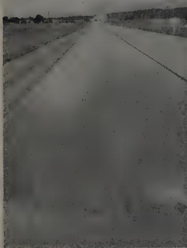
GOOD spread of the natural rubber treated asphalt. Results apparently related to viscosity.
