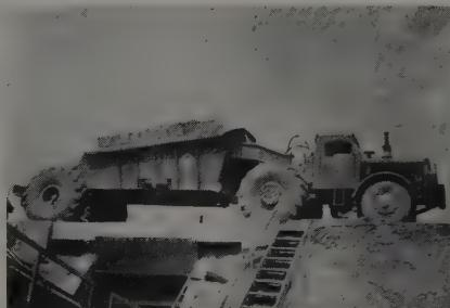
**Bottom-Dumps** carry payloads of 13, 17 and 25 cu. yds. struck...are powered by 218 to 335 h.p. engines...have top speeds up to 34 mph. Full length, unobstructed door openings make these "Eucs" ideal for dumping free-flowing material into drive-over hoppers.
