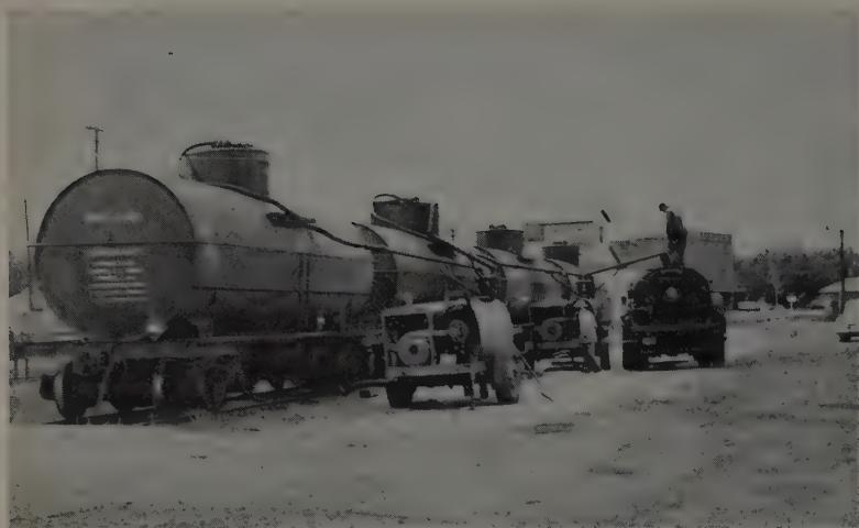
COVERING chips were applied by a Flaherty spreader. Crushed gravel was used on most of the test sections. Equipment and crews were provided by the highway department.
