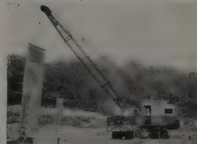
Truck-mounted Lima Type 44-T sets concrete forms for highway interchange near Philadelphia.
