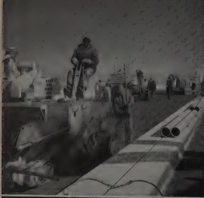
To lay Asphalt concrete on bridge decks in winter the contractor used three, 12-foot finishing machines. By paving simultaneously cold, longitudinal joints were prevented. Finishers were followed immediately by 2-and-3-axle tandems.
