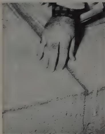
concrete along the joint is retained, infiltration of foreign matter is prevented until the joints are sealed, and blowing out of the joints is eliminated prior to placing the seal. ConSeal consists of two parallel ribbons of mastic set about 1½ in.
