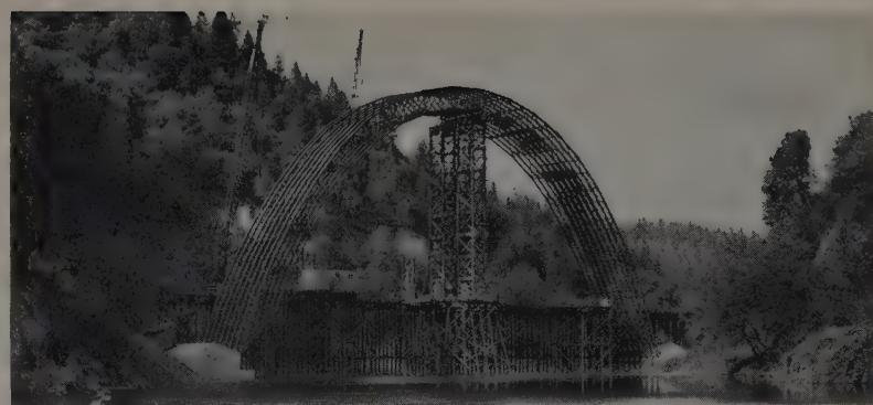
**COMPLETED FALSEWORK** for center span. Fine adjustments in elevation are made by jacking and shimming at the skewbacks and top of supporting tower. Falsework will be re-used for side spans.
