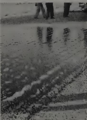
POOR spreading and lack of uniformity produced this result. Cover removed by traffic.
