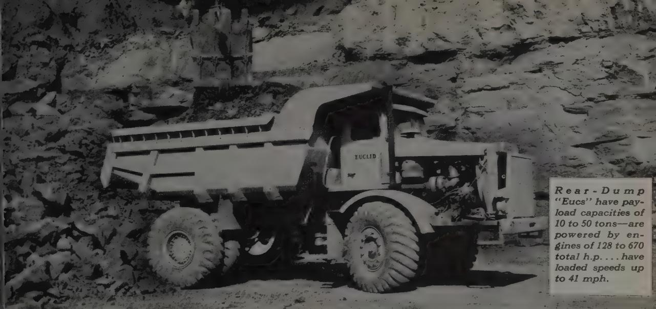
**Rear-Dump "Eucs"** have payload capacities of 10 to 50 tons—are powered by engines of 128 to 670 total h.p....have loaded speeds up to 41 mph.
