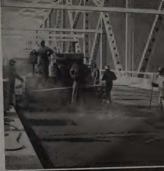
Before and after rolling, luteman, raker and straight-edge man check the mat. Despite 2-inch high expansion and contraction plates every 100 feet, mat goes down true to grade. A 13-20 ton roller irons wearing surface to final smoothness.
