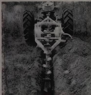
power takeoff and a 3-point hitch can operate this trencher. A special device moves the tractor forward at the correct rate of speed digging trenches from 6 to 14 in. wide. With a forward speed up to 500 ft. per hour, the unit digs a clean trench to a maximum depth of 4 ft. with a boom extension available for deeper trenching. Material is conveyed to the side of the cut with a screw type earth mover. The unit weighs about 700 lb.
