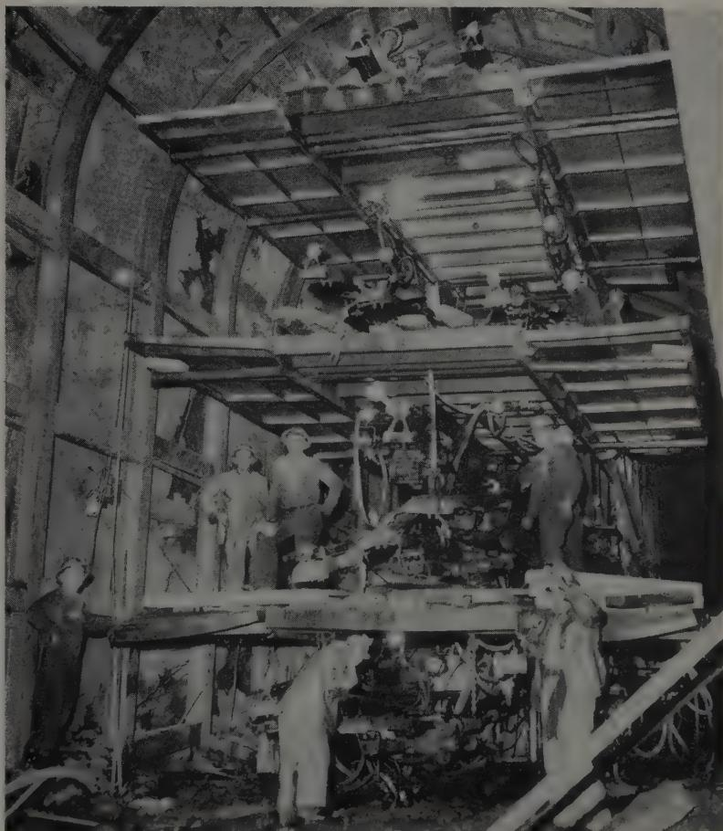
JUMBO with platforms extended easily covers full face. There are eleven drifters on four levels which drill an average of 100 holes per round. In center is 6-in. drill for burn cut.
