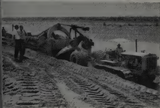
Assistant General Superintendent Buster Morrison and C.I.T. representative Tom Lynn watch a Cat-powered scraper prepare the river bank for surfacing. Cobblestones had to be hauled 42 miles for the job.
