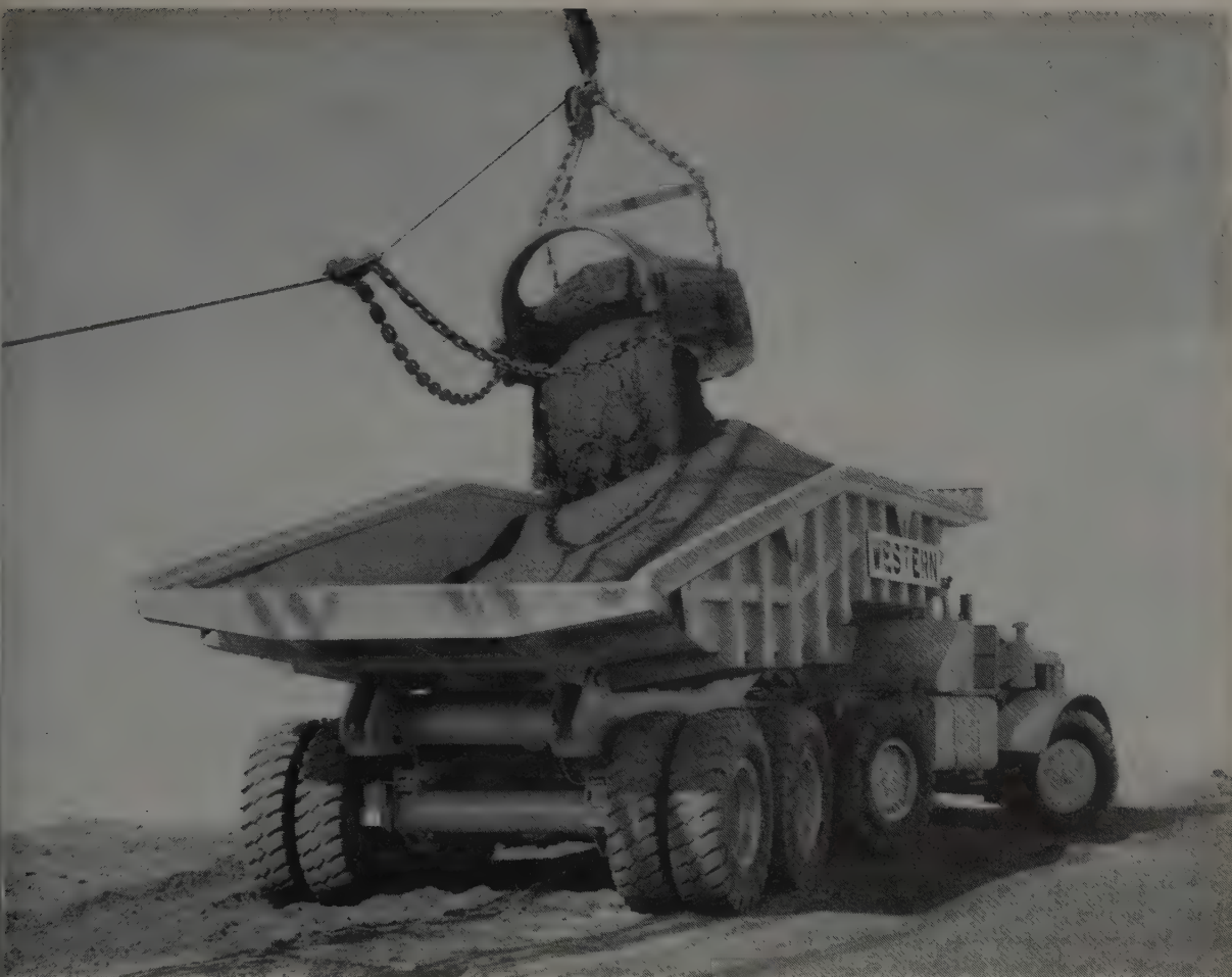
A giant Euclid in action—with a 120-ton haul capacity, the world's largest dump truck.
