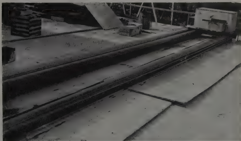
AWAITING next pour is 28-ft. Clary screed. Controls at far end are protected by job-made box. Mechanical finishing speeded concrete work but required heavy rails shown in top photograph.
