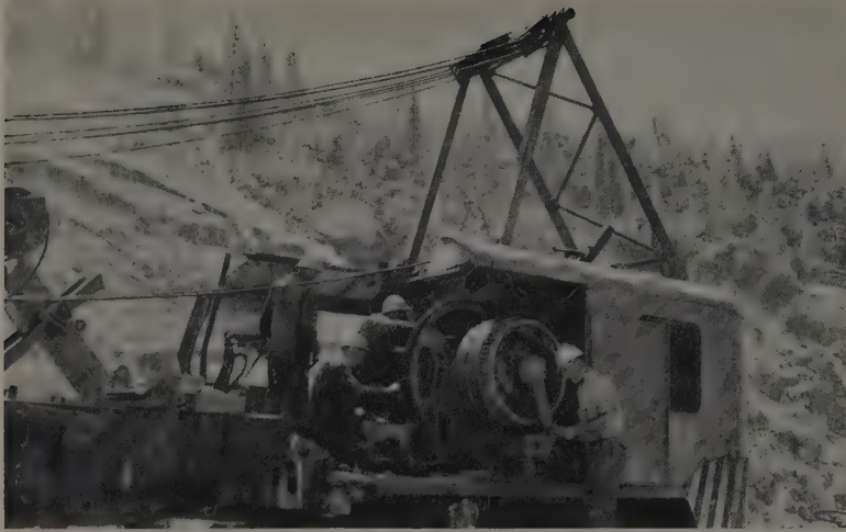
ROUGH GOING causes breakdowns occasionally, but a good maintenance system keeps resulting down-time to a minimum. When repairs are made in the field, as shown above, a special form is used by mechanics to record the nature of the repair, parts used, man-hours, and down-time.
