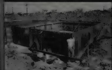
ORDINARY FOUNDATION JOB — Minimum alignment and bracing needed
