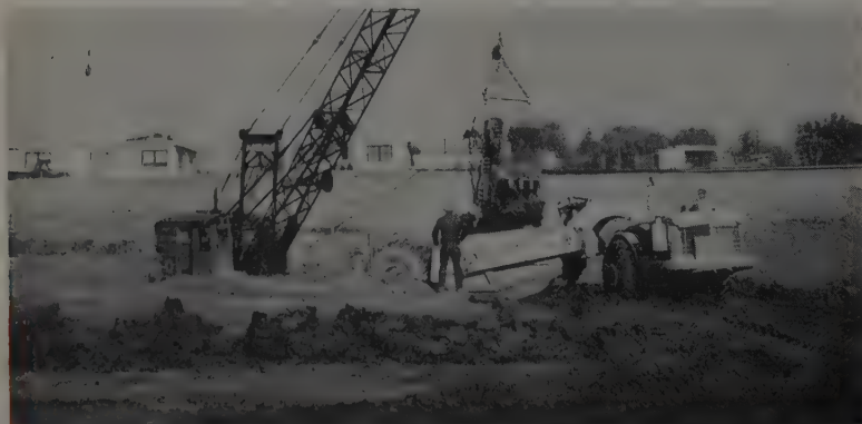
LAYER OF BLUE CLAY was encountered which was very difficult to excavate. Scrapers lost traction and tended to bog down. Draglines were used. Above, Northwest loads a Euclid scraper.
