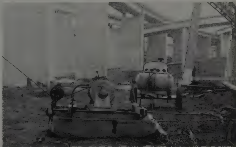
FORMS were lowered 125 ft. to ground with this sled-mounted Gardner-Denver hoist supplied by Ingersoll-Rand compressor. Concrete piers in background were constructed by slip-form method (Western Construction, Sept., 1956). Visible on opposite page is the famous "big cut".
