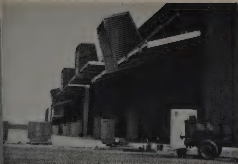
"BUBBLES" were framed with structural aluminum to reduce weight, but still represented an added load on the opening mechanism that had to meet exact specifications for opening time.
