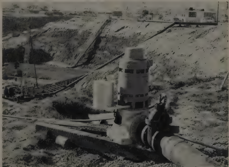
ELECTRIC-POWERED pump, one of six, runs continuously to keep deep excavation in the dry. The pumps removed water at rate of 16,000 gpm. during early phase of earthmoving operation.
