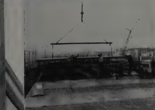
In carefully planned sequence of operations, prefabricated shoring towers were positioned, screw-jacked to required height. Deck form sections were then crane lifted into position.
