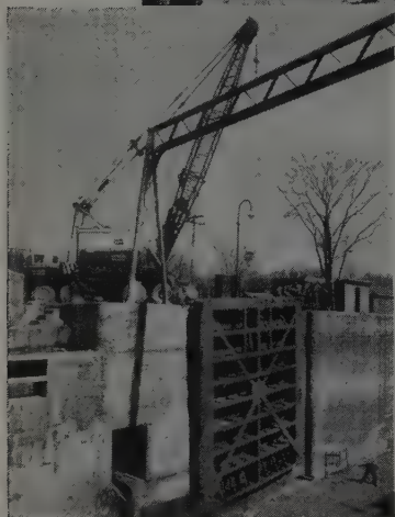
Powering Crane (boom)—140-GK Waukesha Gasoline , six cylinders, 4½-in. x 5½-in., 525 cu. in. displacement.
