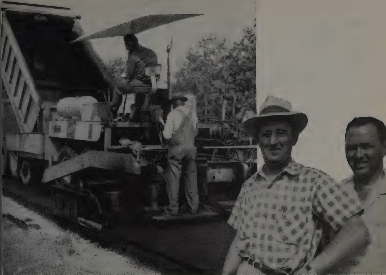
Paver resurfacing 15 miles of U. S. Highway 70 south of Huntington, Tennessee. Warren Brothers also used Blaw-Knox Wideners on their portion of the $1,200,000 project. Express Paver is laying upwards of 1,000 tons per day in a 1½ inch layer. Job Superintendent Bragg is shown at left and General Superintendent Duckworth at right.
