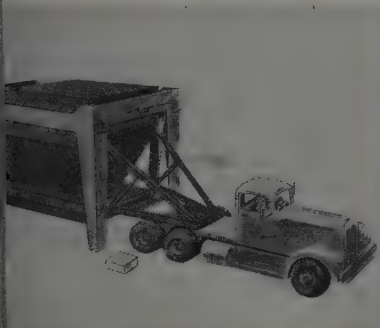
MOBILE HOIST-AND-BIN SECTION IS MOVING INTO PLACE.
