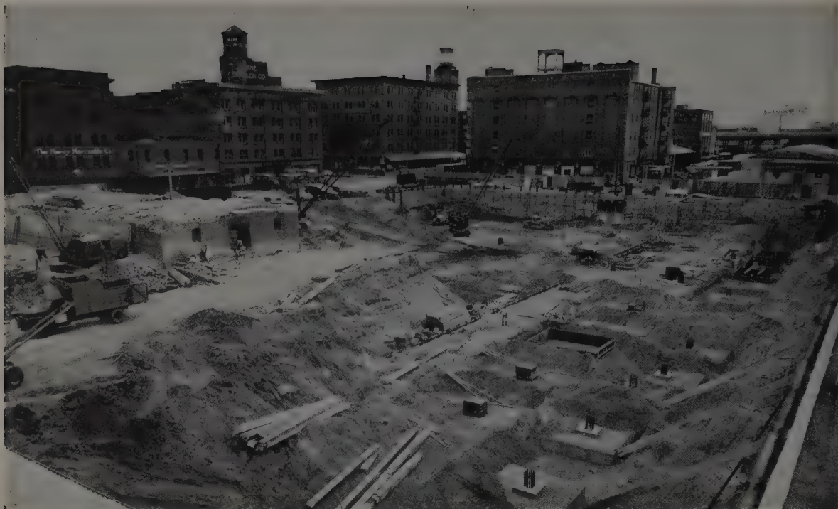
FOOTINGS for Denver Post Office Terminal Annex are protected by T-shaped wellpoint system. Placement was complicated by existing buildings.
