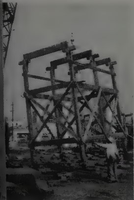
In carefully planned sequence of operations, prefabricated shoring towers were positioned, screw-jacked to required height. Deck form sections were then crane lifted into position.
