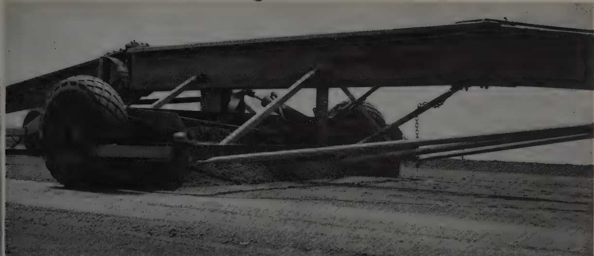
BUCKET of the plane shown running full as it picks off the top of a high spot and moves it forward to fill a depression.
