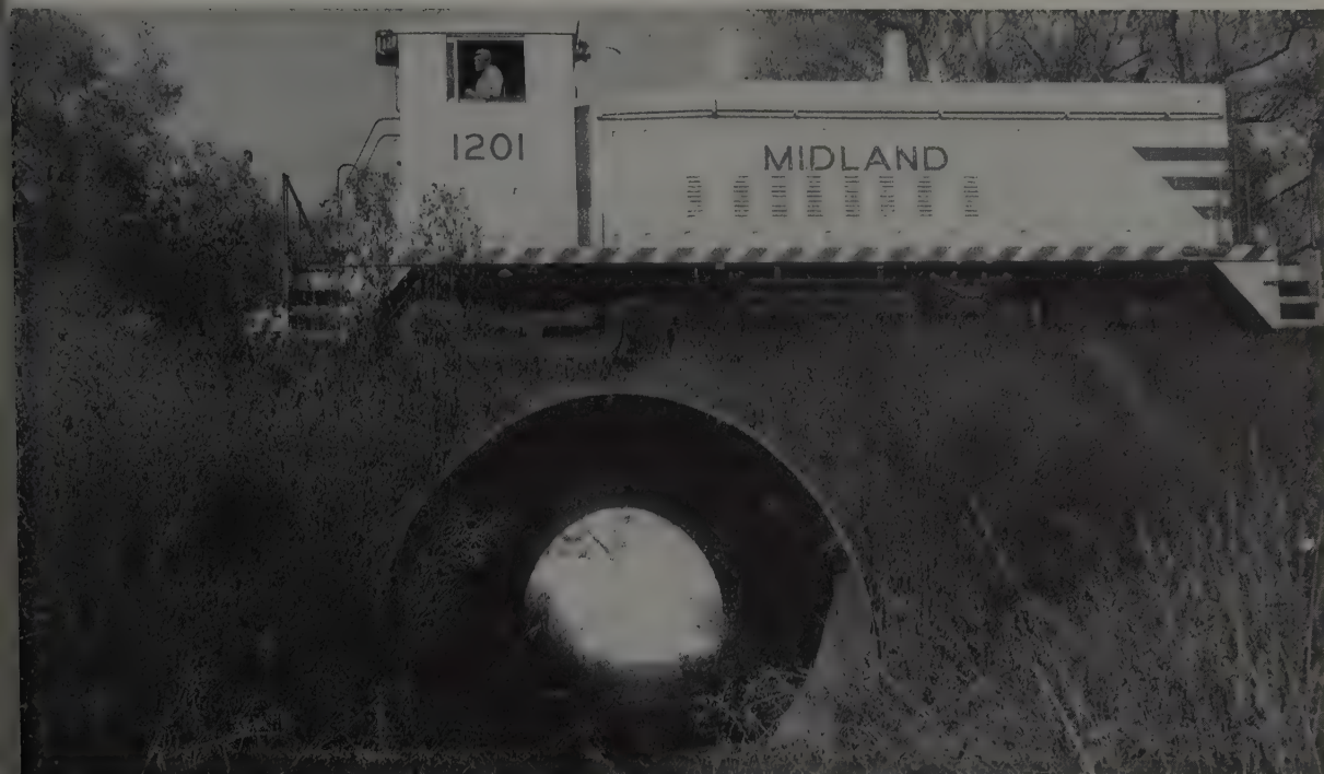
Under this industrial railroad to the Midland Collieries, Inc., is an Armco MULTI-PLATE Pipe, 102 inches in diameter. Many other Armco Drainage Structures are installed under this same line.
