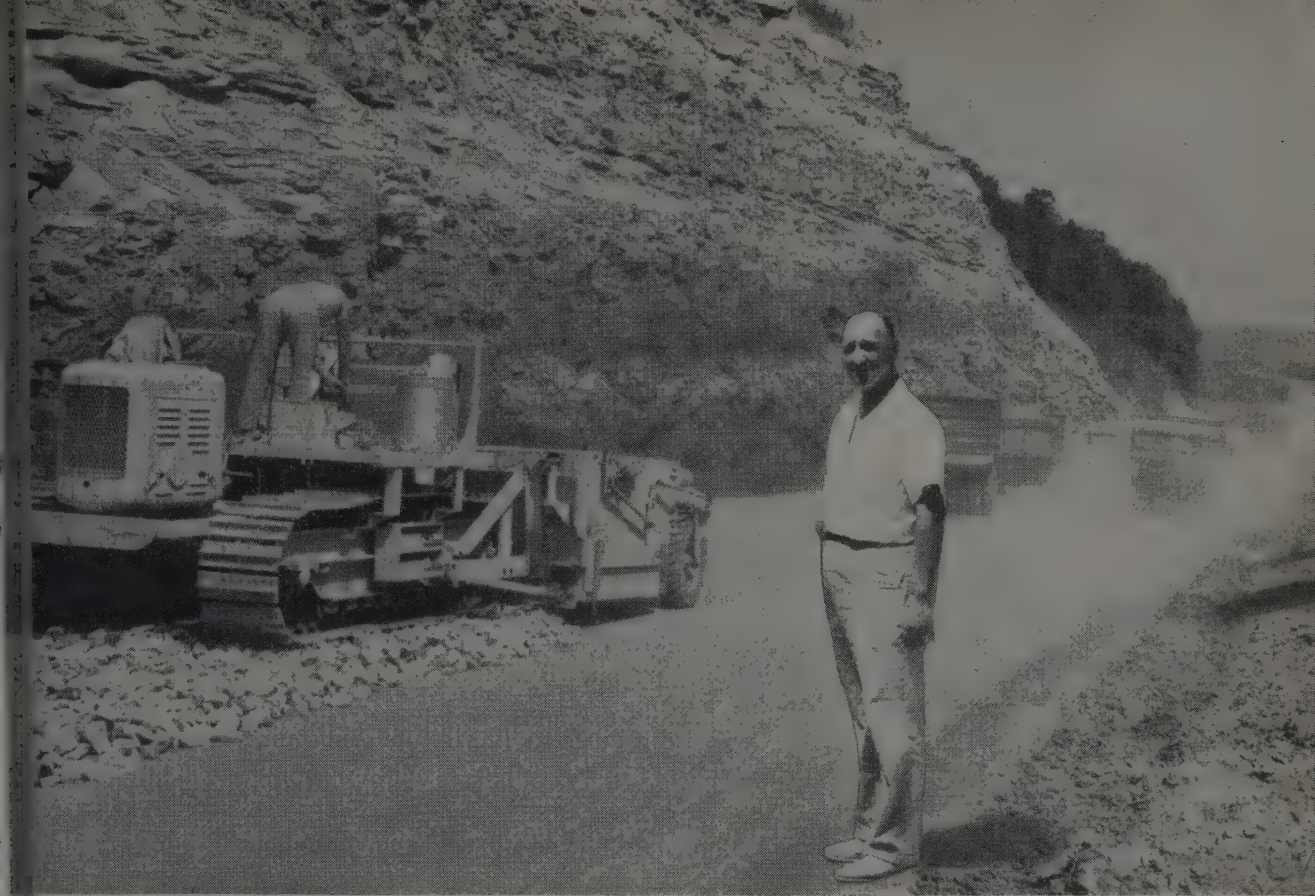
Dick Ellis watches Blaw-Knox Base Paver lay down six inch stone on a nine mile stretch of U. S. Route 27 between Stanford and Somerset, Kentucky.
