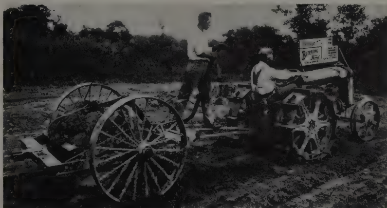
USE of agricultural-type tractors by contractors dates back almost 40 years as this picture of an early Fordson shows. On this tractor-pulled scraper rig, the sign on the tractor advertises "Hauling, grading, excavating, hoisting, snow plowing, etc., etc., etc."
