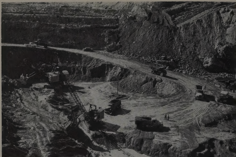
TAKING OUT 1,000,000 yd. of cut-off excavation to a depth of about 100 ft. below streambed. Material consisted of 40 ft. of alluvial sand and gravel underlain by a "mud-flow" of volcanic origin. The seal to bedrock consisted of a double row of steel sheet piling filled with concrete.
