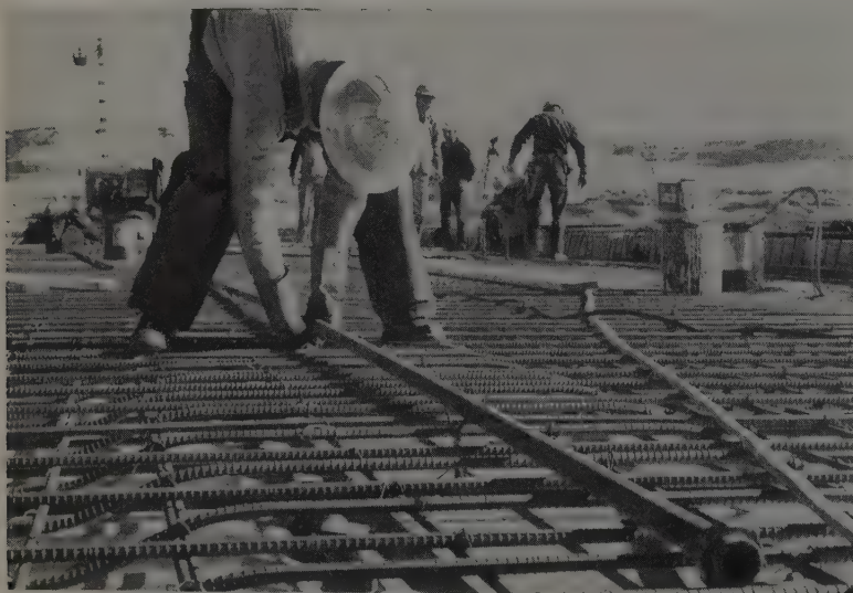
SCREED RAILS are being placed during concreting of deck. Rails are simply 1-in. pipe resting on finely adjustable screed chairs. Transit in background will be used to set rail at exact elevation. Bottom slab forms are corrugated steel, left in place permanently.
