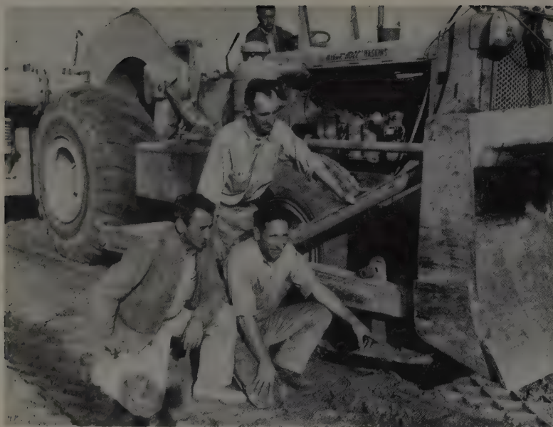
SKID SHOE is pointed out by Bernard Piombo, master mechanic (right), Melvin DeMattei, superintendent (left), and Arthur Haskins, owner (standing). The shoe is mounted behind the 'dozer blade of a DW-20 used to pull a pneumatic compactor. The shoe knocks off high spots as the rig moves over the fill.
