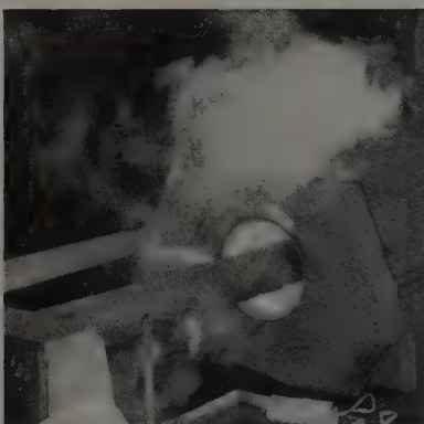
PIPE TAKES SHAPE... Molten iron in this rapidly rotating mold assumes its form as pipe—one of many manufacturing steps.
