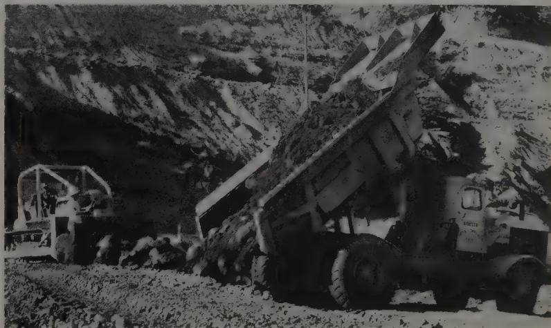
ON THE EMBANKMENT the agglomerate (volcanic) was placed in 15-in. layers. Work continued during one 2-month period when 47 in. of rain fell. Compaction was carried out with two 50-ton Southwest rubber-tired rollers. Placement hit a peak of 66,000 cu. yd. per day.
