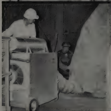
"ECONOMY" MODEL Oil fired. Electric motor powered. New "379" jet burner; some dependable controls. Up to 270,000 BTU capacity.
