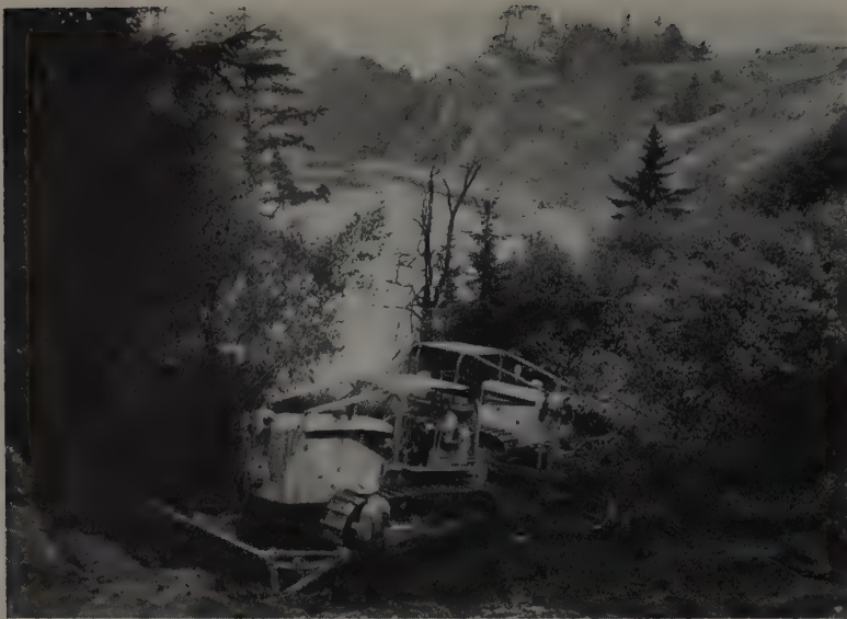
CANOPIES are normally required only when tractors are working in the clearing phase of a construction job, as on this Oregon highway project. Shown are two Caterpillar D8's.
