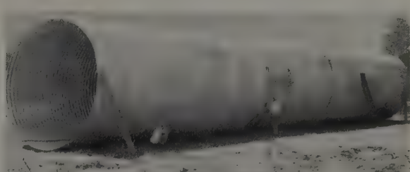
Here is another Armco MULTI-PLATE Pipe, 168 inches in diameter, in final stages of assembly, for installation under the same railroad line.
