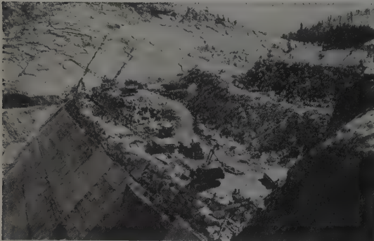
Courtright Dam: Brunner & Lay Rok-Bits used practically 100% in drilling out rock fill here, after some trial and error. Crawler type drills at Wishon Dam fitted with Brunner & Lay Rok-Bits also.
