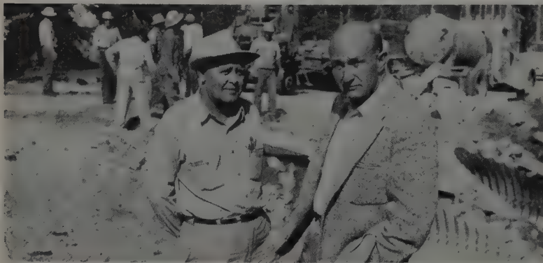
J. A. "JIM" SHELDON (right) is project manager, and Al Pearce is superintendent for $1,200,000 of high Sierra highway relocation in upper Yosemite National Park in California. Harms Bros. crews are in their second season at the 8,140-ft. Lake Tenaya job site on the project, and will require a third for completion. This and adjoining work will eliminate the last 21 mi. of the old Tioga Pass mine road built in 1883.
