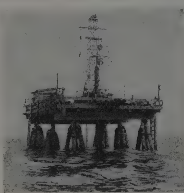
BORING SETUP—NEW YORK HARBOR
