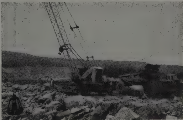
An O. & G. truck crane places a huge boulder in place on the face of the dam. Heavy-duty jobs like this and the solid bed rock conditions required the most durable equipment available.
