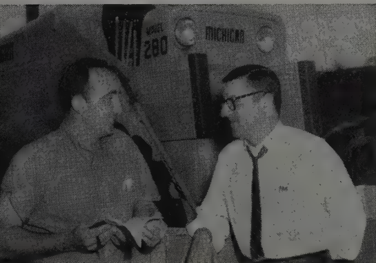
George Oneglia, Vice President of Building Materials, Inc., and George Allis of C.I.T. discuss progress of the job which has a completion target date of spring 1960. Mr. Oneglia says: "It's a big job requiring large capital resources. That's one reason why we have found C.I.T. Corporation to be extremely helpful."
