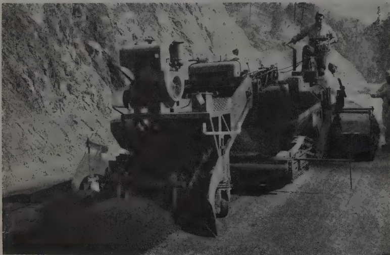
TO REDUCE delays at the paver and permit uninterrupted operations, the trucks dumped the mix in a windrow where it was picked up by this Ko-Cal loader.
