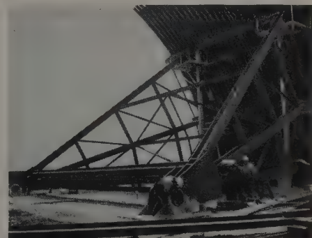
Each radial gate was assembled at the plant, match marked, then disassembled and shipped on gondola cars to the site—four cars to a gate!
