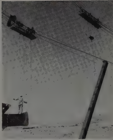
BOTH CABLEWAYS are used at once to set 162-ft. long vertical column. Process is described at right.
