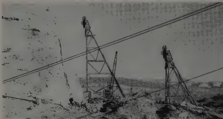
CABLEWAY TOWERS for placing concrete in the dam are now complete and 4-in. diameter lock coil guts have been strung between them. Lines cutting diagonally across pictures are tie-back cables used during bridge construction. At left is landmark called "Beehive Rock".
