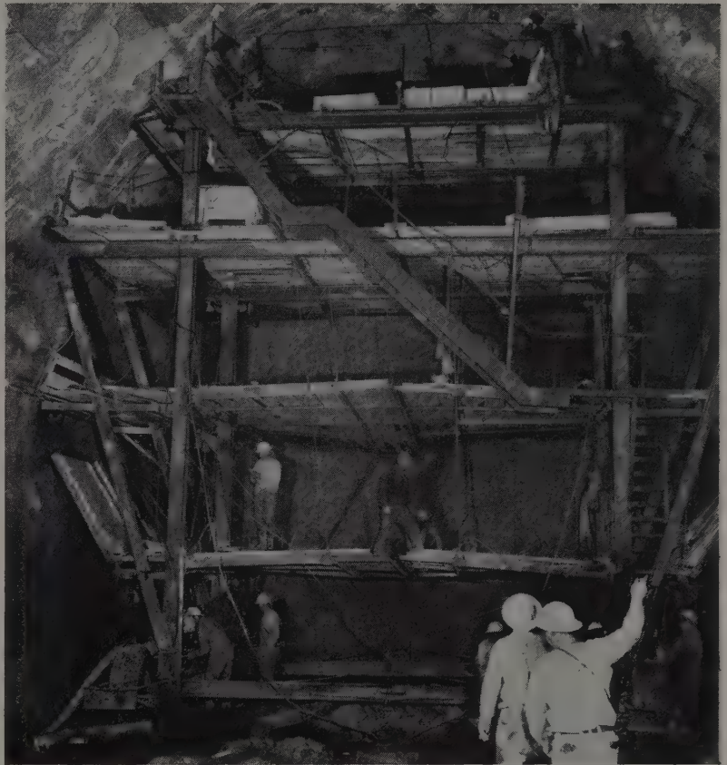
TUNNEL JUMBO used by Mountain States Construction Co. to drive the right diversion tunnel was mounted on pneumatic tires and featured platforms which raised to pass mucking machines.
