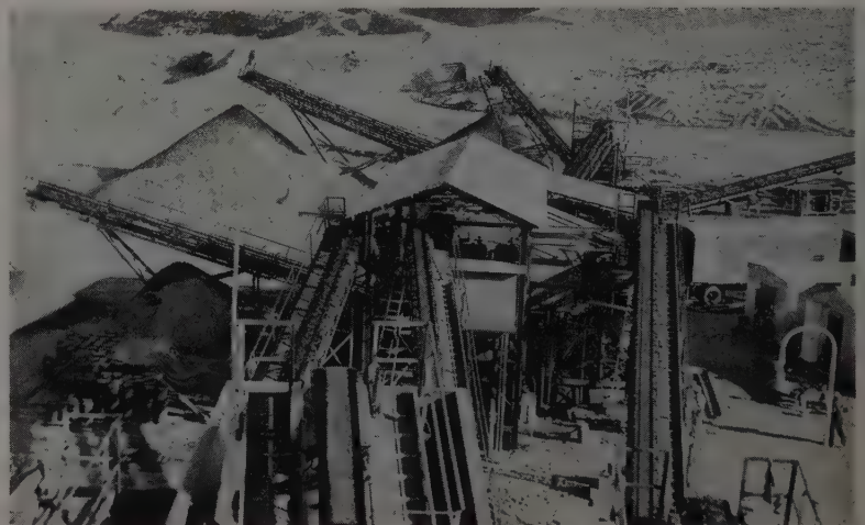
HEAVY MEDIA separation plant, equipped with Barber-Greene conveyors, isolates heavy aggregate for use in exterior concrete. Process is rare for a construction project.
