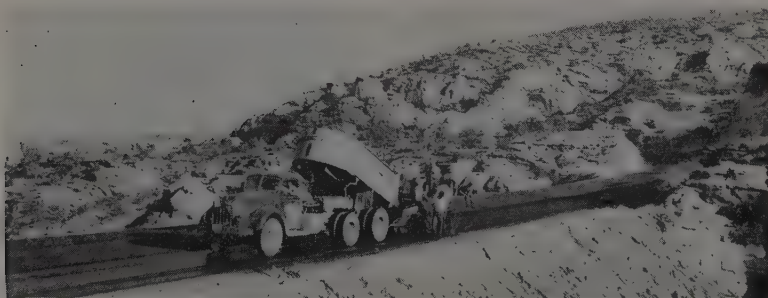
ACCESS ROADS across desolate desert were first order of business. Shown is a Barber-Greene paver working on the Bitter Springs road leading to the job from the south.
