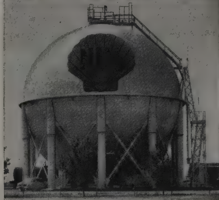
Ammonia. 64 ft dia, 55 lb working pressure
