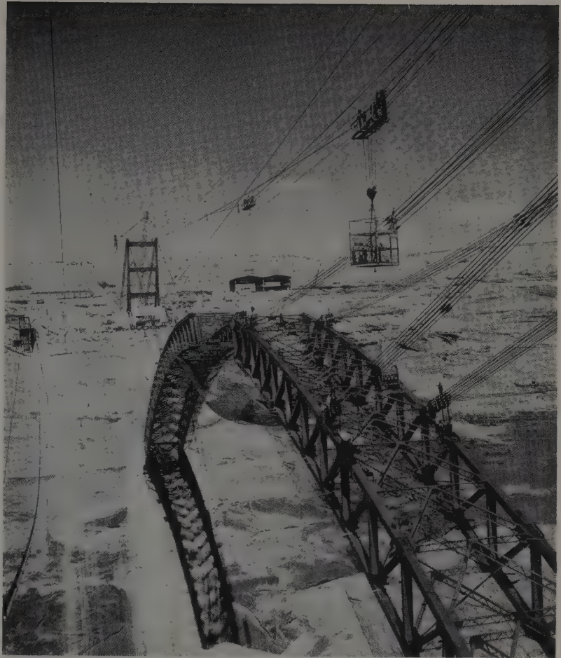
TIE-BACK CABLES hold arch in position as closure point is neared. Cage on auxiliary cableway is used to carry men and tools. Carriage of main cableway is visible above highest point of arch. Faintly visible in background is main cableway tower, luffed to right.
