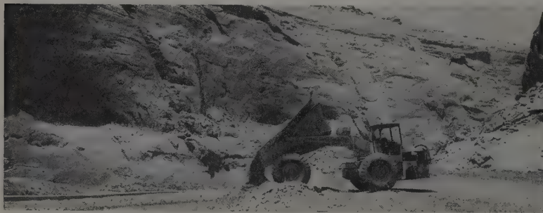
SUBCONTRACTORS have large machines at work also. Here is a LeTourneau-Westinghouse Model D rear dump at work for Frazier-Davis, subcontractor for the underground work.
