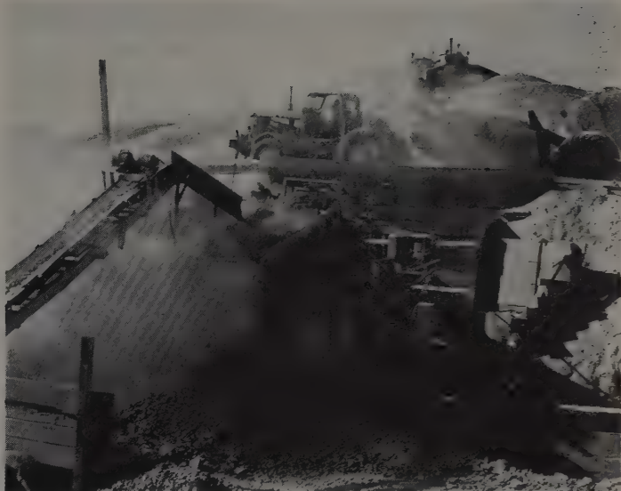
Dozers and scrapers charge the dump hopper for the twin KOLMANs.
