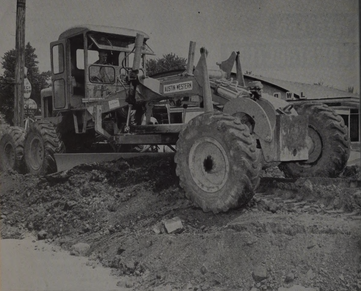
Vernon (Stub) Faber doing a rough grading operation on a highway widening project inside the city limits of Milwaukee, Wis. The machine is an Austin-Western Super 99 with 6-wheel drive and 6-wheel steer.
