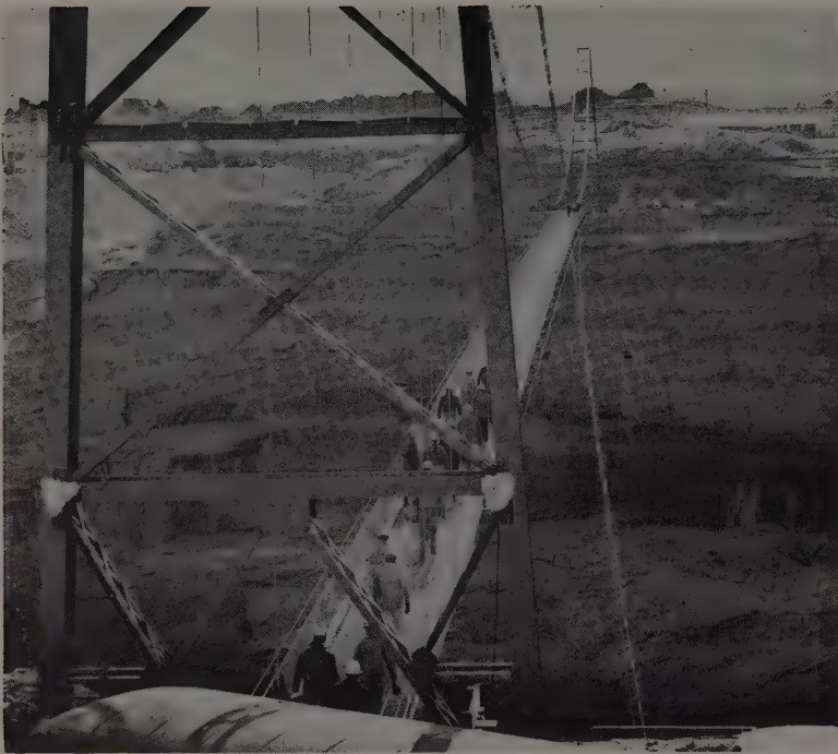
SUSPENSION FOOTBRIDGE has mesh walkway to minimize wind resistance. Newcomers find it disconcerting to look between their shoes and see the river 700 ft. below.
