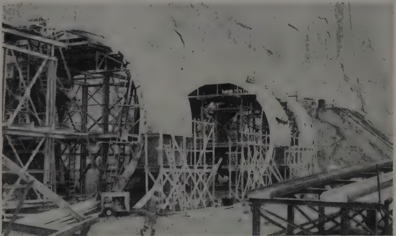
TUNNEL FORMS , made by Blaw-Knox, were used to line diversion tunnels. All steel, they were carried on a rail-mounted collapsible gantry. Tunnels were over 45 ft. in diameter.
