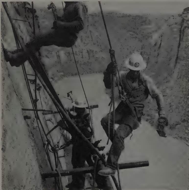
EXCAVATION of the skewbacks for the Colorado River Bridge was a difficult task. Men are shown with quarry bars on which drilling equipment was mounted. Small charges were used to avoid disturbing adjacent rock. Hazardous operation was completed without mishaps.
