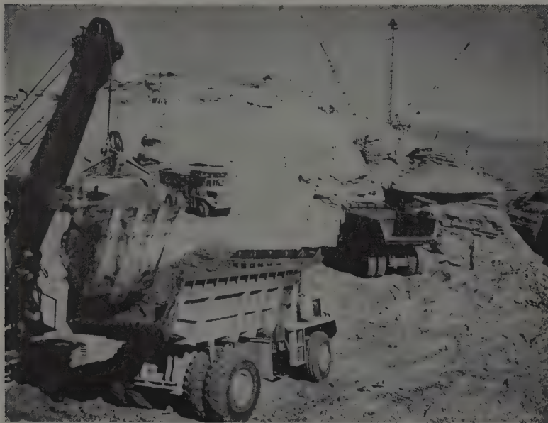
LIMA SHOVEL loads a fleet of I-H Payhaulers during excavation of right keyway. The Payhaulers were kept on this job until the haul road became an impossible 23%.
