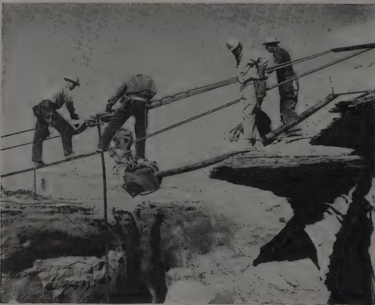
WORKING 700 ft. above the river, workmen make adjustments on pulling rigs before hauling the largest lock-coil cable ever made 2,000 ft. across canyon. Note "jewel" on cable end. Cable can carry 50-ton loads during concrete placement for the dam.
